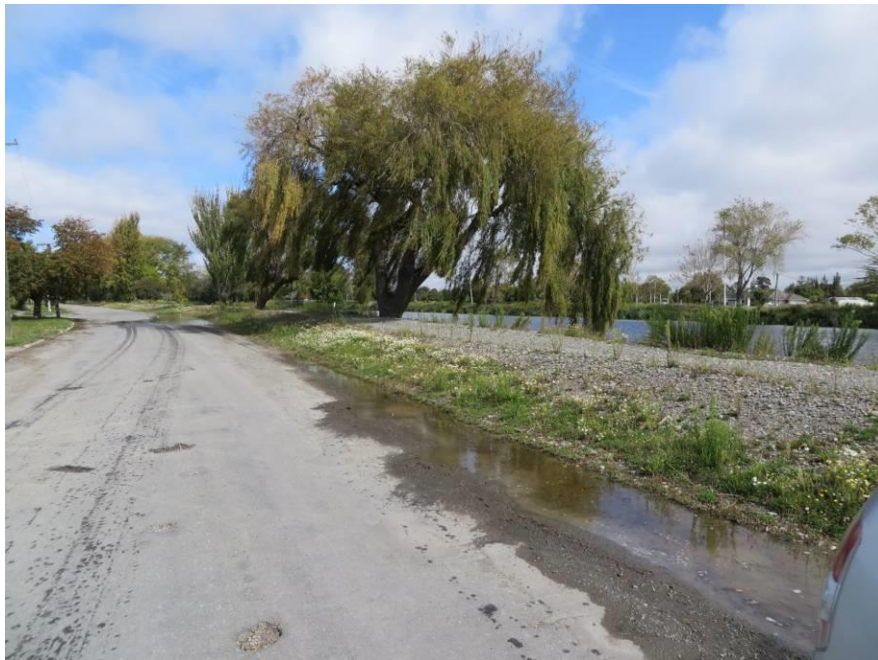
Figure 2-5 Stopbank along the Avon River on Avonside Drive (-43.503590°, 172.683632°).
