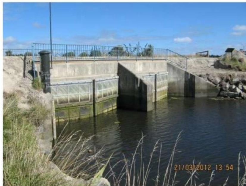
Figure 2-4 Tide-gates on the Styx River at Brooklands (Christchurch City Council, 2012).
