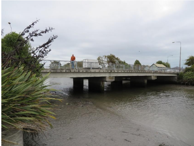
Figure 6-20 Rutherford Street Bridge on 20 March 2014.
