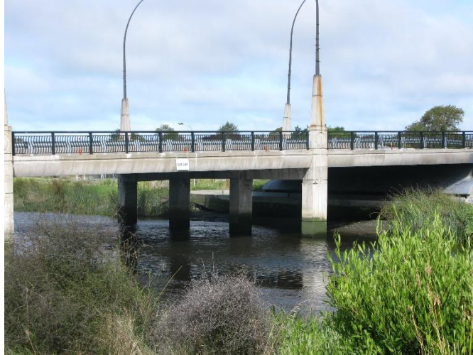
Figure 6-14 Anzac Drive Bridge on 19 April 2014.
