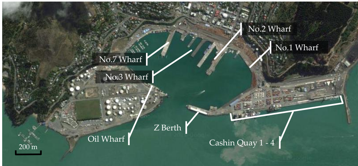
Figure 6-23 Layout of Lyttelton Port of Christchurch highlighting the main wharves (Ragued et al. 2014).
