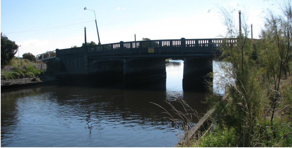
Figure 6-11 Pages Road Bridge on 19 March 2014.
