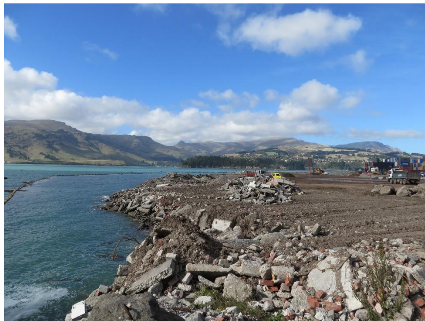
Figure 6-26 Te Awaparahi Bay land reclamation area on 21 March, 2014.
