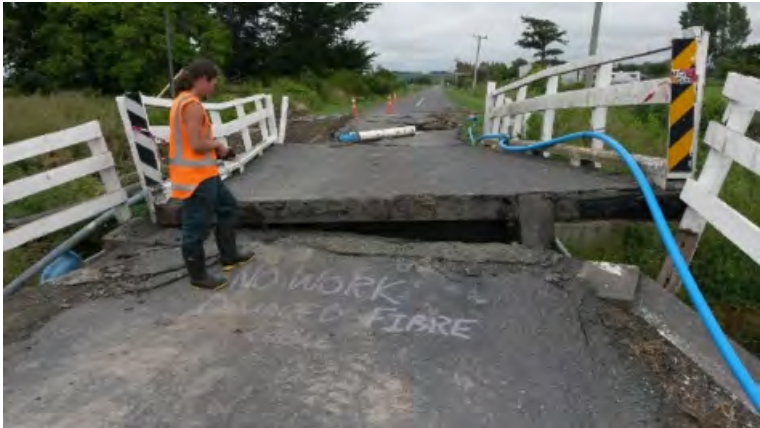
Figure 6.67: Eastern side of Lyell Creek Bridge [-42.3892, 173.6773]. Photo facing west.
