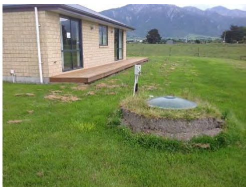
Figure 4.106: Floation of septic tank at SE corner of house on Mt Fyffe Road (8 Dec 2016, S42.3876, E173.6621, facing N).
