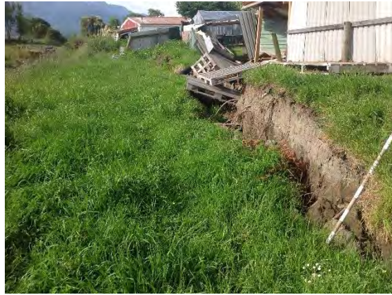
Figure 4.111: Large vertical offset (50 cm) associated with the ground movement north of Gillings Lane (– date to be added in V2.0 of report, S42.3841, E173.6784).
