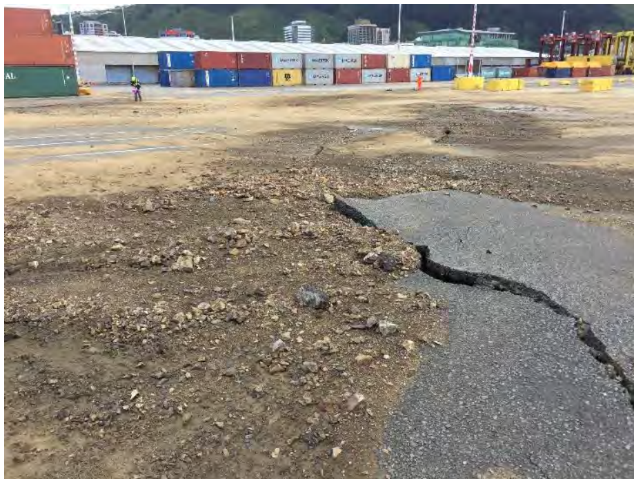
Figure 5.34: Widespread liquefaction of gravelly end-dumped quarry rock reclamation in container stacking area inland of Thorndon Wharf (S41.276608° E174.786309°, taken on 21NOV16)
