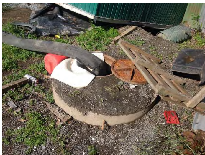
Figure 4.113: Floatation of manhole on Beach Road near to Lyell Creek (– date to be added in V2.0 of report, S42.3848, E173.6783).
