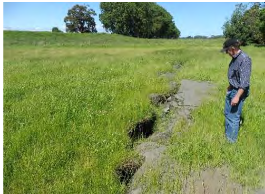
Figure 4.50: Cracks and ejecta on the foundation soil between the secondary stopbank and the river (5 Dec 2016, S41.440967, E173.980122, facing NE).
