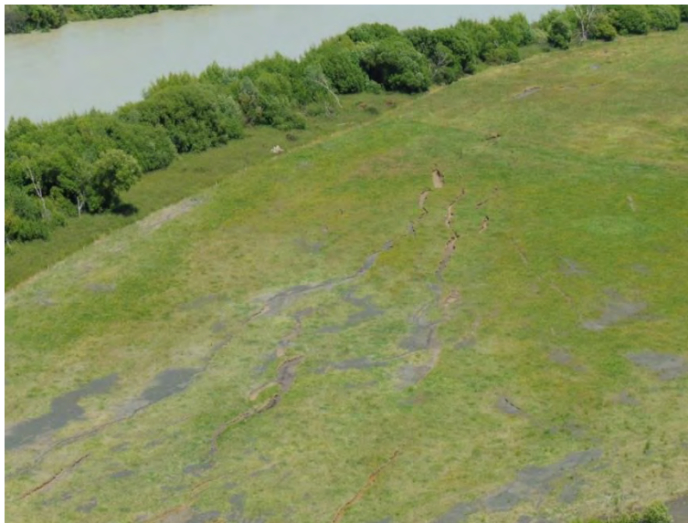
Figure 4.55: Lateral spreading and liquefaction ejecta on the eastern banks of the Lower Wairau River (18 Nov 2016, S41.4854, E174.0160, taken facing W).
