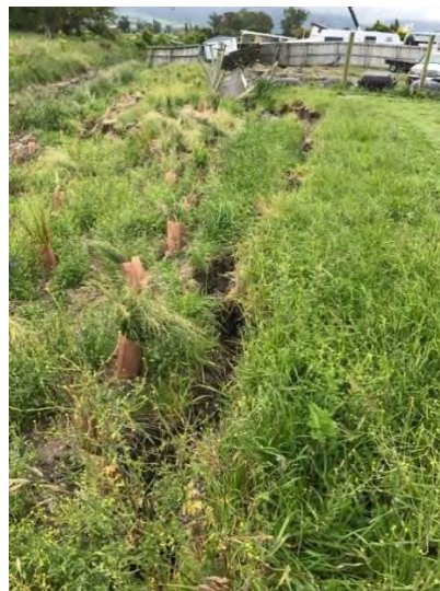
Figure 4.120: Lateral displacements at 105 Beach Road. Note: Cracks are associated with vertical offsets and blocks have rotated away from the river (i.e., slumped) (9 Dec 2016, S42.3902, E173.6777).
