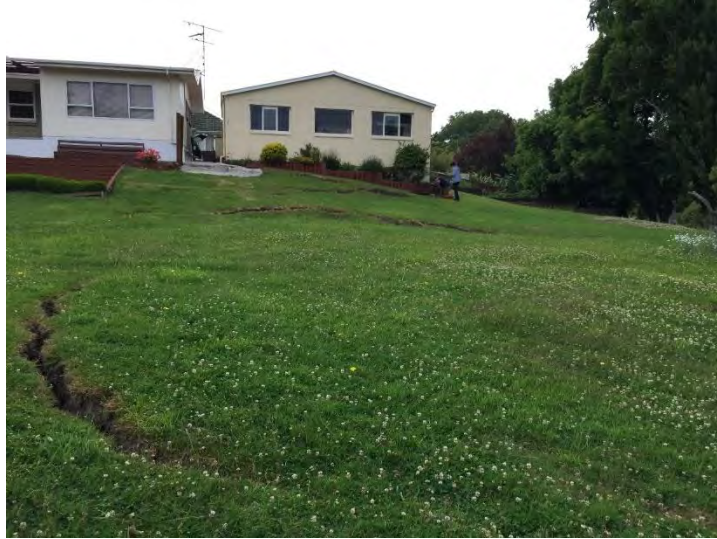
Figure 4.25: System of lateral spreading/slumping cracks at Elizabeth Street (7 Dec 2016, S41.5089, E173.9636, facing E).
