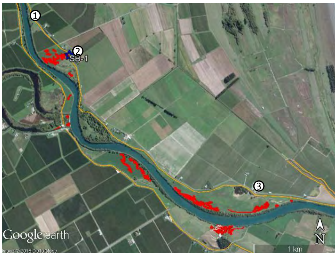
Figure 4.53: Summary of liquefaction induced damage along the banks of the Lower Wairau River, with red areas indicating cracking and ejecta locations. Stopbank damage is shown by the red symbols in this figure. (Approx. centre of image: S41.4799, E174.0006).
