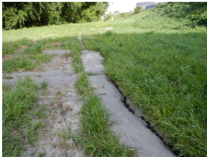
Figure 4.17: Crack parallel to Opaoa River surrounded by grey ejecta to the north of the Park Terrace properties (7 Dec 2016, S41.5121, E173.9651, facing E).
