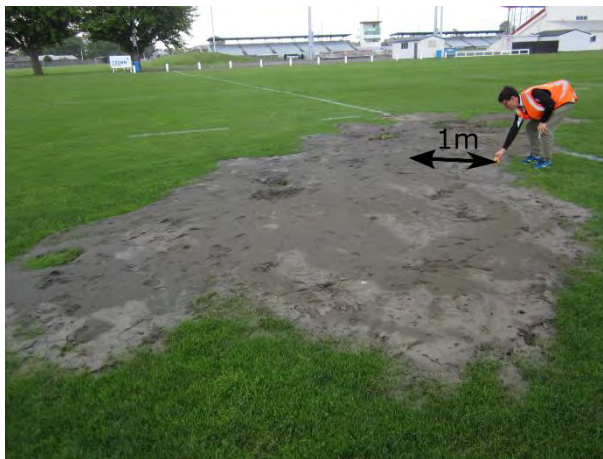
Figure 4.12: Largest liquefaction feature at Lansdowne Park (17 Nov 2016, S41.4996, E173.959, facing W).
