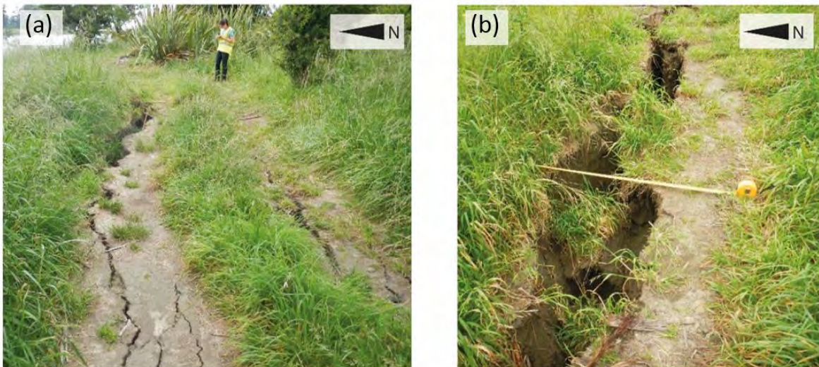
Figure 4.37: Cracking of the southern bank of the Wairau Diversion: (a) 17 Nov 2016, S41.4406, E174.0215; (b) 17 Nov 2016, S41.4406, E174.0215.
