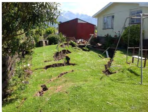
Figure 4.110: Lateral displacements (approx. 1.5 m in total) caused a loss of support at the NW corner of a house on Beach Road, causing cracking in the brick wall (date to be added in V2.0 of report, S42.3823, E173.6800).
