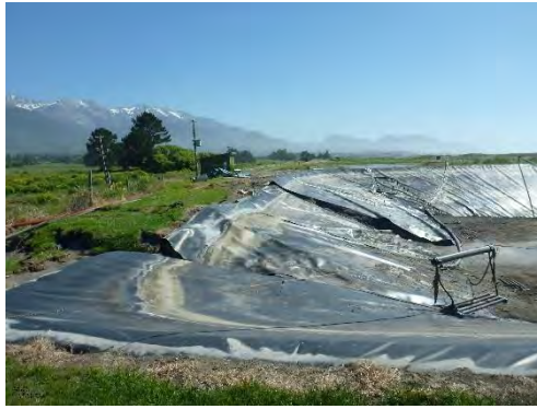
Figure 4.129: West edge of KK-OPS. Large differential settlements of the crest are visible (– date to be added in V2.0 of report, S42.3668, E173.6865, facing N).
