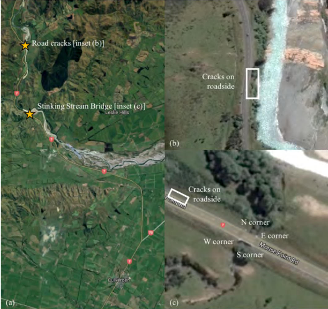
Figure 6.33: Highway 7 area: (a) Site locations for areas of interest; (b) Road crack site layout [-42.6310, 172.7718]; (c) Stinking Stream Bridge site layout [-42.6724, 172.7748].
