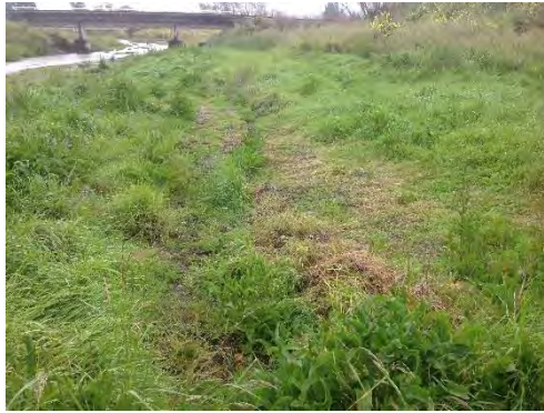
Figure 4.126: Lateral spreading in the bank on south edge of oxidation ponds (– date to be added in V2.0 of report,, S42.3672, E173.6866, facing W.)
