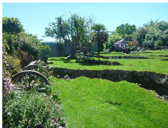
Figure 4.118: Lateral displacement with vertical offsets close to Hawthorne Road Bridge (– date to be added in V2.0 of report, S42.3885, E173.6776).
