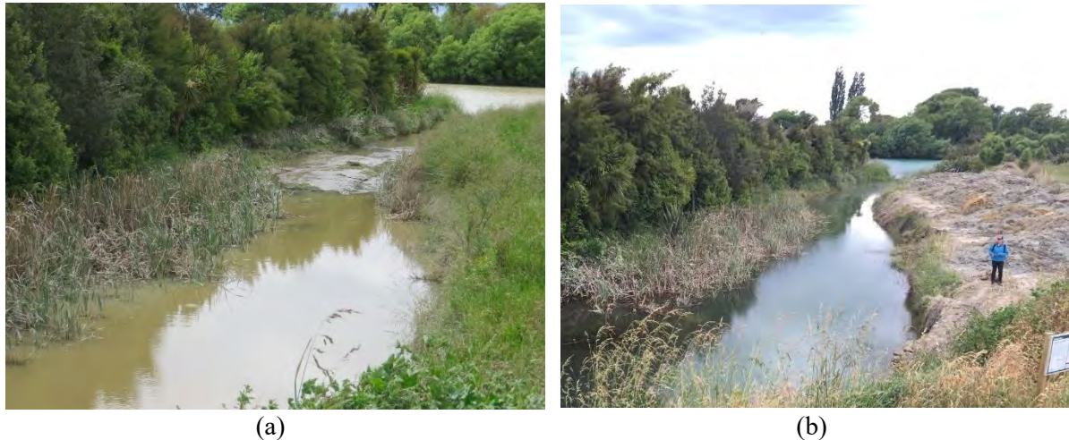
Figure 4.81: a) Ejected sand evident in the drain channel (14 Nov 2016). b) Pile of excavated ejecta from the drain channel (6 Dec 2016, S41.4754, E173.9854, facing E).
