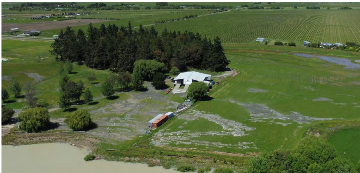
Figure 4.67: Aerial view of liquefaction manifestation at the Blenheim Rowing Club looking south (18 Nov 2016, approx. centre of image: S41.4890, E174.0094, Marlborough Regional Council, 2016).
