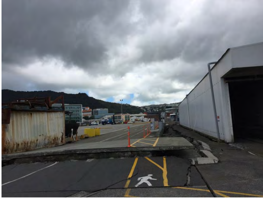
Figure 5.42: Looking North along bulkhead of King's Wharf. Approximately 560 mm of ground settlement relative to deck at southeast corner of King's Wharf. The west wall of the Cold Store shed is visible to the right of the photograph. (S41.281142° W174.784444°, taken at 1416 hrs on 21NOV16)
