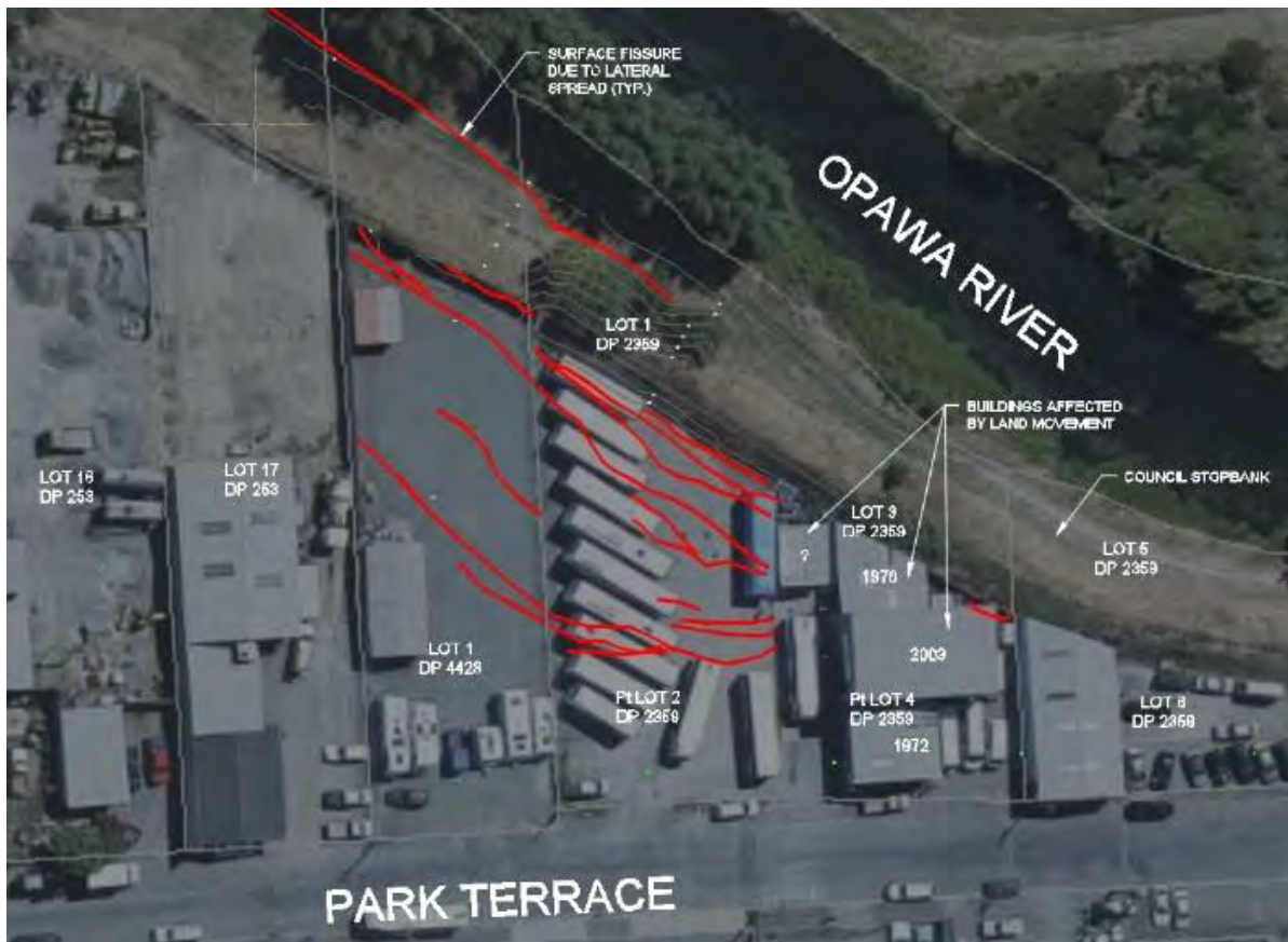
Figure 4.16: Summary of damage at the Park Terrace site. Dashed line indicates location of the historic stopbank (approx. centre of image: S41.5122, E173.9649).
