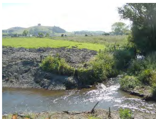
Figure 4.123: Recent earthworks on west side of Lyell Creek, opposite 87 Beach Road. (9 December 2016, S42.3922, E173.6777).
