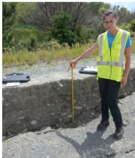
Figure 4.33: Maximum vertical settlements of 50 cm were observed along the cracks in the northern stopbank (17 Nov 2016, S41.4386, E174.0216, facing N)
