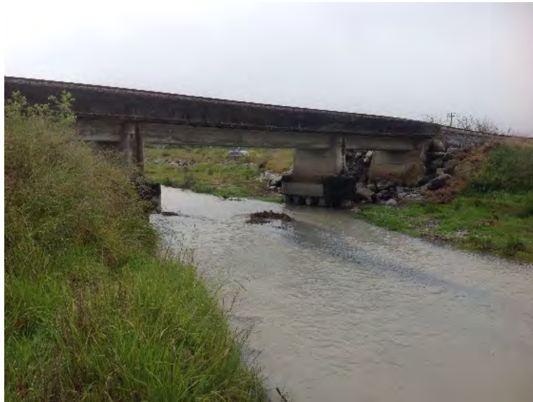
Figure 6.69: Middle Creek Railway Bridge (facing northwest) [-42.3672, 173.6862].
