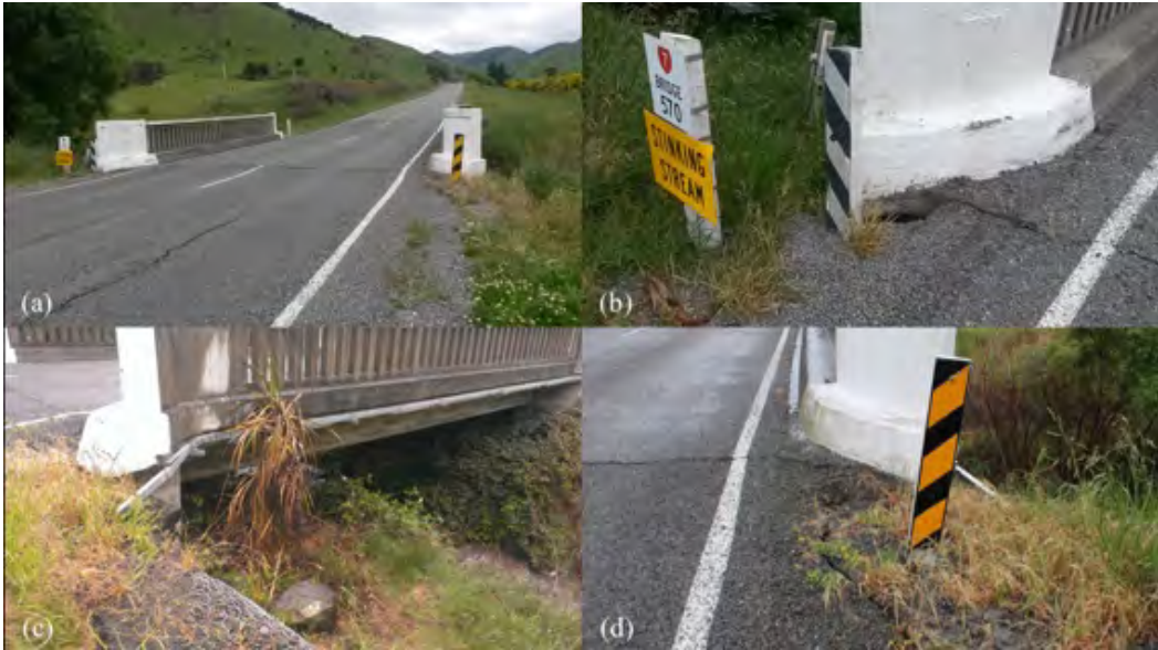
Figure 6.34: Stinking Stream Bridge [-42.6724, 172.7748]: (a) Looking north on 14 November; (b) Southern corner on 14 November; (c) and (d) Eastern corner on 17 November.
