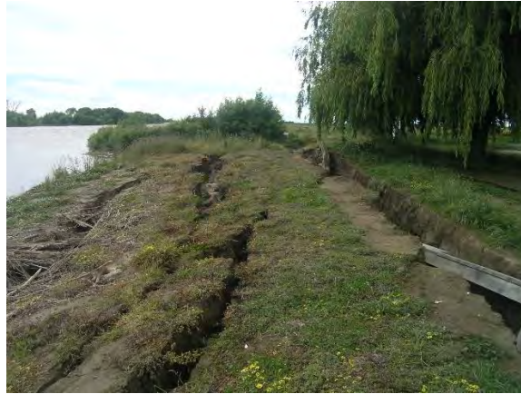
Figure 4.70: Lateral spreading at the west end of the rowing club site. (17 Nov 2016, S41.4881, E174.0101, facing E).
