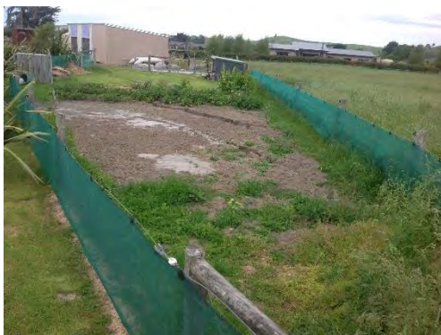
Figure 4.95: Liquefaction in a vegetable patch on Mt Fyffe Road. Note the ejecta issued from ground cracks (-date to be added in V2.0 of report, S42.3813, E173.6622, facing S).
