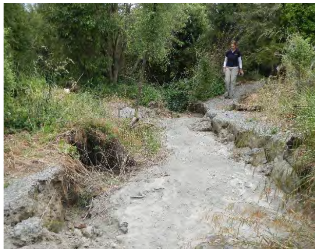
Figure 4.79: Lateral spread crack approximately 2 m wide filled with fine grey ejecta (6 Dec 2016, S41.4761, E173.9860, facing NE).
