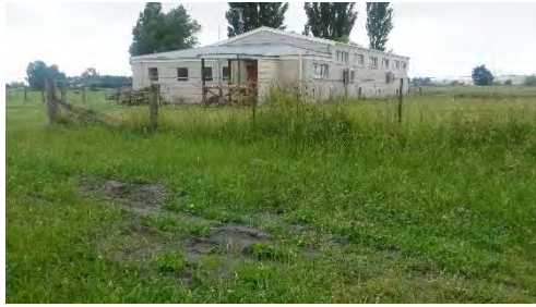
Figure 4.93: Liquefaction ejecta on Schoolhouse Road where sample SR-1 was taken (-9 Dec 2016, S42.3681, E173.6496, facing SE).
