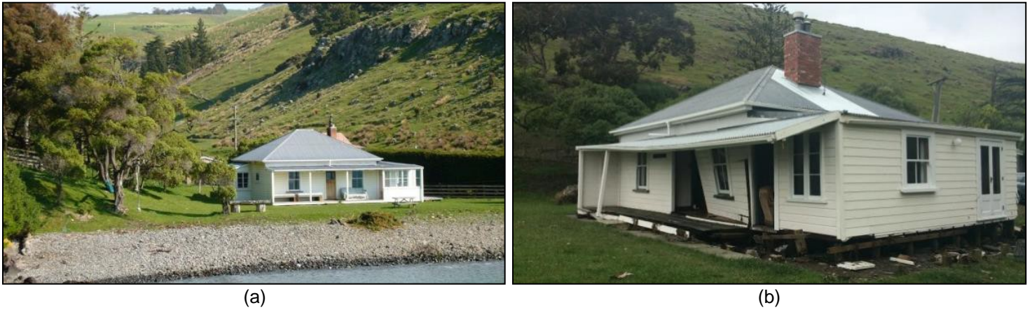
Figure 9. Before (a) and after (b) pictures of a cottage damaged by the tsunami at the north end of Little Pigeon Bay (photos: Stuff website 13 ). The deck of the house was detached and deposited on the beach.
