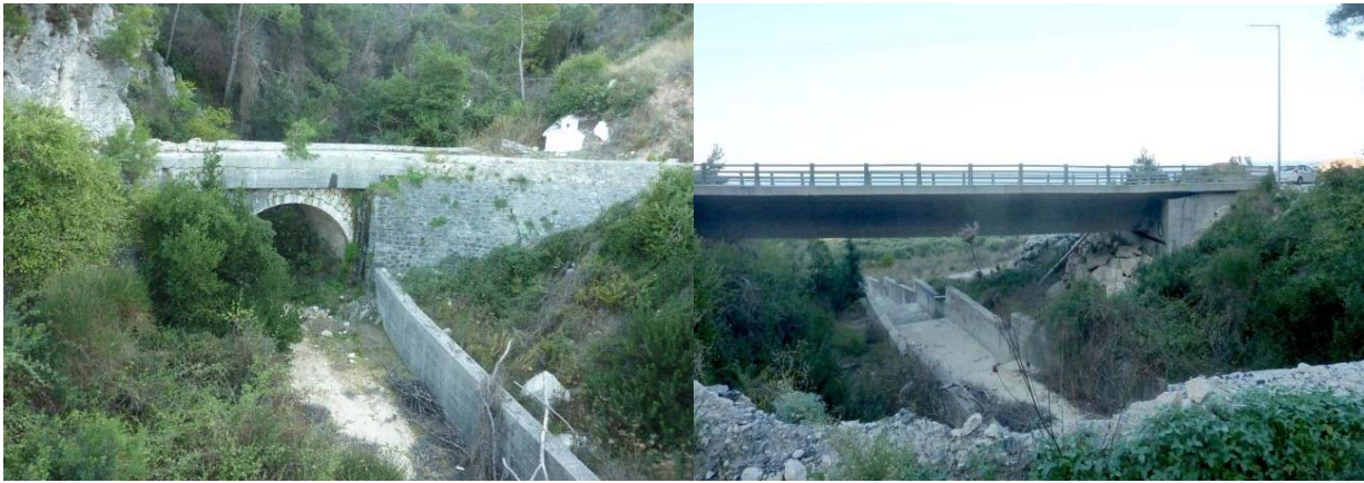
Figure 7.100. Stone and reinforced concrete bridges along the roadway network of Samos
