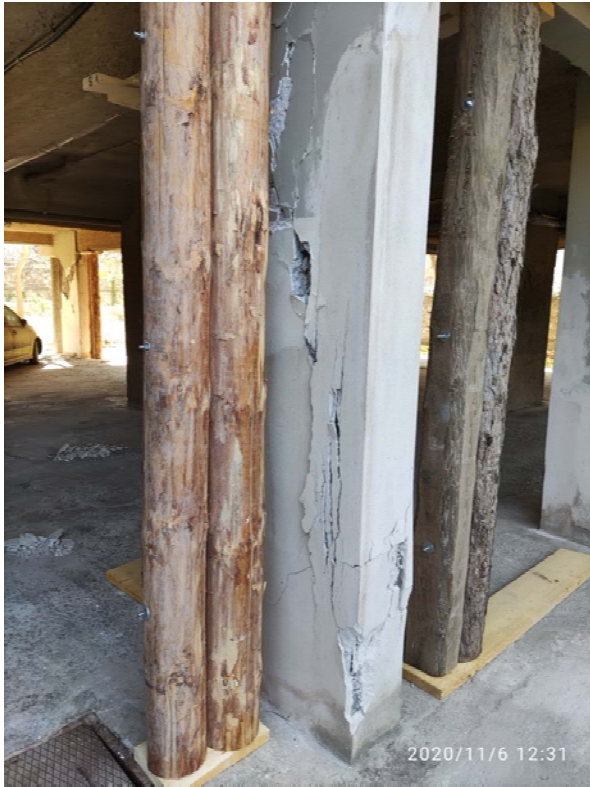
Figure 7.59. Soft-story failure of a five-story residential building in Karlovasi.
