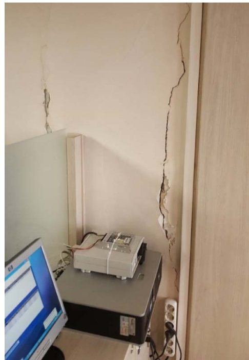
Figure 7.23. İzmir Commerce Building. Observed damages from inside the structure
