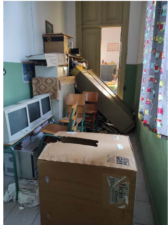
Figure 7.77. Primary school at Kontakeika: Major shear failure at the masonry walls, delamination of coating and overturning of equipment.
