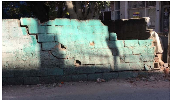
Figure 5.33. No signs of soil liquefaction. Tilted and partially collapsed very poor safety walls (38°27'24.6"N 27°10'53.1"E/ 11:10/ 04.11.2020).
