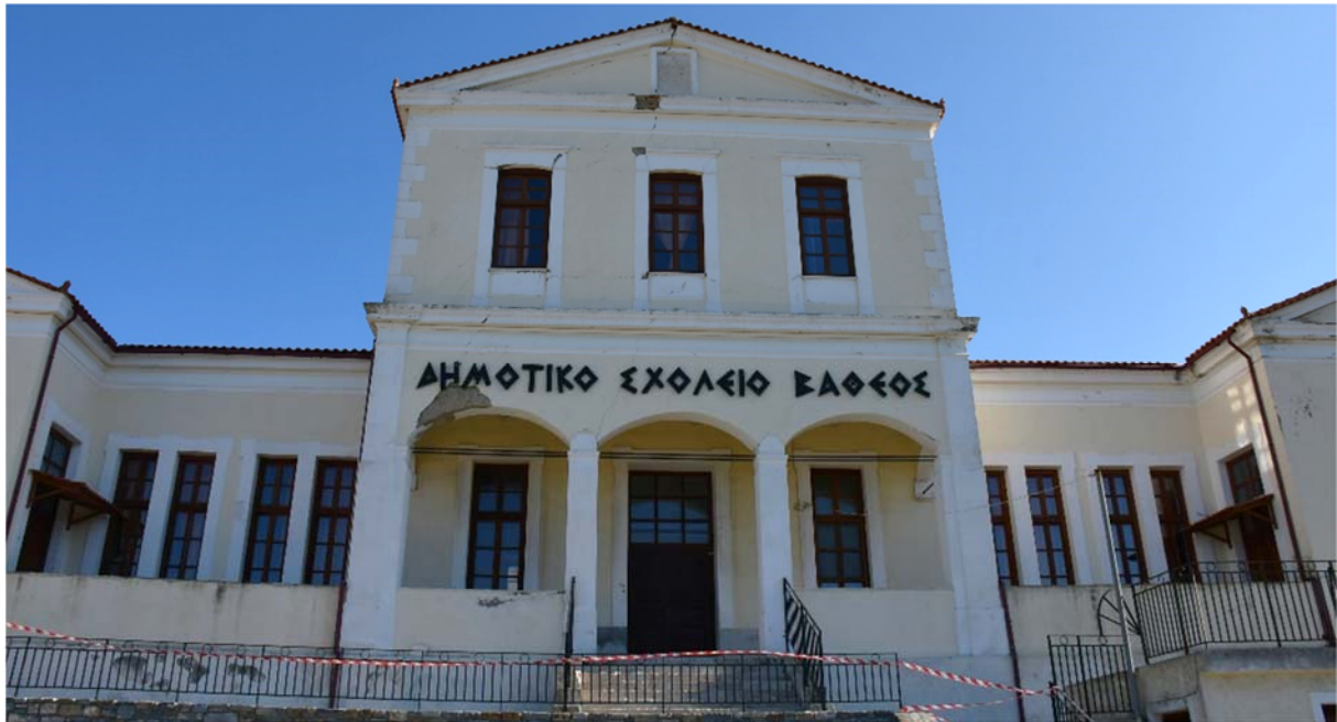
Figure 7.75. Damage to the primary school at Vathy.
