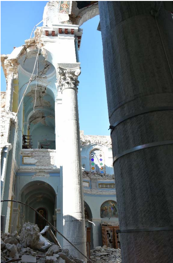
Figure 7.83. Poor construction of the dome-and-arches system.
