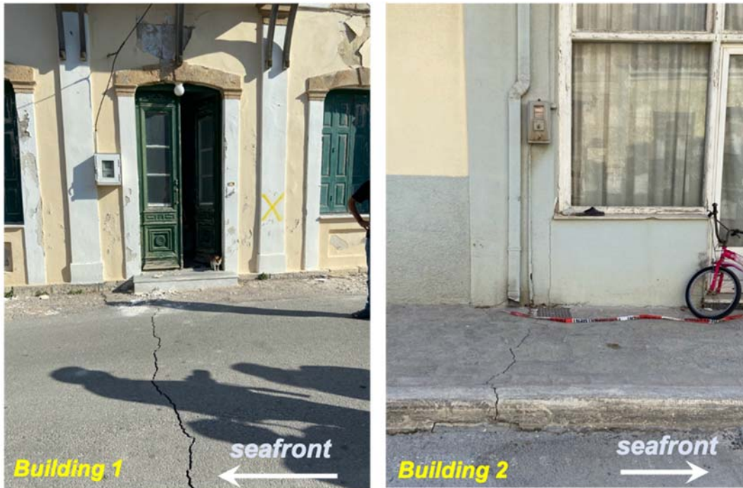
Figure 5.20. Buildings likely affected by lateral spreading towards the seafrent in the neighborhood of Vyrsopepsia in Karlovasi (left: 37^{\circ}47'57.6''N 26^{\circ}42'12.5''E and right: 37^{\circ}47'59.3''N 26^{\circ}42'20.0''E ) [photos taken by the HAEE reconnaissance team]
