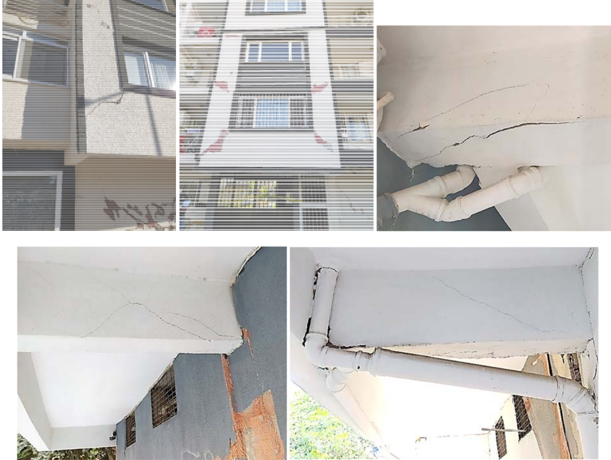
Figure 7.14. Overhang damages
