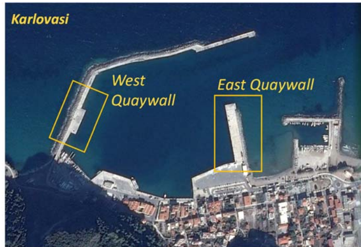
Figure 5.46. Satellite view of east and west quay walls of Karlovasi port.
