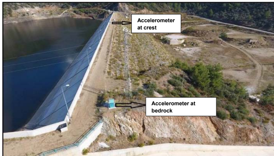
Figure 6.2. Accelerometer configuration on Derince Dam, Muğla (modified from Ateş et al. 2019)
