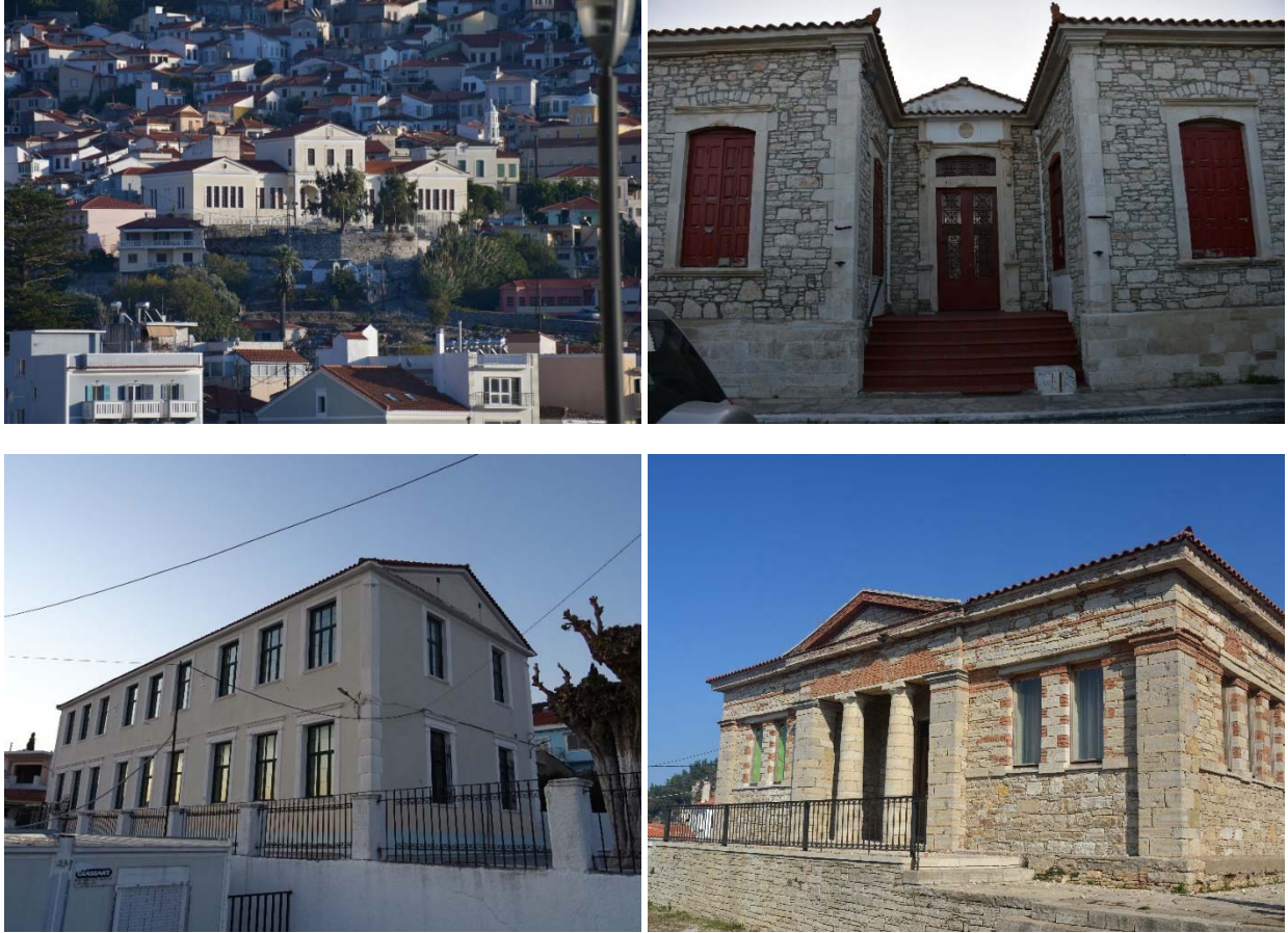
Figure 7.74. School buildings at Vathy. Limited damage was observed.
