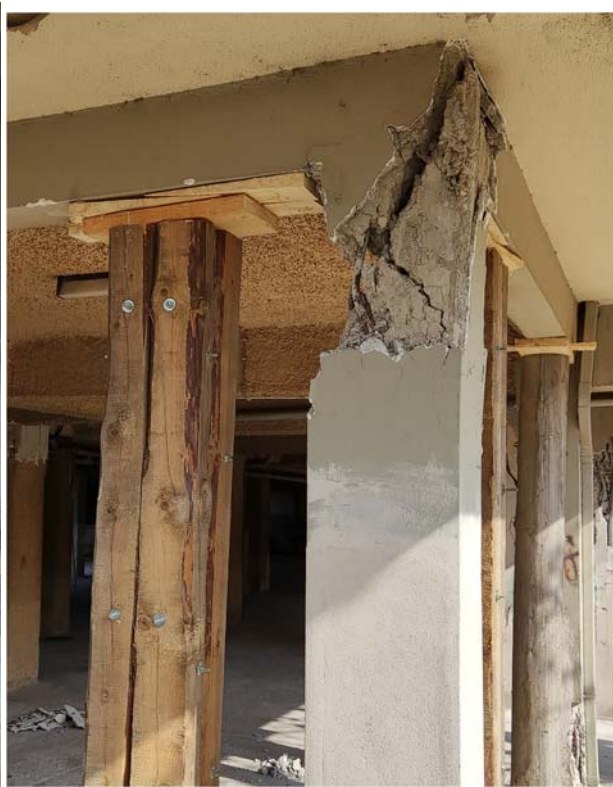
Figure 7.59. Soft-story failure of a five-story residential building in Karlovasi.
