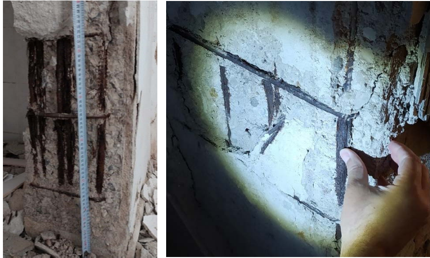
Figure 7.16. Corrosion damages
