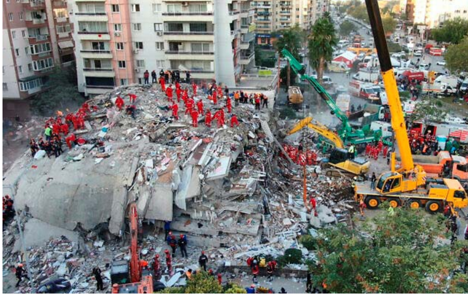
Figure 4.15. Doganlar residential building, fully collapsed after the event (courtesy of Ali Aksoyer)
