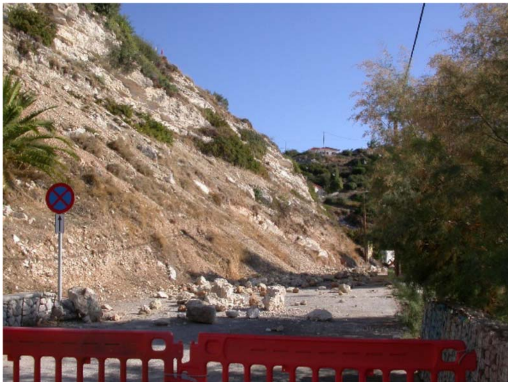
Figure 5.28. Limestone segments falls to a provincial road in Remataki region (photo reported in Lekkas et al. 2020).
