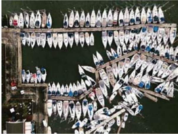
Figure 2.27. Floating Piers in Teos Marina after tsunami attack.
