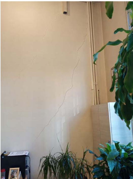
Figure 7.23. İzmir Commerce Building. Observed damages from inside the structure
