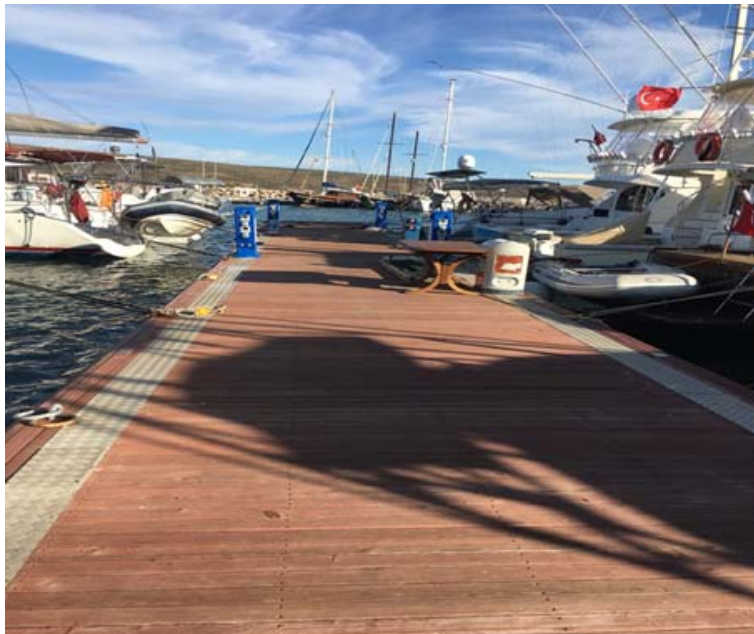
Figure 2.32. Concrete Pontoons in Alacati Marina.
