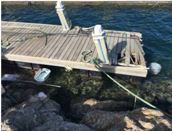
Figure 2.30. Damages in the pontoons and rings at the fairleads.
