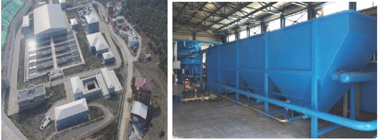
Figure 6.14. The Gordes Dam Kavaklıdere (left) and Karaburun Mordogan Potable Water Treatment Facilities in İzmir (Izsu, 2020)
