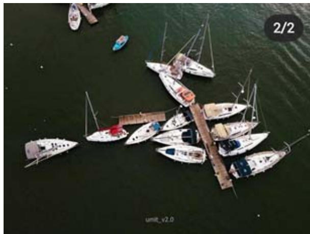
Figure 2.28. Drift of floating piers in Teos Marina after tsunami attack.
