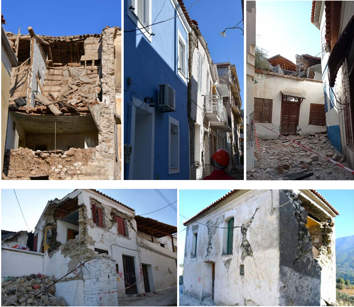
Figure 7.71. Partial collapse of residential masonry buildings.
