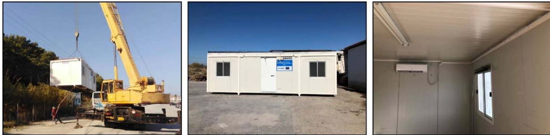
Figure 8.13: Container-type structures used as temporary housing for the homeless, for classrooms and warehouses in the earthquake-affected Samos Island. They were transported to Samos after cooperation of the Municipalities of the Western and Eastern Samos with the Municipality of Mytilene (Lesvos Island, North Aegean Sea) and the Ministry of Migration and Asylum.
