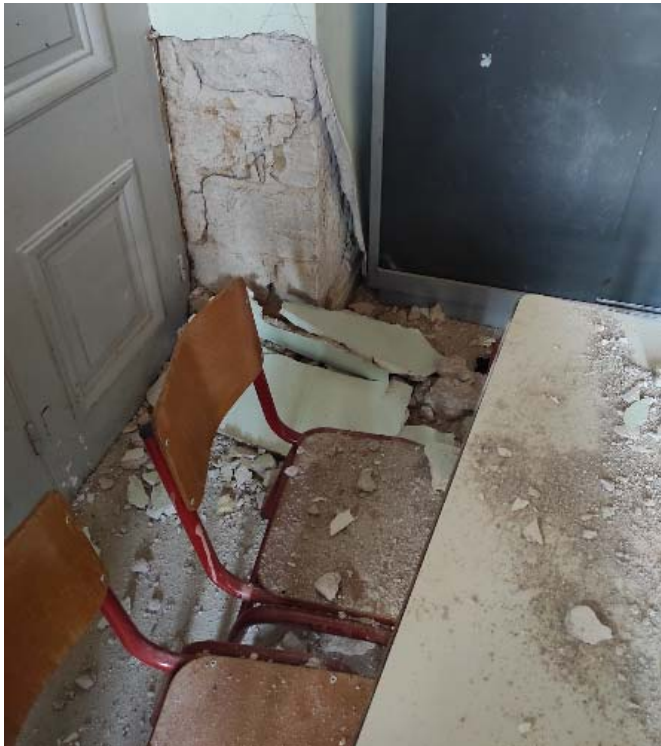
Figure 7.77. Primary school at Kontakeika: Major shear failure at the masonry walls, delamination of coating and overturning of equipment.
