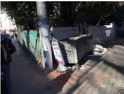
Figure 5.33. No signs of soil liquefaction. Tilted and partially collapsed very poor safety walls (38°27'24.6"N 27°10'53.1"E/ 11:10/ 04.11.2020).
