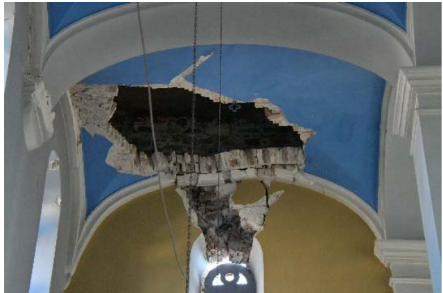
Figure 7.83. Poor construction of the dome-and-arches system.
