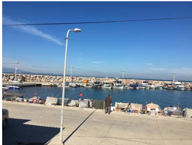
Figure 2.26. Rubble Mound Breakwater without crown wall in Guzelbahce Fishery Harbor.
