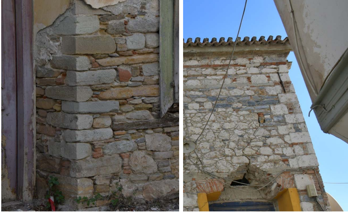
Figure 7.66. Connection of transverse walls.
