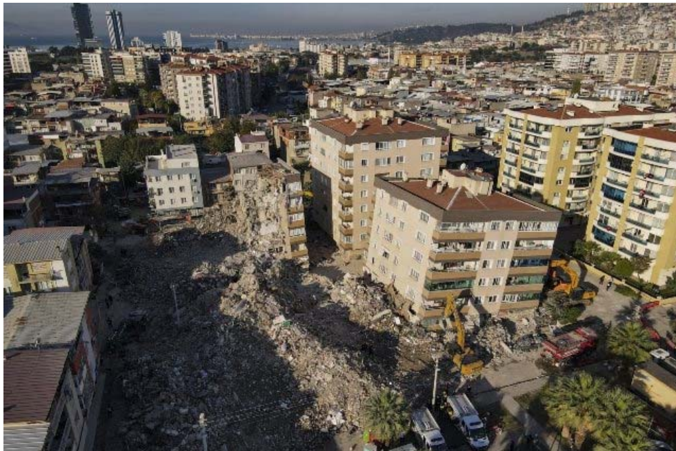
Figure 8.17. Collapsed buildings in Izmir on Friday, Oct. 30, 2020.
