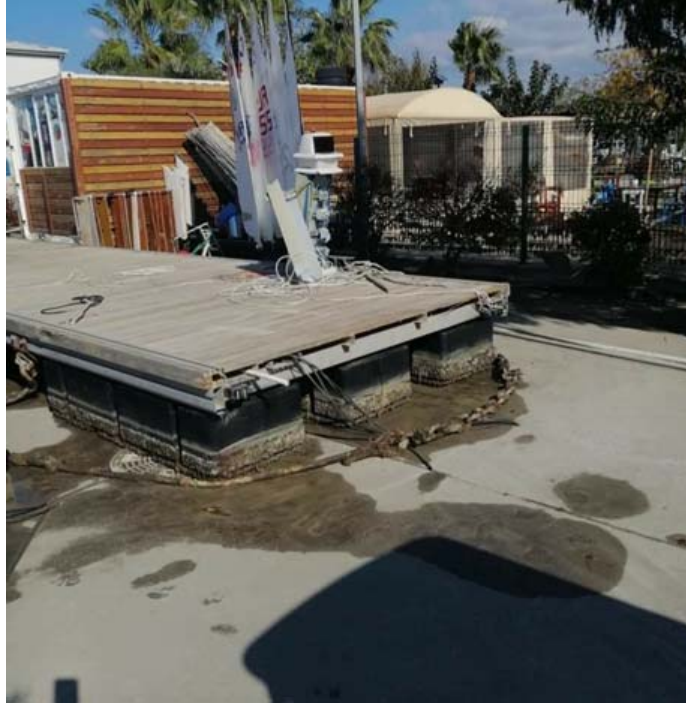
Figure 2.29. One of the pontoons used in Teos Marina (floaters are at the bottom).
