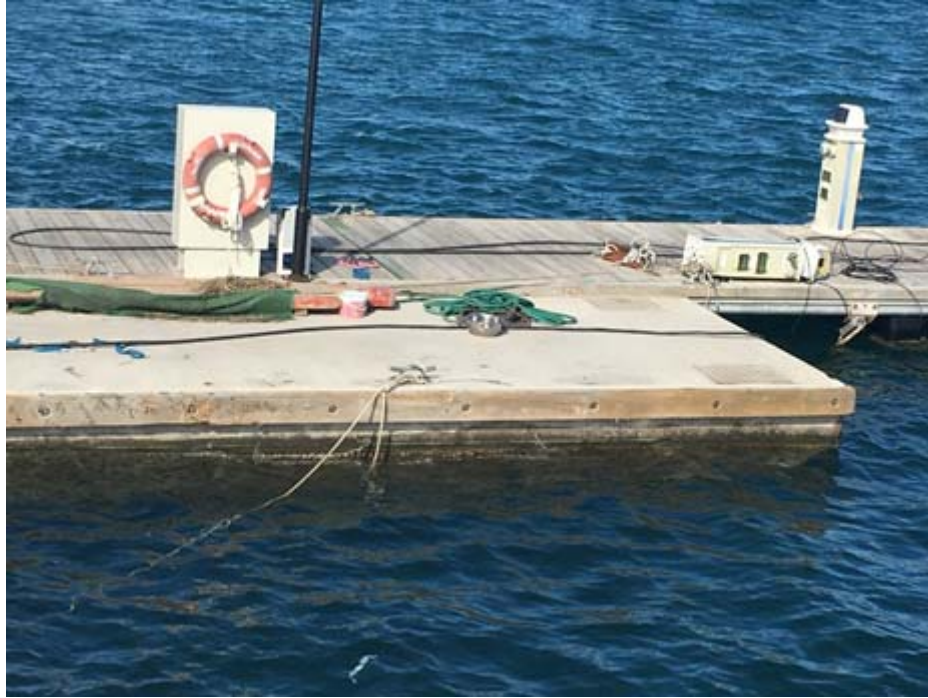
Figure 2.31. Undamaged concrete pontoon in Teos Marina.
