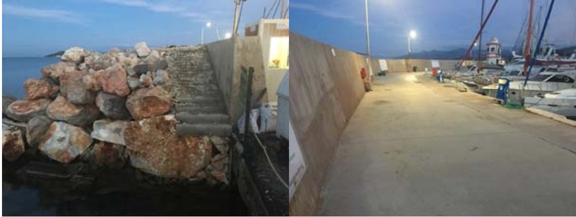
Figure 2.25. Rubble Mound Breakwater with the crown wall in Urla Fishery Harbor.
