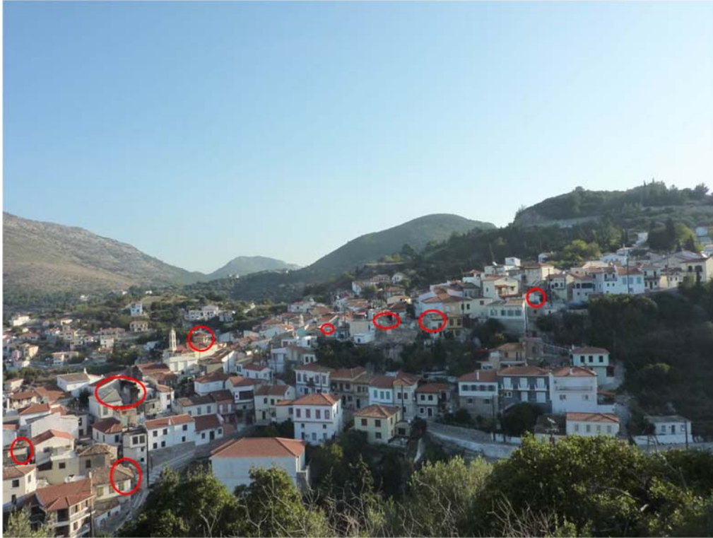
Figure 4.21. Ano Vathy hill: Red circles denote damaged buildings. (Photo by Christos Giarlelis, HAEE/ETAM Team).
