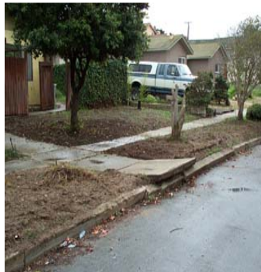
Sidewalk damaged by lateral spreading, Norswing Dr., Oceano
