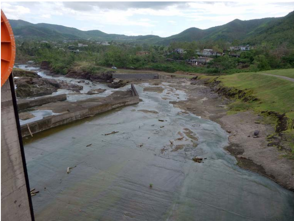
Figure B-6: Lago Guayabal Dam; Lat: +18.08733, Lon: -66.50503; 2017.10.31; #3564.
