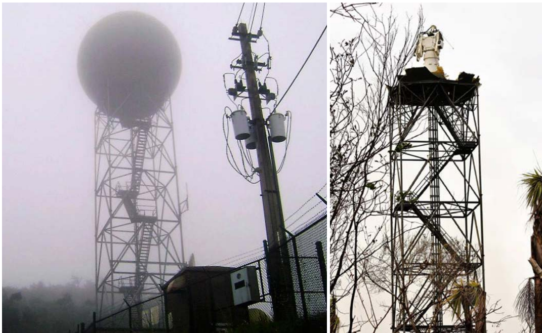
Figure 7-1: Before and after pictures of the NEXTRAD NOAA Doppler radar in Cayey, PR. (photo credit: Dr. Luis Suarez) (Lat: +18.115483, Lon: -66.077978).
