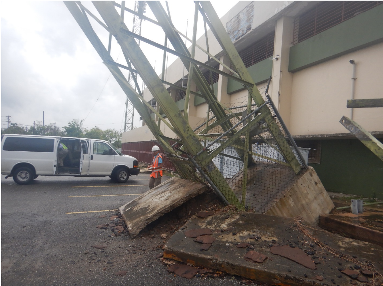
Figure 6-10: Photo of foundation failure of illumination tower at Site F4 in Ponce.
