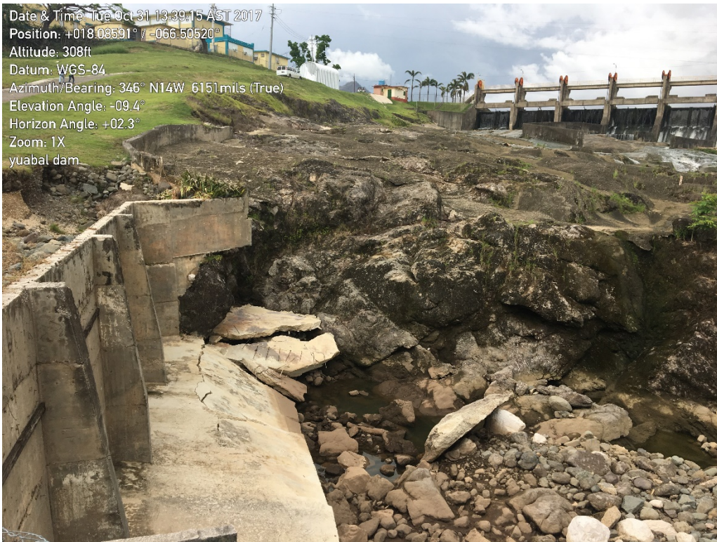
Figure B-5: Lago Guayabal Dam; Lat: +18.08591, Lon: -66.50520; 2017.10.31; #3552.
