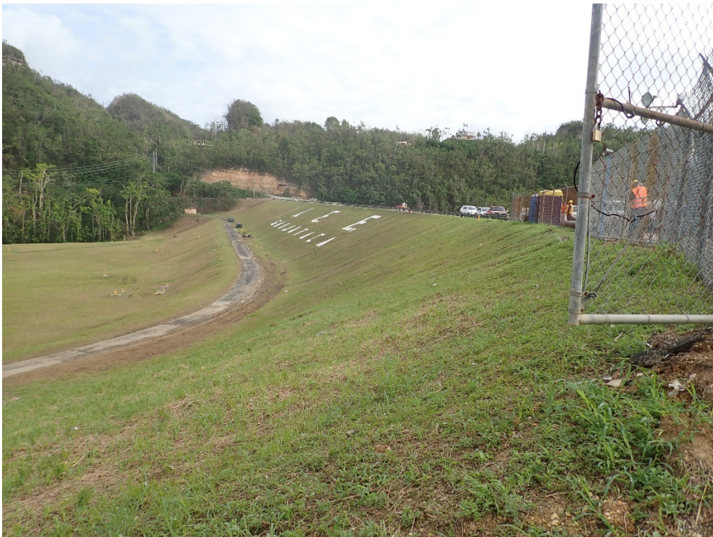
Figure B-2: Guajataca Dam; Lat: +18.39642, Lon: -66.92497; 2017.10.30; #2707.
