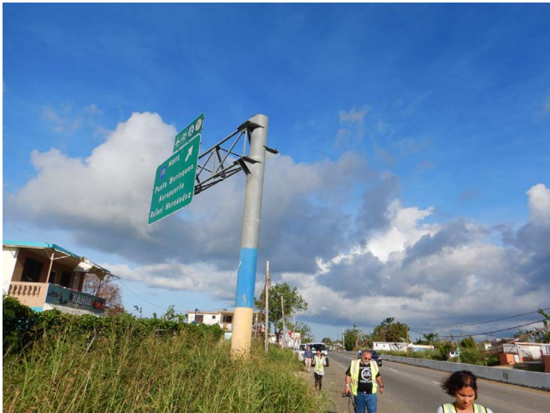
Figure 6-2: Photo of Cantilevered sign foundation failure at Site F1.
