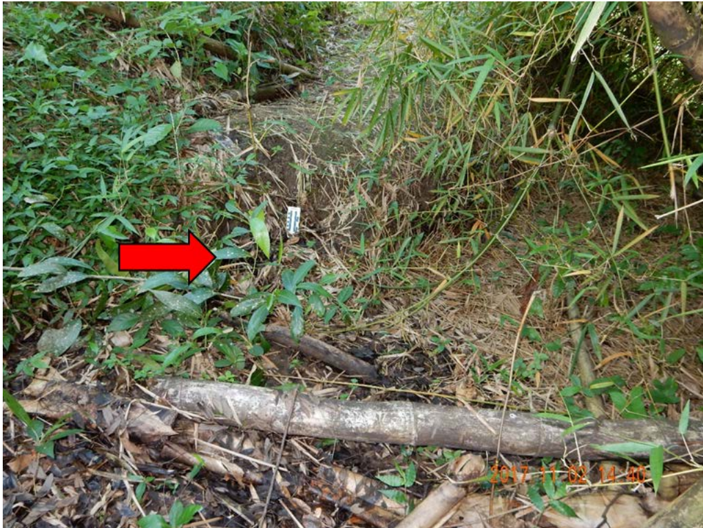
Figure A-32: Utuado, PR-146, Km 9.3, Rio Limón Slide, Toe; Lat: +18.32237833, Lon: -66.59932833; 2017.11.02; #3931.
