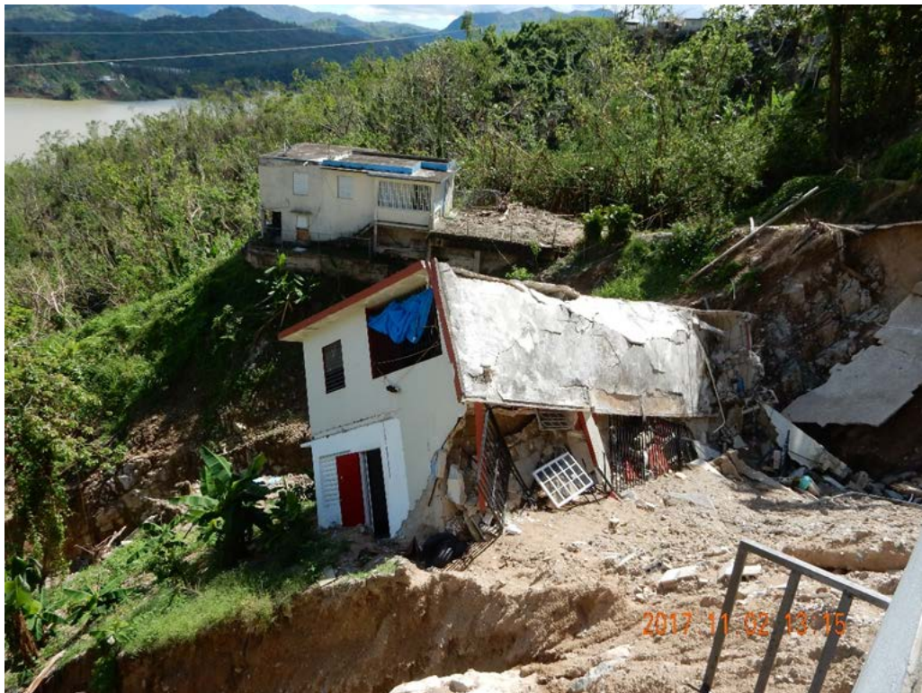
Figure A-28: Utuado, PR-140, Km 26.1, rusty cast iron pipe at head scarp; Lat: +18.26700333, Lon: - 66.66004833; 2017.11.02; #3876.
