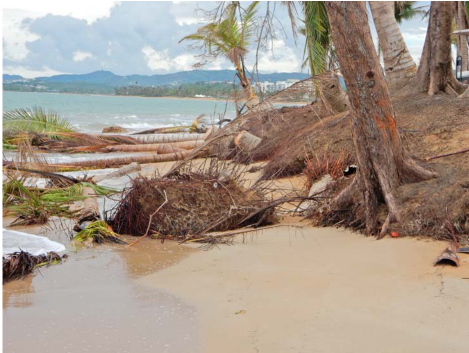
Figure 4-26: Coastal erosion at Site CE7 - Playas del Yunque, Rio Grande, PR (Lat: +18.39821, Lon: -65.76466).
