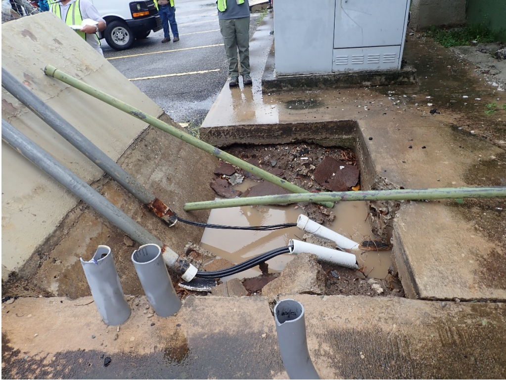
Figure E-7: Photo of the foundation spot of the tower (Lat: +18.00207, Lon: -66.63098; 2017.10.31).
