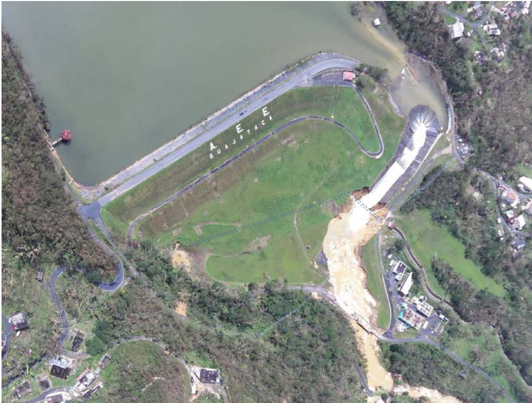
Figure 3-11: Location of 54-inch water line and siphon structure under the spillway.
