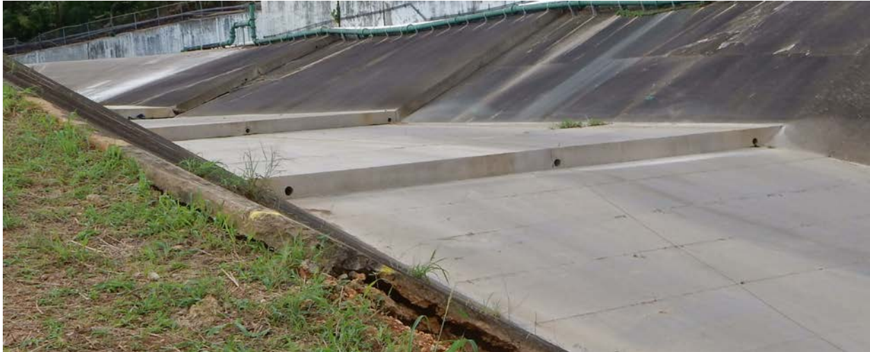
Figure 3-14: Spillway aeration pipes (Lat: +18.39684, Lon: -66.92561).
