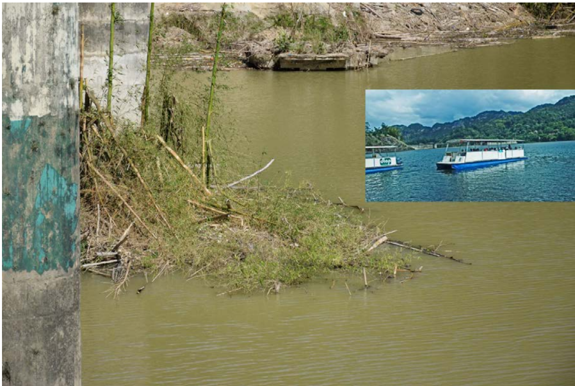
Figure 3-1: Debris along the upstream face of the gravity dam at Lago Dos Bocas. Compare the dark brown color of the water in the reservoir to the historical blue color (before Maria) (Lat: +18.27691, Lon: -66.6561).
