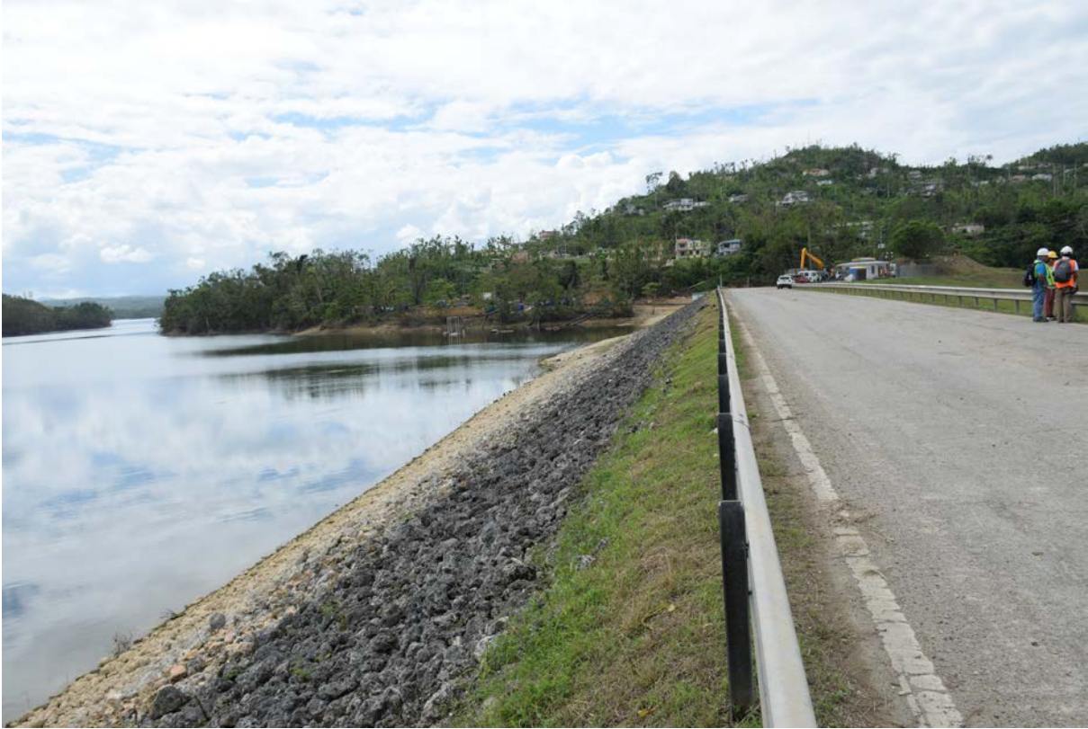
Figure 3-17: Dam crest (Lat: +18.39733, Lon: -66.92374).
