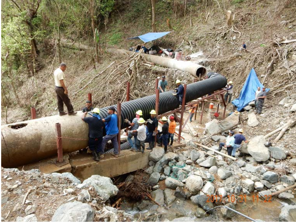
Figure A-16: Temporary repairs; Lat: +18.15865, Lon: -66.49810; 2017.10.31; #3506.
