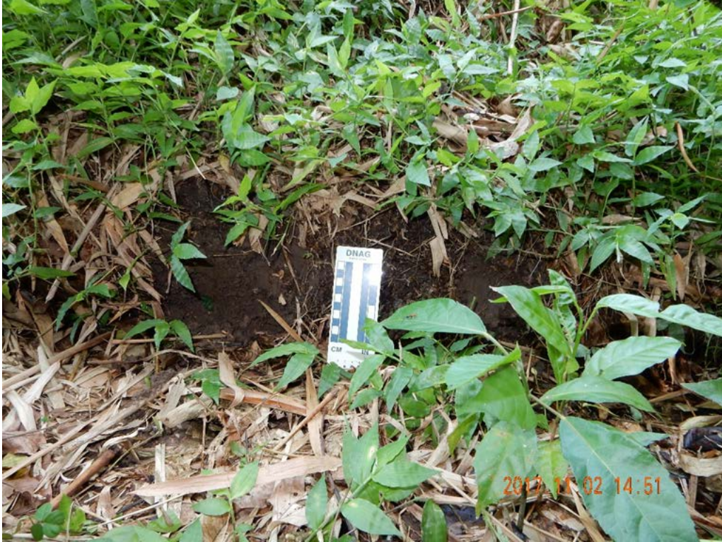
Figure A-33: Utuado, PR-146, Km 9.3, Rio Limón Slide, Toe; Lat: +18.32237833, Lon: -66.59932833; 2017.11.02; #3934.
