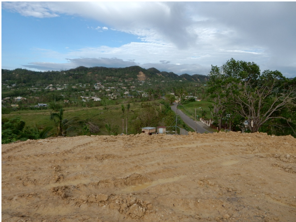
Figure A-9: Moca, PR-110 failures from a distance; Lat: +18.38861, Lon: -67.07504; 2017.10.29; #3305.
