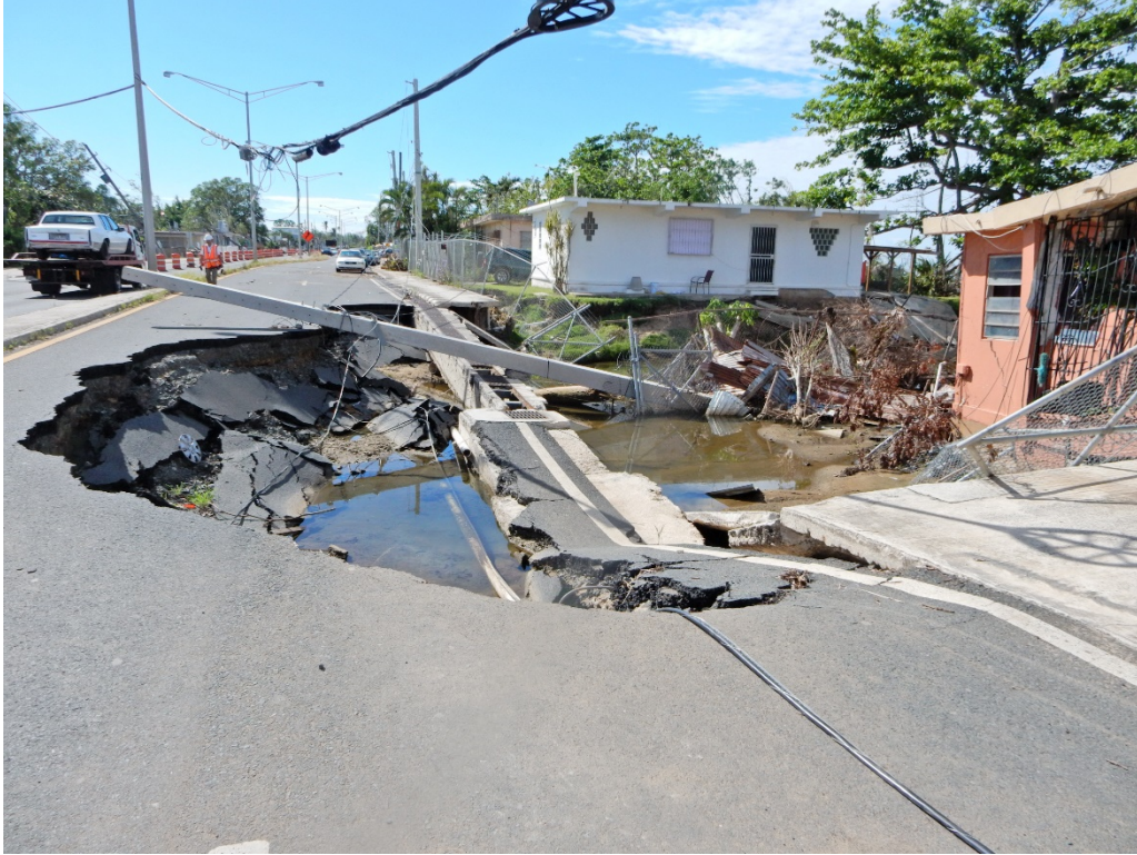
Figure C-8: Coastal erosion at El Maní, Mayagüez; Lat: +18.24457, Lon: -67.17390; 2017.11.04; #4151.
