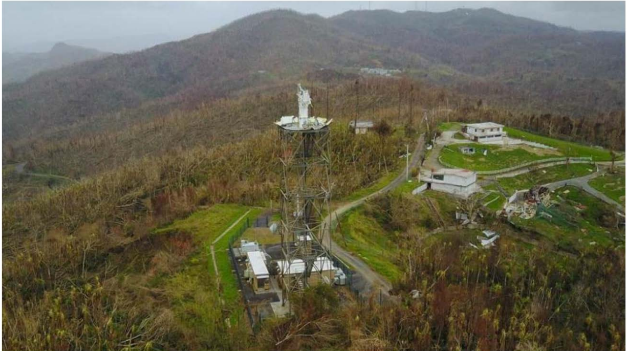
Figure 10. The remnants of the San Juan WSR-88D radar after its destruction by Hurricane Maria. Photo credit: WFO San Juan.
