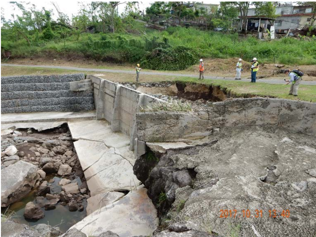
Figure B-4: Lago Guayabal Dam; Lat: +18.08618, Lon: -66.50519; 2017.10.31; #3551.
