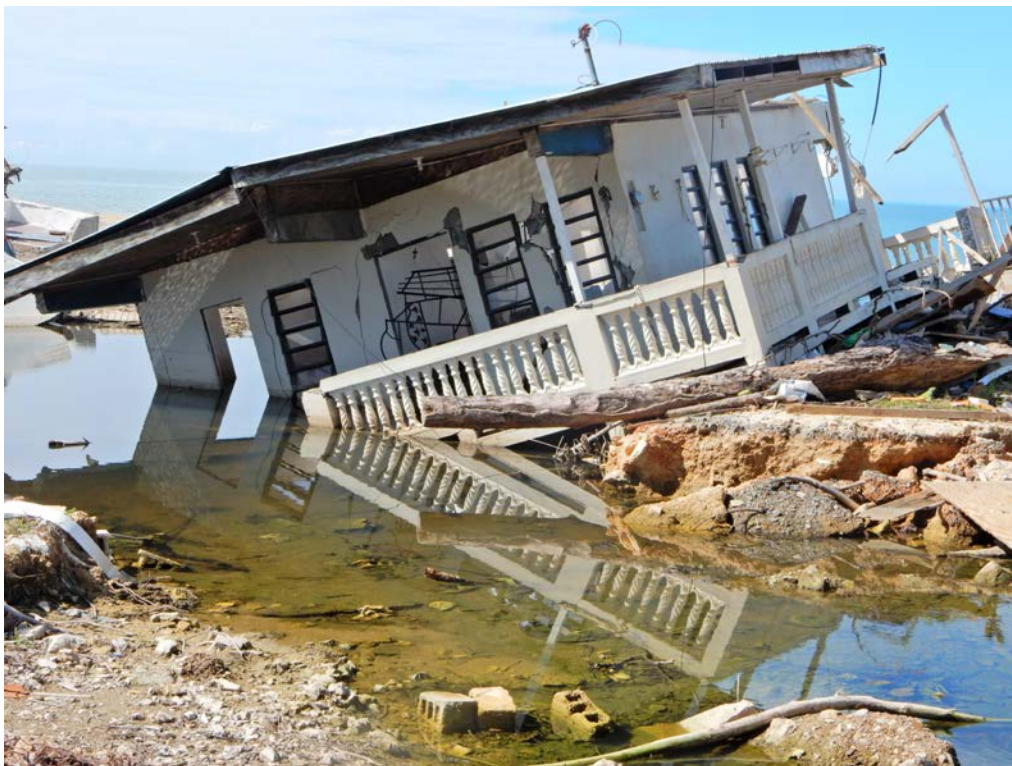
Figure 4-25: Coastal erosion at Site CE6 - Playa El Maní, Mayagüez, PR.
