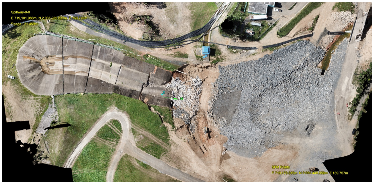
Figure G-1: The orthomosaic of the damaged spillway at Guajataca dam from a hybridized model of SFM imagery analysis and TLS LIDAR data.
