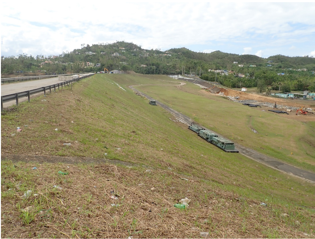
Figure B-1: Guajataca Dam; Lat: +18.39878, Lon: -66.92330; 2017.10.30; #1159.
