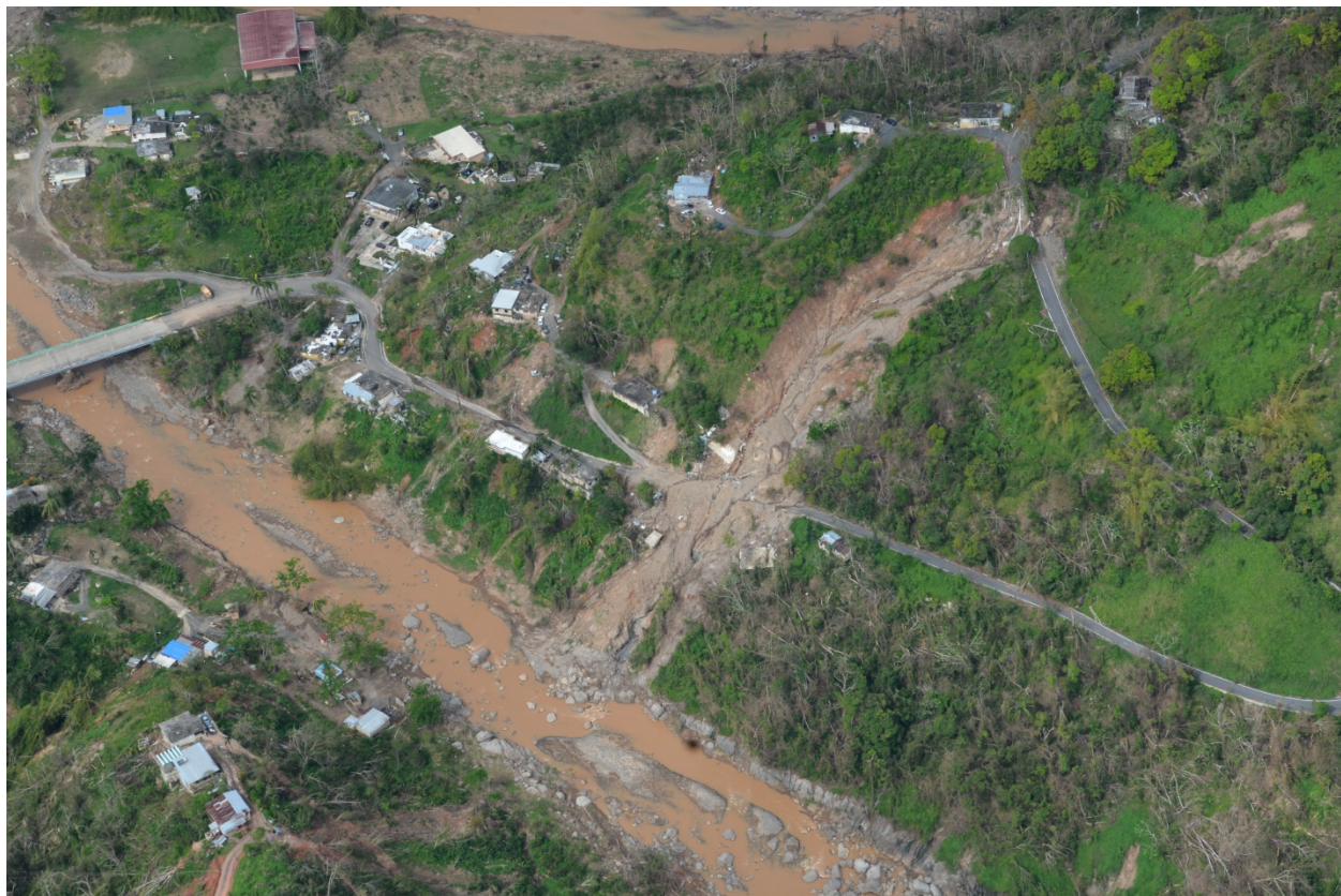
Figure 2-10: Photo taken by the Civil Air Patrol on October 15, 2017 of the PR-4131 debris flow site (Lat: +18.247885, Lon: -66.882794).
