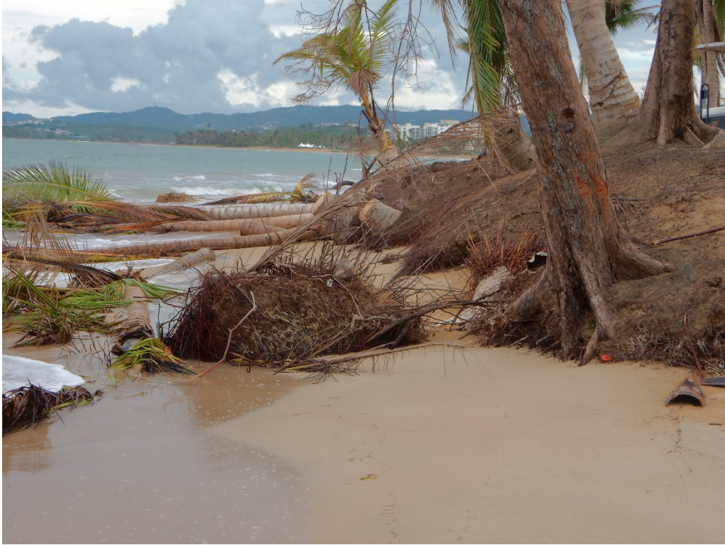
Figure C-1: Coastal Erosion, Yunque Mar, Rio Grande, PR; Lat: +18.39770, Lon: -65.76260; 2017.10.28; #3209.
