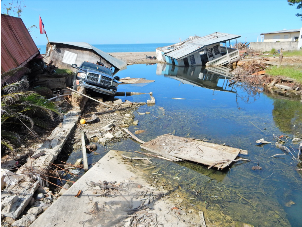
Figure C-9: Coastal erosion at El Maní, Mayagüez; Lat: +18.23323, Lon: -67.17270; 2017.11.04; #4180.
