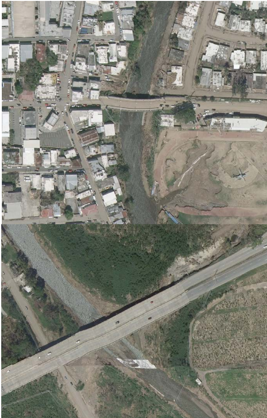
Figure 5-3: Images showing induced curvature on bridges near Yauco, PR, due to heavy river flows during Hurricane Maria (images from NOAA taken a few days after Maria).
