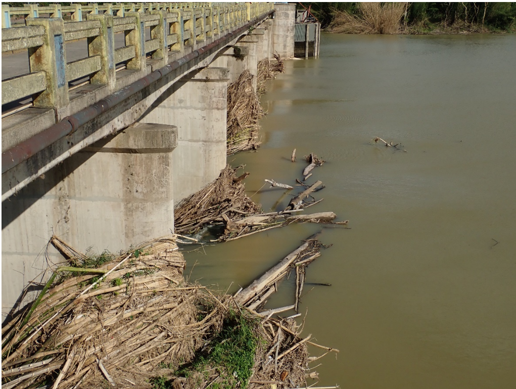
Figure B-10: Utuado, Dos Bocas Dam; Lat: +18.33570, Lon: -66.66798; 2017.11.02; #3941.
