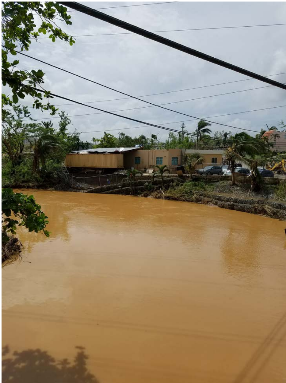
Figure 4-41: River bank erosion failure of Guaynabo River at Site RE3 (Photo by Geo-Cim) (Lat: +18.37356, Lon: -66.13253).
