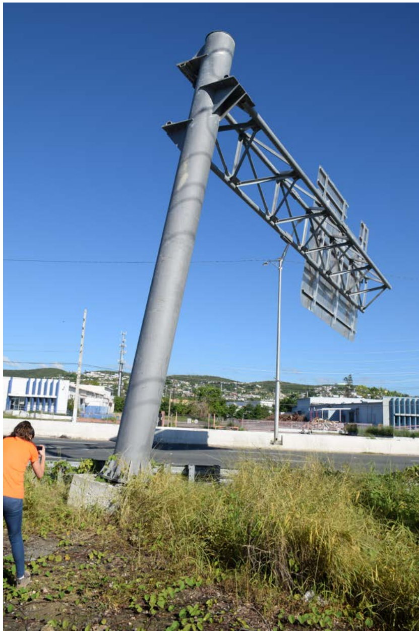
Figure 6-9: Photo showing the rotation of the traffic sign at Site F3.
