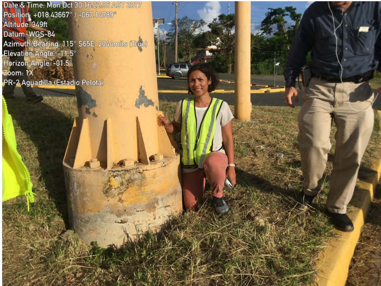
Figure 6-6: Photo of drilled shaft foundation of traffic sign at Site F2.
