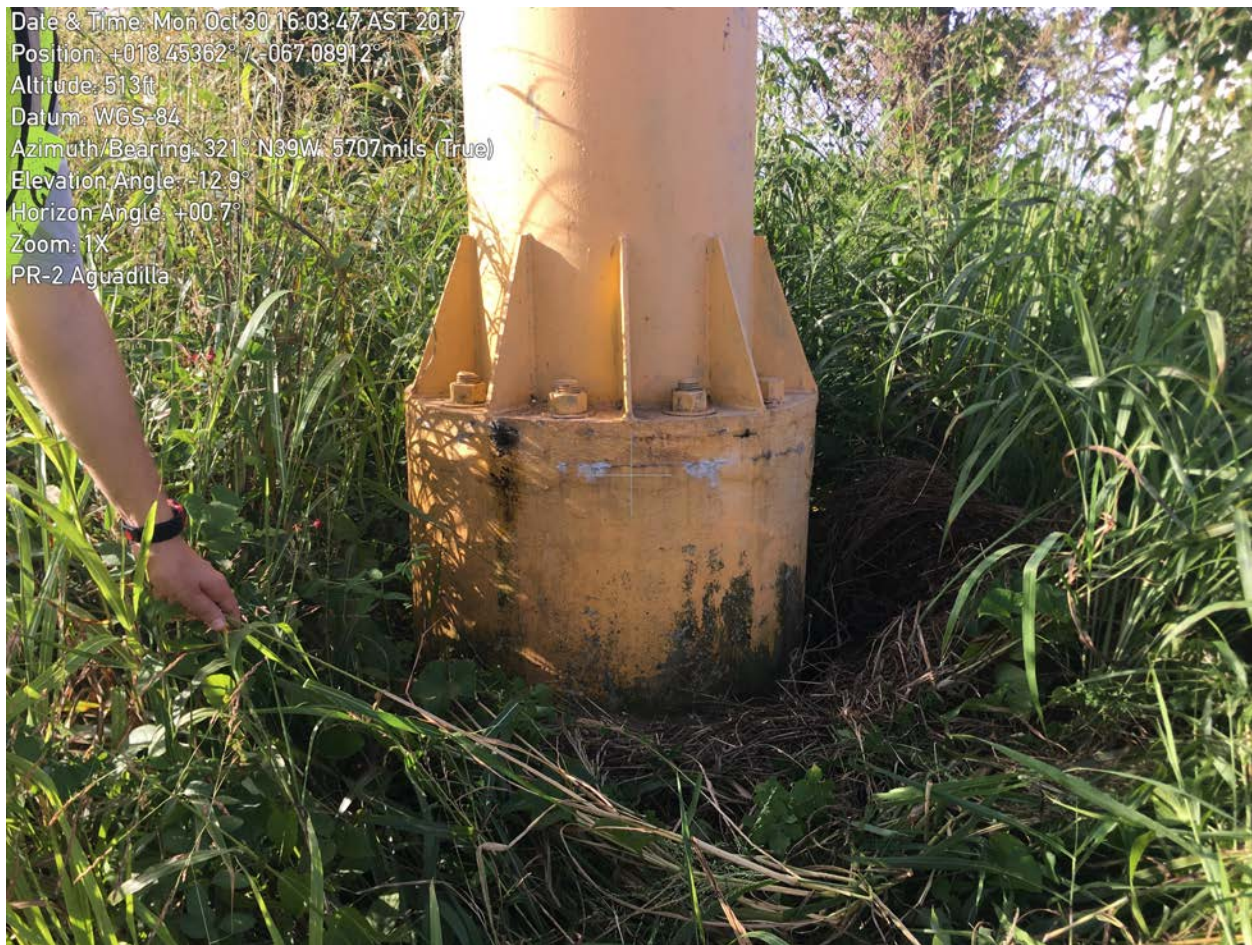
Figure 6-4: Photo of drilled shaft foundation of traffic sign at Site F1.
