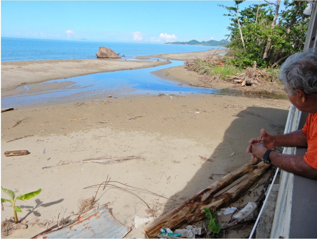
Figure C-10: Coastal erosion at El Maní, Mayagüez; Lat: +18.24732, Lon: -67.17516; 2017.11.04; #4176. Previously grassy area after Hurricane María.
