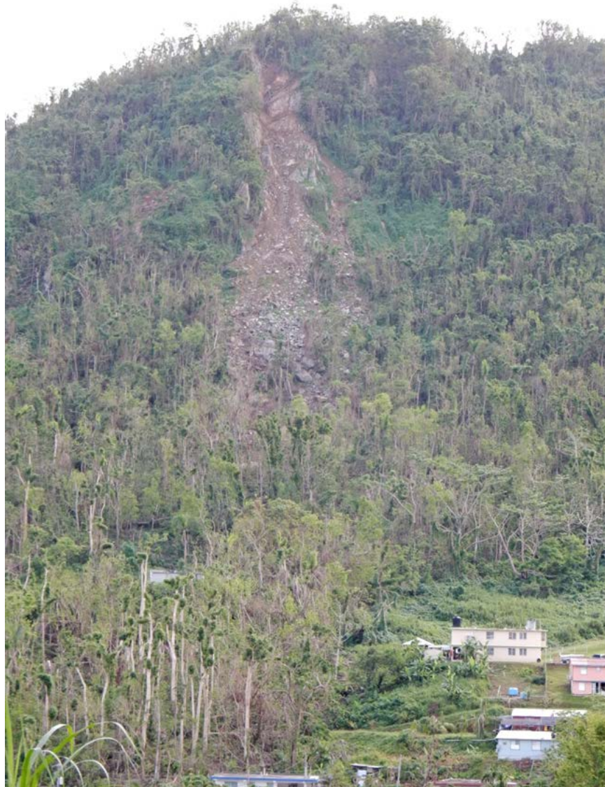
Figure A-39: Debris flow; Lat: +18.309755, Lon: - 65.89074333; 2017.11.05; #4231.
