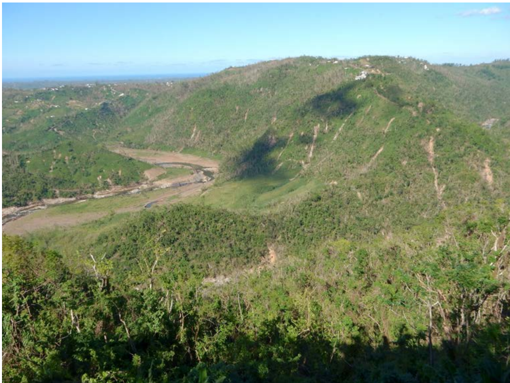
Figure A-21: Debris Flows; Lat: +18.28422, Lon: -66.40087; 2017.11.01; #3700.
