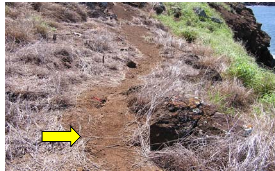
Figure 25: Location 23, Kuakini Trail. Tension cracks behind cliff top (arrow).
