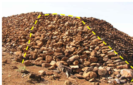
Figure 34: Location 29, Pu'ukoholā heiau, northeast corner. Dashed lines indicate boundary of ravel zone.
