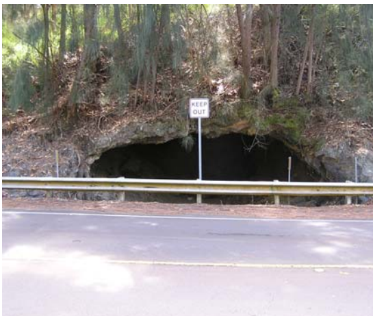
Figure 16: Location 7, Hwy 240, near Kapulena, north of Honokaa. Lava tube, with apparently little rockfall from roof and walls.
