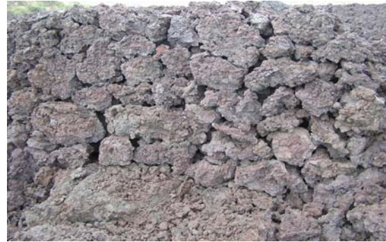
Figure 29: Location 11, Saddle Road (Hwy 200). Stacked rock wall of a'a clinker.
