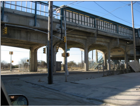
Figure 6.26 Elevated subway structure at Beach 44 th Street showing little visible damage, Arverne, Queens (40.593287° N, -73.775318° W, November 4, 2012)
