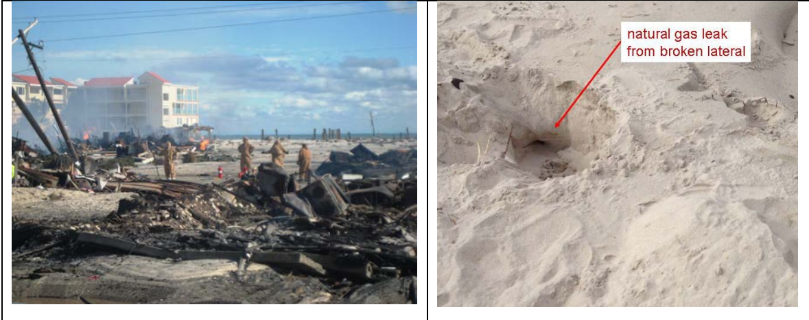
Figure 6.95 Natural gas leak and fires (NJ Task Force 1, 2012)
