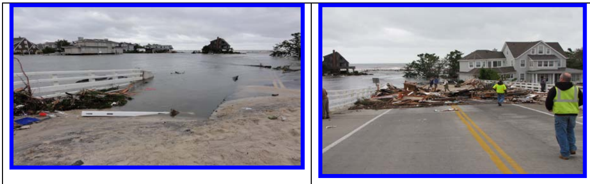
Figure 5.19 Approach to Mantoloking Bridge, which was flooded soon after the storm and inundated by debris (40° 2'24.21" N, 74° 3'6.79" W , Ocean County Engineering, 2012)
