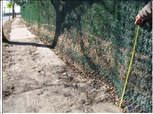
Figure 6.57 High water mark at 2.5 feet on fence, north side of Lido Blvd at Buxton Street, Long Beach (40.588431 °N, 73.627142 °W, November 4, 2012)
