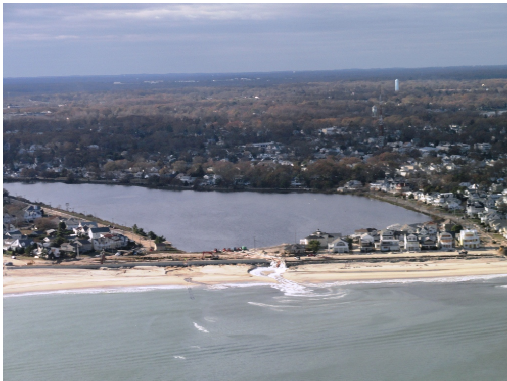
Figure 6.100 Lake Como, Borough of Como, with dewatering pumps, 40°10'1.50"N, 74° 1'1.65"W (NJ Task Force 1, 2012)
