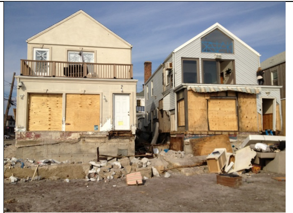
Figure 6.36 Beachfront houses with concrete wall foundations, Rockaway, Queens (November 18, 2012 – MRCE in collaboration with NYCDOB)
