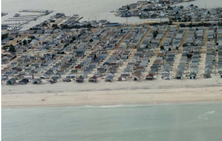
Figure 6.99 Homes partially buried in ocean sand, Borough of Lavallette (A. Brenner, 2012)
