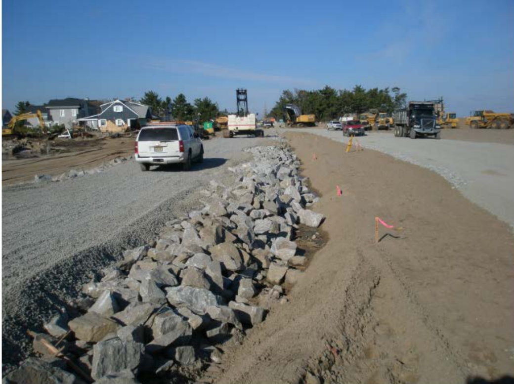
Figure 5.24 NJ-35 in Mantoloking looking north towards the bridge (40° 2'22.95"N, 74° 3'0.53"W, NJDOT, 2012a)
