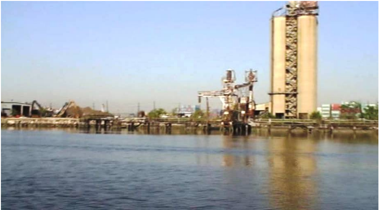
Figure 7.50 Passaic River Shoreline near Newark Bay
