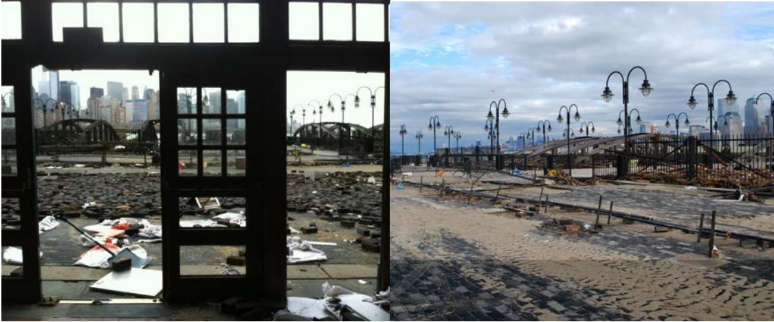
Figure 6.112 Damage to stone pavers at Liberty State Park occurred but these protected subsoil from erosion (40°42'26"N, 74°02'05"W).
