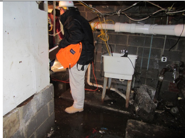
Figure 7.11 Typical flooded basement, South Street seaport (40.708301° N, 74.000605° W, November 4, 2012).
