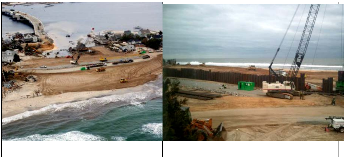
Figure 6.92 Installation of sheet piles to allow backfilling erosional channel and rebuilding of Route 528, Borough of Mantoloking, 40° 2'24.21"N, 74° 3'8.32"W (Mantoloking, 2012).
