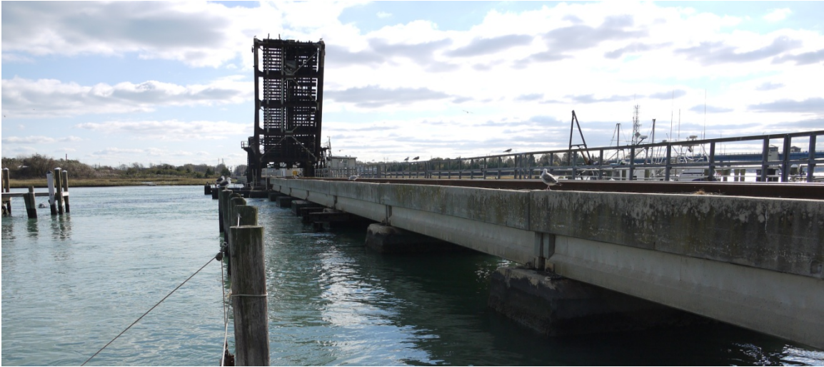
Figure 5.4 Railroad draw bridge at Manasquan River looking south (40.10700°N, 74.04998°W, November 5, 2012)
