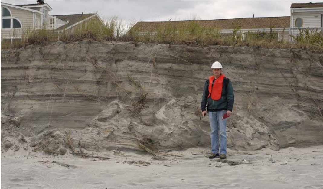
Figure 6.77 Barrier dune erosion (39.40929 ° N, 74.35996 ° W, November 3, 2012)
