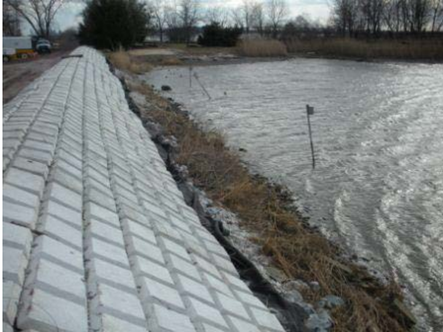
Figure 6.111 Repair work was completed by placing articulating concrete mats over displaced pipeline.
