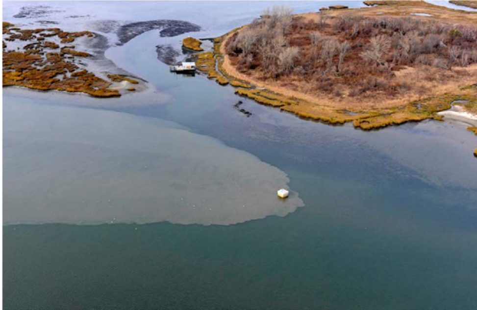
Figure 7.33 Overflow from the Bay Park Sewage Treatment Plant in East Rockaway, N.Y. Hurricane Sandy resulted in over 2 billion gallons of sewage overflow from this facility. Some of this overflow (estimated at 68 million gallons) was released adjacent to the Western Long Island South Shore Estuary (above). Photo courtesy of Doug Kuntz. Modified from Kenward, Yawitz and Raja, 2013.
