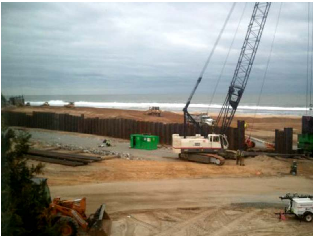
Figure 5.23 Sheet Piles driven in Mantoloking along the breached section (40° 2'22.95"N, 74° 3'0.53"W, NJ Task Force 1)
