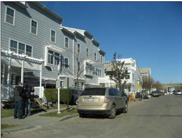
Figure 6.31 Three-story buildings with little visible structural damage, Beach 76 th Street and Rockaway Beach Blvd, Rockaway Beach, Queens (40.588689° N, 73.803595° W, November 4, 2012)
