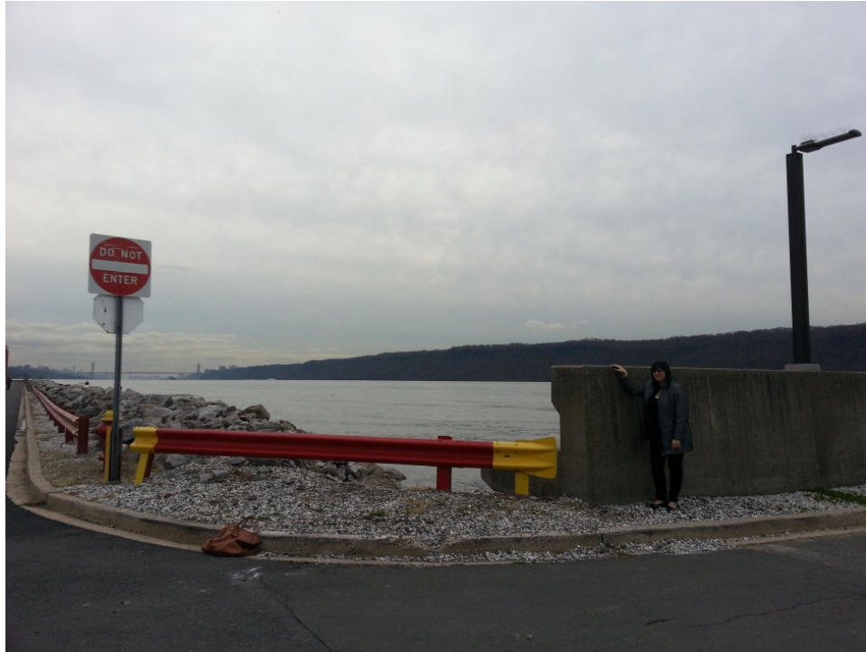
Figure 7.35 Junction of rip-rap revetment and seawall, looking south.
