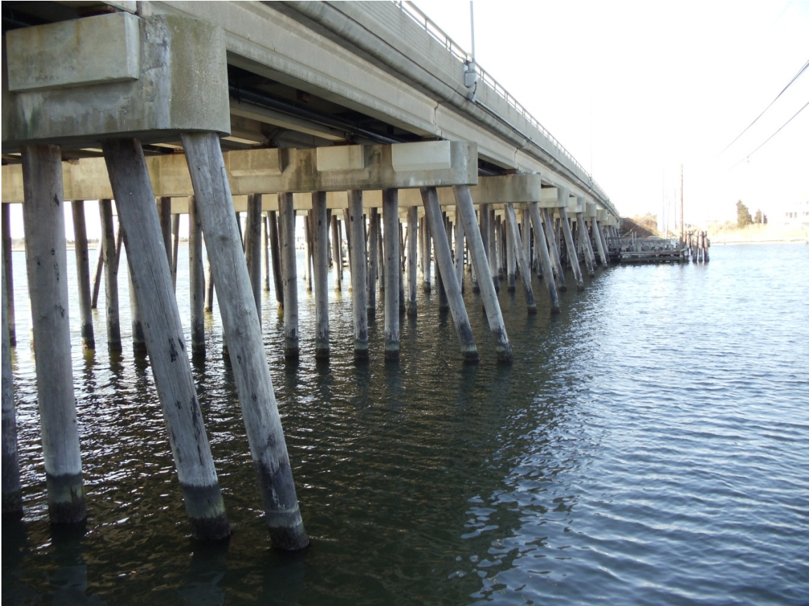
Figure 5.25 Easternmost section of the Highway 72 Bridge looking westward (39°39'13.77"N, 74°11'4.11"W).
