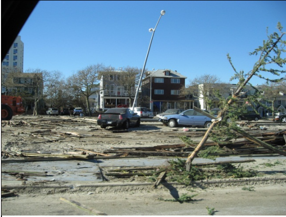
Figure 6.33 Debris and cars moved inland, Beach 94 th Street and Shore Front Road, Rockaway Beach, Queens (40.584691°N, 73.815873° W, November 4, 2012)
