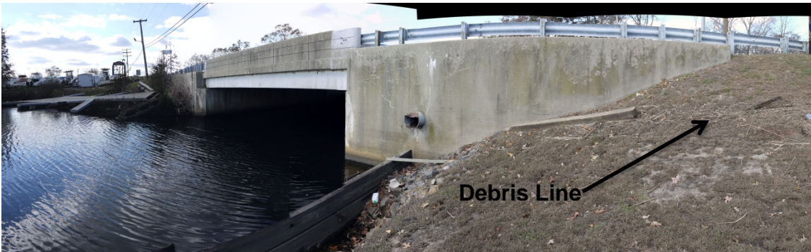
Figure 5.9 Route 70 bridge over the Metedeconk River (40.06607°N, 74.13284°W, November 5, 2012)
