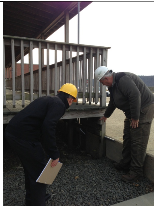
Figure 7.38 Ultimate flood water elevation indicated by plant superintendent.
