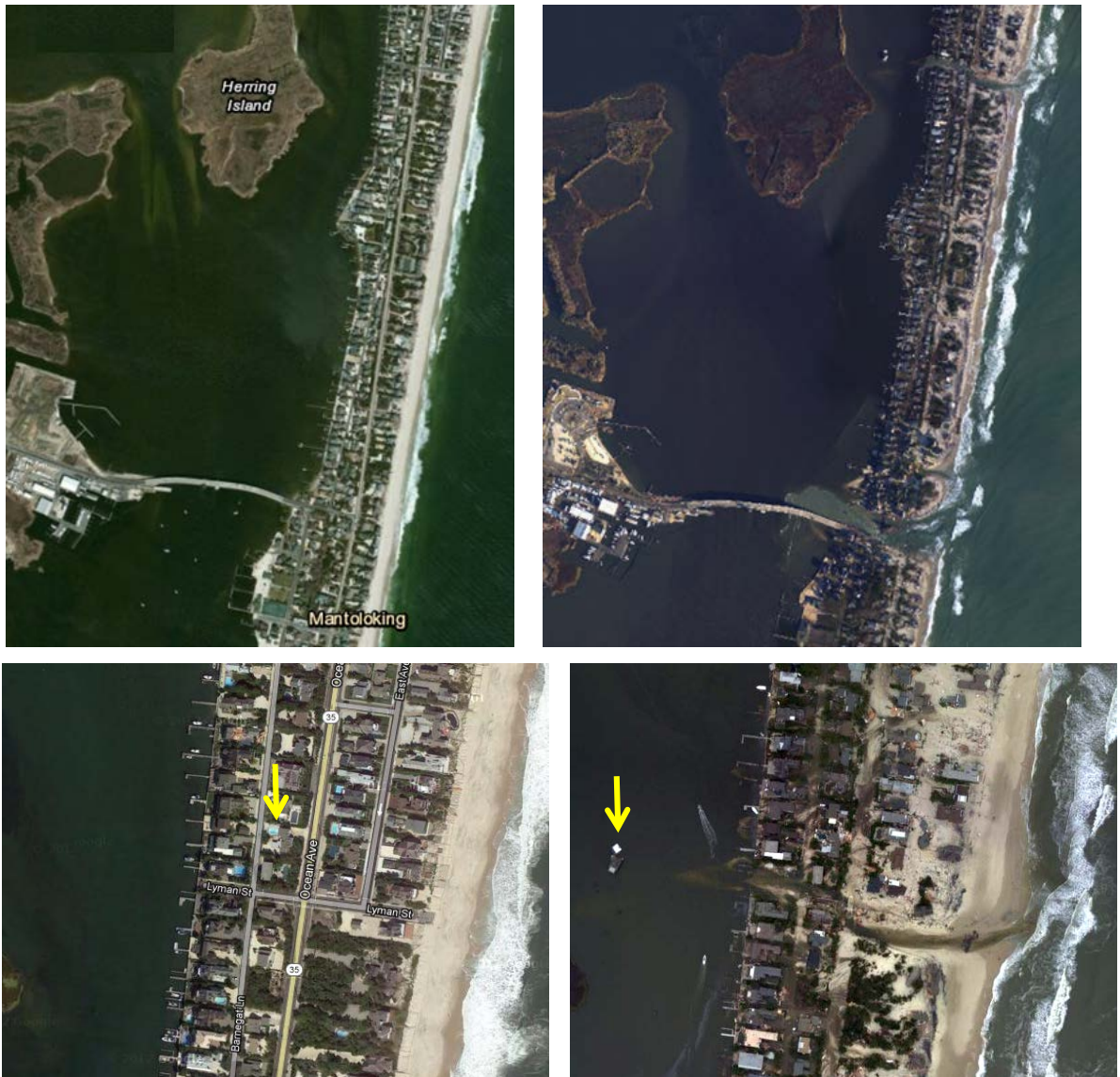
Figure 4.11 Before and after photos – Houses destroyed and new Inlet formed at Mantoloking – Bayhead, NJ. note home with pool moved 100 yards west into the bay [developed by Schick, K., NJDEP] Ref: tmappevents.esri.com/website/swipe_sandy/
