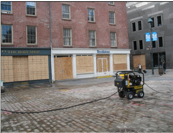
Figure 7.6 Flood damage, South Street seaport (40.706685° N, 74.003554° W, November 3, 2012).
