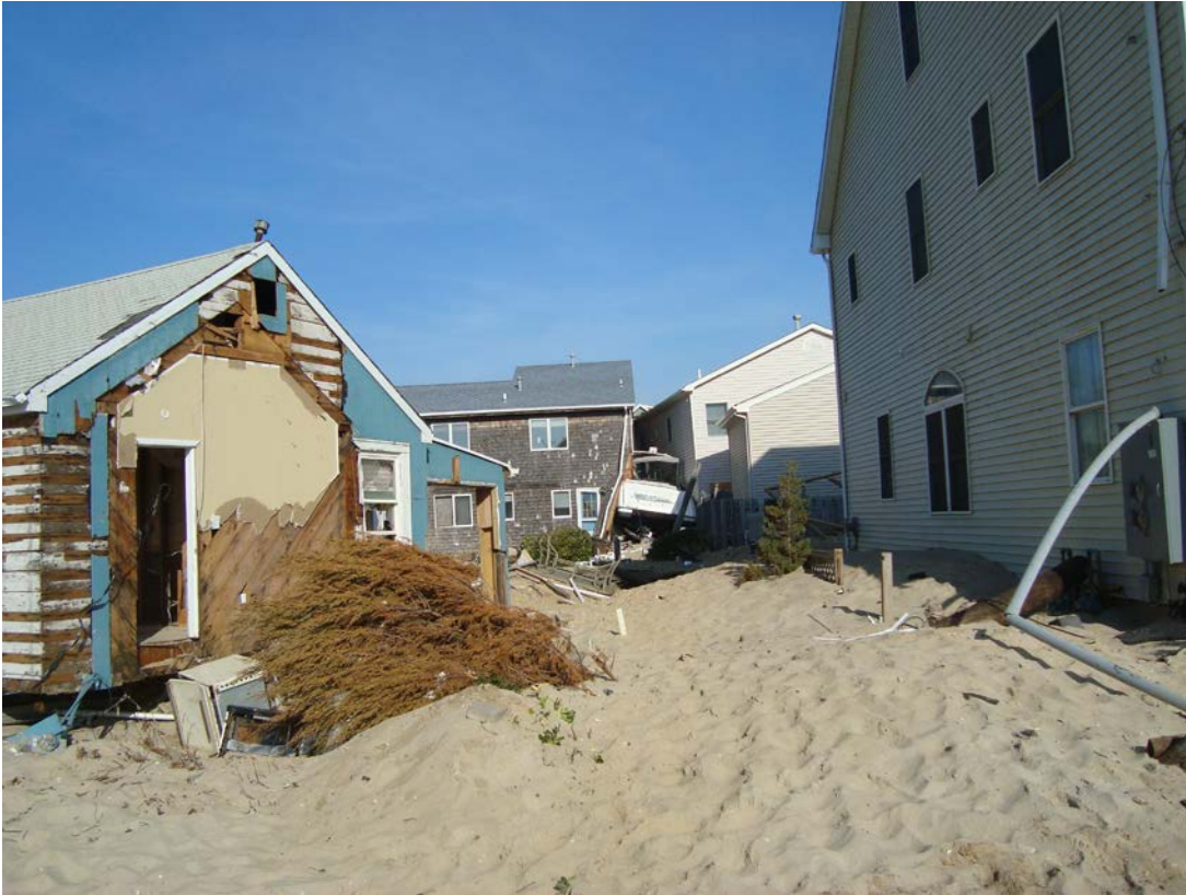
Figure 6.102 The building on the left, which was on shallow foundations was displaced. In the far end, there is a boat that is stuck in between the buildings.
