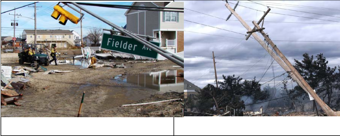
Figure 6.93 Foundation failures of utility poles (left) and damage to traffic signals, 39°57'12.03"N, 74° 4'25.09"W (NJ Task Force 1, 2012)
