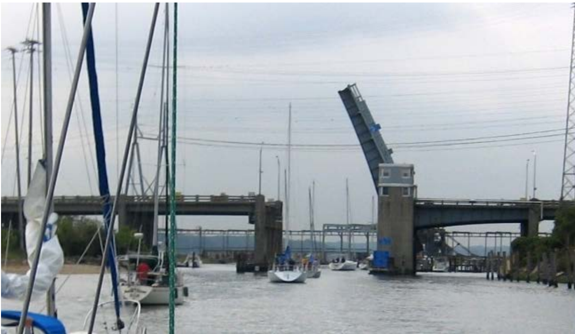
Figure 5.2 Cheesequake River Drawbridge looking eastward (NJDOT 2012b)
