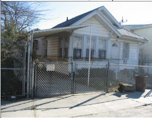
Figure 6.28 High water line on house, Beach 46 th Street, Rockaway Beach (40.594443° N, 73.77725° W, November 4, 2012)
