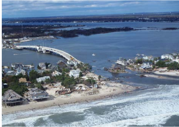
Figure 6.91 Post-Sandy conditions, Borough of Mantoloking. The bay has joined the ocean at the Route 528 Bridge, 40° 2'24.21"N, 74° 3'8.32"W (NJ Task Force 1).
