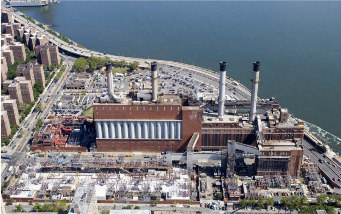
Figure 7.30 Consolidated Edison's East 13 th Street complex, which was flooded in Hurricane Sandy. Photo credit: Consolidated Edison, in Khinda et al (2013).
