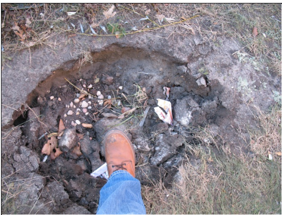
Figure 6.58 Typical sinkhole near Long Beach Blvd, Long Beach (40.585174 °N, 73.65811° W, November 4, 2012)
