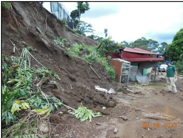
Fig. 5.7 – Slope failures near built dwellings and roads. (a) Collapse of steep bank on to small house; (b) Light construction single story and carports built on top of steep slope with water utilities located a toe of slope, likely contributed to the slope failure.
