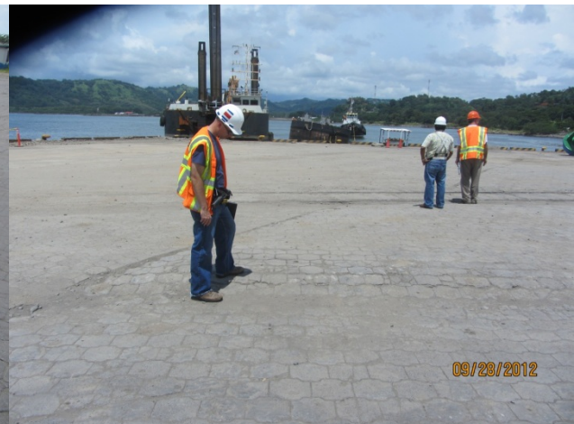
Fig. 3.3 - Apparent heave of rectangular area on the (a) west (9.91170° N 84.72194° W) and (b) east (9.91246° N 84.71811° W) ends of the port.
