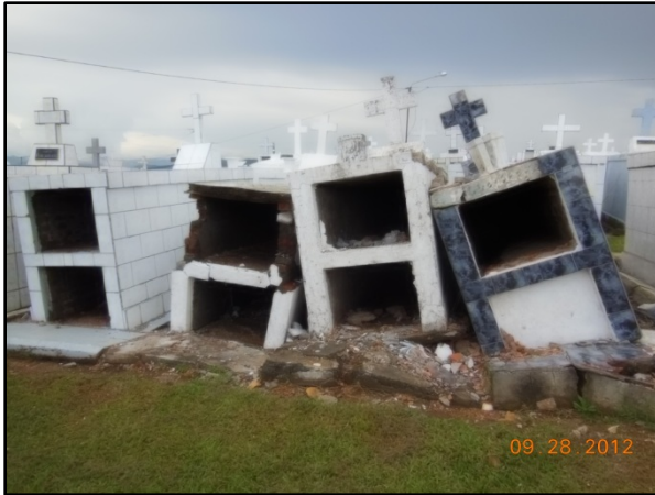
Fig. 5.6 – Cemetery damage in the town of Grecia (a) Excessive tilting, subsidence, and bearing capacity failures; likely due to construction over old underground burial sites; (b) Perimeter gravity retaining wall failed at different locations.
