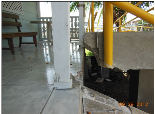
Fig. 2.6 – Structure tilted toward the west side (a) west side bottomed out at the top of the water tank; (b) new handicapped ramp detached from building front porch.
