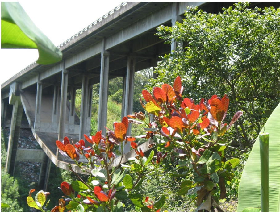
Fig. 4.23 - Inverted arch section of Rafael Iglesias bridge
