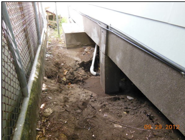
Fig. 2.6 – Structure tilted toward the west side (a) west side bottomed out at the top of the water tank; (b) new handicapped ramp detached from building front porch.
