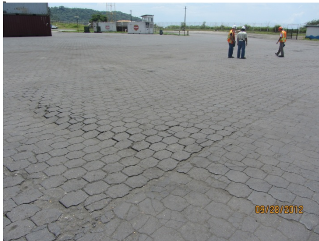
Fig. 3.3 - Apparent heave of rectangular area on the (a) west (9.91170° N 84.72194° W) and (b) east (9.91246° N 84.71811° W) ends of the port.
