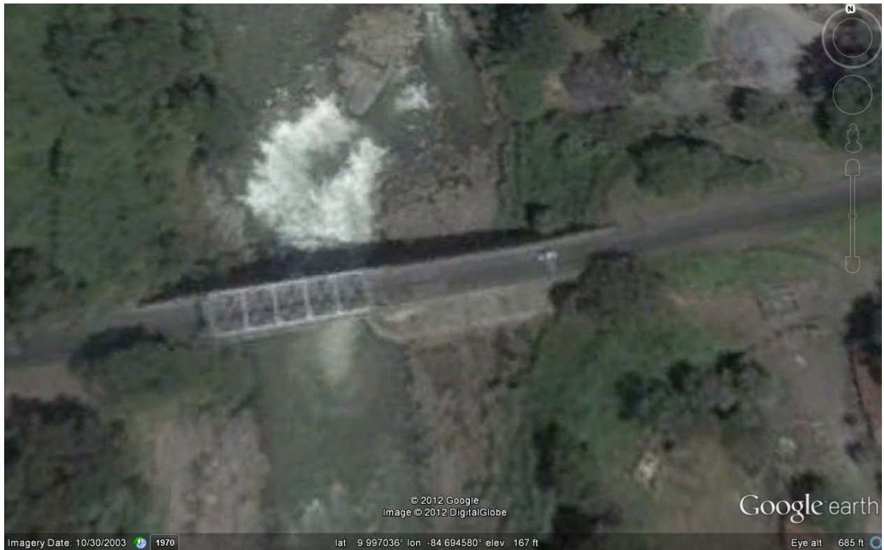
Fig. 4.2 - Aerial view of the Rio Barranca Bridge (courtesy of Google Earth™). (9.9970° N 84.6946° W).
