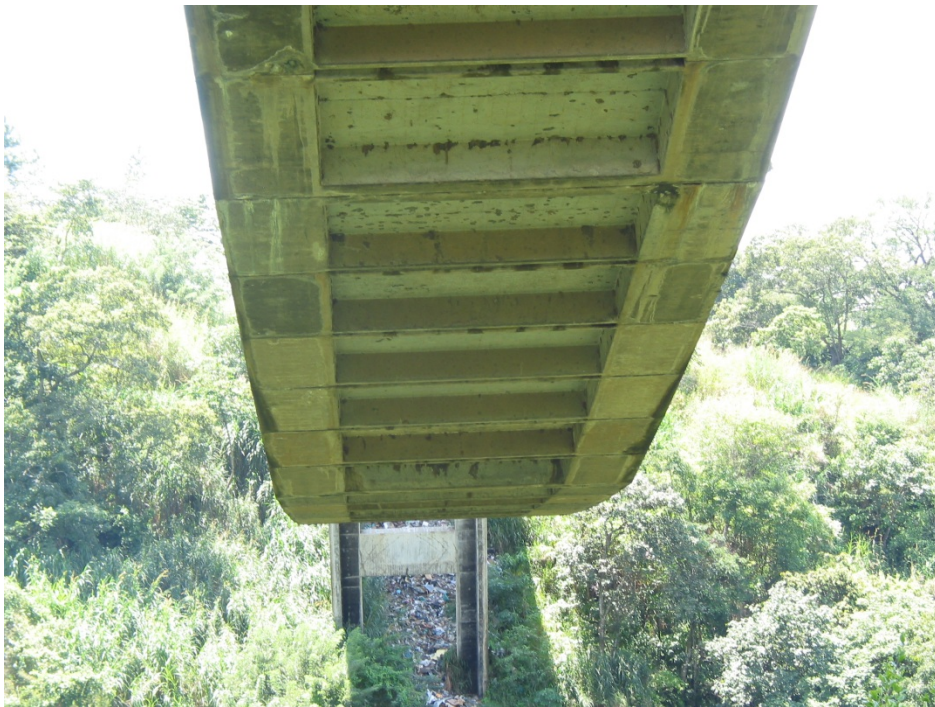
Fig. 4.24 - View of segmented inverted arch section, Rafael Iglesias bridge
