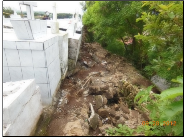
Fig. 5.6 – Cemetery damage in the town of Grecia (a) Excessive tilting, subsidence, and bearing capacity failures; likely due to construction over old underground burial sites; (b) Perimeter gravity retaining wall failed at different locations.
