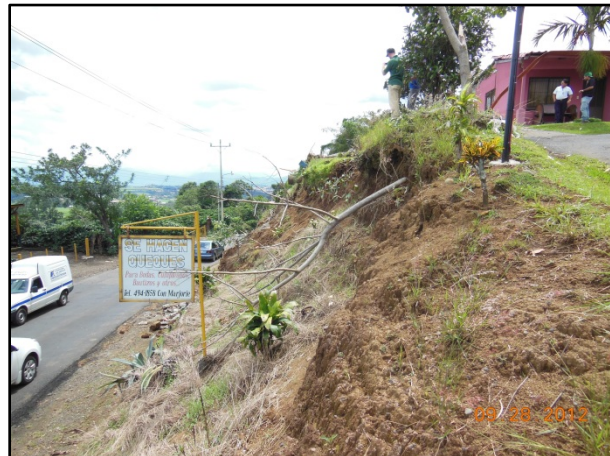
Fig. 5.7 – Slope failures near built dwellings and roads. (a) Collapse of steep bank on to small house; (b) Light construction single story and carports built on top of steep slope with water utilities located a toe of slope, likely contributed to the slope failure.
