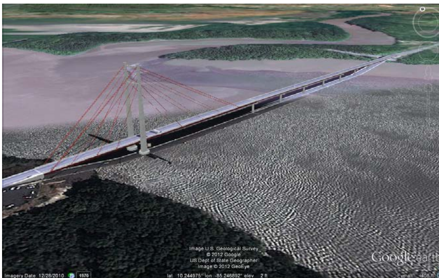
Fig. 4.15 - 3-dimensional representation of the bridge over the Rio Tempisque (courtesy of Google Earth™) (10.2468° N 85.2468° W).
