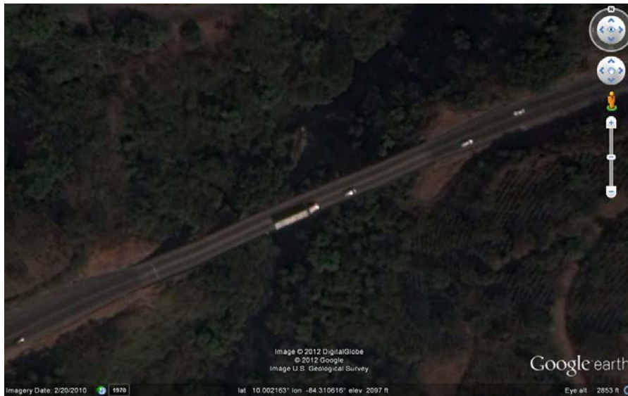
Fig. 4.8 - Aerial image of the Poas River Bridge (courtesy of Google Earth™). (10.0021° N 84.3107° W).
