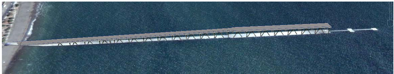
Fig. 3.5 - Aerial view and 3-dimensional representation of the Puerto Puntarenas (courtesy of Google Earth™)
