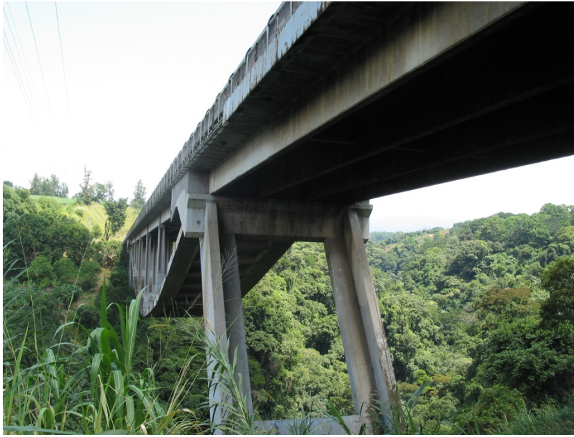
Fig. 4.22 - Pivot and inverted arch, Rafael Iglesias bridge (10.01907° N 84.35651° W).
