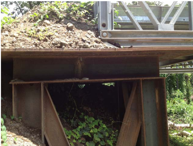
Fig. 4.30 Pin connection between bridge and pile supported abutment consisting of eight H piles.
