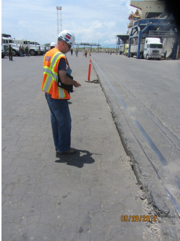
Fig. 3.2 - (a) Earthquake induced settlement in local zones adjacent to the longitudinal beam running parallel to the wharf (9.91197° N 84.72112° W). (b) Settlement was approximately 100 mm (4 inches).
