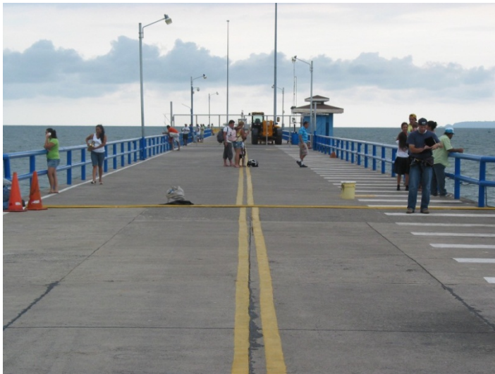
Fig. 3.8 - Lateral offset between pile- and caisson-supported sections of the pier (facing south).
