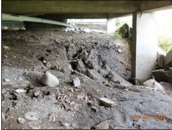
Fig. 2.5 – Foundations Punching through liquefied ground (a) exterior column, north side; (b) interior column, left behind a 60cm crater.
