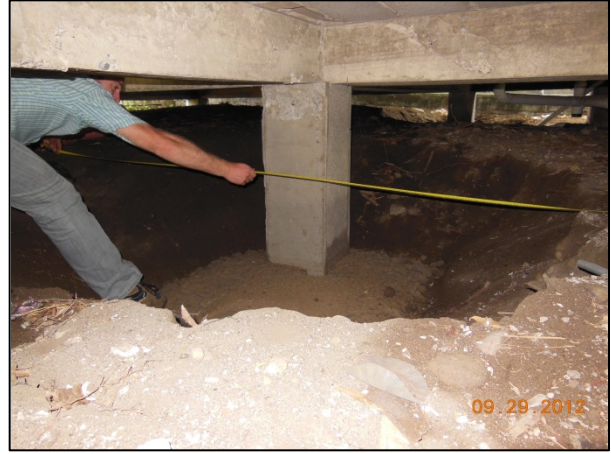
Fig. 2.5 – Foundations Punching through liquefied ground (a) exterior column, north side; (b) interior column, left behind a 60cm crater.
