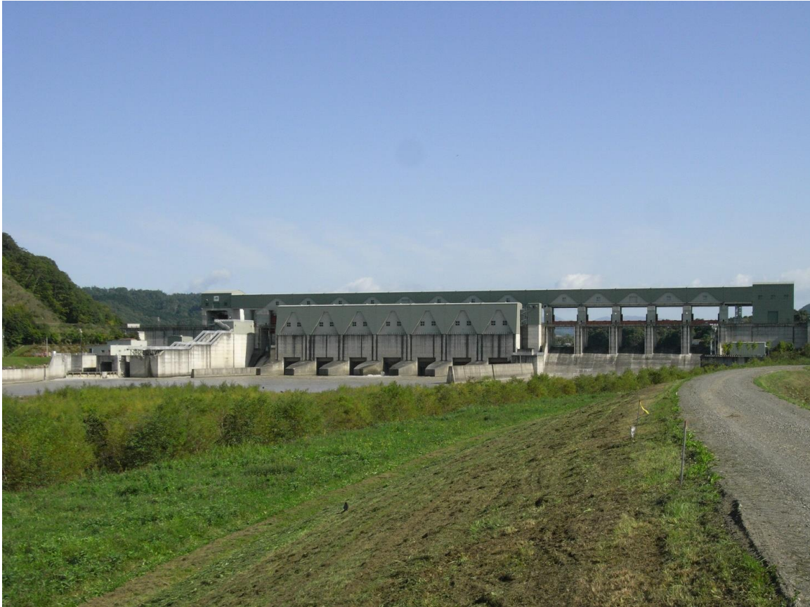
Figure 7-10. Downstream view of the Nibutani Dam from upstream right abutment 42.629302, 142.148654.
