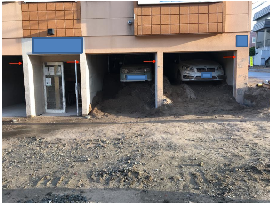
Figure 6-15. Deposition zone of the Satozuka flow-failure slide. Nearly all depositional material was removed prior to reconnaissance (red arrows indicate deposit highpoints). Rafted cars originally in closed garage bays that were damaged and filled with pumice.
