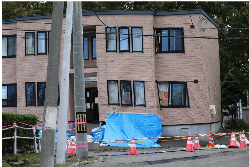
Figure 6-13. Modern apartment building with severe structural damage due to flow liquefaction. 42°59'21.3"N 141°27'22.6E.
