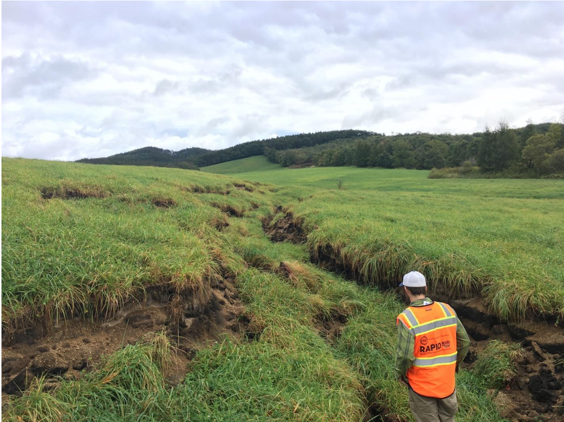
Figure 5-8. 'Low-angle' slide along a \sim 12^\circ slope within pastureland near Atsuma 42.7644^\circ , 141.8778^\circ ]. Sliding plane \sim 1.5 - 2 m in depth, with relatively intact sliding of the failed mass. A smaller failure along the facing hillslope (right of this image) with little permanent deformation was also observed. These landslides were not mapped by the GSI from aerial images.
