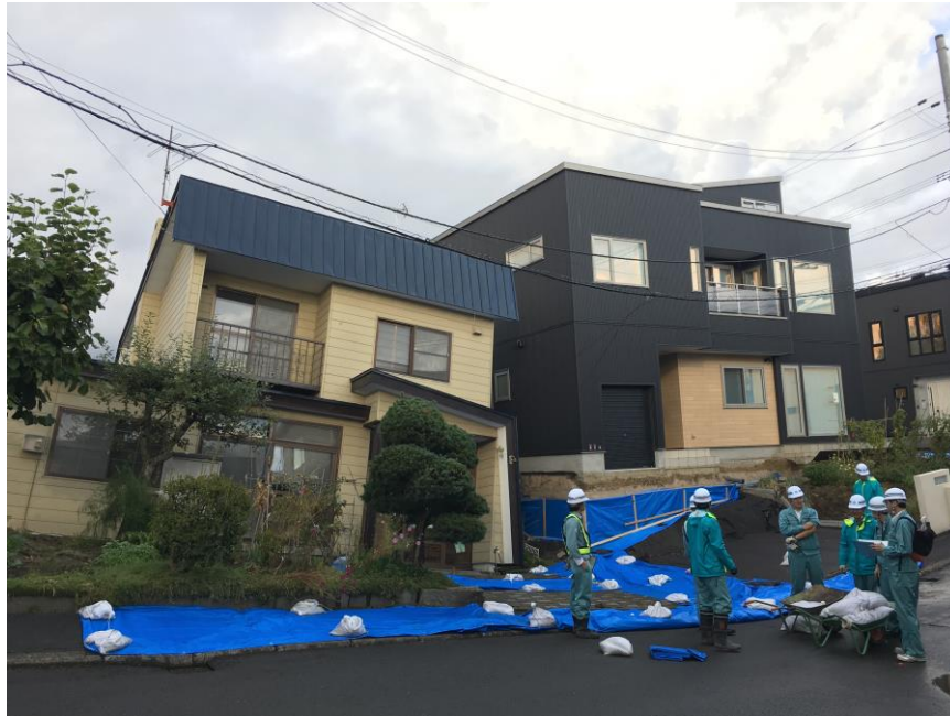
Figure 6-10. Contrasting building ages and foundations showing significantly different performance during the Satozuka flow-failure (main channel of deformation passes through these homes). Left, older mat foundation home with significant rotation and differential settlement. Right, contemporary home on piles, structure stable relative to down dropped surface (~2m).
