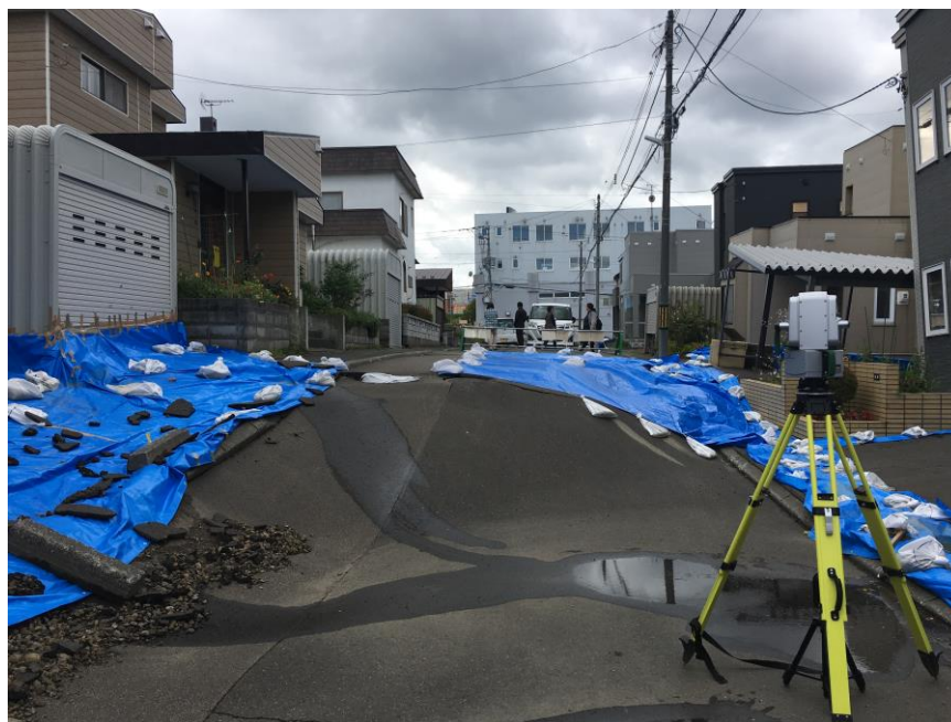
Figure 6-7. Head scarp of the Satozuka flow-failure. The full extent of cracking and potential damages was obscured by tarping and ongoing repairs, vertical offset at this location ~4ft (1.22m).
