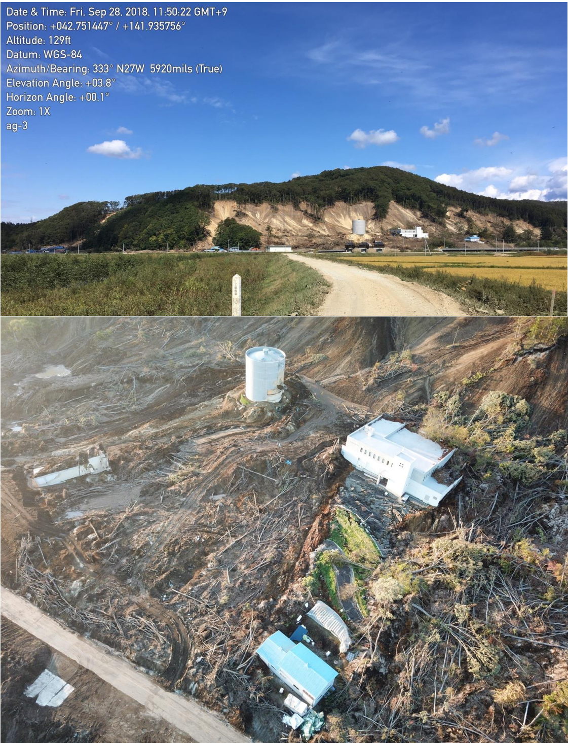
Figure 5-9. Landslide damages at the Tomisato Water Treatment Plant. Top, overview of slope failure. Bottom, UAV-image showing the displaced stairway (left) and protected shadow zone by the surviving main-building. Both water tower and main building are founded on deep piles
