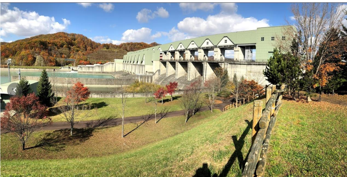
Figure 7-12. Downstream view of Nibutani Dam from left abutment 42.629302, 142.148654.
