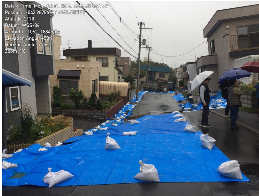
Figure 6-8. Looking down-slide from above the head scarp. Tilt of structure at end of street typical.
