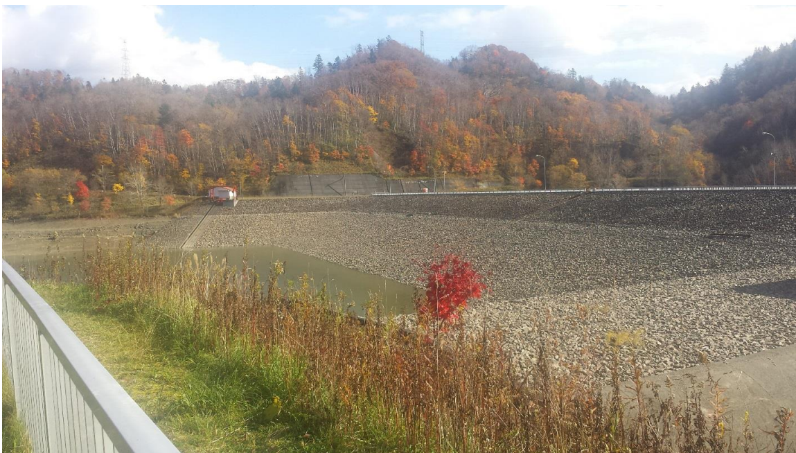
Figure 7-6. Upstream view of Hobetsu Dam from right abutment. 42.885648, 142.179387,
