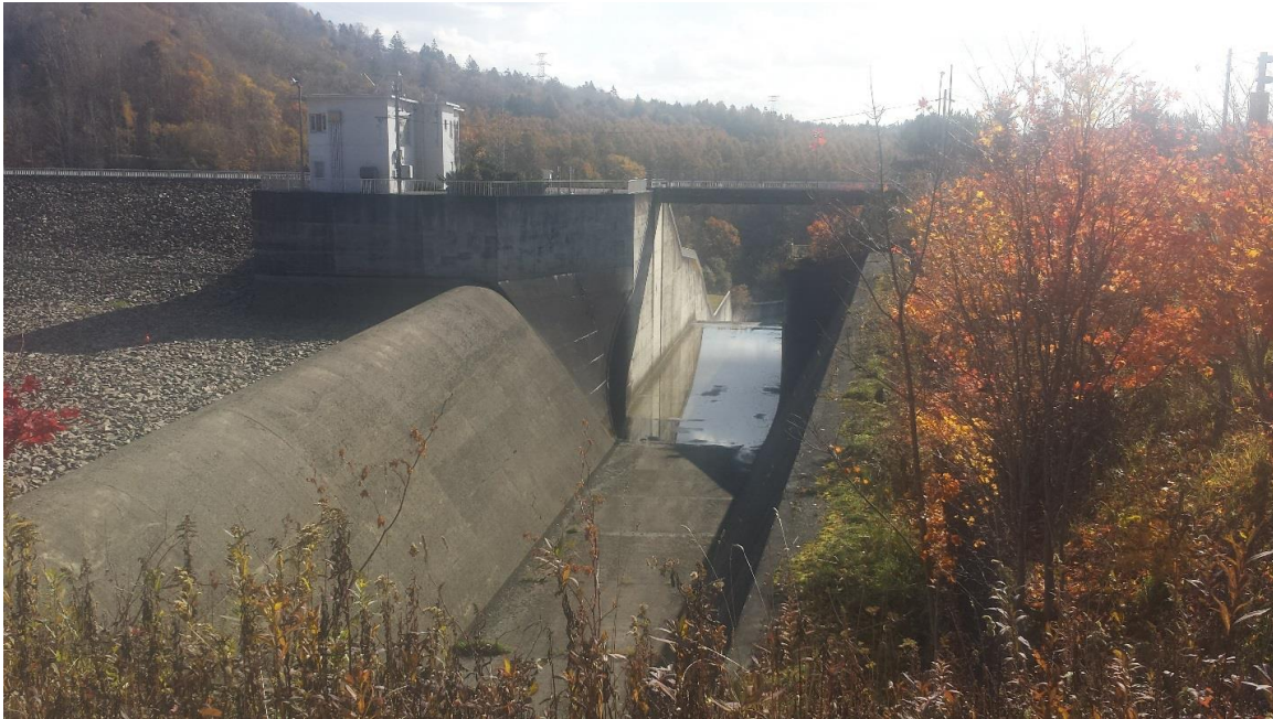
Figure 7-7. Hobetsu Dam Spillway.
