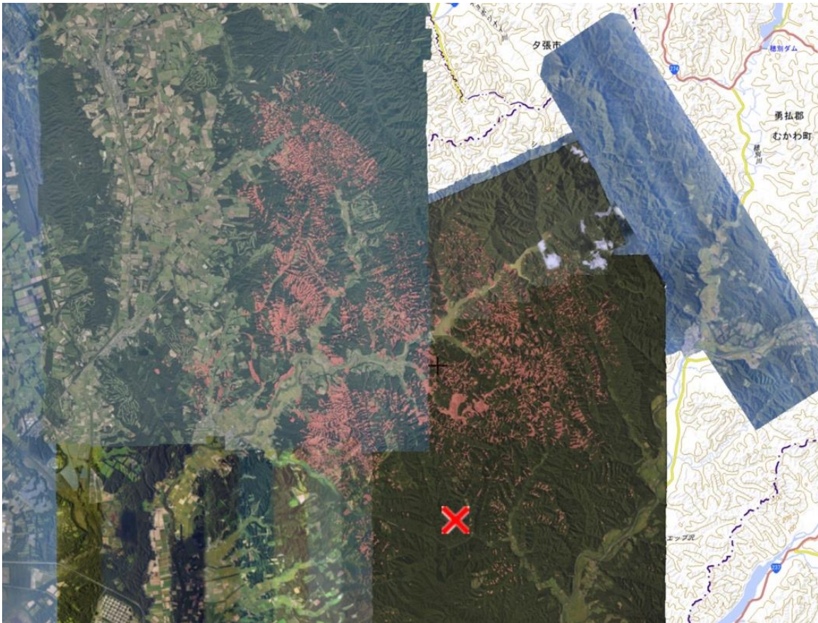
Figure 5-1. Post-earthquake aerial photos collected Sept 6 – 11 and coseismic landslides mapped by the Japanese Geographical Survey Institute ( http://www.gsi.go.jp/BOUSAI/H30-hokkaidoiburi-east-earthquake-index.html#10 , last accessed Oct, 2018). M6.6 epicenter [GSI] marked by red 'X', landslides shown as pink polygons
