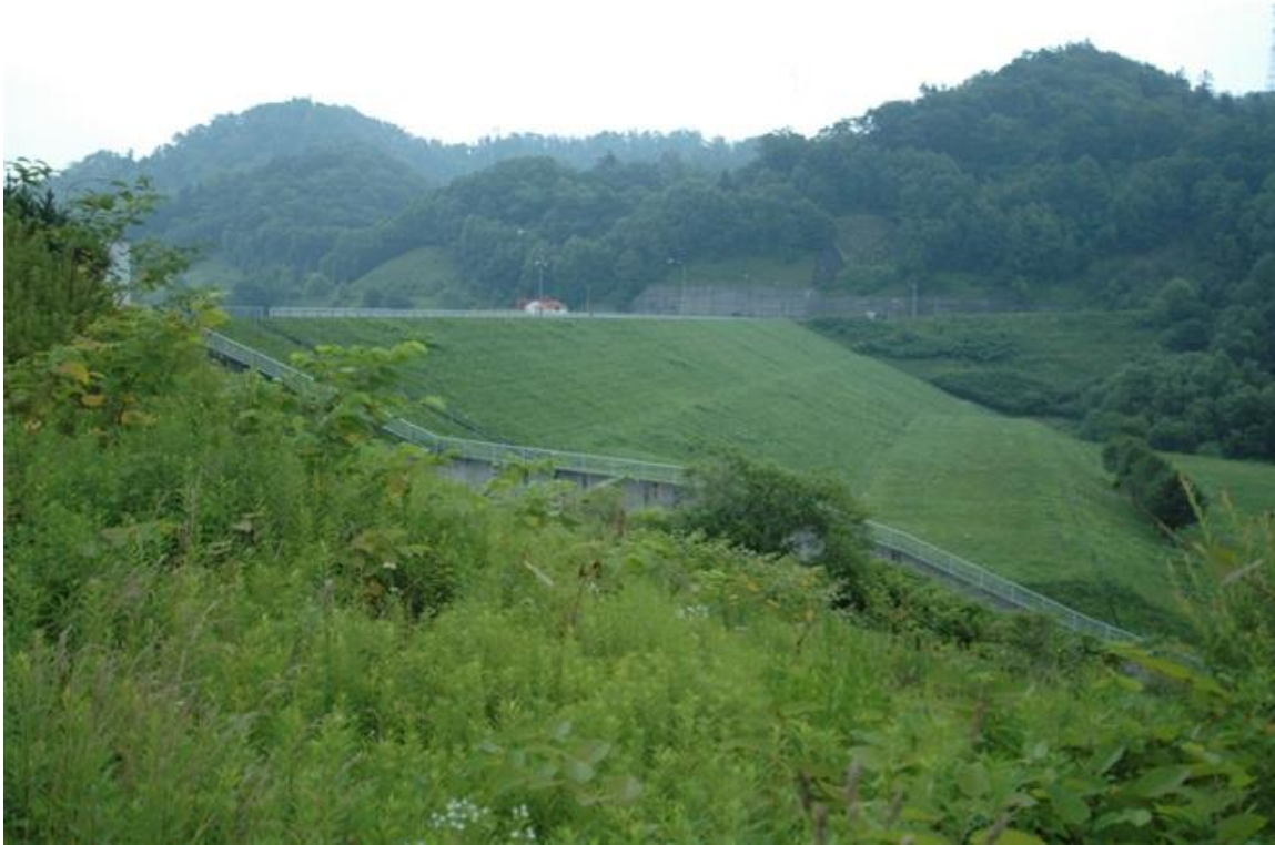
Figure 7-3. Downstream view of Hobetsu Dam from right abutment (Image from the Japan Dam Foundation http://damnet.or.jp/cgi-bin/binran/enPAL.cgi?idm=9645 ). 42.885648, 142.179387,
