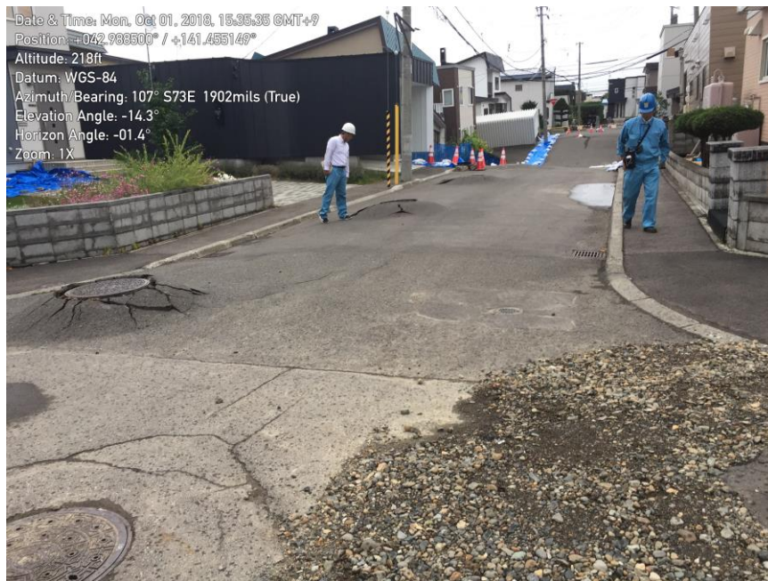
Figure 6-9. Stable manhole covers revealing the broader vertical settlement of Satozuka outside the more intense channelized material evacuation. Local utilities were placed on the underlying soils at depths of up to 10m and did not show vertical displacements during liquefaction.
