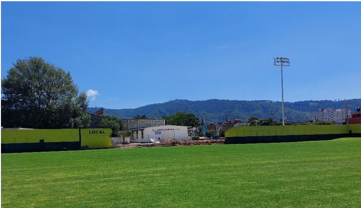
Figure 27. Partial collapse and cracking of perimeter wall of local stadium, Ciudad Guzman, Jalisco. Waypoint Station 38 (Coordinates: 19.702541°, -103.471109°)
