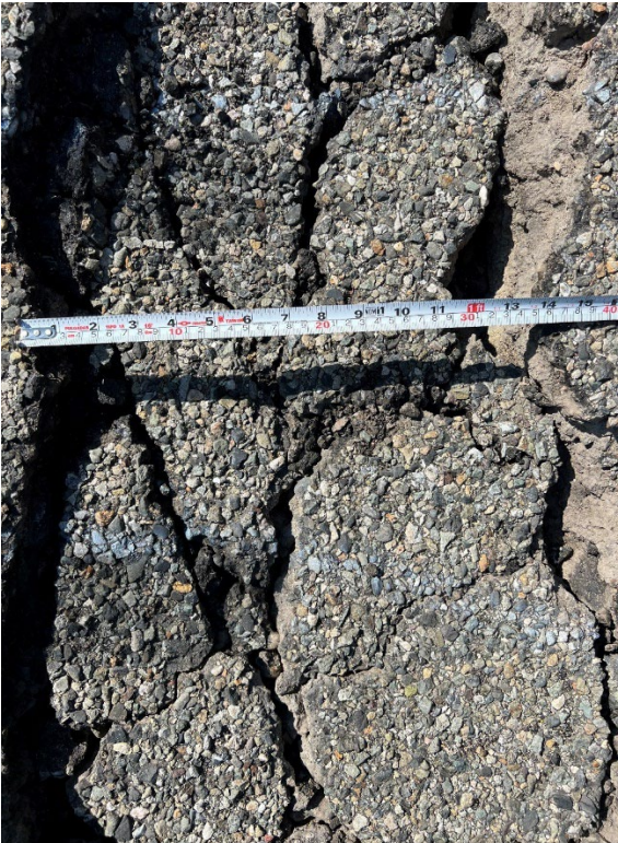
Figure 28b. Severe longitudinal cracking on road due to lateral expansion, Maruata, Michoacan. Waypoint Station 27 (Coordinates: 18.282195°, -103.358294°)
