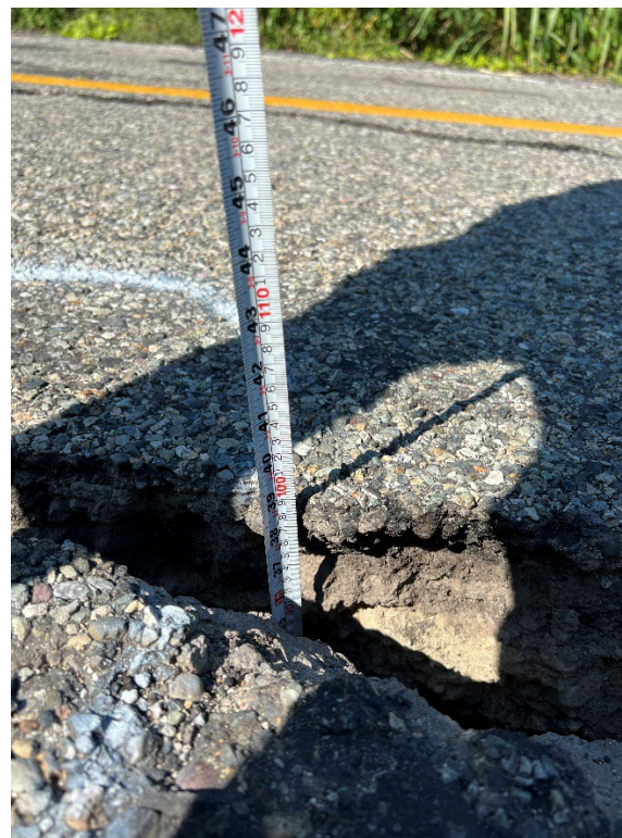
Figure 28b. Severe longitudinal cracking on road due to lateral expansion, Maruata, Michoacan. Waypoint Station 27 (Coordinates: 18.282195°, -103.358294°)
