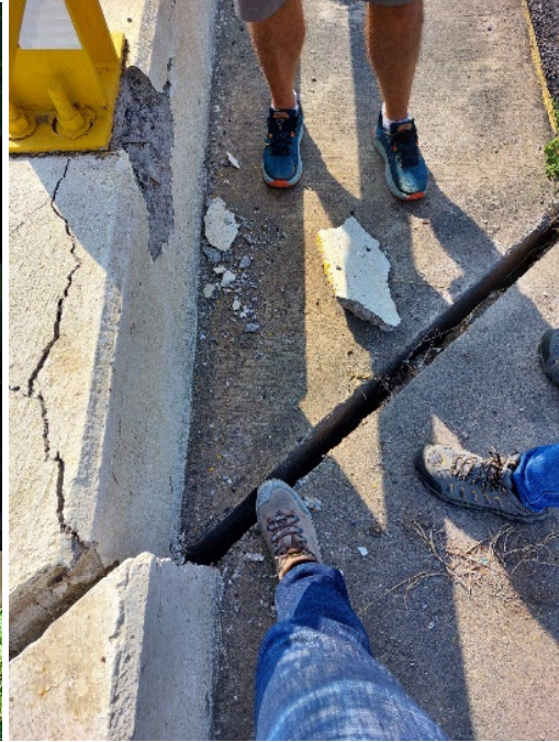
Figure 32. Lateral displacements of decks and damage in pier caps of bridge, Arturo Noriega Pizano, Colima. Waypoint Station 17 (Coordinates: 18.72438°, -103.722248°)
