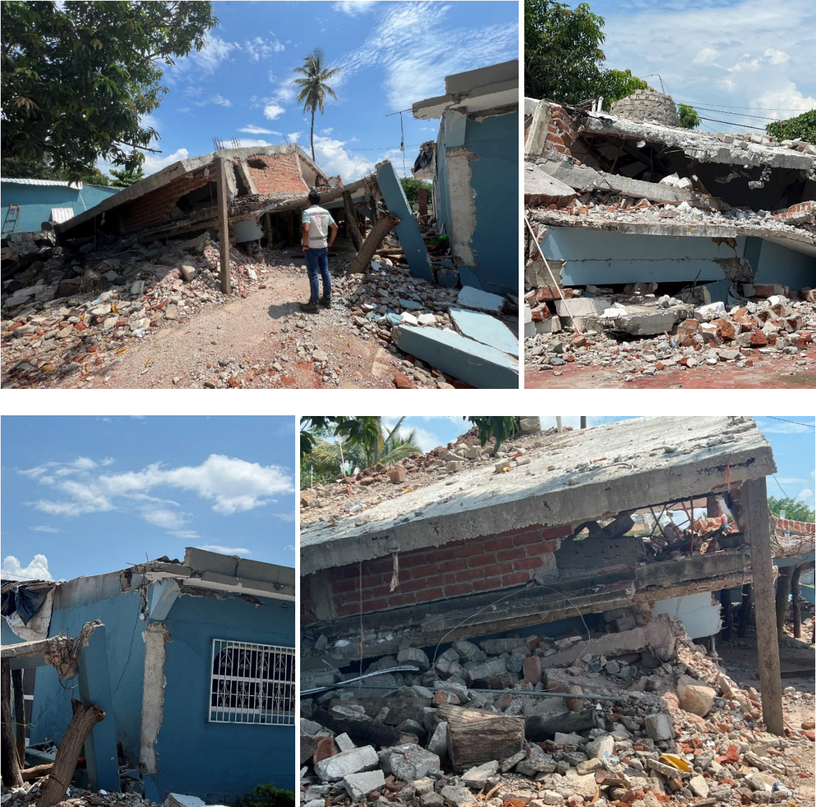
Figure 19. Total collapse of a two-story house with soft first floor, Coahuayana, Michoacan, Waypoint Station 22 (Coordinates: 18.728643°, -103.687277°)
