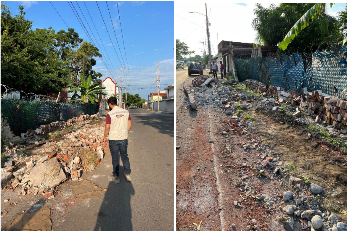
Figure 14. Collapse of perimeter wall of automobile workshop, Tecoman, Colima, Waypoint Station 12 (Coordinates: 18.918219°, -103.870195°)
