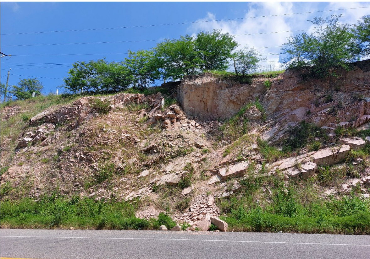
Figure 37. Rock wedge failure on cutting slope along the road, La Cumbre, Jalisco. Waypoint Station 2 (Coordinates: 19.860358°, -105.323112°)
