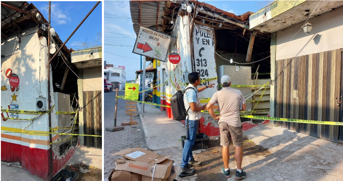
Figure 15. Collapse of local grocery store, Tecoman, Colima Waypoint Station 13 (Coordinates: 18.911143°, -103.871476°)
