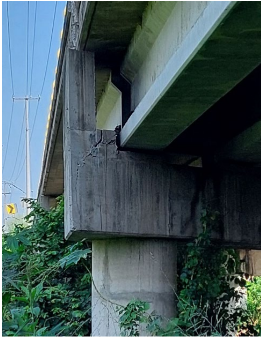
Figure 32. Lateral displacements of decks and damage in pier caps of bridge, Arturo Noriega Pizano, Colima. Waypoint Station 17 (Coordinates: 18.72438°, -103.722248°)
