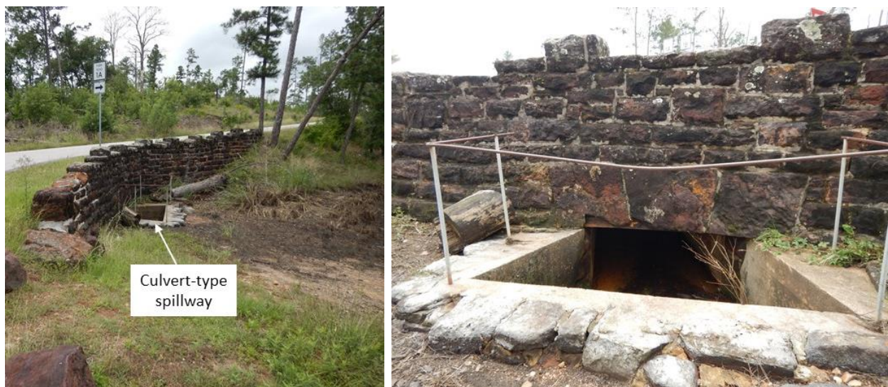
Figure 18. Culvert-type spillway on west abutment
