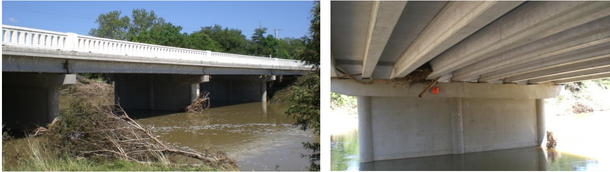
Figure 10. LP 163 Bridge relatively undamaged
