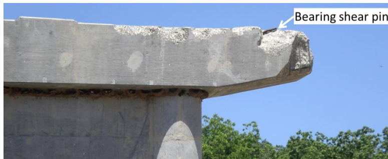
Figure 4. Damage to wall piers
