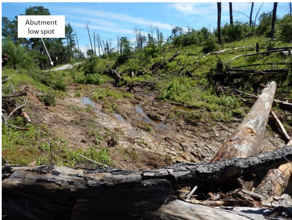
Figure 19. View of erosional channel just downstream from the low spot in the east abutment.
