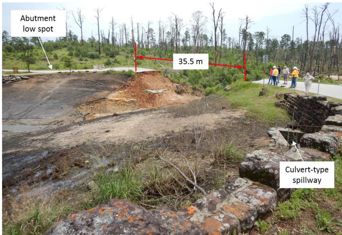
Figure 14. View of dam failure from upstream of the west abutment.
