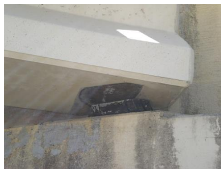
Figure 9. Shifting of girders at west abutment
