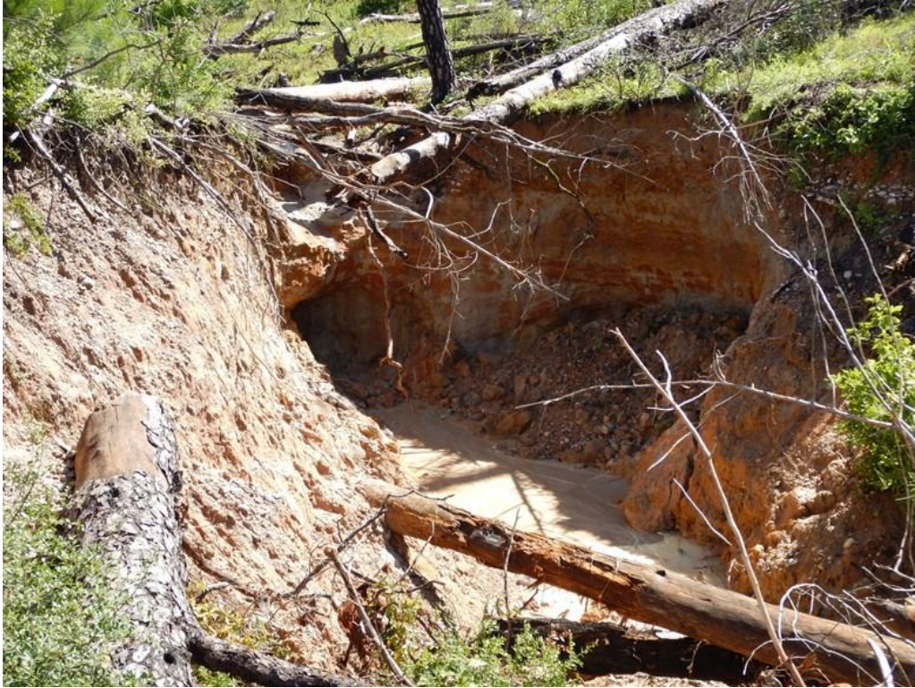
Figure 20. View of erosional crevasse about 70 m downstream from the low spot on the east abutment.
