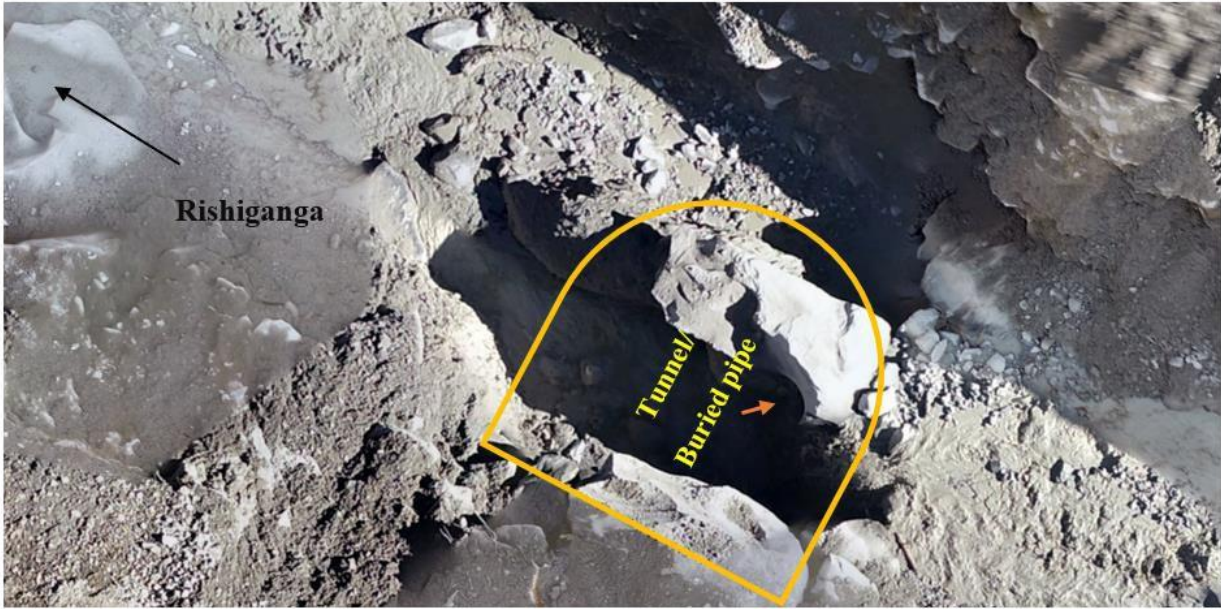
Figure 3.20 Buried pipe/tunnel structure@ 30°28'56.39"N 79°41'49.20" E
