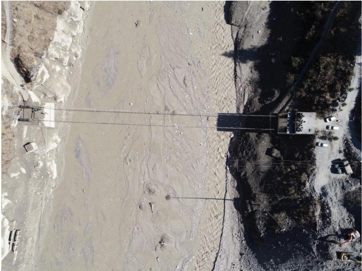
Figure 3.41: Close-up of collapsed bridge-1 U/s of Tapovan Barrage site(dated 11/2/21)@ 30°29'34.41"N 79°37'47.92"E
