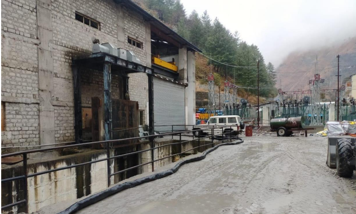
Figure 3.3 Inside view of the powerhouse(Photo courtesy: Sikim, native) @30°29'5.11"N 79°41'40.46" E
