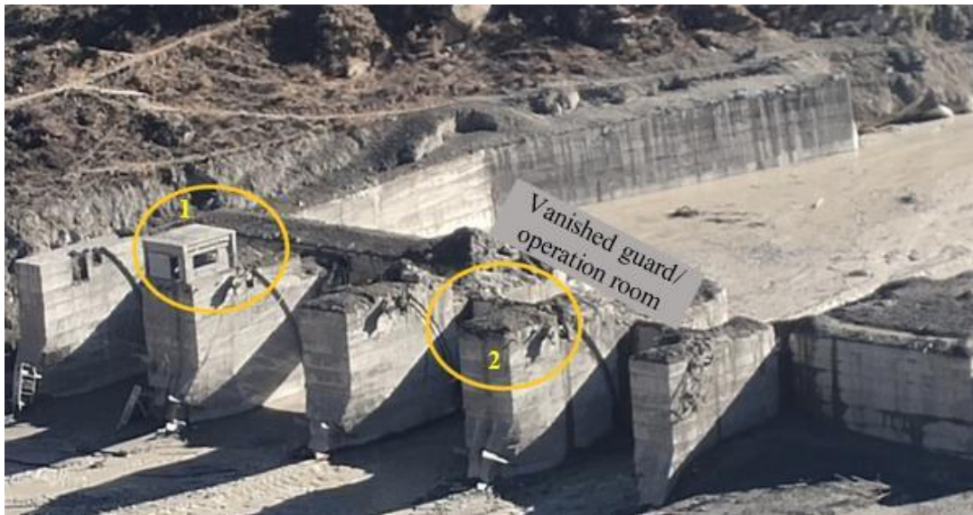
Figure 3.40 Yellow solid line circles indicating the guardrooms a) snapshot taken from a video presents the two guard rooms just before the event (Source: Sikim (native), February 7 th , 2021) b) sustained and washed away guard rooms (Source: DSLR, February 11 th , 2021) @ 30°29'35.89"N 79°37'41.67"E (Dated:11/02/2021)
