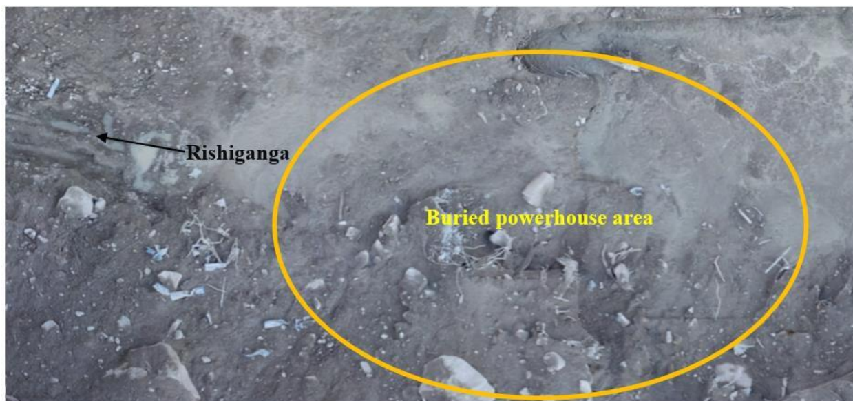
Figure 3.22 Buried powerhouse region @30°29'5.11"N 79°41'40.46" E (Dated: 11/02/2021)
