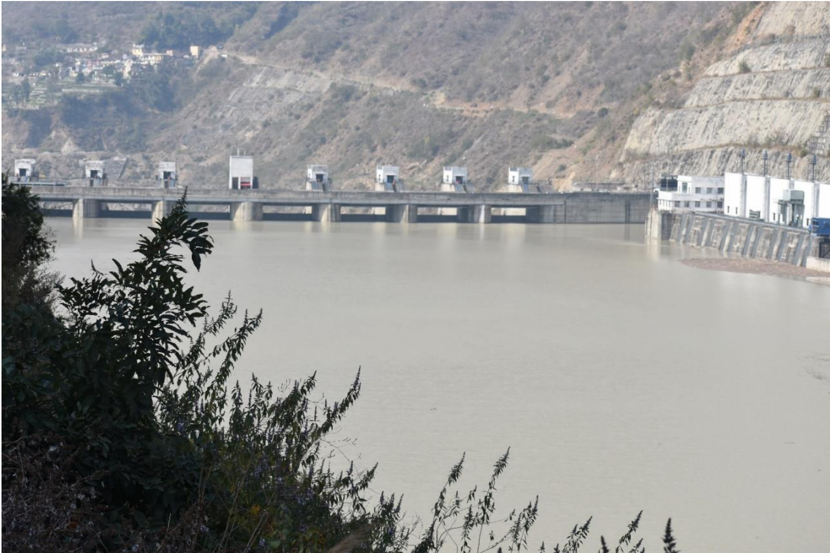
Figure 1.4 Srinagar Dam with turbid water (Dated 11/02/2021) (30°14'31.28"N, 78°49'20.41"E)
