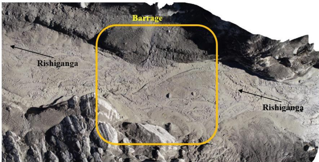
Figure 3.17 Barrage region, 30°28'42.68"N 79°42'0.50" E (Dated: 11/2/2021)
