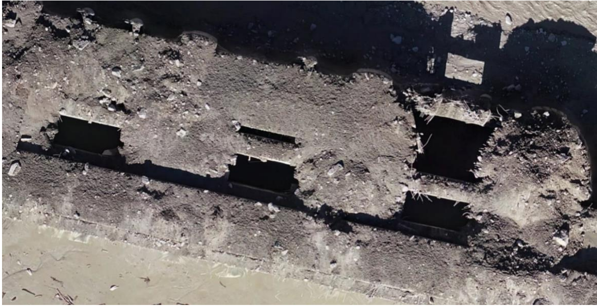
Figure 3.35 Close-up view of the Intake structure@ 30°29'35.89"N 79°37'41.67"E (Dated:11/02/2021)
