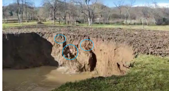
b) Upper portions of the block are falling.
