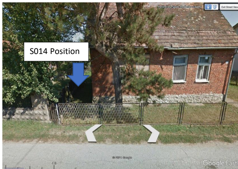
Figure 6.30 Street view of the house and S014 position (45.282822N, 16.429389E).
