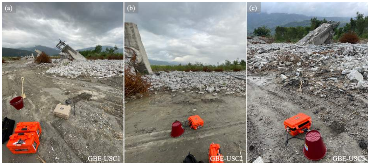
Figure 2.8. Photo of sensor setup at Gaoliao bridge (Eastern end). (a) GBE-USC1; (b) GBE-USC2; (c) GBE-USC3.
