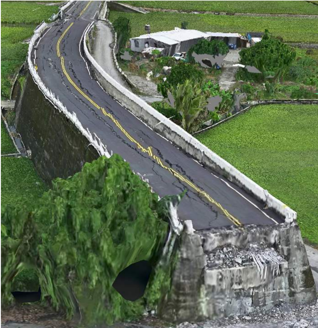
Figure 5.39. Drone view of the east abutment looking east (approx. 23.38522° 121.34690°)
