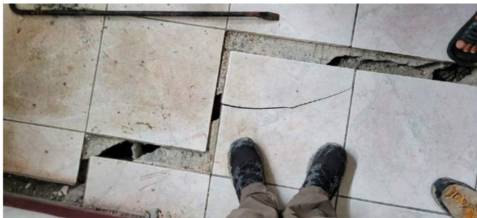
Figure 4.14: Partial collapse of URM structure along the LVF. Rupture propagated beneath the house. Lat: 23° 10' 26.201999", Lon: 121° 14' 54.605400"
