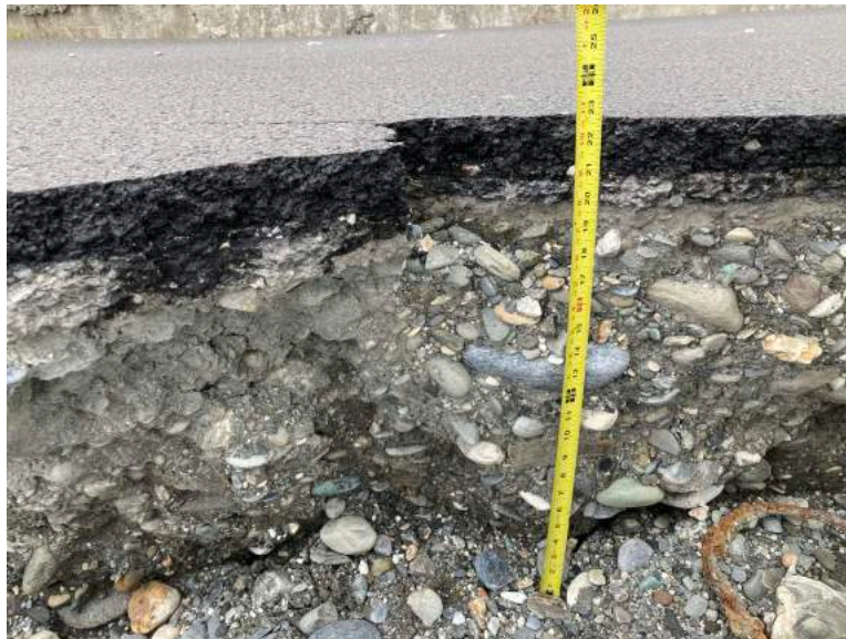
Figure 5.44. Typical profile of backfilled soils (23.38509° 121.34773°)
