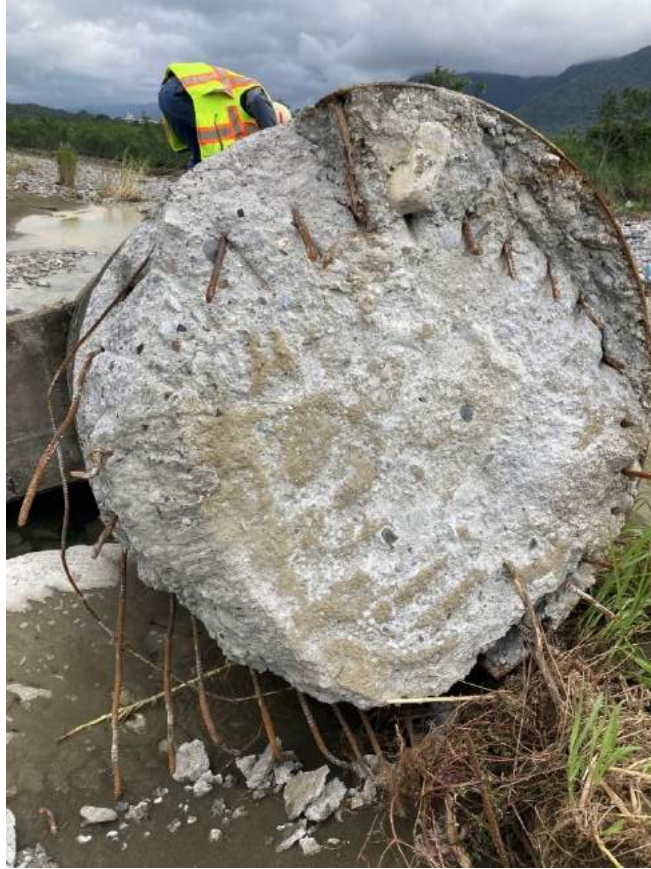
Figure 5.13. View of a failed pier with irregular longitudinal rebar spacing. Same pier as and concrete pad as Figure 5.14. (23.217653° 21.270928°)
