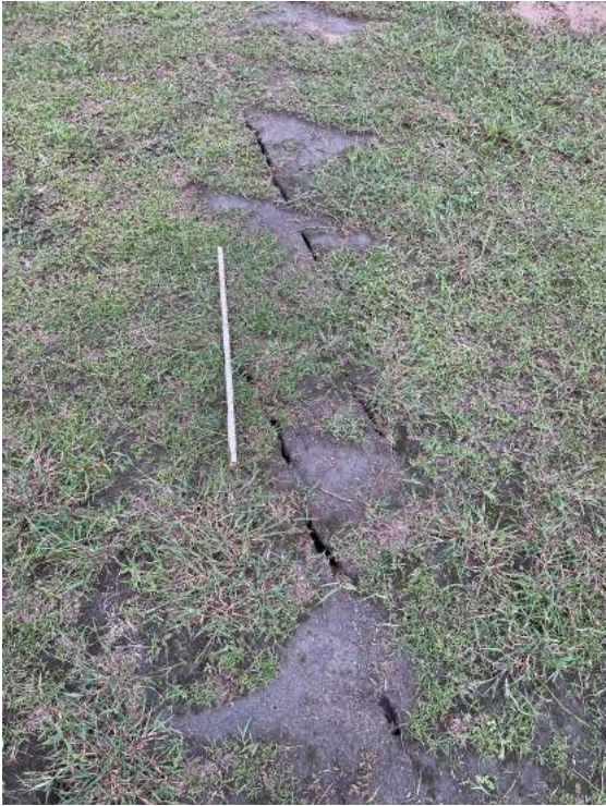
Figure 4.40: En-echelon tension cracks with apparent ejected sands at the Yuli High School athletic field. Lat: 23° 20' 31.165800", Lon: 121° 19' 11.031959"
