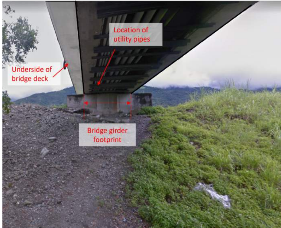
Figure 5.8. Looking west at the 2 nd pier from the east abutment prior to the earthquake. Note the location of the utility pipes on the pier cap. Photo from Google Street View from 2012 (near 23.21457^\circ 121.27268^\circ )
