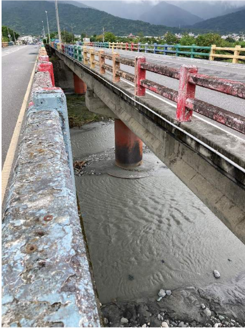
Figure 5.28. View of the substructure of the North Yuli bridge. Similar structural components on the south bridge. (23.32320° 121.32780°)
