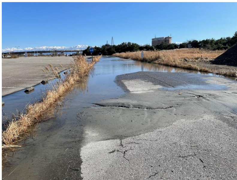
Figure 5.9. After fountain caused by liquefaction (Imizu City, Toyama Prefecture). Lat: 36.78097°, Lon: 137.09959°
