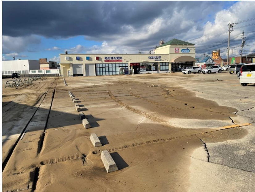
Figure 5.12. Liquefaction damage in old river channel (Takaoka City, Toyama Prefecture). Lat: 36.75944°, Lon: 137.00375°
