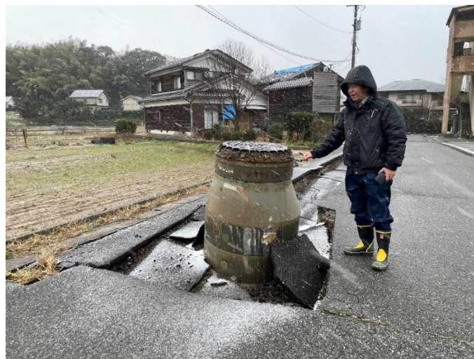
Figure 5.5. Liquefaction causes manholes lifting phenomenon (Wajima City, Ishikawa Prefecture). Lat: 37.39358°, Lon: 136.91582°
