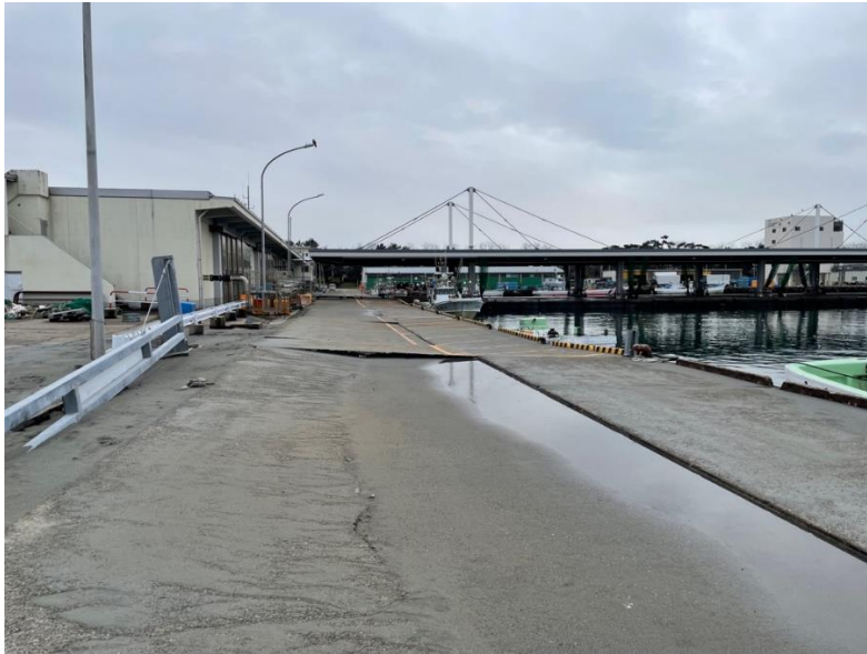
Figure 5.10. Damage to Shinminato Fishing Port due to liquefaction (Imizu City, Toyama Prefecture). Lat: 36.78250°, Lon: 137.09720°
