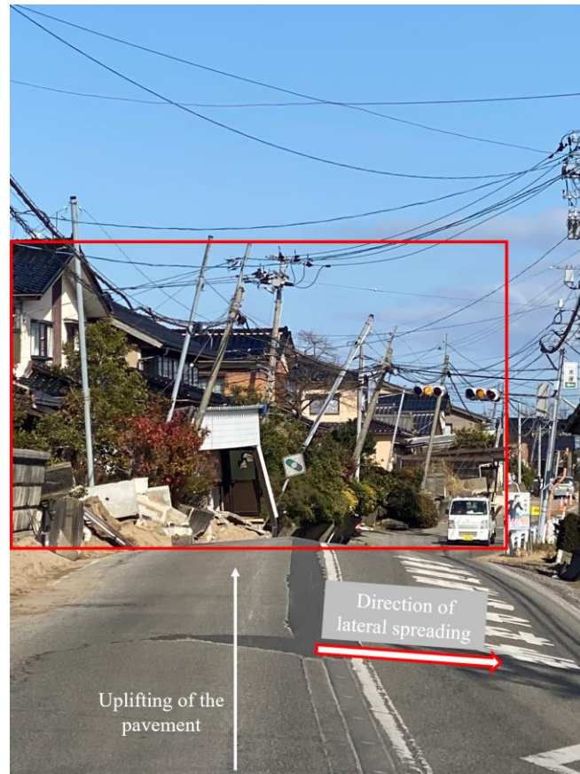
Figure 5.23. Significant uplift of the left side of Prefectural Road 8 with tilted poles clearly visible. Lat: 36°40'41.64", Lon: 136°40'4.80"
