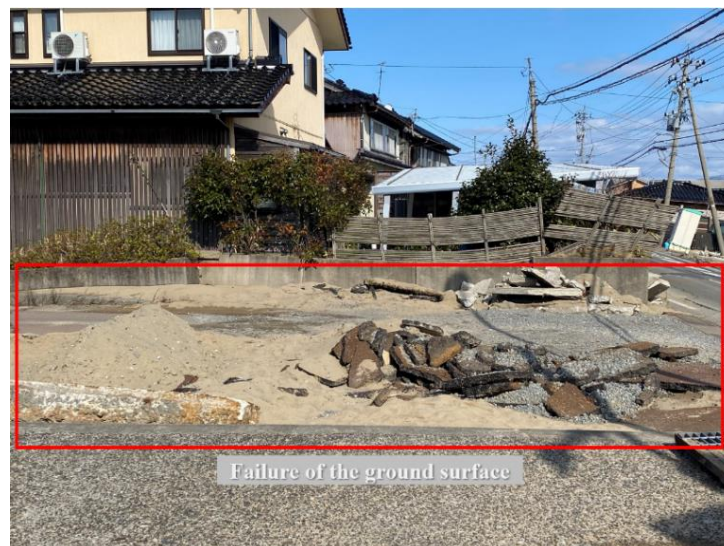
Figure 5.22. Settlement of the ground surface adjacent to the Prefectural Road 8. Lat: 36^{\circ}40'41.70'' , Lon: 136^{\circ}40'4.36''
