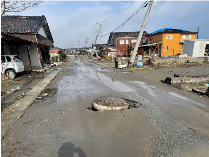
Figure 5.4. A utility pole leaning toward the sea (Suzu City, Ishikawa Prefecture). Lat: 37.39912°, Lon: 137.24358°
