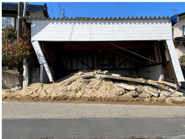
Figure 5.26. Collapse of the parking shed. Lat: 36°40'43.62", Lon: 136°40'6.50"
