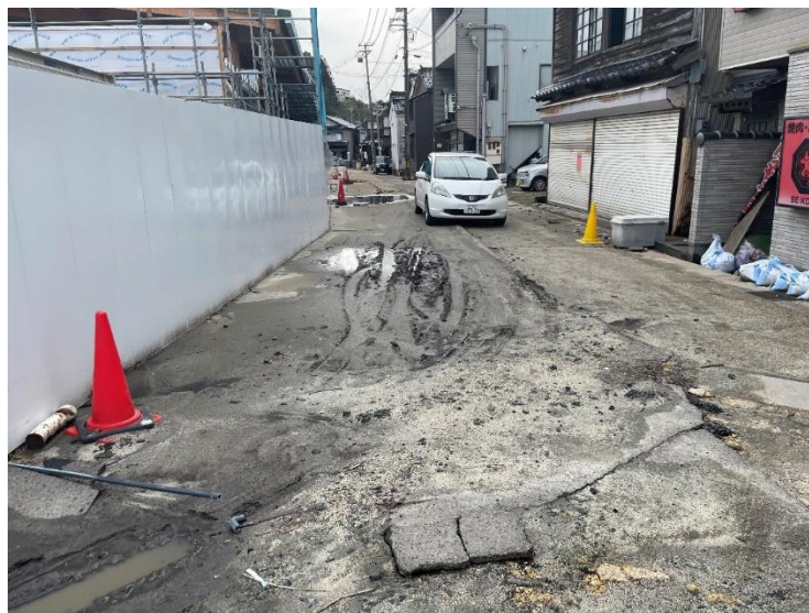
Figure 5.7. Liquefaction around private houses near Uitsu Port(Noto Town, Ishikawa Prefecture). Lat: 37.30706°, Lon: 137.15016°
