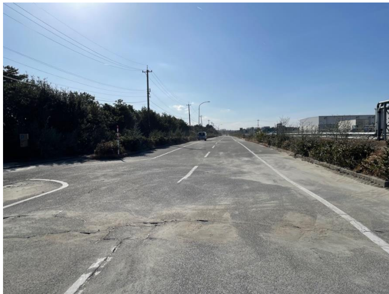
Figure 5.11. Liquefaction damage on a road in Toyama Fushiki Port (Takaoka City, Toyama Prefecture). Lat: 36.80089°, Lon: 137.06691°
