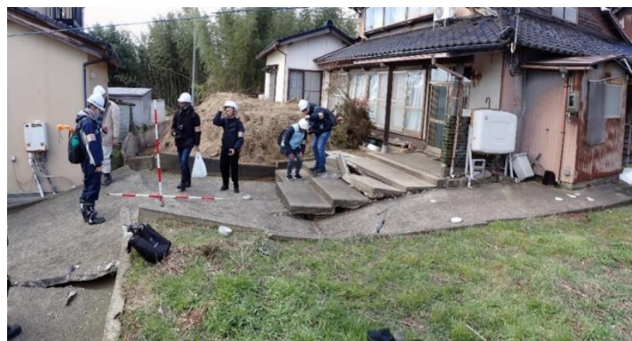
Figure 5.17. Damage in the Ohsaki area of Kahoku City (Uplift of road and lateral movement of houses). Lat: 36°42'23.62", Lon: 136°41'27.08"
