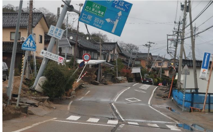
Figure 10.6. Compression and upliftment of prefectural road no. 8 (Near Nishi Araya area)
