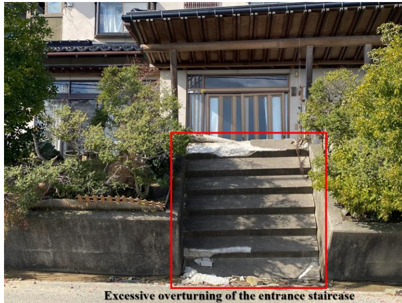
Figure 5.25. Significant tilting of the entrance staircase towards Prefectural Road 8. Lat: 36°40'43.99", Lon: 136°40'6.88"
