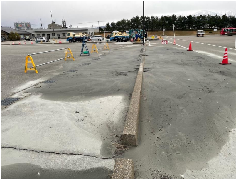
Figure 5.15. Sediment eruption at Uozu Fishing Port (Uozu City, Toyama Prefecture). Lat: 36.82440°, Lon: 137.39305°
