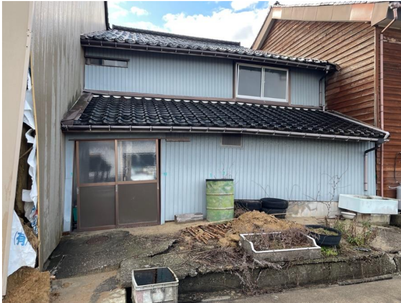
Figure 5.14. A house that deflects from side to side due to immobile subsidence caused by liquefaction (Himi City, Toyama Prefecture). Lat: 36.86425°, Lon: 136.98546°
