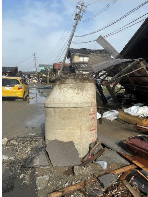
Figure 5.2. Liquefaction causes manholes lifting phenomenon (Suzu City, Ishikawa Prefecture). Lat: 37.40073°, Lon: 137.24304°
