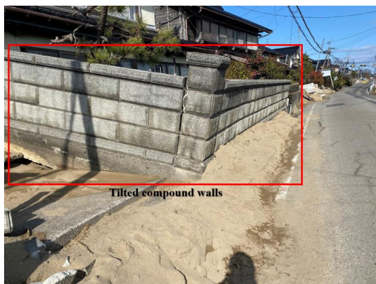
Figure 5.24. Close-up view of the building's compound wall tilted towards Prefectural Road 8. Lat: 36°40'42.03", Lon: 136°40'5.18"
