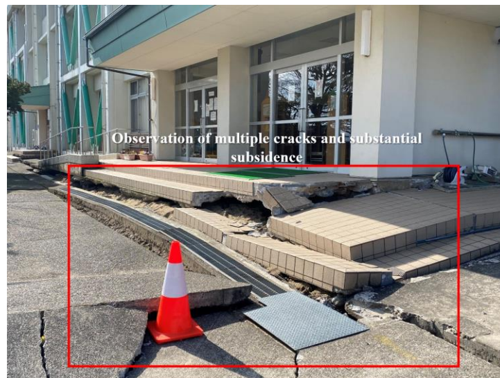
Figure 5.27. Damage to the entrance of Nishi Araya elementary school. Lat: 36°40'42.25", Lon: 136°40'3.53"
