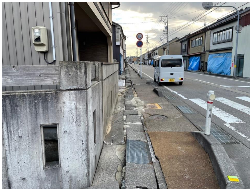
Figure 5.13. Damage to gutters due to liquefaction (Himi City, Toyama Prefecture). Lat: 36.87181°, Lon: 136.98319°
