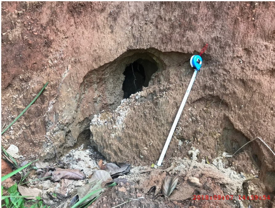
Figure A-21: Another view of the pipping @ 10.0088132° N 77.0257597° E
