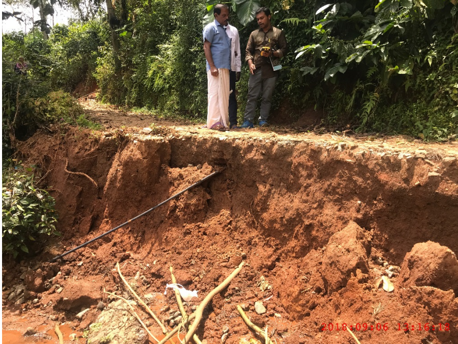
Figure A-5: Landslide scarp @ 9.7968694° N 77.0675658° E
