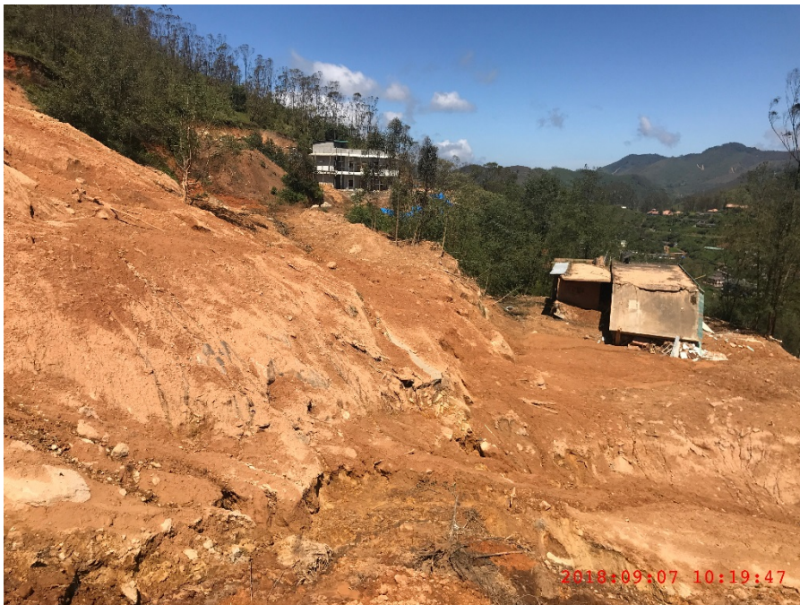
Figure A-17: Munnar college landslide showing the destroyed college building @ 10.0822577° N 77.0734317° E
