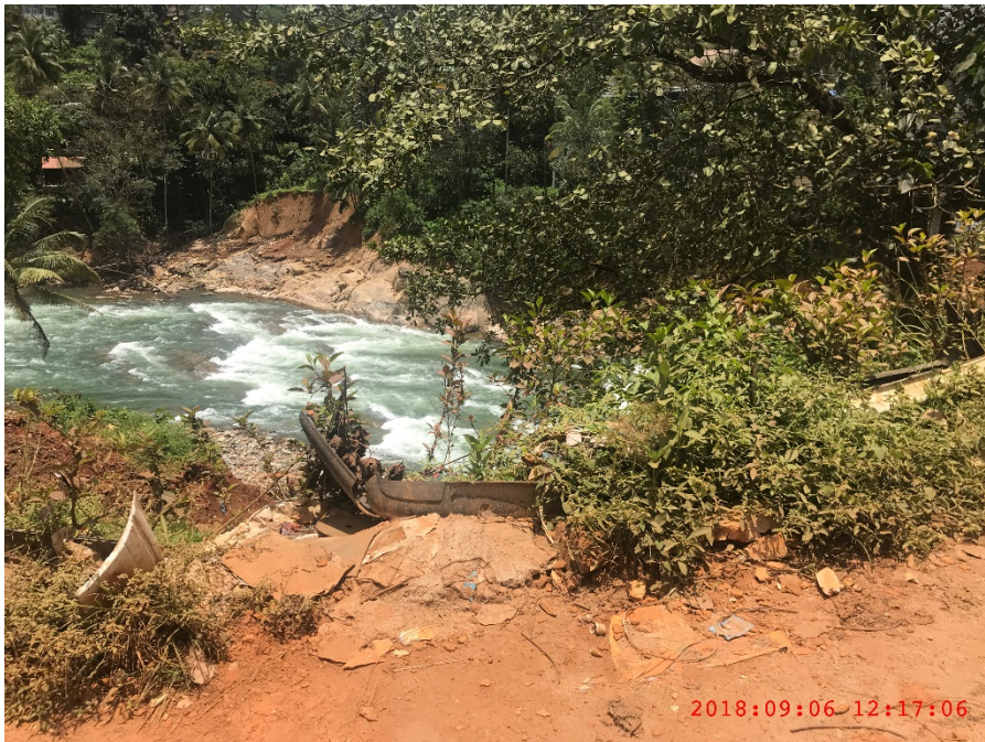
Figure B-3: River erosion @ 9.8585518° N 76.9639427° E
