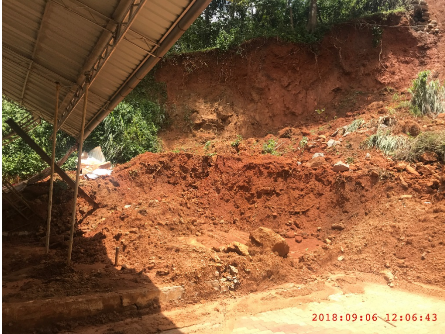
Figure A-3: Landslide near a gas station @ 9.8549653^{\circ} N 76.9619187^{\circ} E
