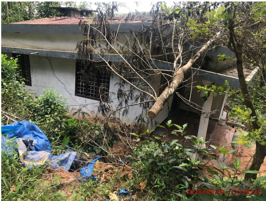
Figure A-6: House destroyed in the landslide @ 9.7968694° N 77.0675658° E
