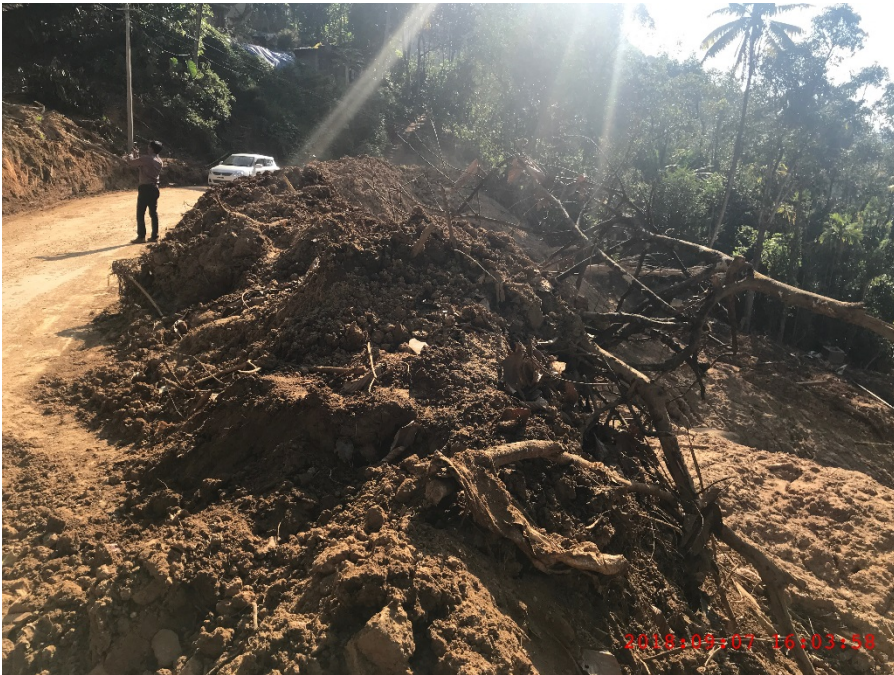
Figure A-26: Panniyarkutty landslide @ 9.9749966° N 77.0429146° E
