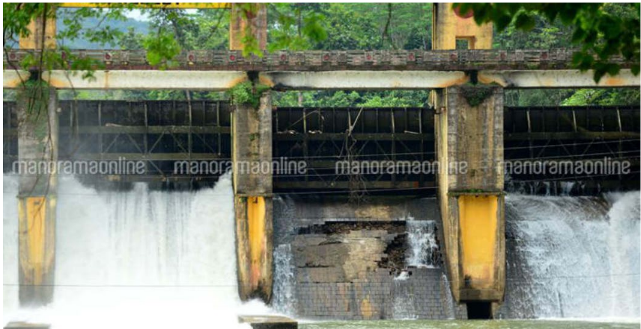
Figure 3.11: Different view of the damage to the downstream surface of shutter-2 at Maniyar Dam (Source: manoramaonline.com).
