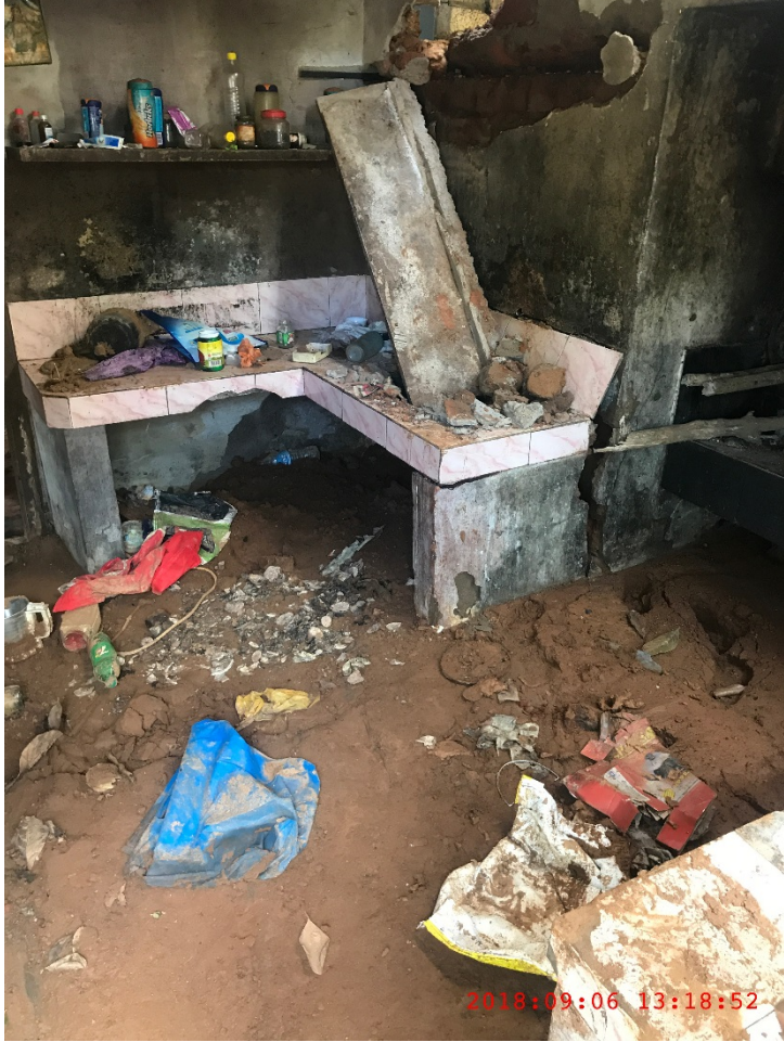
Figure A-7: Interior of a house destroyed in landslide and debris flow @ 9.7966953° N 77.0678775° E
