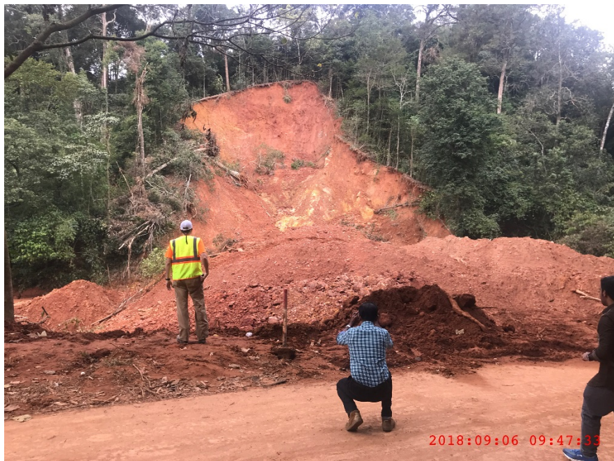
Figure A-2: Landslide that blocked the road @ 9.8263274° N 76.9197930° E
