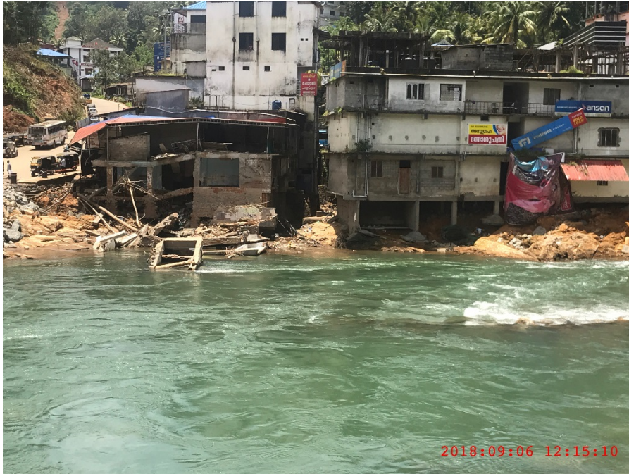
Figure B-2: River erosion @ 9.8575868° N 76.9636007° E
