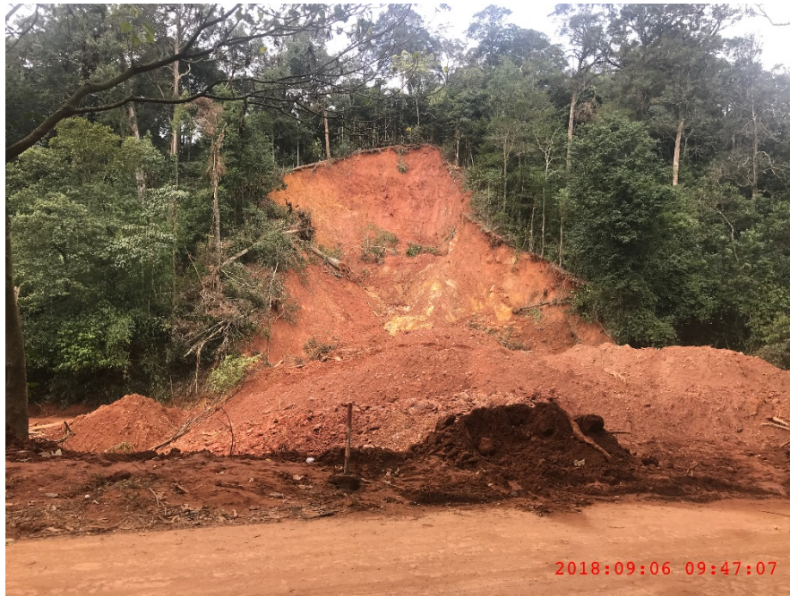
Figure A-1: Landslide that blocked the road @ 9.8263274° N 76.9197930° E
