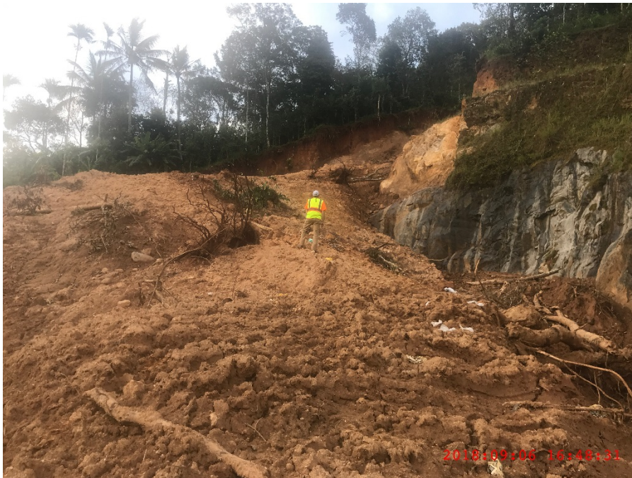
Figure A-14: Major landslide that buried a two storey building that was in construction @ 9.7644641 o N 77.1096940 o E
