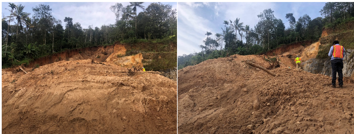
Figure 2.9: Photographs of the Kattappana Landslide located at (notice Dr. Coffman within the slide extents preparing to take photographs, Latitude=9.79655°, Longitude=77.0685°).
