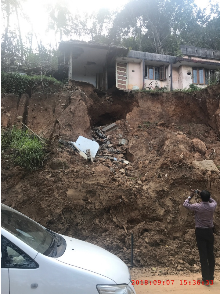
Figure A-24: Another view of the piping channel @ 9.9756741^{\circ} N 77.0216901^{\circ} E
