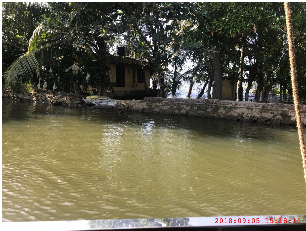
Figure 5.4: A minor bund failure @ 9.5032131 0 N 76.3768638 0 E.
