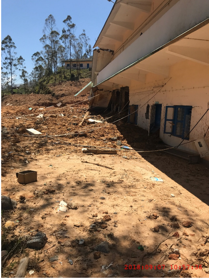
Figure A-18: Destroyed Munnar College building @ 10.0826962^{\circ} N 77.0726538^{\circ} E
