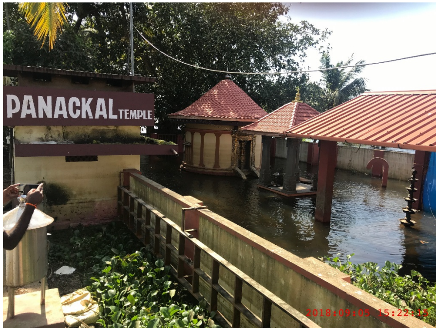
Figure 5.6: Flooded temple complex from the bund failure @ 9.5033596 0 N 76.3771085 0 E
