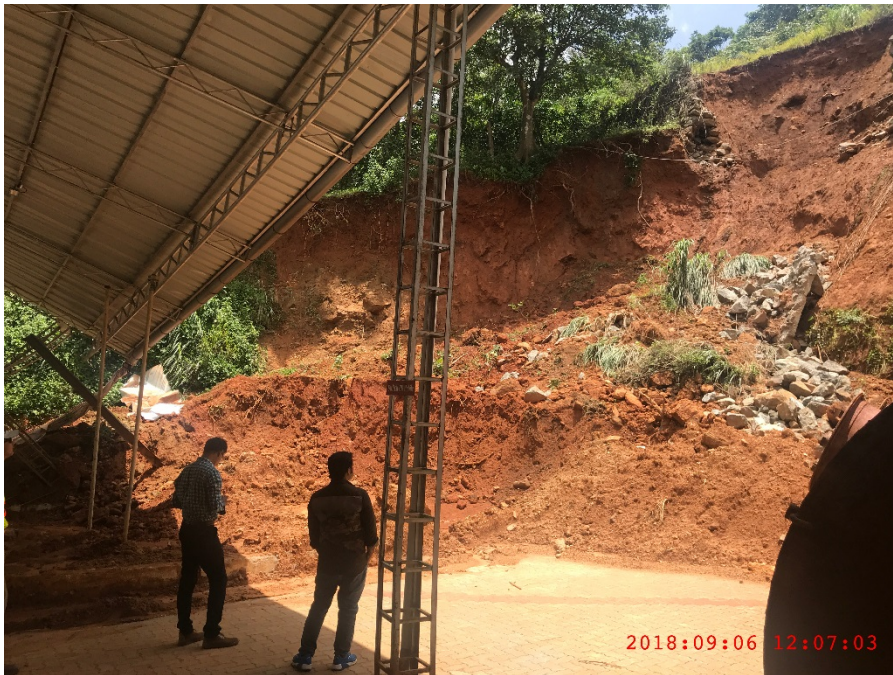
Figure A-4: Landslide near a gas station @ 9.8549653^{\circ} N 76.9619187^{\circ} E
