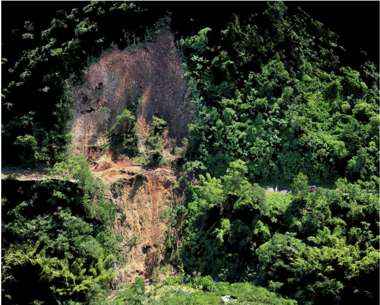
Figure 23: Photo mosaic of over 250 aerial photographs of a large rotational slump landslide along PR-409 in Las Marías (18.2061, -66.94397). Vehicles at the right center of the photo for scale.
