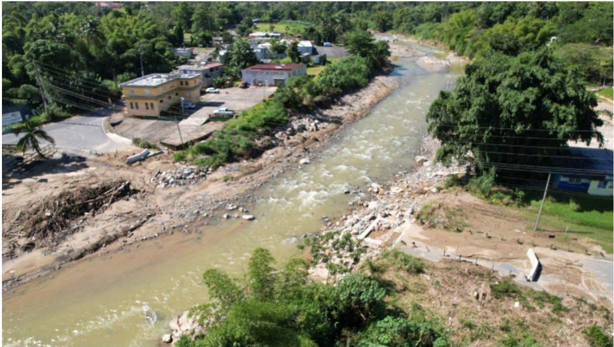
Figure 30: Aerial photograph looking south at the location where a temporary bridge structure across the Río Grande de Arecibo in Utuado was washed away during Hurricane Fiona. Video of bridge failure here: https://www.telemundopr.com/noticias/puerto-rico/colapsa-puente-en-utuado/2394672/
