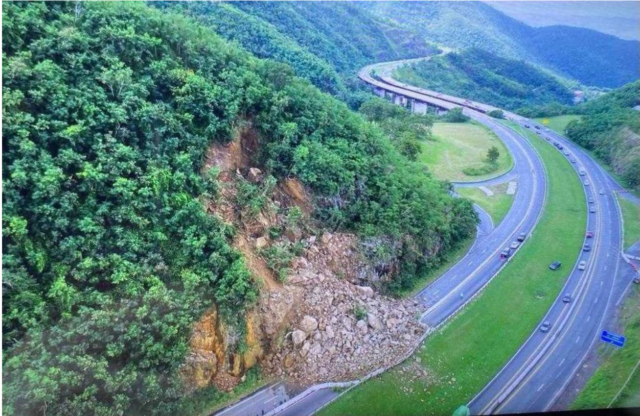
Figure 21: Rockfall along PR-52 in Salinas, near the border with Cayey (18.0711, -66.2172). Photo is from https://www.primerahora.com/noticias/puerto-rico/fotogalerias/fotos-graves-danos-a-carreteras-a-causa-de-las-fuertes-lluvias
