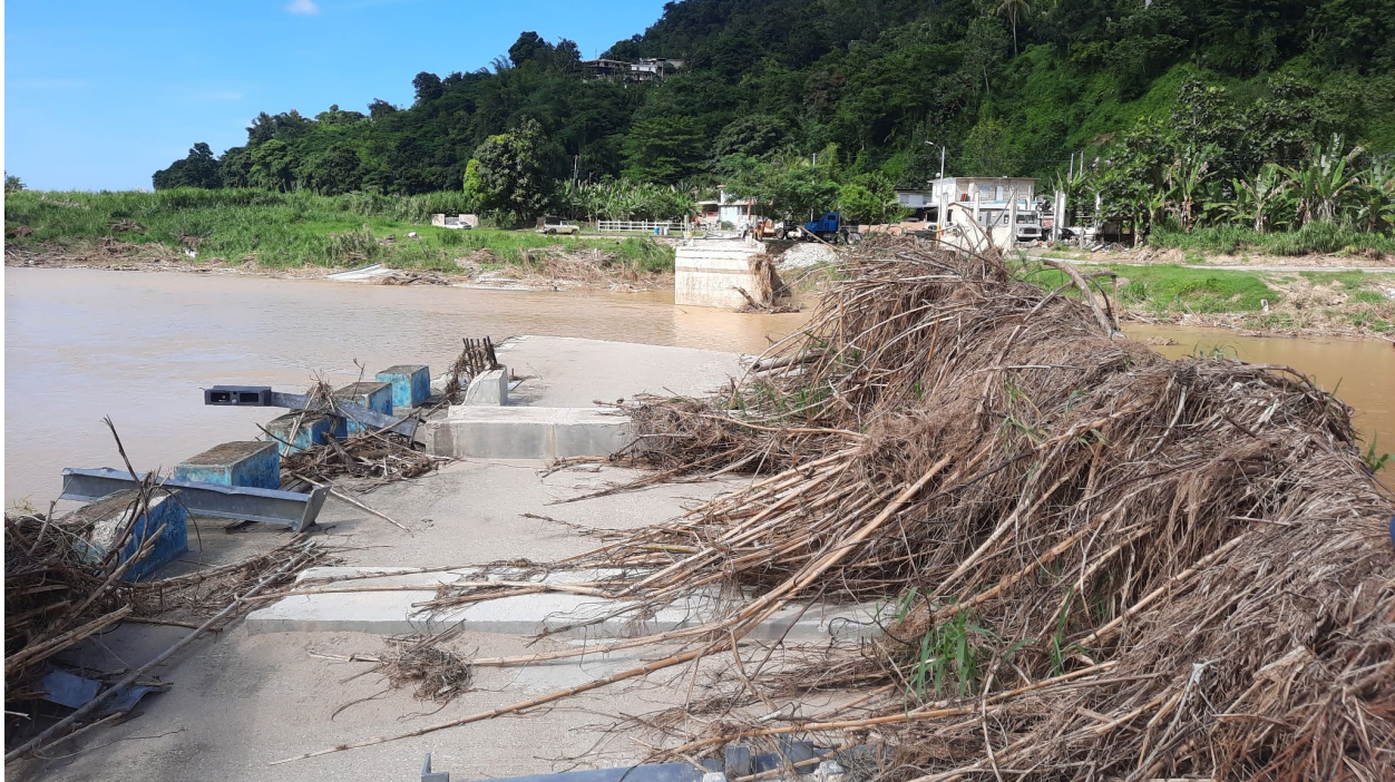
Figure 35: View of the missing segment of the temporary bridge of Rio Grande de Arecibo in Arecibo. Note the sheared rebar at center left of the photo that was used to anchor the temporary segment.
