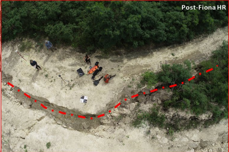
Figure 27. Aerial photos of the Ponce landslide indicating the landslide failures.
