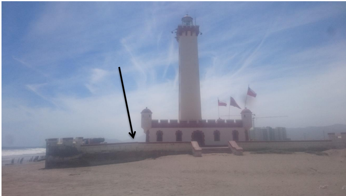
Figure 5.4. El Faro photograph looking north (29.90541S; 71.27411W). Note the break in the outer wall (i.e., change in angle indicated with the black arrow) where the western edge of the El Faro wall subsided with a westward tilt apparent at the top of the wall. This happened prior to this earthquake and was patched and painted over, however during the 2015 earthquake, cracks opened up along these fractures that suggest renewed subsidence.
