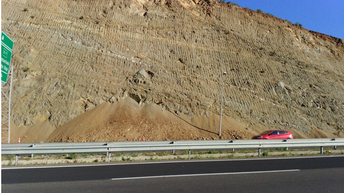
Figure 4.14. Km 280, southbound lane (photograph looking west from northbound lane). Rockfall closed one lane, damaged street light and exit sign (GPS RF2: 31.44367S; 71.56376W).
