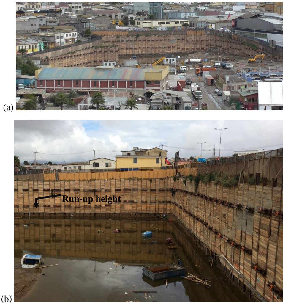
Figure 3.1. Flooded excavation in Coquimbo. No damage observed on the soldier piles and anchors (29.958151S; 71.337849W).
