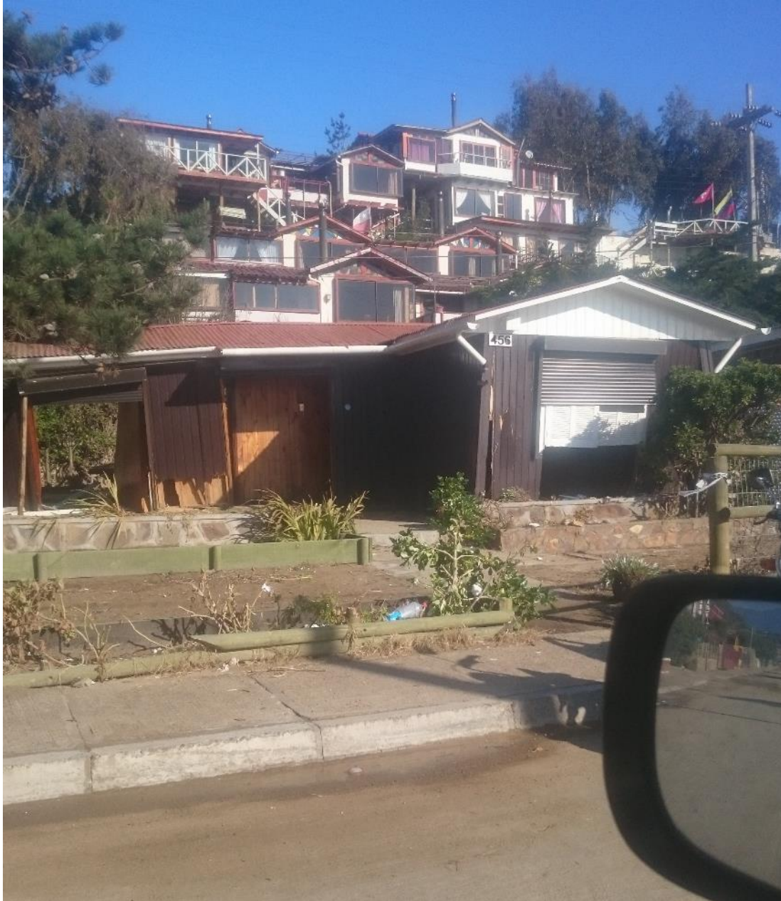
Figure 6.14. Field photograph looking east of a house at street level along the Costanera Av. in Los Vilos that was destroyed by the tsunami waves. Note that the house is tilted, and the backyard of the house is visible where the back wall was washed away. Many of the houses along this road were completely destroyed or greatly damaged by the waves. The beach here is just behind the photographer on the other side of the road (31.906212S; 71.500804W).
