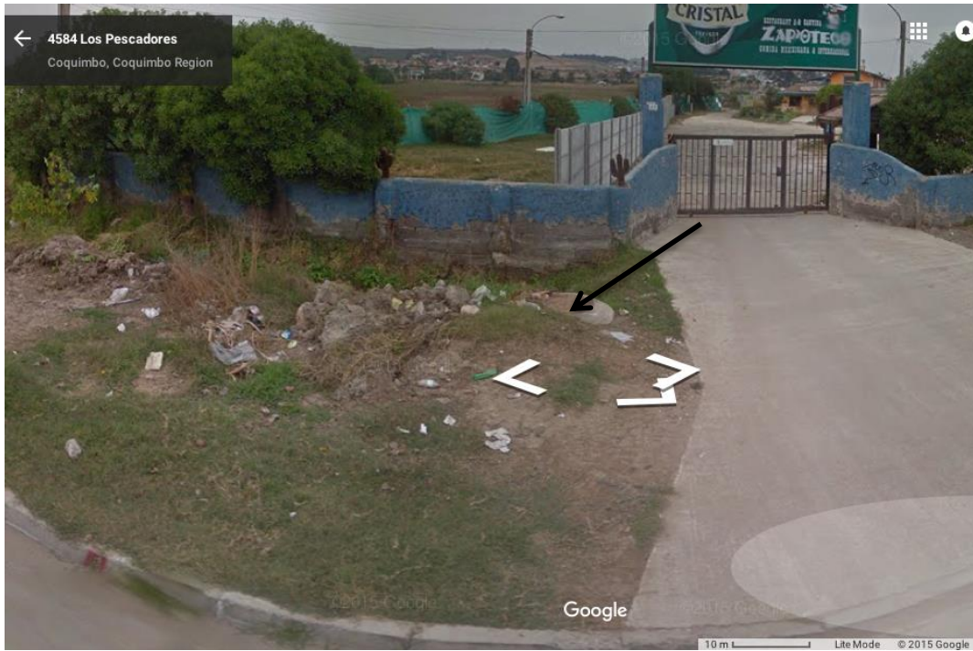
Figure 5.15. Google “Street View” of the same manhole cover seen in the previous figure pre-earthquake from ~ 4584 Los Pescadores (1 block southeast of the seaside). Note that it is flush with the ground surface and black arrow indicates manhole (29.95068S; 71.29456W).
