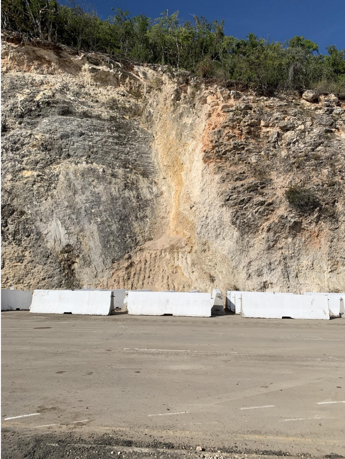
Figure 51: Part of the cut slope failure along the PR-2 landslide. The site suffered continuous failures during aftershocks and the 4 lanes of the roadway were shifted seaward.
