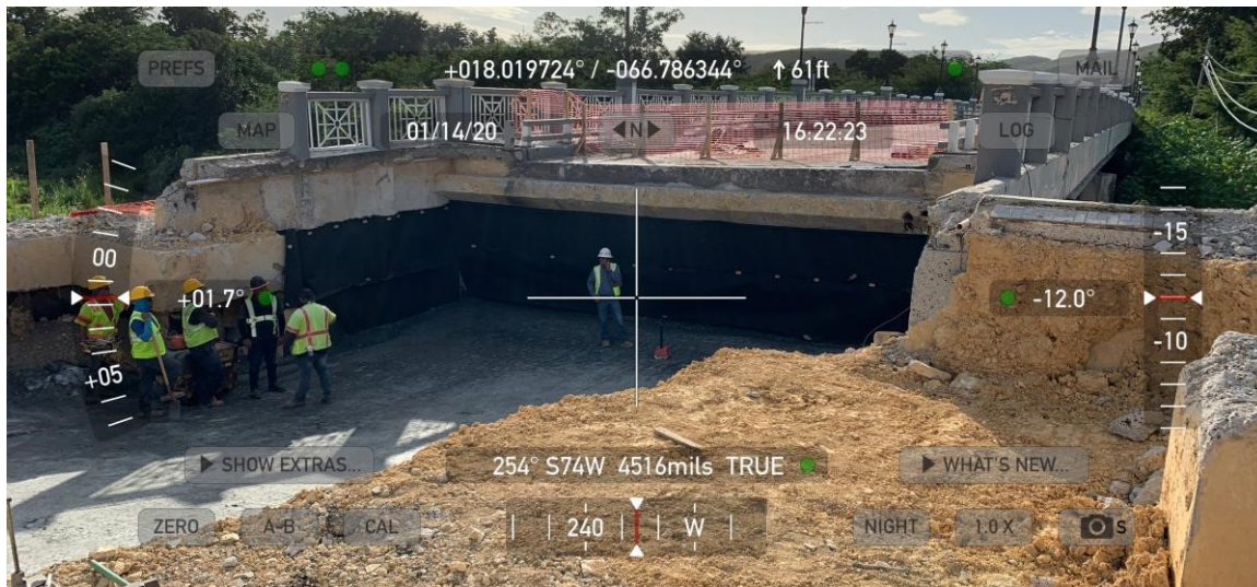
Figure 56. PR-127 bridge over Rio Guayanilla showing the east abutment already demolished.
