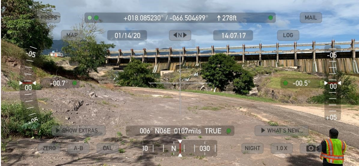
Figure 68. Downstream area at Guayabal dam. No damage was reported.
