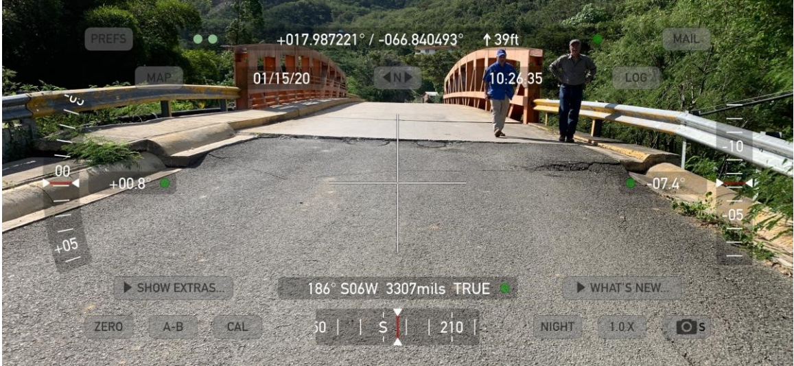
Figure 61. PR-335R bridge over the Rio Yauco north abutment showing ground settlement near the joint between flexible and rigid pavement. This settlement lead to a complete break of the sidewalk.
