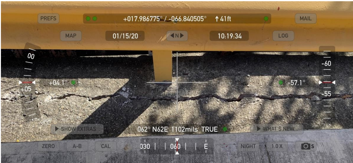
Figure 60. Detail of the ground cracks show in the previous figure.
