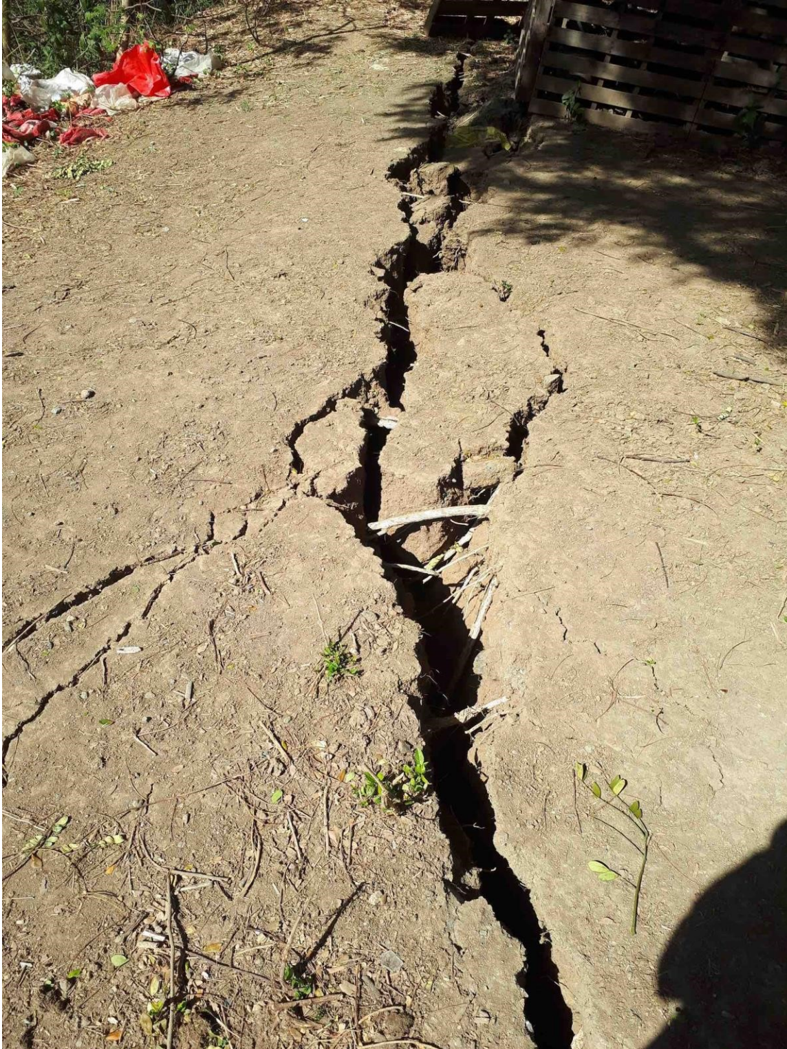
Figure 63: Lateral spreading at the same PR-335R bridge site as previous photo. The Rio Yauco is just a few meters to the right of the field of view (17.987162N, 66.840456W).
