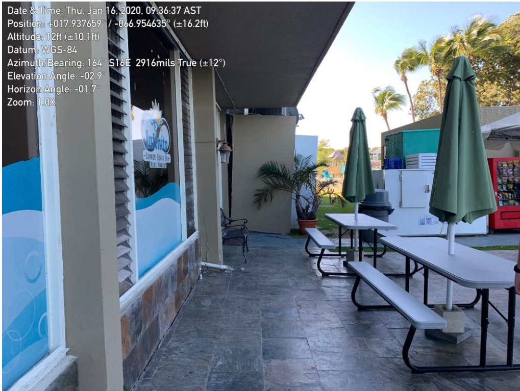
Figure 25. Subsidence of the floor slab due to ground settlement.
