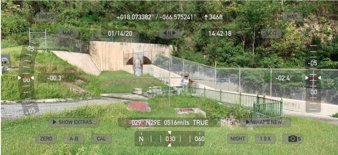
Figure 70. Discharge tunnel area at Cerrillos dam. No damage was reported.
