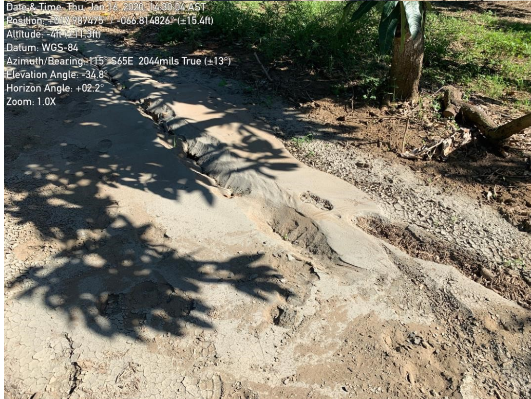
Figure 41. Ground cracks showing enormous amounts of sand ejecta at the mango fields in Tropical Fruit Farm.
