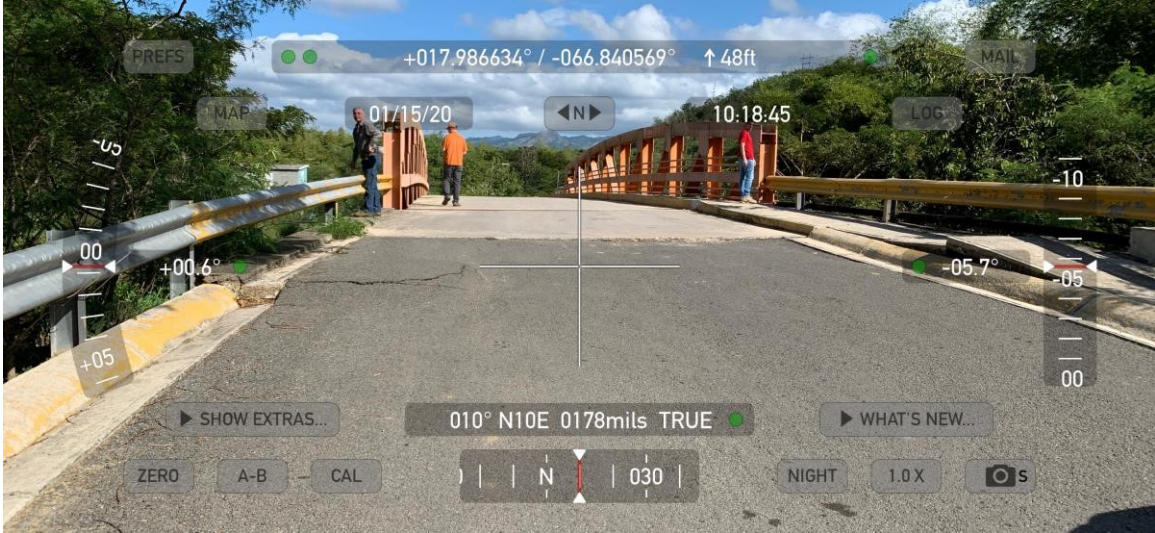
Figure 57. PR-335R bridge over the Rio Yauco south abutment showing damage near the joint between flexible and rigid pavement. Also, the sidewalk shows major displacement.
