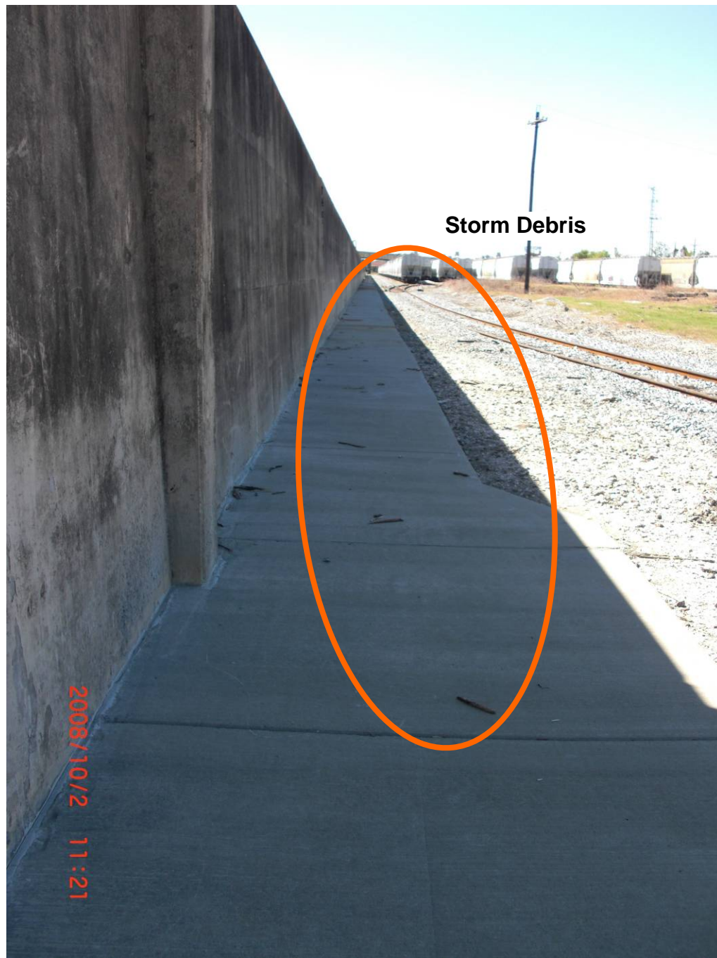
Fig. 2.4.2-4 Photograph from Oct. 2, 2008 of IHNC west side T-wall (same section as shown during Gustav in Fig. 2.4.2-2). Picture taken looking south on the protected side (IHNC is to the left and Claiborne Ave. Bridge is in the background). Waves overtopped this wall based both on the photos during Gustav (Fig. 2.4.2-2) and the debris still there on Oct. 2, 2008 (see above). The concrete splash apron was added here after Katrina to protect from erosion. After Gustav, there was evidence of minor erosion in the ballast of the railroad tracks to the right, but no evidence of distress to the wall itself or to the splash apron. (R. Gilbert)
