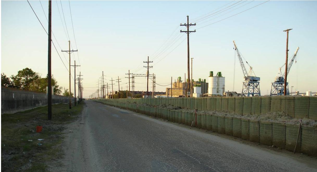
Fig. A.3-4. Temporary Bin Wall, IHNC northwest along France Road (L. Wooten)
