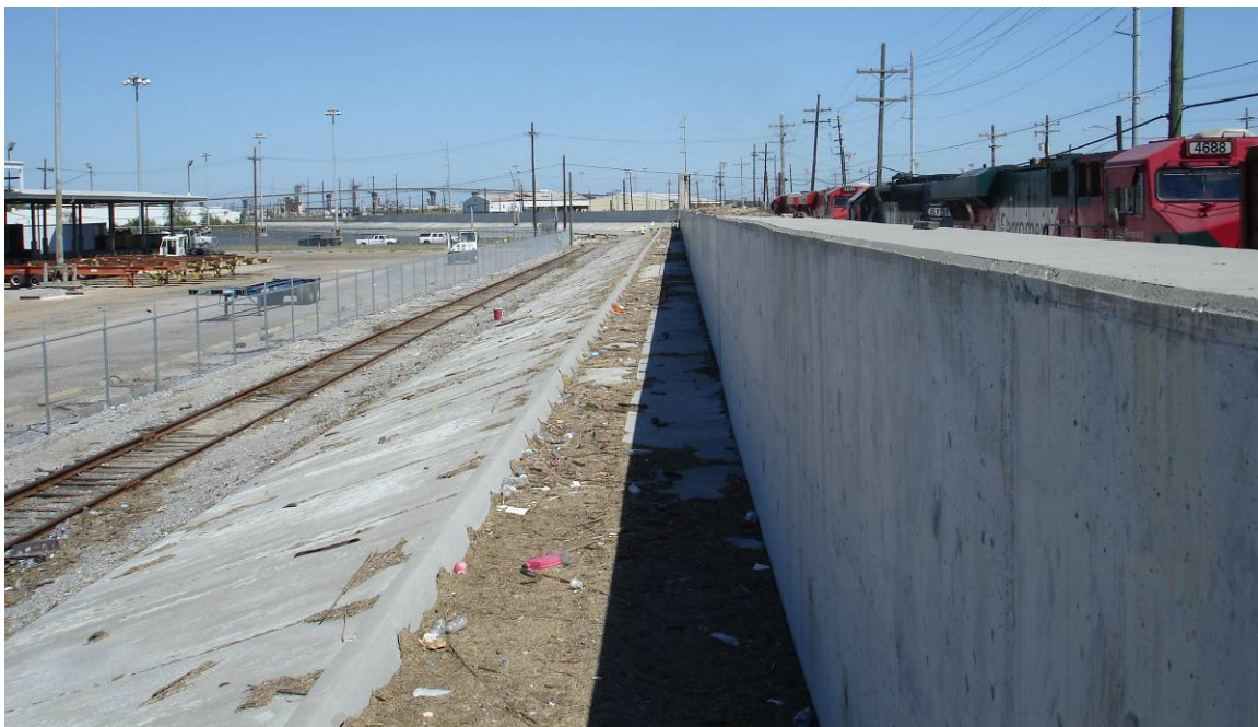
Fig. 2.4.1-8 Protected side of new L-wall along IHNC West. Note debris left by overtopping on floodwall and slope protection. October 2008 (L. Wooten)
