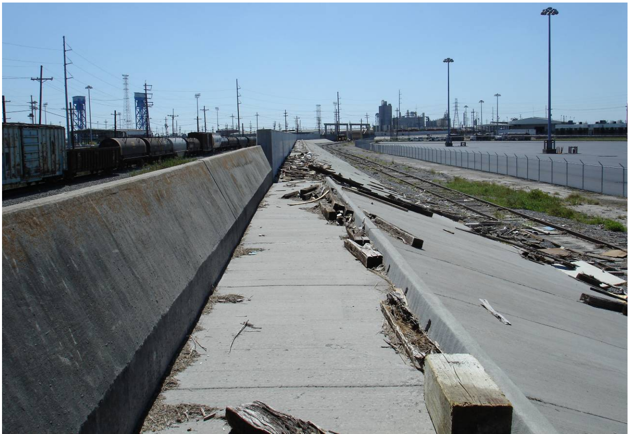
Fig. A.3-3. I-wall and splash apron, IHNC west along France Road; new T-wall and splash apron in background (L.Wooten)
