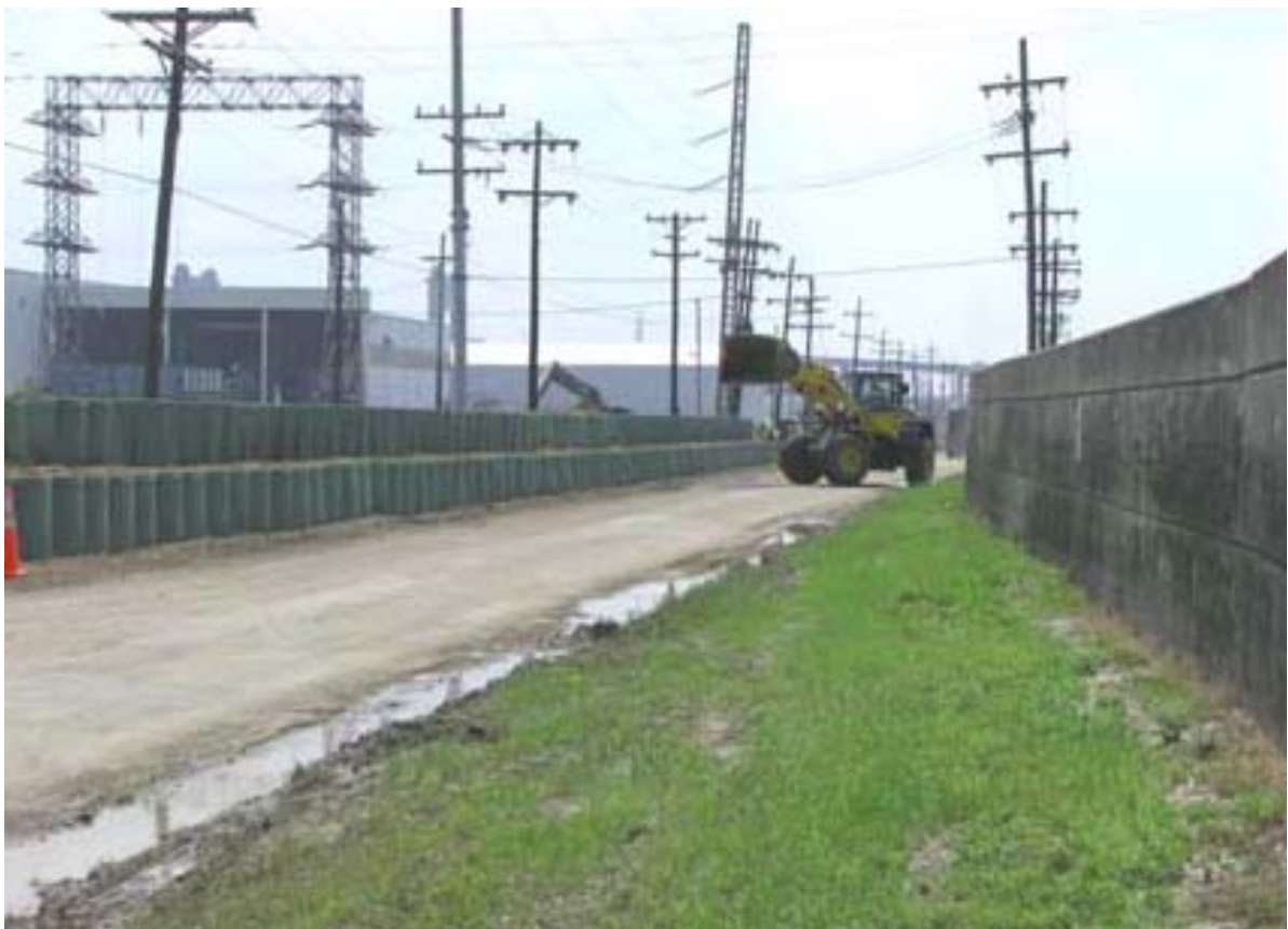
Fig. 2.4.5-1. Temporary Bin Wall under construction, IHNC northwest along France Road ( http://www.mvn.usace.army.mil/HPS/Status%20Report%20Newsletters/Sept_9_2008.pdf )
