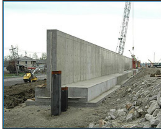
Figs. 1.2.3-1 & 2. T-wall schematic and T-wall under construction ( http://www.mvn.usace.army.mil/hps2/hps_outfall_canals.asp )
