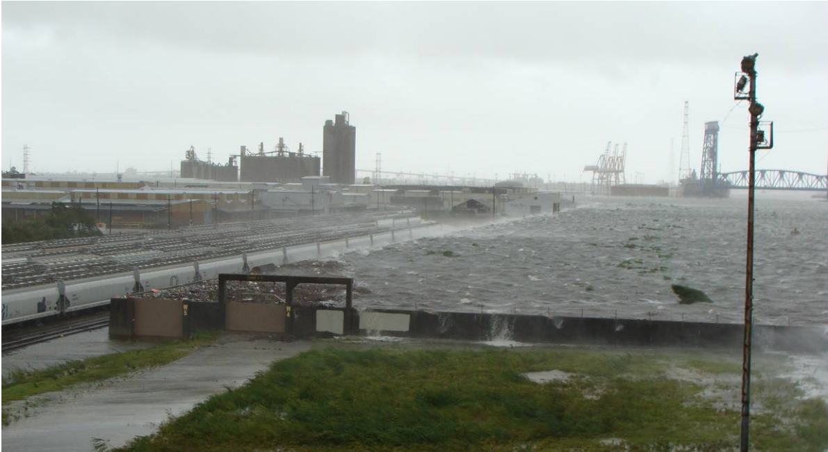
Fig. 2.4.2-2. Photograph from Sept. 1, 2008 of Gustav storm surge. Photograph taken from Claiborne Ave. Bridge looking north. The waves are overtopping the T-wall. (USACE)
