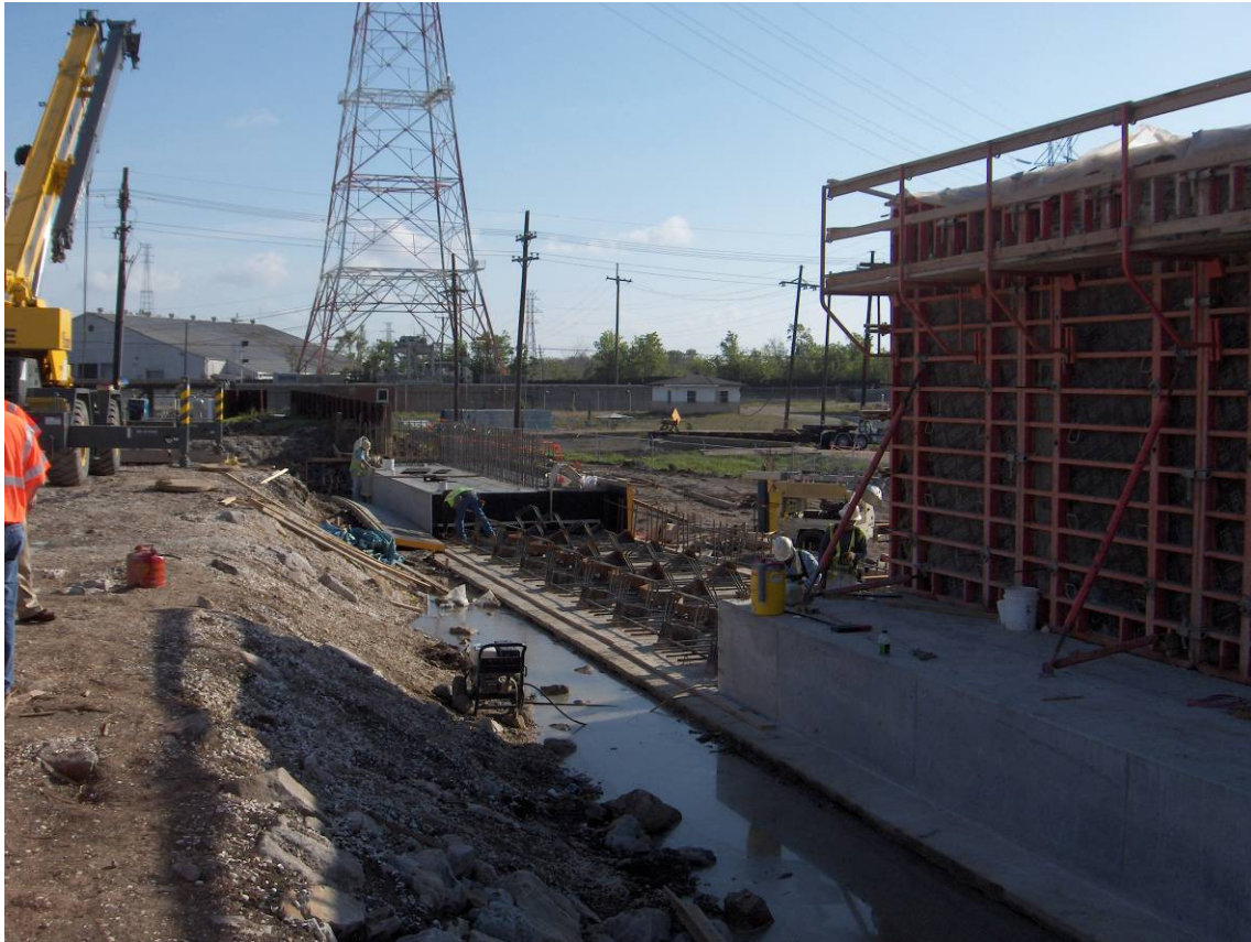
Fig. 2.4.3-5 Photograph from 2006 of T-wall being constructed to replace the I-wall that breached in two locations on the east side of the IHNC during Katrina. Photograph taken looking north at about the same location as the northern-most breach near Florida Ave. (see Fig. 2.4.3-4). (ASCE External Review Panel, May 2006)
