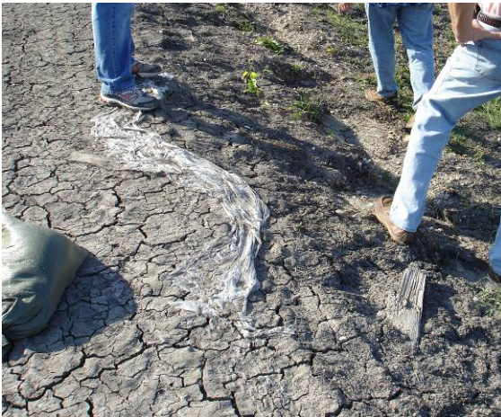
Figs. 2.6-6 and 2.6-7. Desiccation cracks on Plaquemines Parish back levee (L. Wooten)
