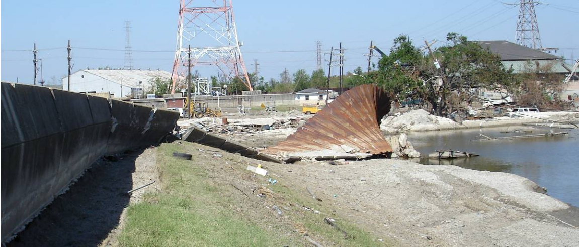
Fig. 2.4.3-4 Photograph from 2005 of northern-most breach that occurred in the I-wall on east side of the IHNC during Katrina. Photograph is looking north, with the IHNC on the left and the Lower 9 th Ward of the right. The breach was 250 feet long and located just south of Florida Avenue. The suspected cause of this breach was a stability failure when the surge level was near the top of the water. (L. Wooten)
