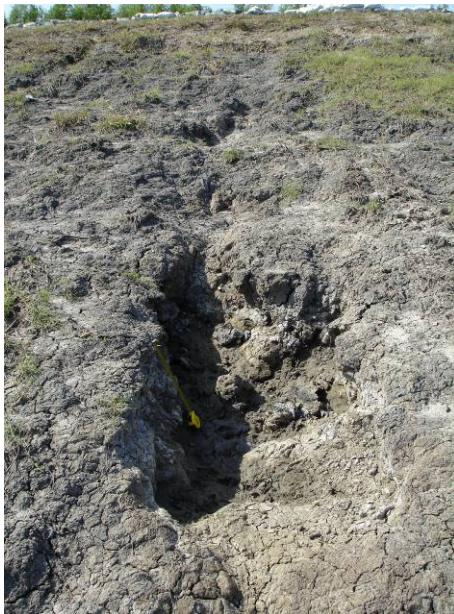
Figs. 2.6-9 and 2.6-10. Overtopping erosion gullies on Plaquemines Parish back levee, protected side (L. Wooten)
