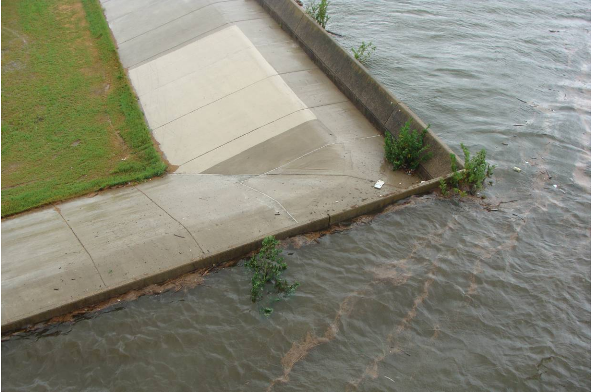
Fig. 2.4.3-7 Photograph from Sept. 1, 2008 of Gustav storm surge. Photograph taken just south of Claiborne Avenue, looking south, south-west. The storm surge is within about 1 foot of the top of the wall. The wall at this location is an I-wall that was overtopped but did not breach during Katrina. The protected side of the wall has been built up to improve stability and covered with a concrete to protect against erosion. The I-wall stick-up on the protected side is just under 4 feet, while that on the canal side is just under 6 feet. (USACE)
