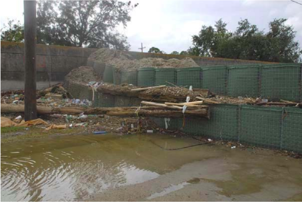
Fig. 2.4.5-2. Post-Gustav Photograph of End of Temporary Bin Wall at Tie-in to I-Wall ( http://www.mvn.usace.army.mil/HPS/Status%20Report%20Newsletters/Sept_9_2008.pdf )
