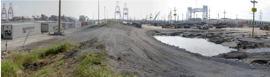
Fig. 2.4.1-2 IHNC West levee Katrina breach site, October 2005 (Breach had been temporarily repaired. Note scour hole.) (L. Wooten)
