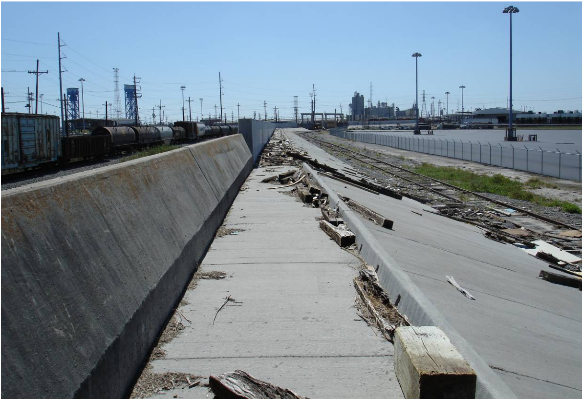
Fig. 1.2.3-3. I-wall and splash apron, IHNC west along France Road; New L-wall and splash apron in background (L.Wooten)
