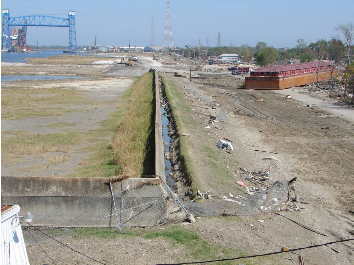
Fig. 2.4.3-3 Photograph from 2005 of southern-most breach and the scour behind the adjacent I-wall on east side of IHNC during Katrina. Photograph is looking north, from the Claiborne Avenue Bridge. (L. Harder)
