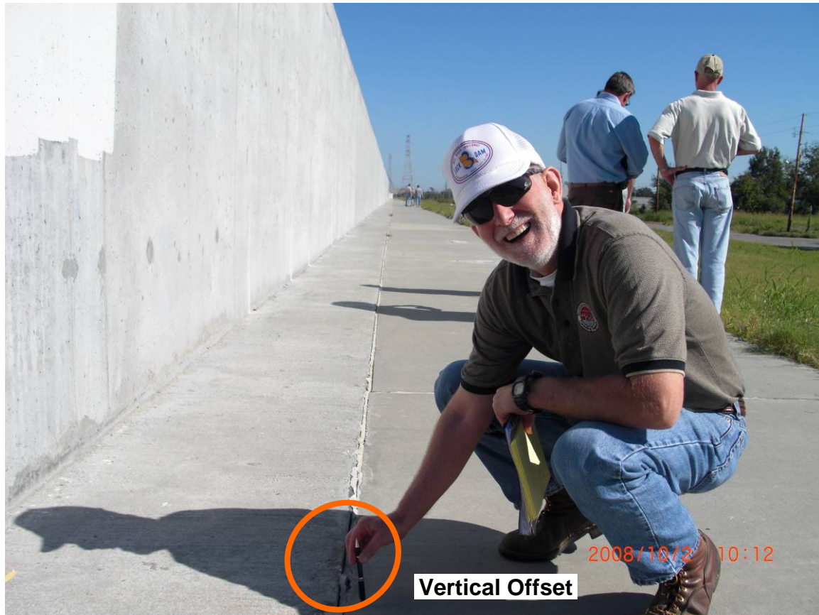
Fig. 2.4.3-11 Photograph from Oct. 2, 2008 of new T-wall section between Claiborne and Florida Avenues (shown in Fig. 2.4.3-9 during Gustav). After Gustav, there were no noticeable signs of distress in this wall. One potentially interesting feature here is the approximately 1-inch-deep vertical offset between the pile-supported base of the wall (to the left of the caulked joint) down to the concrete slab-on-grade splash apron (to the right of the caulked joint). If this splash apron was cast to be flush with the base of the wall, then this offset is possibly an indication of differential settlement between the pile-supported wall and the surrounding ground. If it is settlement, the rate is approximately 1 inch over two years, or 0.5 inches per year, and is likely occurring in the upper 70-feet of the profile (because the piles tip is approximately 70 feet below the ground surface – see Fig. 2.4.3-6). (R. Gilbert)
