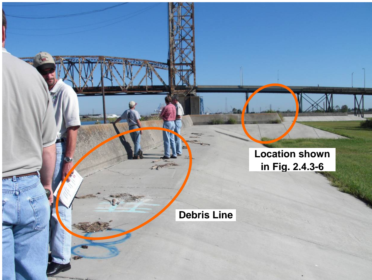
Fig. 2.4.3-8 Photograph from Oct. 2, 2008 of I-wall shown during Gustav above in Fig. 2.4.3-6. Photograph taken looking north on protected side (IHNC is to the left and Lower 9 th Ward to the right); location shown in Fig. 2.4.3-7 is circled. This wall was loaded with the surge within about 1 foot of the top of the wall (Fig. 2.4.3-7), and apparently had waves that overtopped it based on the debris line (circled in photo). After Gustav, there were no noticeable signs of distress here, including movement of the wall due to the surge load or erosion at the toe due to waves overtopping the wall. (R. Gilbert)
