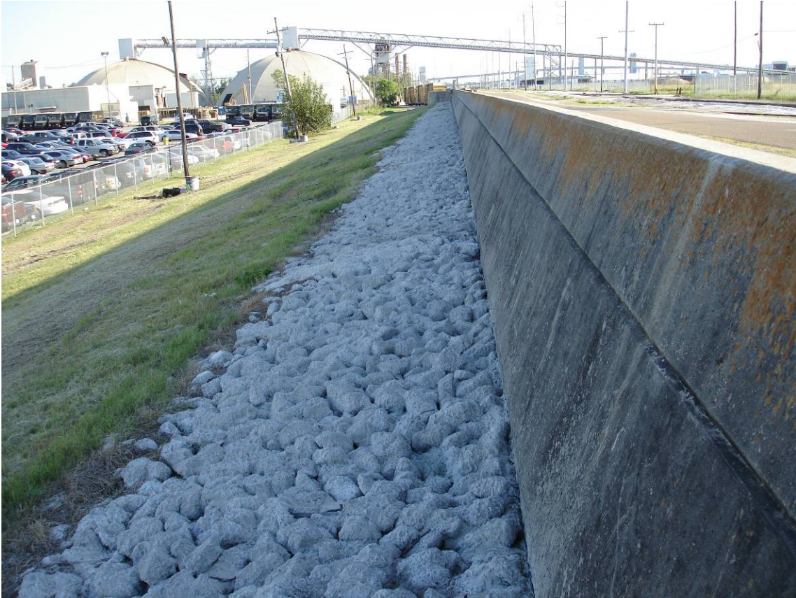
Fig. 2.4.4-1 IHNC Floodwall near East Morrison Road. Note splash apron (center) and relief wells (left). (L. Wooten)
