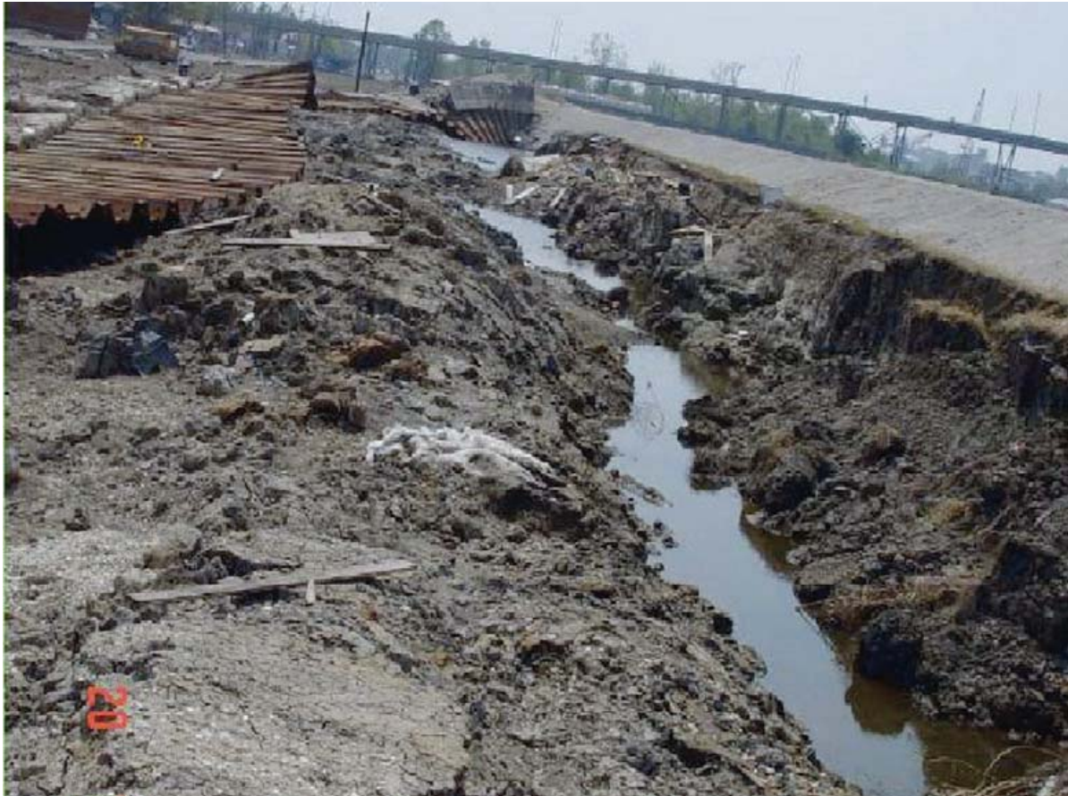
Fig. 2.4.3-2 Photograph from 2005 of southern-most breach that occurred in the I-wall on the east side of the IHNC during Katrina. Photograph is looking south, with the IHNC on the right and the Lower 9 th Ward of the left. The breach was 850 feet long and located about 100 yards north of the Claiborne Avenue Bridge (seen in background). The suspected cause of this breach was erosion of the toe on the protected side due to water pouring over the top of the wall when the surge level exceeded the top of the wall. ("Performance Evaluation of the New Orleans and Southeast Louisiana Hurricane Protection System, Volume V: The Performance - Levees and Floodwalls," Final Report of the Interagency Performance Evaluation Task Force, June 2007)
