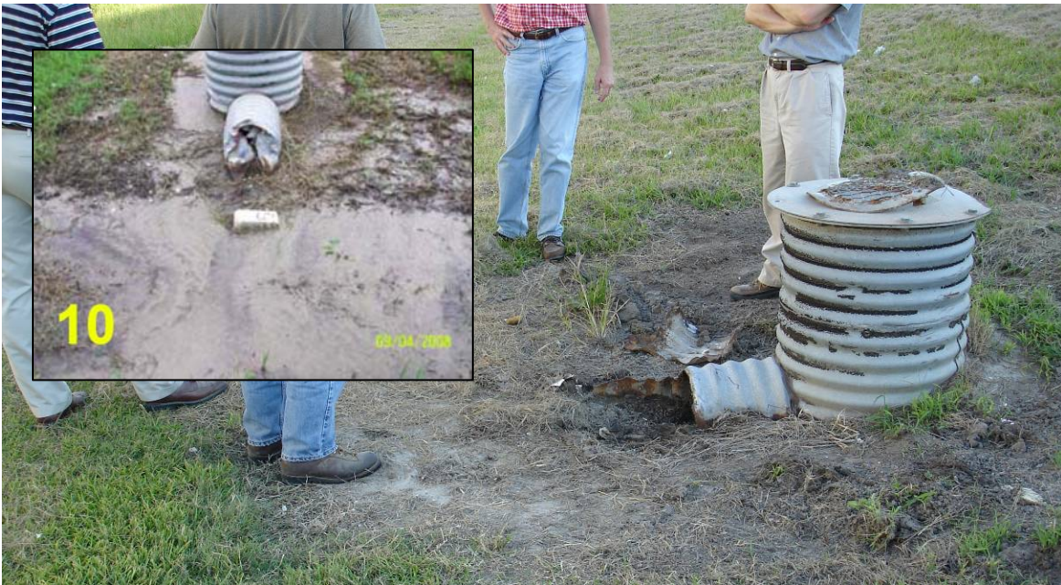
Fig. 2.4.4-2 Relief Well Cover, October 2008 with inset taken from USACE Hurricane Gustav Damage Assessment Team SITREP 05 Sep 08 (L. Wooten)
