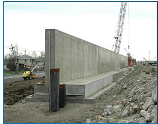
Figs. A.3-1 & 2. T-wall schematic and T-wall under construction ( http://www.mvn.usace.army.mil/hps2/hps_outfall_canals.asp )
