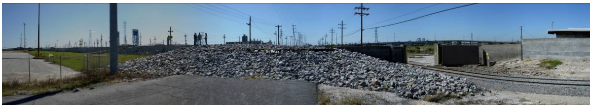
Fig. 2.4.1-5 IHNC West repaired breach at railroad gate transition, October 2008 (L. Wooten)
