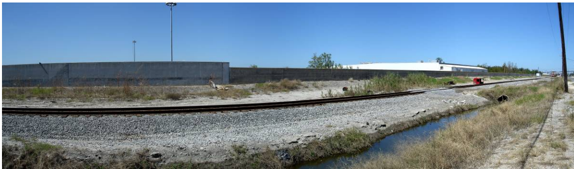
Fig. 2.4.1-7 New L-wall – old I-wall transition near location of Katrina I-wall breach on IHNC West (L. Wooten)
