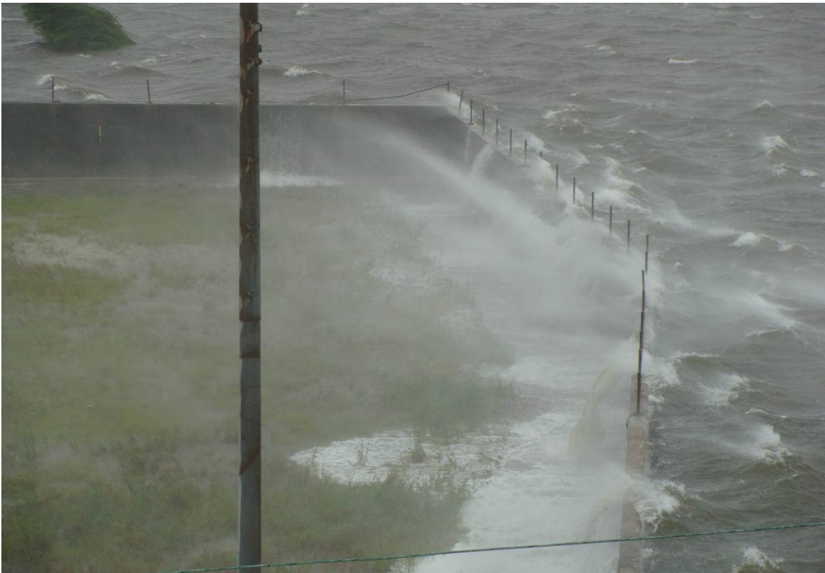
Fig. 2.4.2-3. Photograph from Sept. 1, 2008 of Gustav storm surge. Photograph taken from Claiborne Ave. Bridge looking north at T-wall southeast of floodwall shown in Fig. 2.4.2-2. (USACE)
