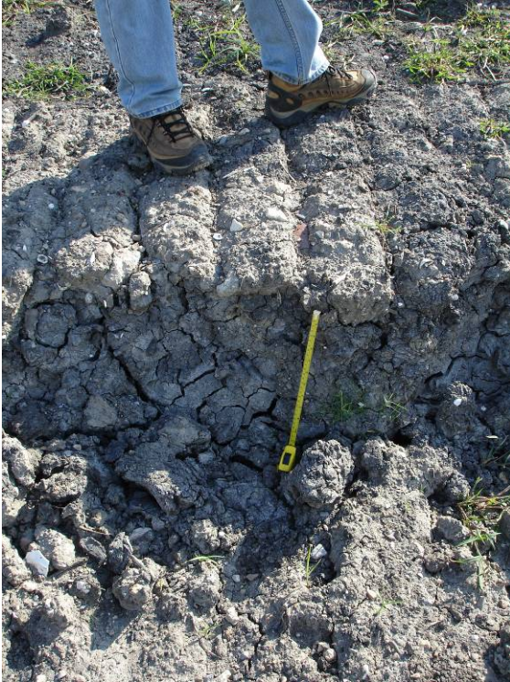
Fig. 2.6-5. Scarp above slide on Plaquemines back levee (L. Wooten)
