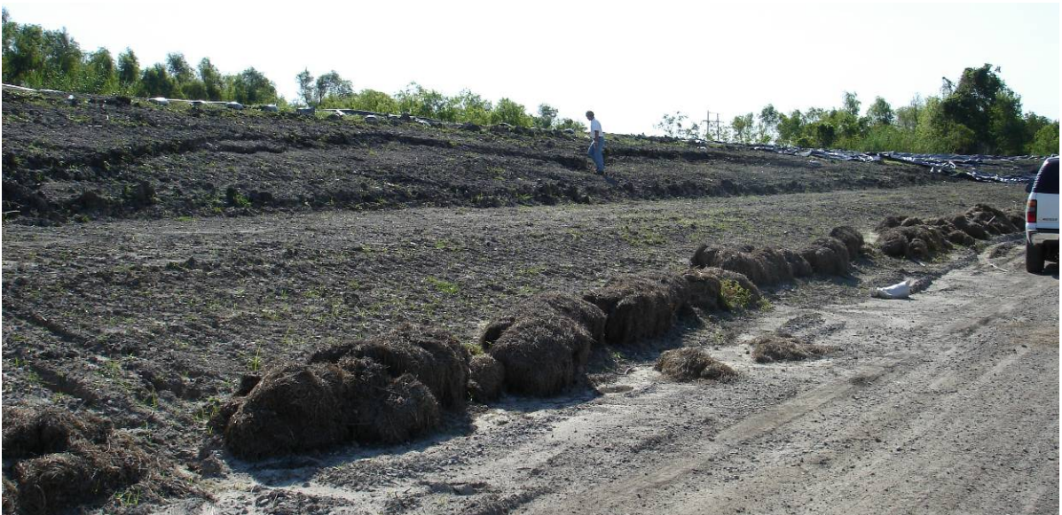
Fig. 2.6-4. Protected side slope of Plaquemines Parish back levee and slide (L. Wooten)
