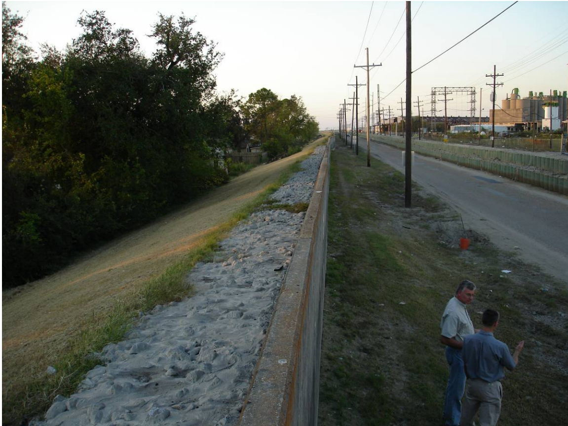
Fig. 2.4.5-3. IHNC I-wall and grouted riprap splash apron (L. Wooten)
