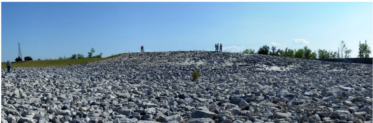
Fig. A.3-5. Transition Protection and Modification, Flood Side of Bayou Dupree Flood Wall (L. Wooten)
