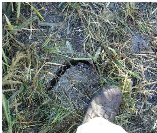
Figs. 2.6-6 and 2.6-7. Desiccation cracks on Plaquemines Parish back levee (L. Wooten)
