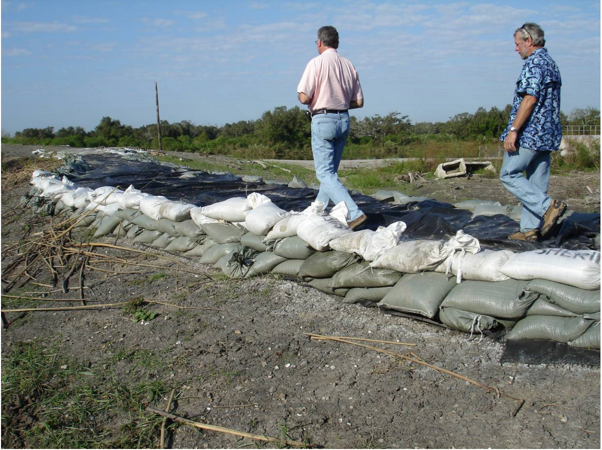
Fig. 2.6-3. Plaquemines Parish Back Levee sand bags and geotextile crest cover (L. Wooten)
