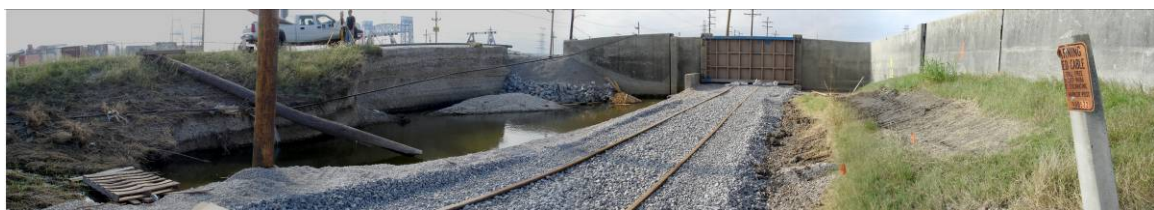
Fig. 2.4.1-4 IHNC West Katrina breach at railroad gate transition, October 2005 (L. Wooten)
