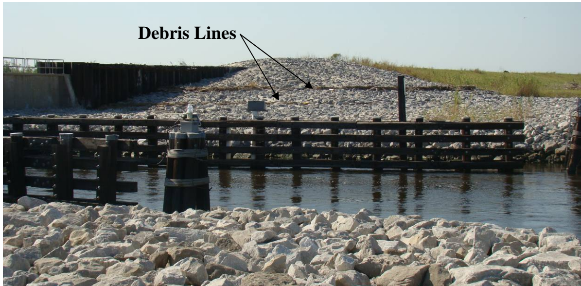
Fig.2.2.2-4 Bayou Dupree Gate, October 2008, northwest flank, MRGO side, looking east. The lower debris line may represent the high water level during Ike. (L. Harder)
