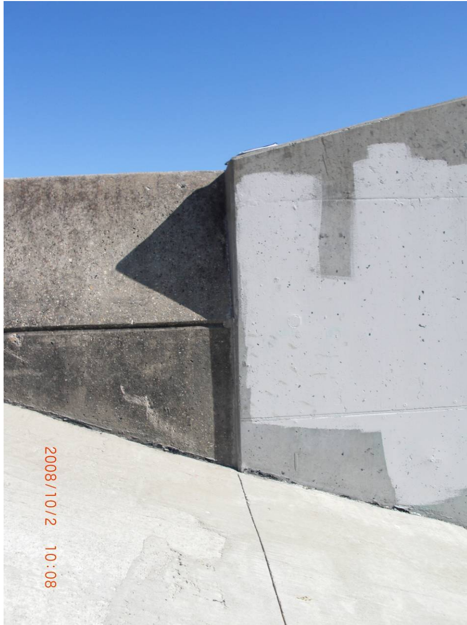
Fig. 2.4.3-10 Photograph from Oct. 2, 2008 of transition between old I-wall and new T-wall (shown in Fig. 2.4.3-3 post-Katrina and Fig. 2.4.3-9 during Gustav). Picture taken looking north from the protected side (same orientation as Fig. 2.4.3-3 and Fig. 2.4.3-9). After Gustav, there were no noticeable signs of distress at this transition. (R. Gilbert)
