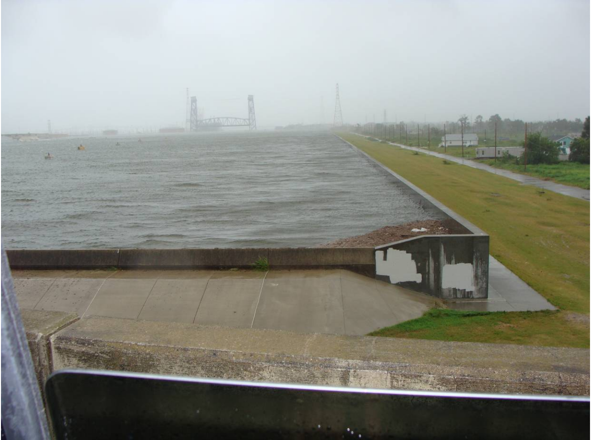
Fig. 2.4.3-9 Picture from Sept. 1, 2008 of Gustav storm surge. Picture taken from the Claiborne Avenue Bridge, looking north toward Florida Ave Bridge (seen in background) from perspective similar to Fig. 2.4.3-3. This location is where the old I-wall section shown in Figs. 2.4.3-7 and 2.4.3-8 transitions to the new T-wall section shown being constructed in Figs. 2.4.3-5 and 6. The storm surge is close to the top of the I-wall and several feet below the top of the T-wall. (USACE)
