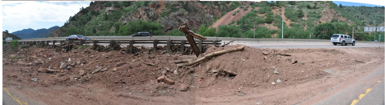
Figure 3.2.12. View of the US 24 westbound on-ramp. Top: view southeast down the westbound on-ramp; some of the sediment cleared from on-ramp is visible on the shoulder between westbound US 24 and the on-ramp. Bottom: panoramic view toward southwest (left) and northwest (right); woody debris around the wood posts of the guardrail may be a suggestion of the flood level in the westbound lanes. Camera position for top photo is +38.8719^{\circ} N, -104.9265^{\circ} W, approximate elevation 6670 feet.
