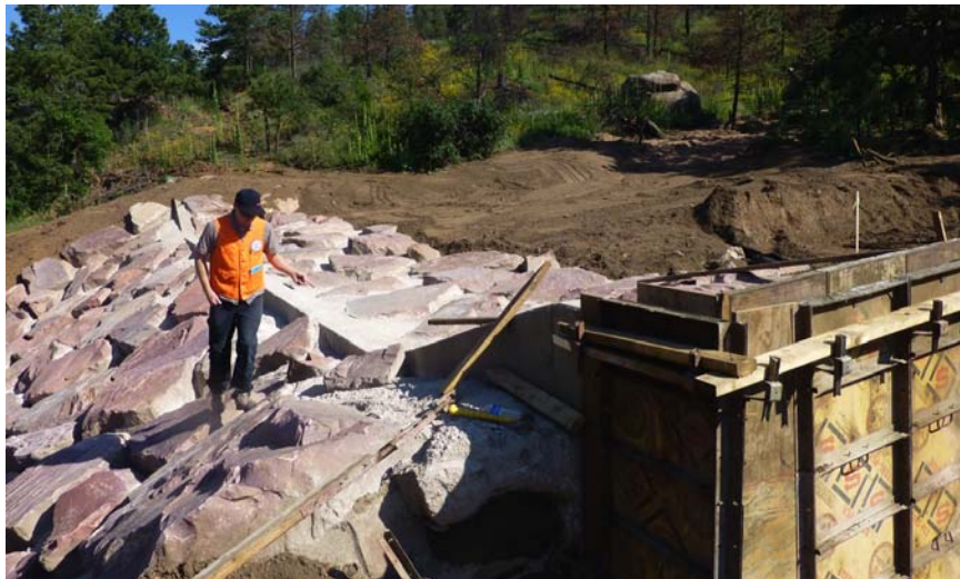
Figure 3.4.14. Partially grouted riprap spillway west of Cascade on US 24. Top: view looking northeast from the shoulder of US 24; camera position was 38.9123° N, -104.9769° W, approximate elevation 7552 ft. Bottom: view looking north from the crest of the riprap spillway; camera position was 38.9125° N, -104.9766° W, approximate elevation 7592 ft. Individual rock blocks are approximately 1 m across; note minimal freeboard between the top of the spillway in the center of the photograph and the natural drainage channel to the right.
