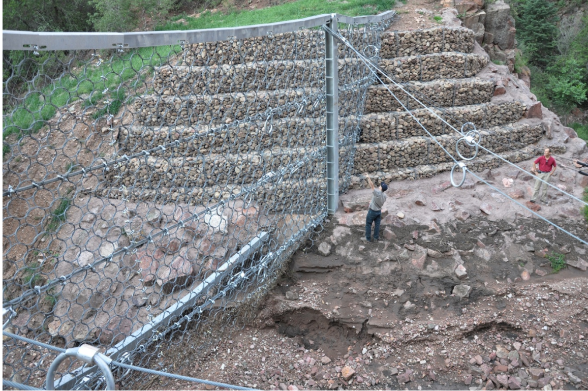
Figure 3.4.21. Ring-net debris fence in Queens Canyon above Glen Eyrie conference center.
