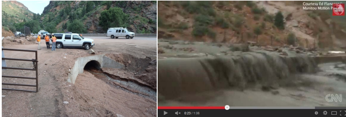
Figure 3.2.1. Mouth of Waldo Canyon at US Highway 24; Waldo Canyon culvert inlet on August 16, 2013, half full of sediment at inlet (left); screenshot of YouTube video by Ed Flanagan taken on August 9, 2013 (right). Left: View toward southeast from +38.887^{\circ}\text{N} , -104.932^{\circ}\text{W} , approximate elevation 6767 feet. Right: View from eastbound lanes showing the center K-rail barrier on US 24 being overtopped by water and sediment discharge from Waldo Canyon apparently after filling the westbound lanes ( http://www.youtube.com/watch?v=Q_iMDHqRV4U ); rock fall fence adjacent to east side of Waldo Canyon is visible.
