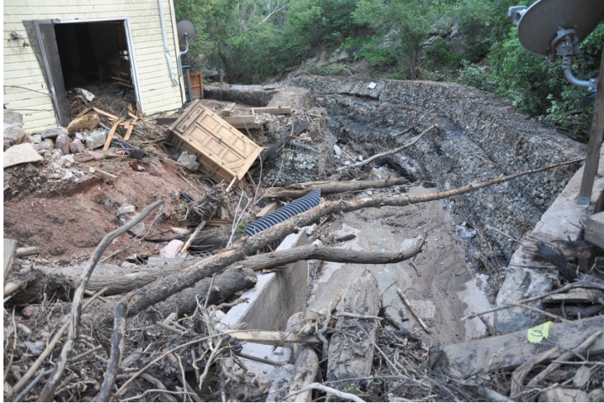
Figure 3.3.8. View looking south from the culvert outlet at the gabion-lined channel in the northern part of Manitou Springs residential area south of US 24. The concrete wall visible in the lower center of the photo is the culvert outlet. The main part of the flood passed through the area shown in this photograph. Substantial flood flows also went around the left side of the yellow house. Camera location: +38.8630° N, -104.9174° W, elevation 6432 ft.
