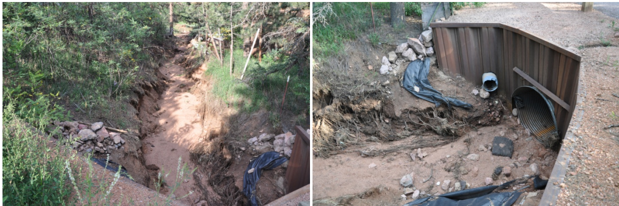
Figure 3.4.7. Unnamed Creek 3 downstream and upstream from Hagerman Road. Top: view looking downstream (southwest) at the concrete channel. Bottom left: view looking upstream (northeast) at the unlined channel. Bottom right: view looking south at the inlet to the metal pipe culvert under Hagerman Road. All views from approximately 38.8971° N, -104.9695° W, approximate elevation 7426 ft.
