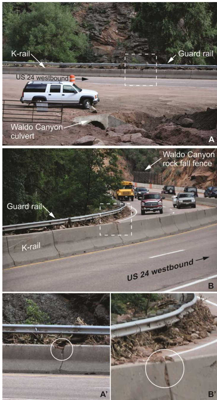
Figure 3.2.6. Rock and woody debris on K-rail and under guard rail on eastbound US 24. A. view from mouth of Waldo Canyon (38.877° N, -104.932° W); B. view from wide shoulder on westbound US 24 (38.8754° N, -104.9292° W). A' and B' are inset photos for A and B, respectively; soil on K-rails marked by open white circles.
