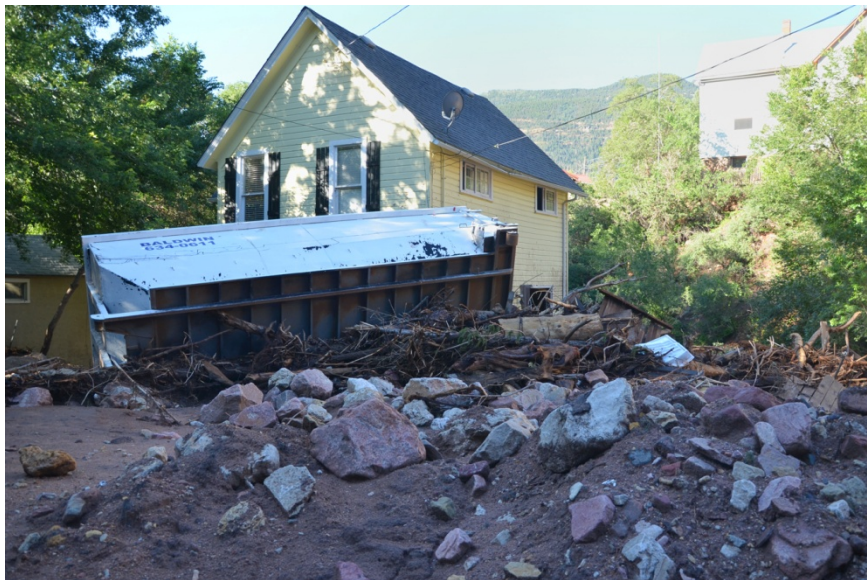
Figure 3.3.7. View looking south along Cañon Avenue and the buried culvert for Williams Canyon drainage. Most of the flood flow passed to the right of the two-story yellow house, but substantial flow also went to the left down Cañon Avenue. Top: photo by GEER team members taken on August 16, 2013. Bottom: photo by Jason Kean, US Geological Survey, taken on August 13, 2013. Camera location: +38.8633^{\circ} N, -104.9173^{\circ} W, elevation 6453 ft.
