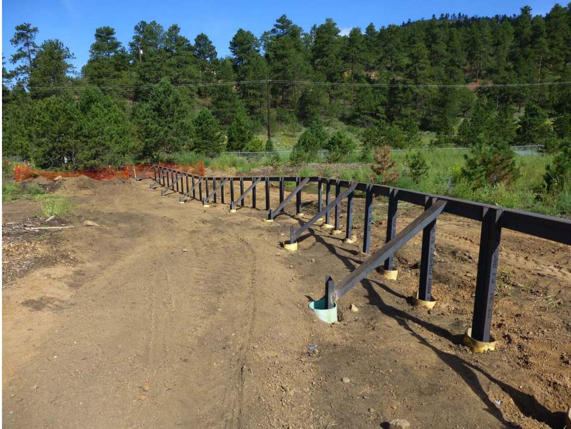
Figure 3.4.17. Debris rack under construction in the mouth of Wellington Gulch south of Wellington Road. Note Sonotubes for grouting of foundation footings, the diagonal support braces, and the welded joints. The rack is oriented perpendicular to the flow direction. View looking north from 38.918603° N, -104.983124° W, approximate elevation 7611 ft.
