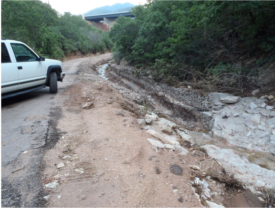
Figure 3.3.4. View looking south along Cañon Avenue at the transition from grouted riprap to gabion baskets lining the channel of Williams Canyon. The US 24 bridge over Williams Canyon is visible in the top center of the photo. Camera location: +38.9320° N, -104.9178° W, elevation 6515 ft.
