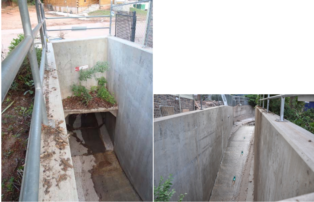
Figure 3.3.11. Views of deep rectangular channel and inlet to box culvert at Cañon Avenue. Left: view to southeast; Cañon Avenue and church at top of photo. Right: view northwest at grade transition from open-channel section to box culvert section. It is difficult to appreciate from these photos that a major flood event occurred one week prior to the date they were taken. Camera location: +38.8616^{\circ} N, -104.9169^{\circ} W, elevation 6405 ft.
