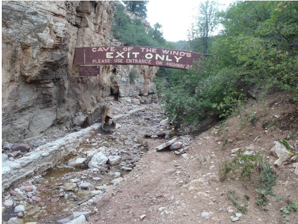
Figure 3.3.2. View looking north (upstream) from the bottom of Williams Canyon at the end of Cañon Avenue at Geneva Trail. The pre-flood channel appears to be the narrow space between the rock cliff and the stone-and-mortar wall; the wider eroded strip appears to be the exit road from Cave of the Winds. Camera location: +38.8655° N, -104.9178° W, elevation 6522 ft.
