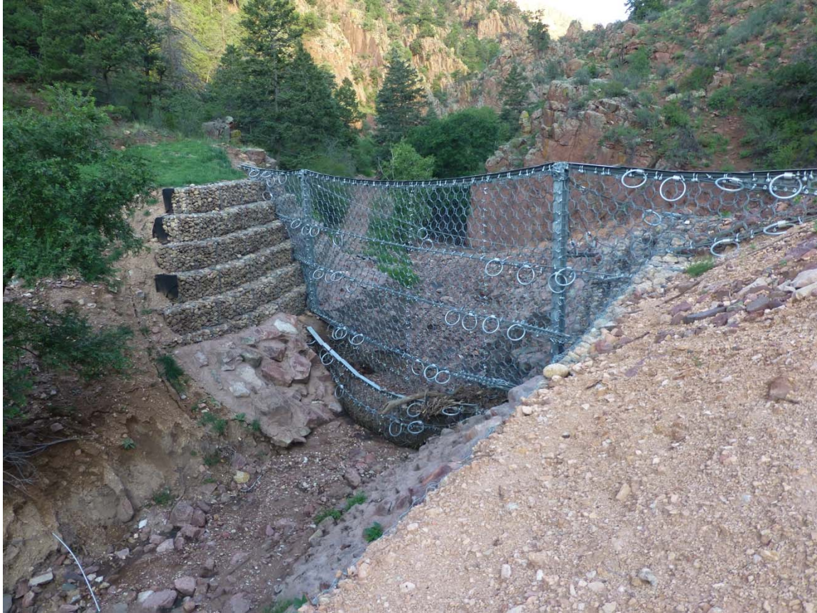
Figure 3.4.20. Ring-net debris fence constructed in the mouth of Queens Canyon above the Glen Eyrie Castle and conference center. View to the west from 38.8937° N, -104.8872° W, approximate elevation 6571 ft. Note gabion walls and grouted riprap protecting the abutments and channel from erosion, the use of two separate fences in the design, and the accumulation of a small amount of mostly gravelly sediment and logs in the lower fence. Prominent circles are loops on cables that are friction brakes to convert mechanical energy into heat and minimize damage to the fence while stopping debris.
