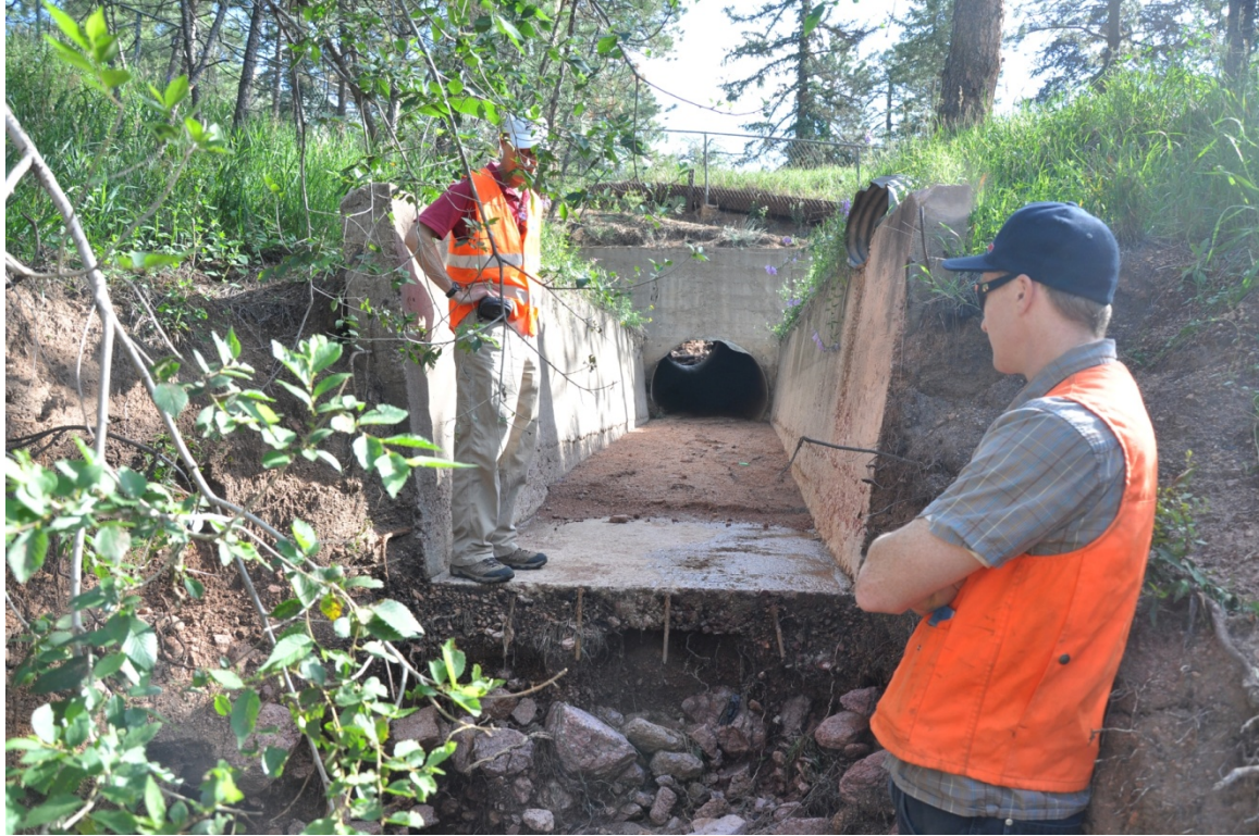
Figure 3.4.6. Concrete open-channel section and metal pipe culvert outlet on west side of Hagerman Road, Town of Cascade. Concrete channel appears to have been constructed after the culvert, probably because of erosion at the culvert outfall similar to the erosion at the end of the concrete channel section. Bare concrete at end of concrete section probably is related to discharge from the 12-inch-diameter corrugated metal pipe at shoulder height across from man standing on the concrete. View looking northeast from 38.8972° N, -104.9695° W, approximate elevation 7421 ft.
