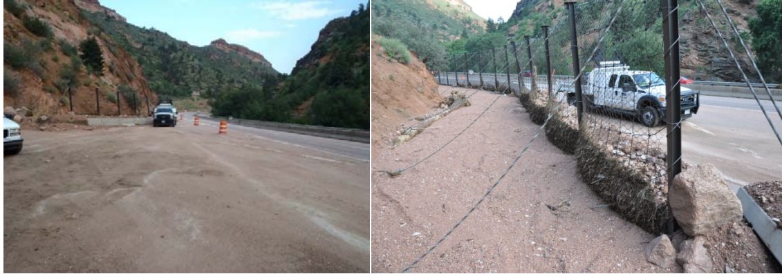
Figure 3.2.5. The rockfall fence adjacent to the mouth of Waldo Canyon. Left: the K-rail barrier and the super-elevation of the highway east of where Waldo Canyon meets US 24 also are visible. View is east-southeast from +38.877^{\circ} N, -104.932^{\circ} W, approximate elevation 6765 feet. Right: view of August 9, 2013, storm debris trapped by rockfall fence on the highway side of the fence.
