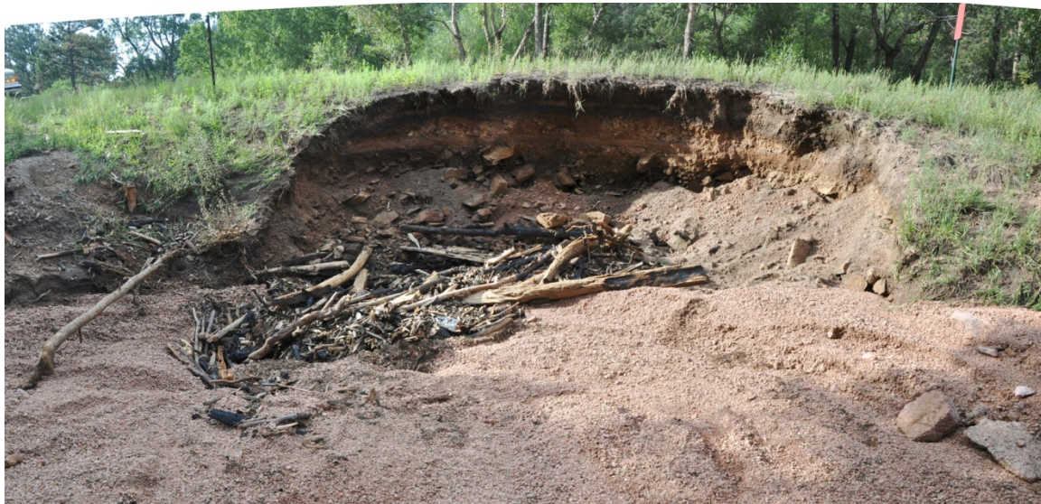
Figure 3.4.2. Unnamed Creek 1 where it enters a culvert under US 24 that was buried by sediment in the August 9, 2013, storm. Top: view looking west across the mouth of Unnamed Creek 1 at US 24. Bottom: view looking south at embankment of US 24 where the culvert inlet has been buried. Location of culvert inlet at westbound US 24: 38.8900° N, -104.9586° W, approximate elevation 7195 ft.
