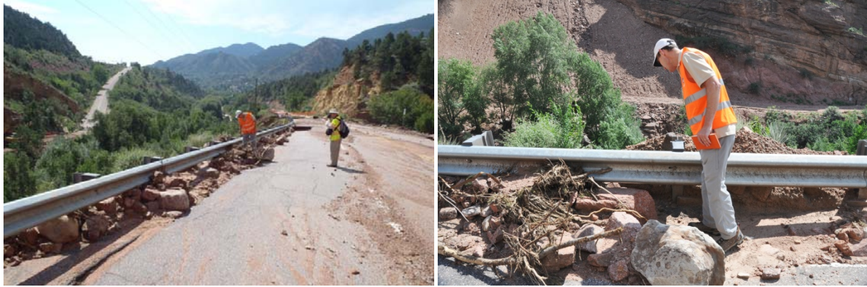
Figure 3.2.19. Debris-clogged guardrail on Manitou Avenue (old US 24). View south from +38.8691° N, -104.9255° W, approximate elevation 6573.
