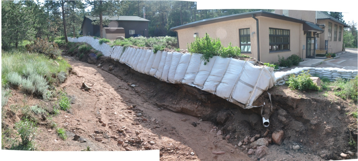
Figure 3.4.9. Unnamed Creek 3 in the lower part of the alluvial fan adjacent to the Ute Pass Branch Library in the Town of Cascade. Panorama view looking northeast; white objects lining the channel are fabric bulk handling bags that are somewhat similar to saddle bags that are able to straddle a ridge or cable. Vegetation growing on soil filling the bags indicates that these bags were in place at the time of the August 9, 2013, flood. This location is just above the intersection point on the Cascade alluvial fan. View from 38.8968^{\circ} N, -104.9702^{\circ} W, approximate elevation 7405 ft
