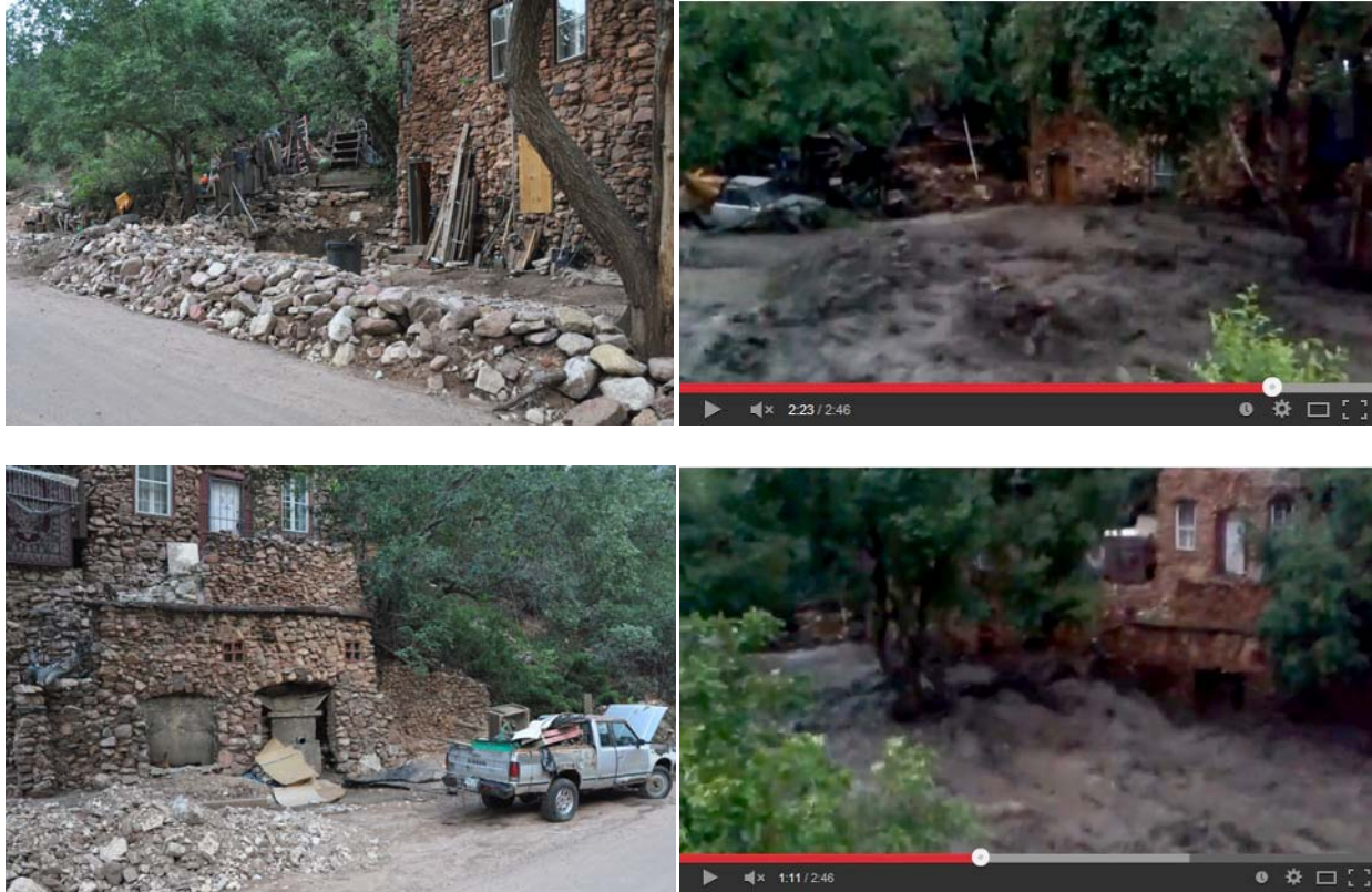
Figure 3.3.6. Stone-and-mortar residence in Williams Canyon north of US 24. Top left and bottom left: photos of residence taken on August 16, 2013. Top right and bottom right: screenshots of YouTube video by Dave McCrary taken on August 9, 2013; Video 1 in Figure 3.3.1. Flood flow is partway up the wall of the residence. Top: door and boarded window in left photo correspond to door and window with white trim in right photo; flow appears to be below the middle of the window. Bottom: distinctive white-trimmed windows and white door above horizontal dark line in left photo are visible in right photo; flow appears to be about the level of the boarded doors in the left photo. Camera location: +38.8641^{\circ}\text{N} , -104.9173^{\circ}\text{W} , elevation 6472 ft.
