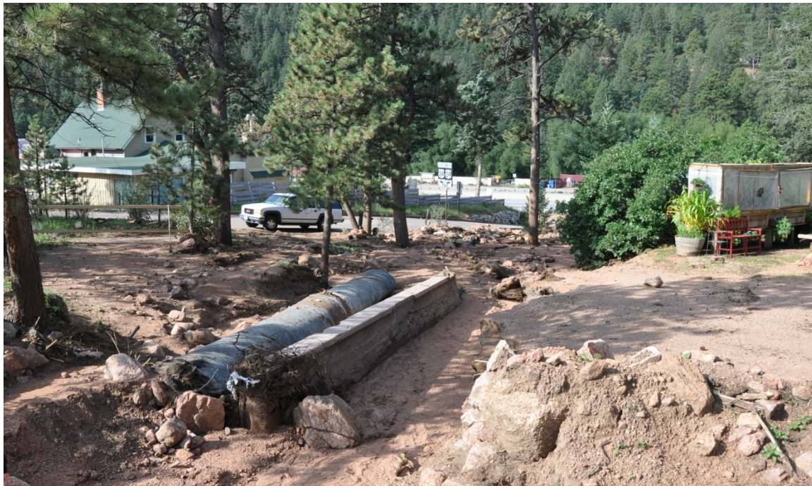
Figure 3.4.8. Unnamed Creek 3 at its intersection point in the lower part of the alluvial fan in the Town of Cascade. Top: panorama view looking northeast (left side) to southeast (right side) from a point near Ute Pass Avenue and Severy Road. Bottom: view looking southwest at exposed concrete wall and oval corrugated metal pipe culvert at a driveway from Severy Road (white truck) to the right side of photo. Camera location for top view 38.8965^{\circ} N, -104.9705^{\circ} W, approximate elevation 7367 ft; camera location for bottom view 38.8968^{\circ} N, -104.9702^{\circ} W, approximate elevation 7405 ft.
