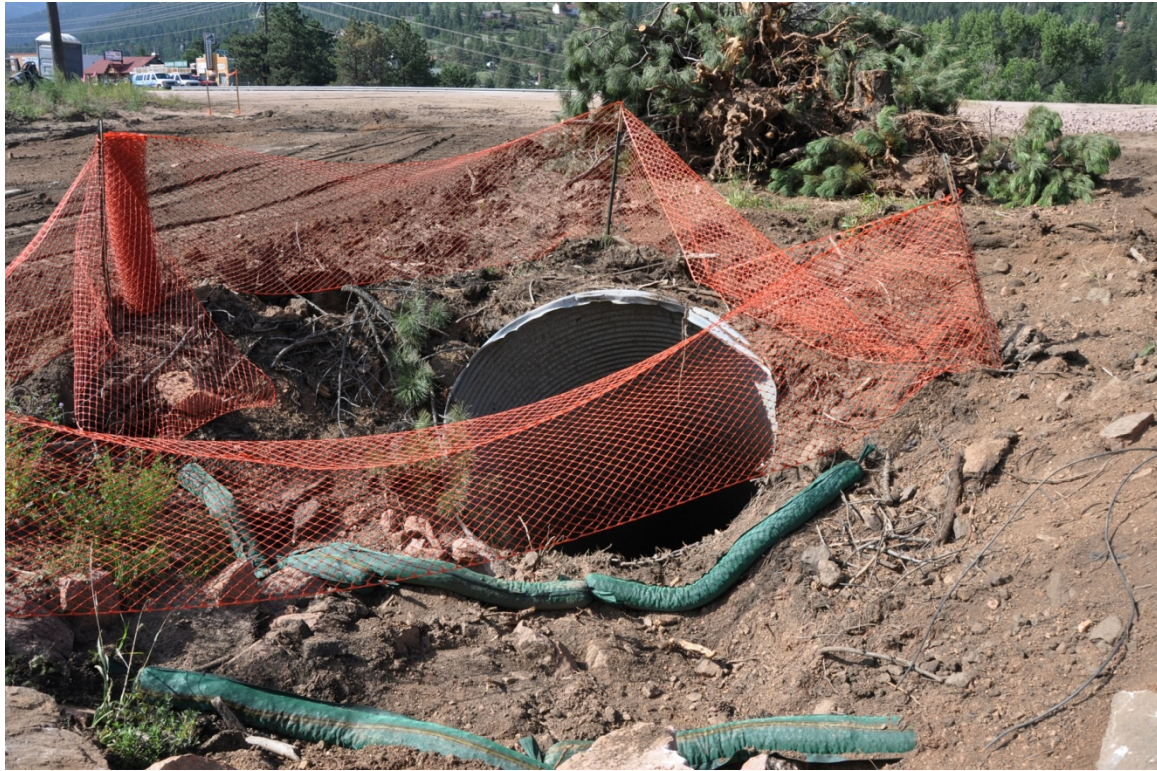
Figure 3.4.19. Inlet to existing corrugated metal pipe culvert at Wellington Gulch. View toward the southwest at US 24 from 38.9185° N, -104.9838° W, approximate elevation 7597 ft.
