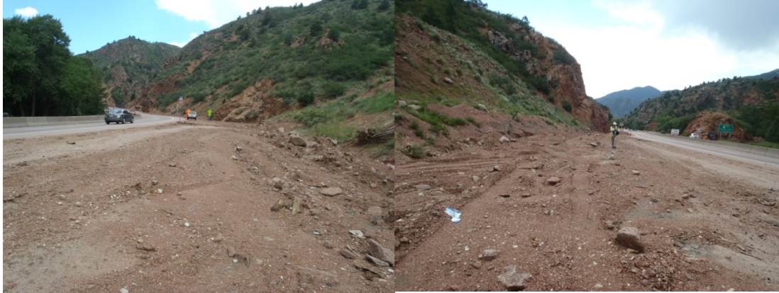
Figure 3.2.10. Looking northwest (left) and southeast (right) from relative high ground along shoulder of westbound US 24. US 24 super-elevation is visible to the left in the left image. Wide shoulder is visible in both images. Camera location: +38.8757^{\circ} N, -104.9295^{\circ} W, approximate elevation 6686 feet. Waldo Canyon is in the distance above car on highway in left image. The earth embankment toe visible in the foreground on the right side of the left image is a placed earth fill of uncertain purpose (see Figure 3.2.9 for aerial oblique view); it could be a stockpile in a material site and may indicate wider DOT Right of Way. Right image shows flattening of highway grade, wide shoulder, and the earth fill embankment toe. The westbound on-ramp is at steeper grade and just beyond the person. The eastbound off-ramp is near the cars and highway sign on the right side of right image.
