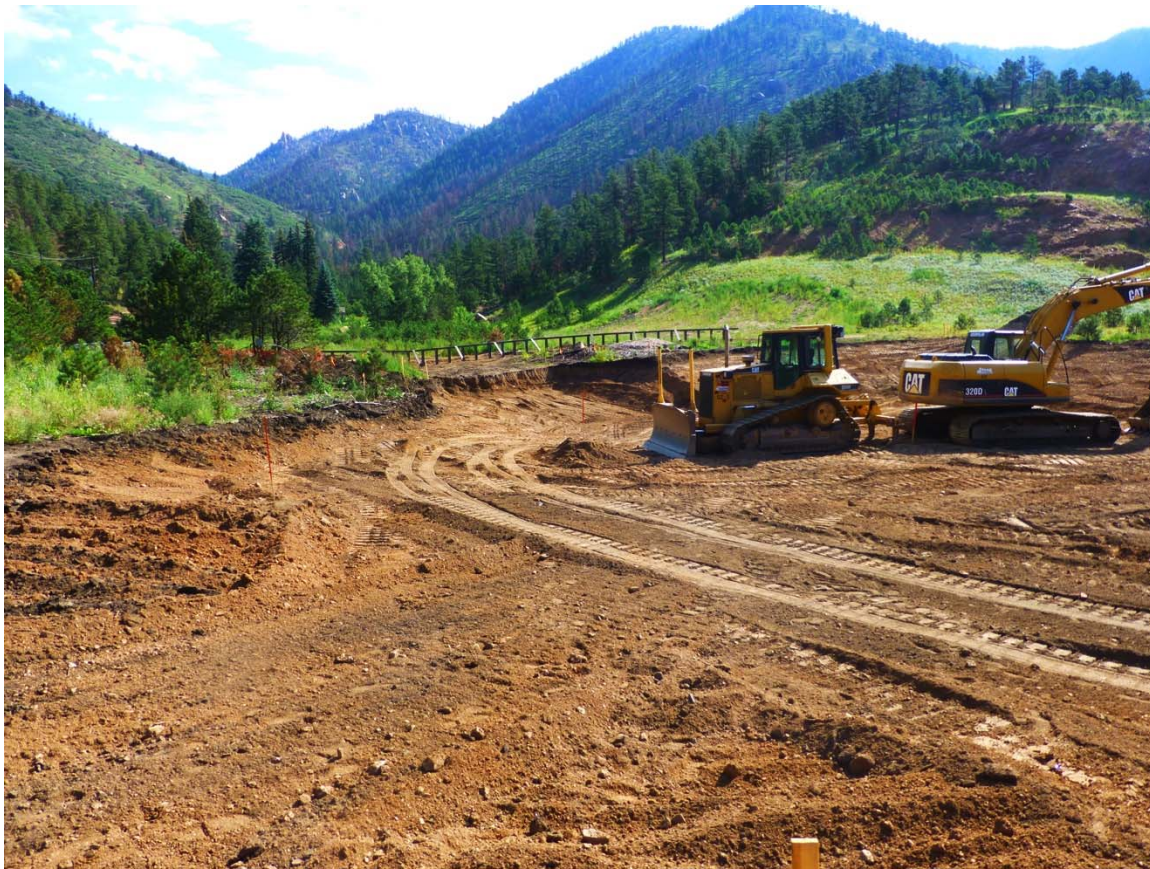
Figure 3.4.18. Sediment basin excavation downstream of debris rack. This basin is not intended as a large capacity storage area, but more as a stilling basin to allow debris and larger particles to drop out in a controlled manner without clogging the drainage culvert inlet. View toward east from 38.9185° N, -104.9840° W, approximate elevation 7597 ft.
