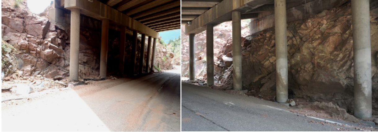
Figure 3.2.13. Southeast abutment of US 24 overpass of Manitou Avenue just before the on-ramp to westbound US 24. Left: view from the east side; note that splash marks go clear to the top of the closest bridge pier and that the flow line itself can be seen about mid-height, and decreasing at subsequent piers farther west. Right: view from the west side; the muddy water mark is easier to see on the cut slope behind the piers; splash marks on the east sides of the piers and the shape of the water mark on the west sides suggests that the water flow was high velocity. Camera position for left photo is +38.8711° N, -104.9257° W, approximate elevation 6651 feet.
