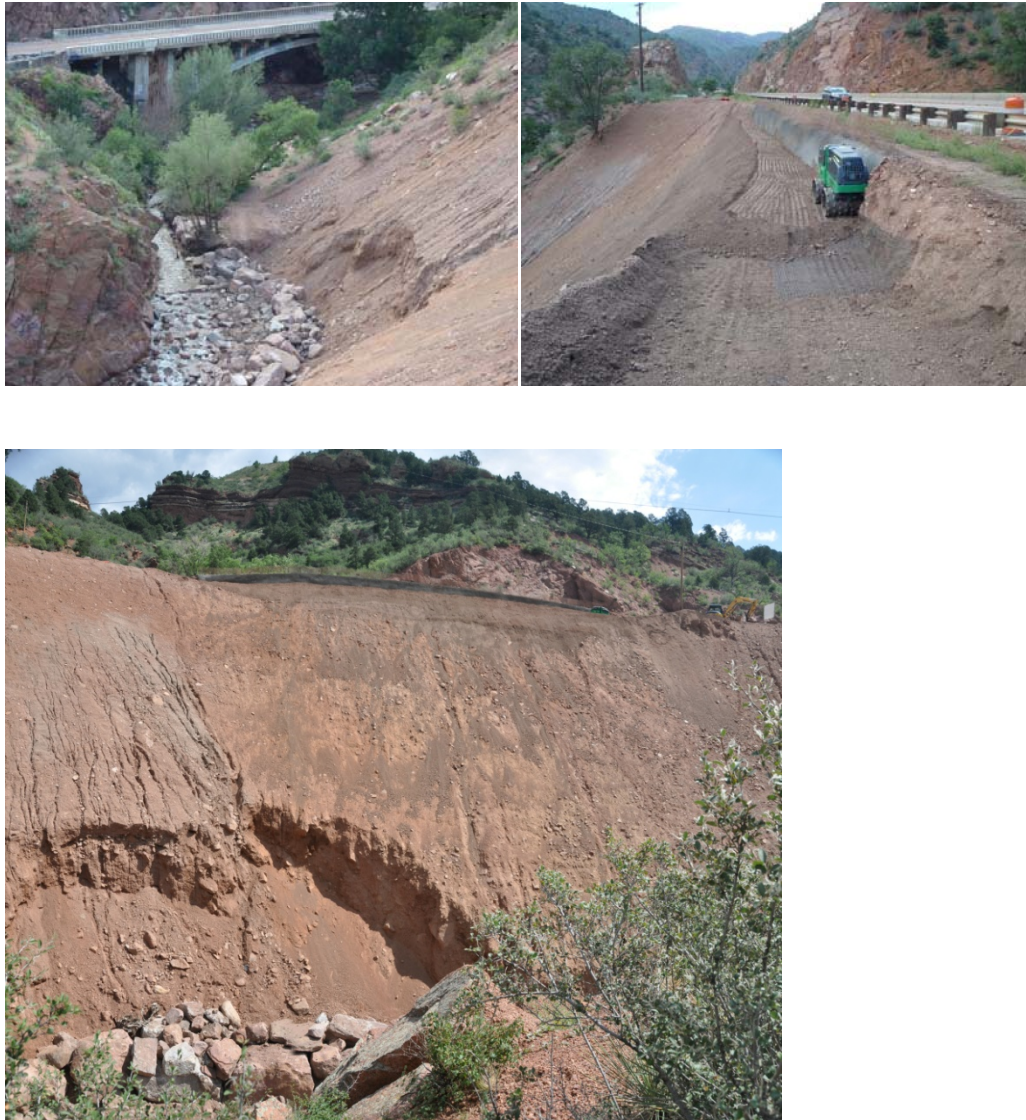
Figure 3.2.23. Riprap and rilling on eastbound US 24 embankment, and Geogrid reinforcement with shotcrete and chain-link facing at crest of embankment. Top left: view to the northwest from +38.8695^{\circ} N, -104.9245^{\circ} W, approximate elevation 6583 feet; Fountain Creek Bridge that carried flood and debris from Waldo Canyon is in the background. Top right: view to the north from +38.8695^{\circ} N, -104.9245^{\circ} W, approximate elevation 6583 feet. Bottom: view to the east from 38.8695^{\circ} N, -104.9250^{\circ} W, approximate elevation 6564 feet; the small green soil compactor visible in the top right photo also is visible in the bottom photo.
