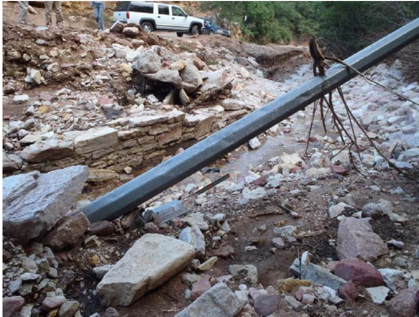
Figure 3.3.3. View looking south (downstream) from the bottom of Williams Canyon near the end of Cañon Avenue at Geneva Trail. Vehicles are parked on Cañon Avenue. Leaning metal feature is a light pole that has a tree branch hanging on it; above the tree branch is smooth steel, whereas dents are present in the pole below the tree branch providing an indication of maximum flood depth. Grouted riprap is visible in the middle-right part of the photo, and gabion baskets are visible at the end of the grouted riprap to the right of the vehicles. Camera location: +38.8655° N, -104.9178° W, elevation 6522 ft.
