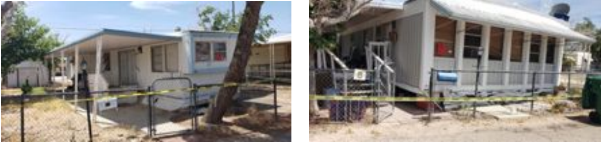
Figure 45. Collapsed mobile homes in Ridgecrest after M7.1 event (35.6444, -117.6733) Photo credit: Jawad Fayaz
