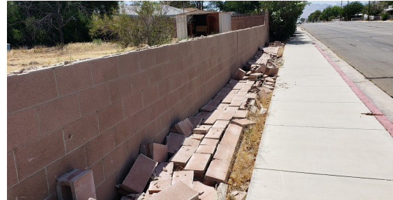
Figure 48. Damages to Masonry components after the M7.1 event (a: 35.7595, -117.7357, b: 35.7592, -117.3766, c: 35.7595, -117.7357, d: 35.6444, -117.6720) Photo credit: Christine Goulet and Jawad Fayaz
