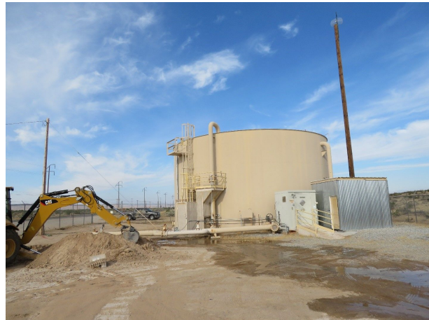
Figure 26. Hilltop Tank elephant foot buckle, pipe repair and continued leaking (35.6260, -117.5916).
