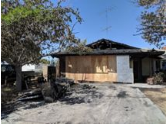
Figure 43. Damaged wood-frame house due to gas leak fire in Ridgecrest (35.6202, -117.6612) Photo credit: Farzin Zareian
