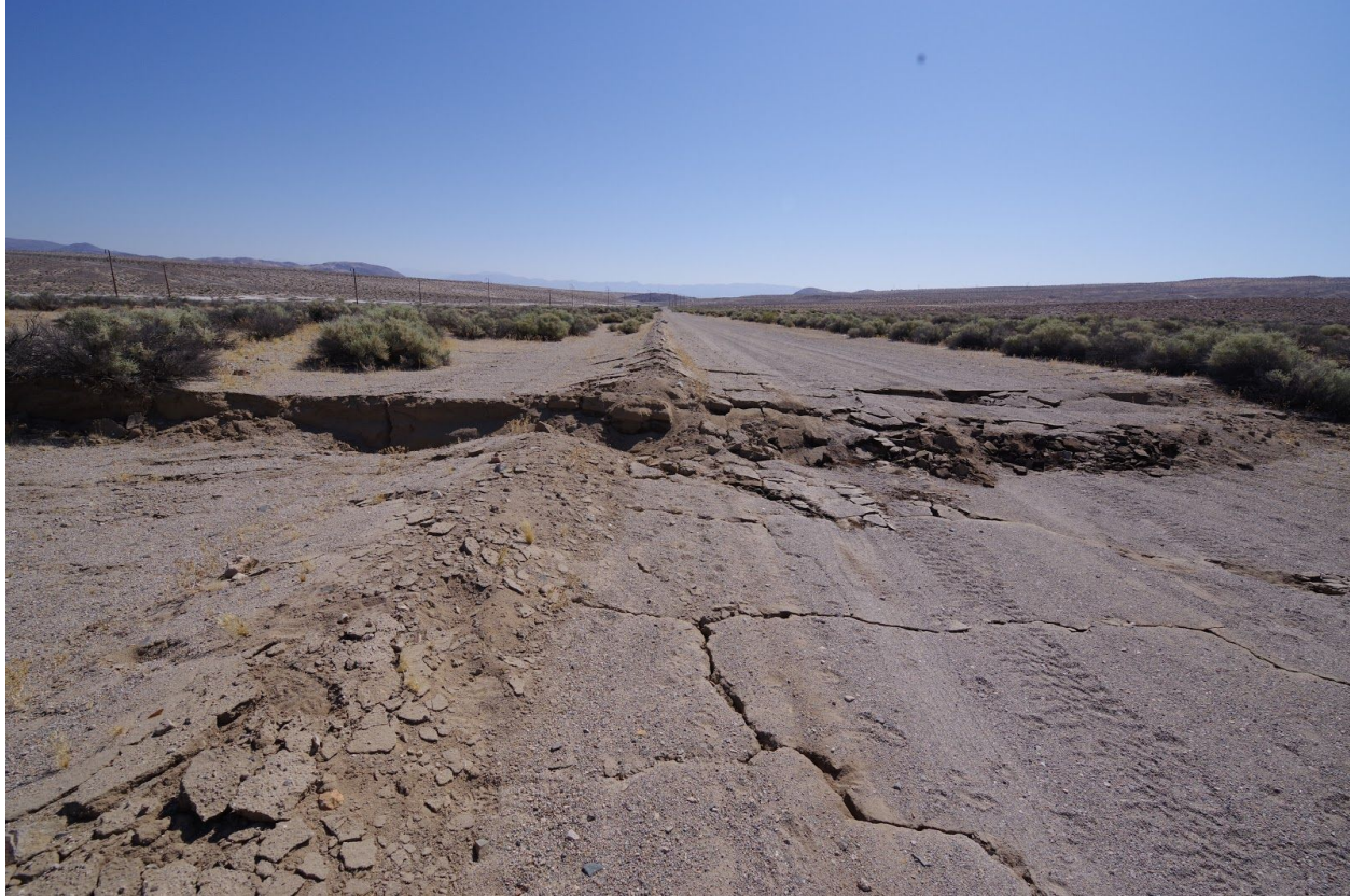
Figure 22. Fault rupture from the M7.1 event showing at a road crossing south of Highway 178 (35.6468, -117.4800). Photo credit Scott Brandenburg.
