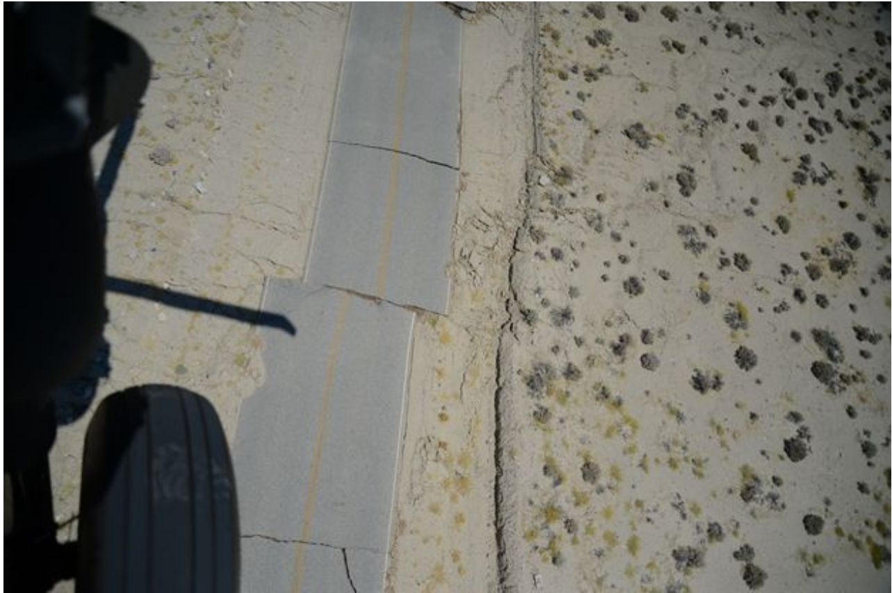
Figure 7. Helicopter Overflight Viewing Access Road Fault Offset. The CGS and USGS, along with National Guard and Navy personnel, view road damage showing 2.5 \pm 0.2 meters of right-lateral motion along the primary rupture associated with the magnitude 7.1 event. This offset access road was broken by the mainshock fault rupture about 600 m southeast of the China Lake playa (Credit: Ken Hudnut, USGS. Public domain)
