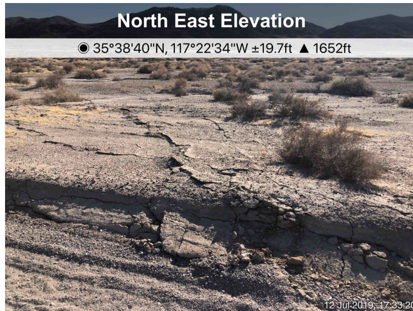
Figure 25. Example of cracks observed along Pinnacles Road. This specific picture was taken at zone 3 and shows where the cracks cut the Pinnacles Road.
