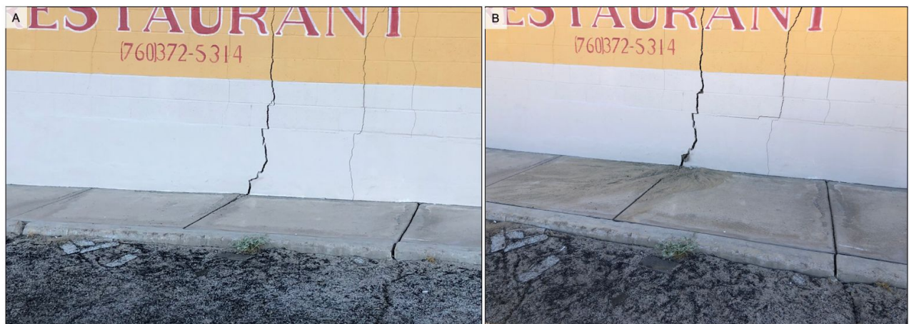
Figure 34. Esparza Restaurant building in Trona that exhibited cracked walls, (A) After the M6.4 earthquake and before the M7.1 and (B) after the M7.1 earthquake. Following the M7.1 earthquake, the horizontal and vertical cracks widened, the roof showed damage and a sand boil appeared at the base of the crack shown in the photo. Photos by Christine Goulet (35.7595, -117.3757).
