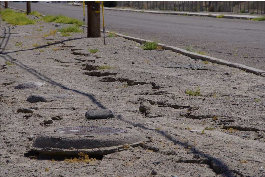
Figure 32. Ground cracks due to liquefaction-induced lateral spreading in Trona. Photo by Scott Brandenburg, (35.7626, -117.3731).
