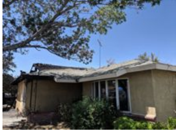
Figure 43. Damaged wood-frame house due to gas leak fire in Ridgecrest (35.6202, -117.6612) Photo credit: Farzin Zareian
