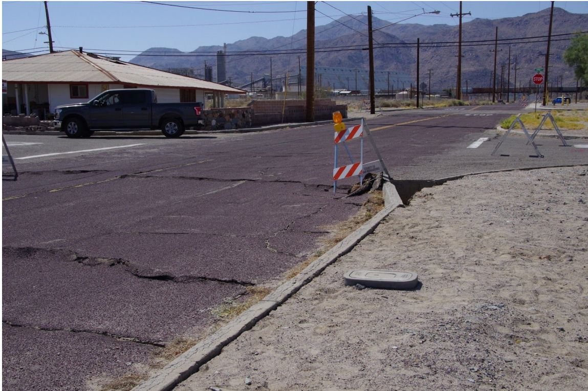
Figure 33. Ground compression, including buckled curb, due to liquefaction-induced lateral spreading in Trona. Photo by Scott Brandenburg, (35.7623, -117.3725).
