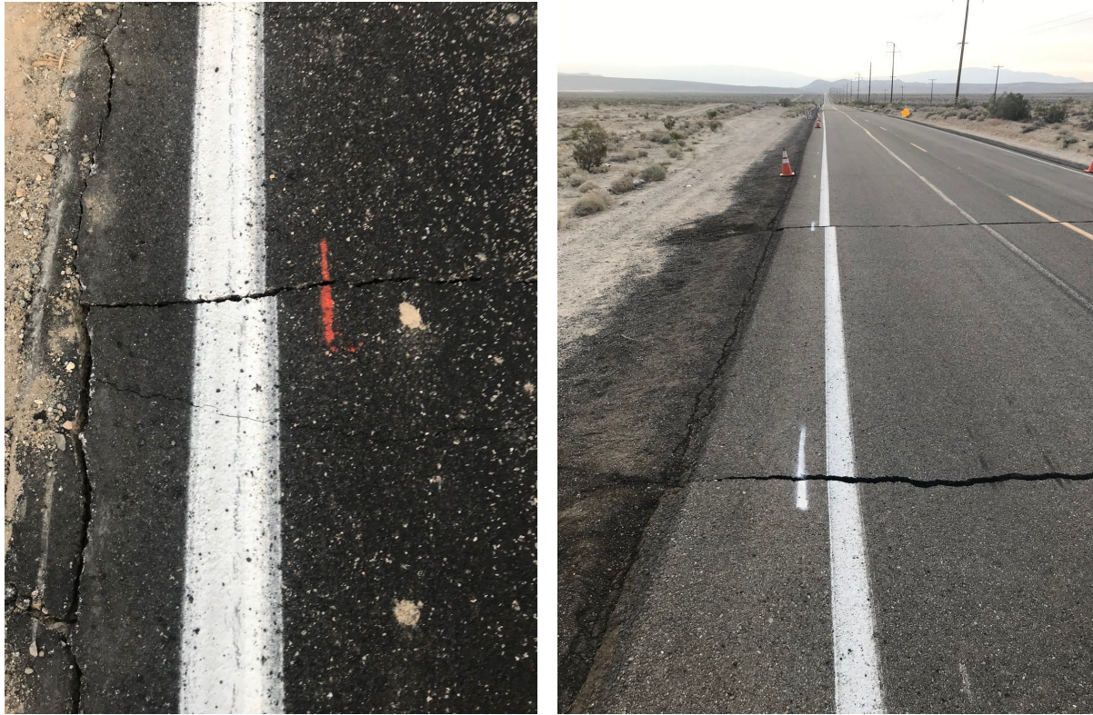
Figure 11. Pavement of Highway 178 offset by M6.4 event fault rupture (shown by white lines) and short painted lines used to monitor afterslip. Locations: Left 35.649, -117.4824 (red line), Right 35.6441, -117.537 (white line). Photo credits: Ben Brooks, USGS
