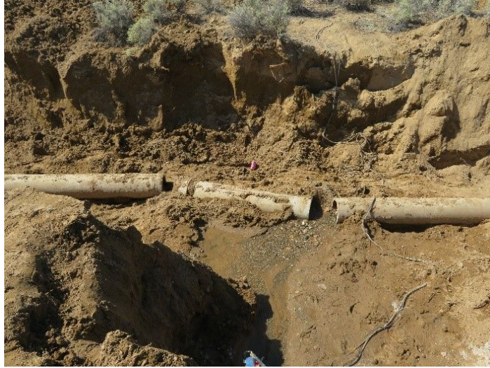
Figure 28. Offset of buried concrete segmented pipeline crossing the M7.1 surface fault rupture. (35.6492, -117.4822).
