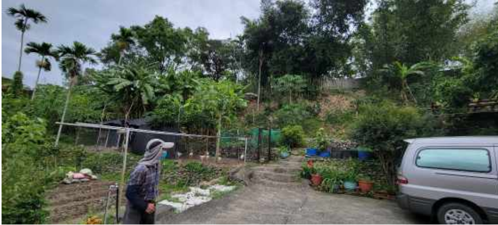
(b) View uphill following presumed trace of fault seen via cracks in pavement. Lat: 23° 10' 28.918199", Lon: 121° 14' 54.926159"
