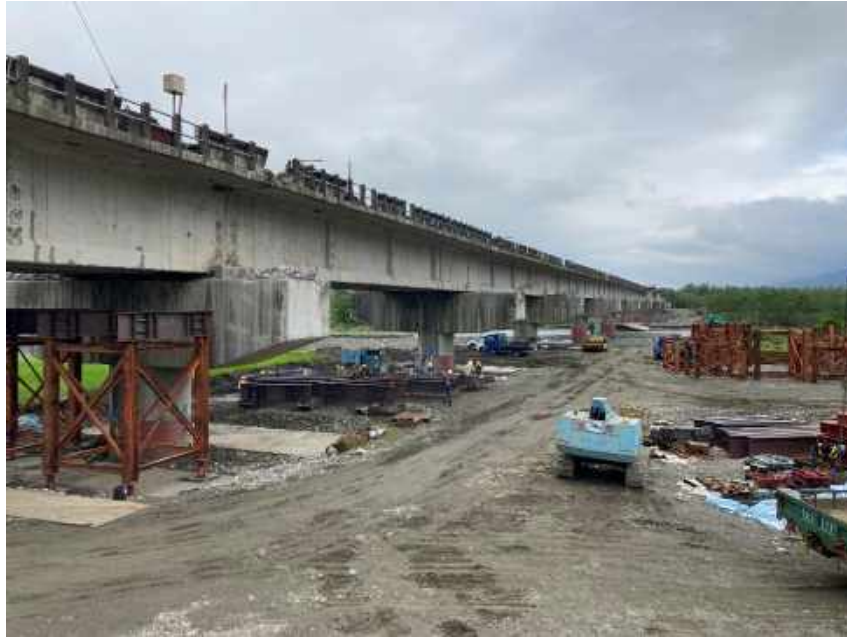
Figure 5.23. View of the Dongli Railroad Bridge during active repair operations. (23.27487° 121.30530°)
