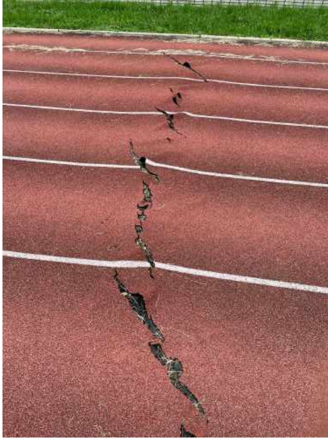
Figure 4.41: En-echelon tension cracks rupturing the track at the Yuli High School athletic field. Lat: 23° 20' 31.715519", Lon: 121° 19' 11.219520"
