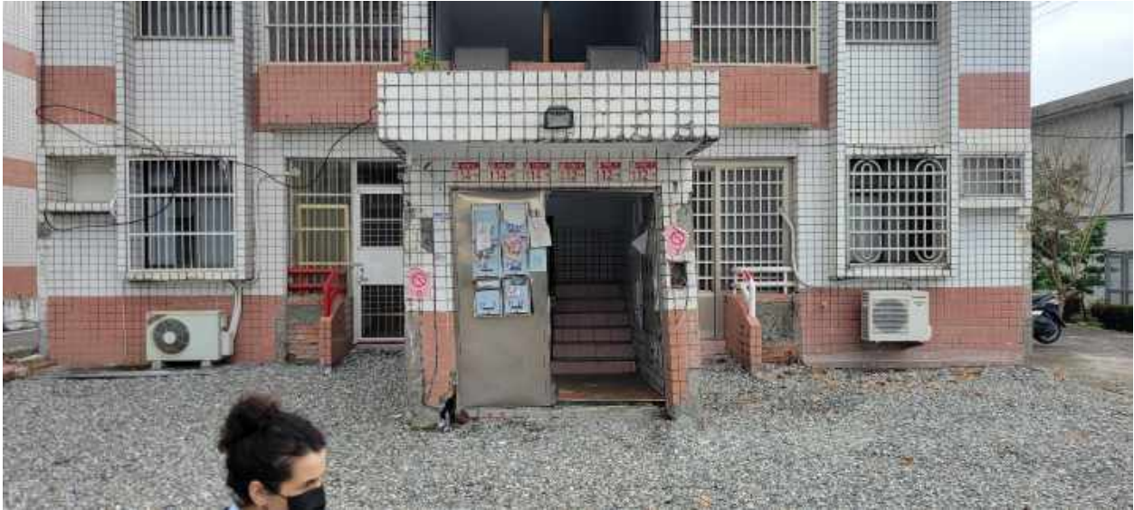
Figure 4.39: Red-tagged structure along path of fault trace. Lat: 23° 20' 20.139000", Lon: 121° 19' 2.544479"
