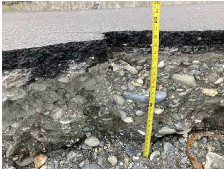
Figure 5.44. Typical profile of backfilled soils (23.38509° 121.34773°)
