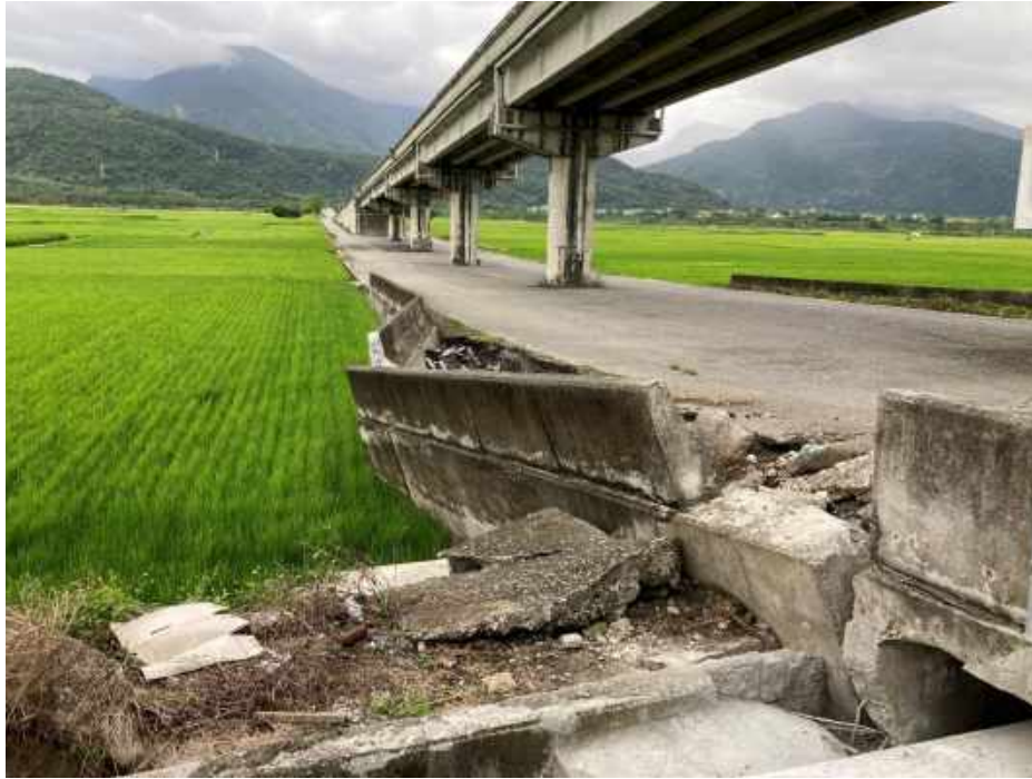
Figure 5.16. Looking west at a bridge main span with a built-up earthen berm in the background. Note the concrete shear keys at the ends of the pier caps retaining the prestressed girders. (23.26477° 121.30019°)
