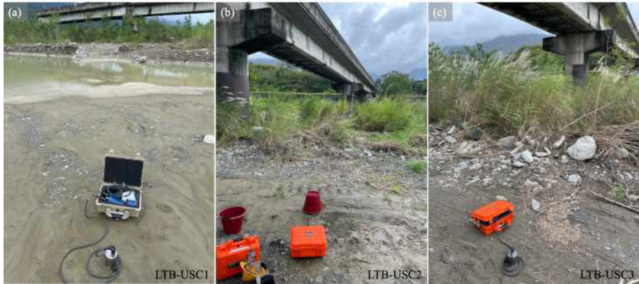
Figure 2.4. Photo of sensor setup at Luntian bridge. (a) LTB-USC1; (b) LTB-USC2; (c) LTB-USC3.
