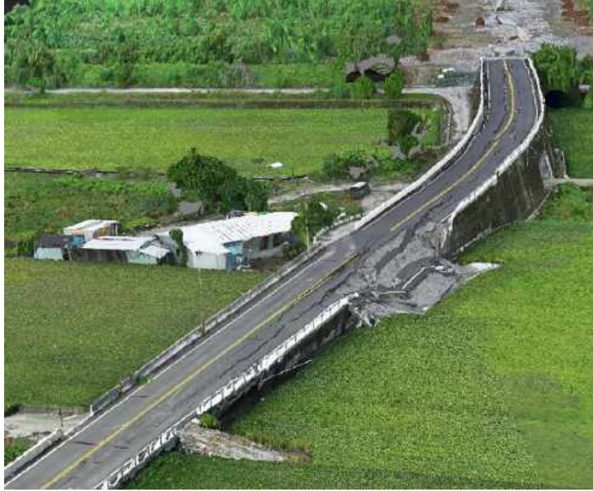
Figure 5.40. Drone view of the east abutment looking west (approx. 23.38481° 121.34911°)
