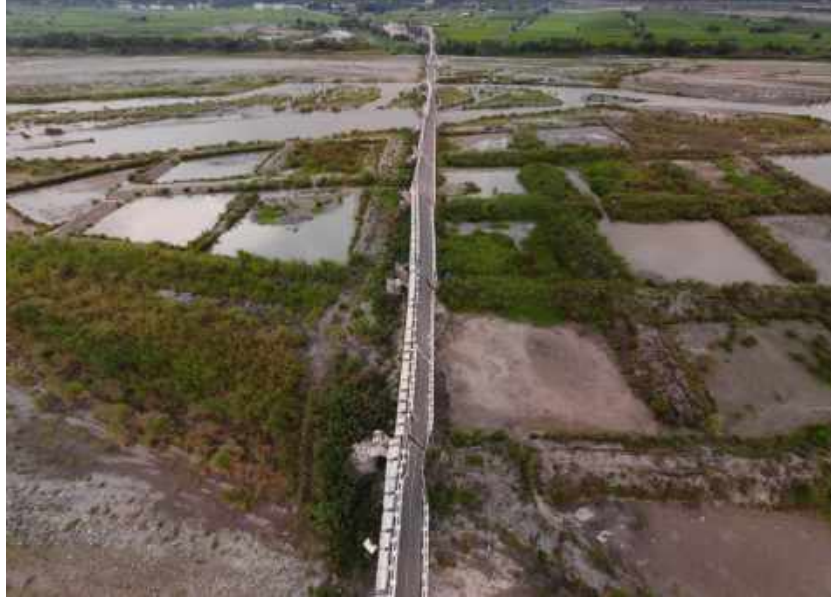
Figure 5.32. Failed spans of the Gaoliao bridge looking west (Image courteous of Zola Zhou, 23.38563° 121.34458°)
