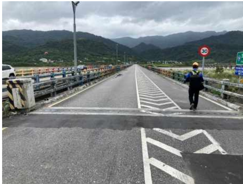
Figure 5.27. View from the west abutment of the south Yuli bridge. ( 23.32332^{\circ} 121.32684^{\circ} )
