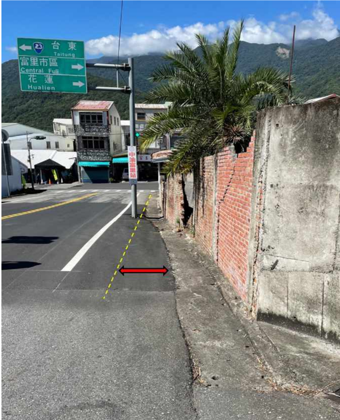
Figure 4.24: West-looking view of offset sewer lateral and brick wall. Total LL offset is ~90 cm, which may include creep and/or surface rupture on the LVF that occurred prior to the September earthquake.
