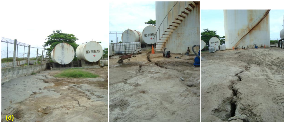
(d) Three view of fuel tanks and multiple ground fissures due to wide spread liquefaction [06/20/2009, 3:12PM, N15.846936, W87.963225]
