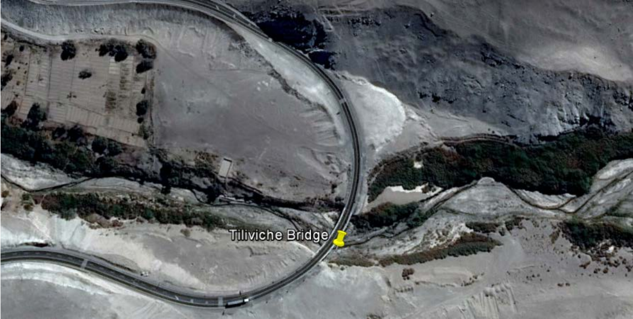
Fig. 3.2 Google Earth image of the curved Tiliviche Bridge composed of three simply supported segments (-19.551966°, -69.940921°).
