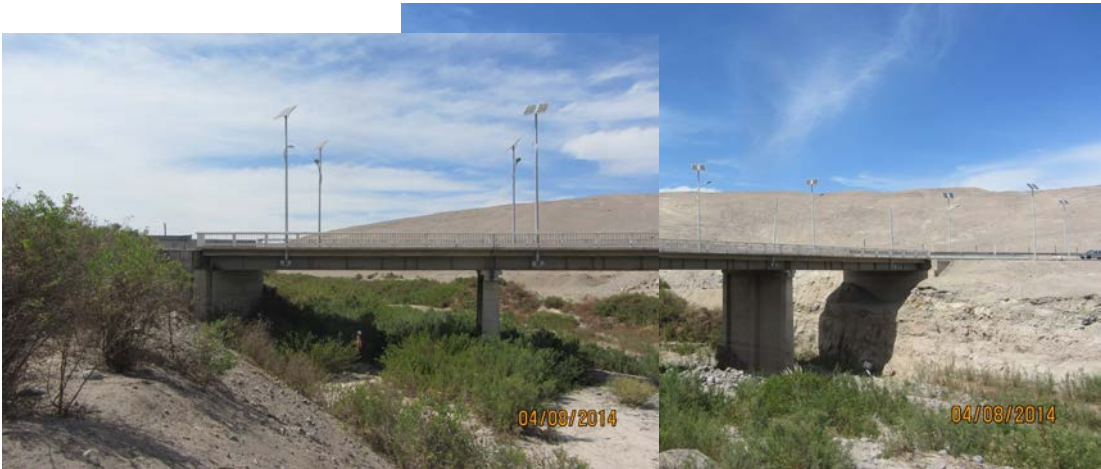
Fig. 3.3. Photo of the Tiliviche bridge elevation (-19.551966°, -69.940921°).
