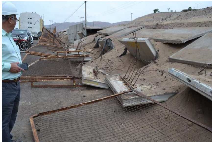
Fig. 4.9. Failure of retaining walls in the upper level and backfill displacements (20.273889°, - 70.123889°) (photograph courtesy of Ramon Verdugo)
