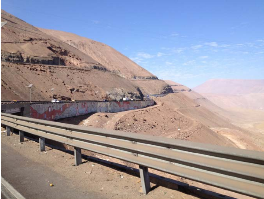
Fig. 6.9. Undamaged Mechanically Stabilized Earth (MSE) retaining walls adjacent to steep slopes (-20.251279°, -70.116173°)
