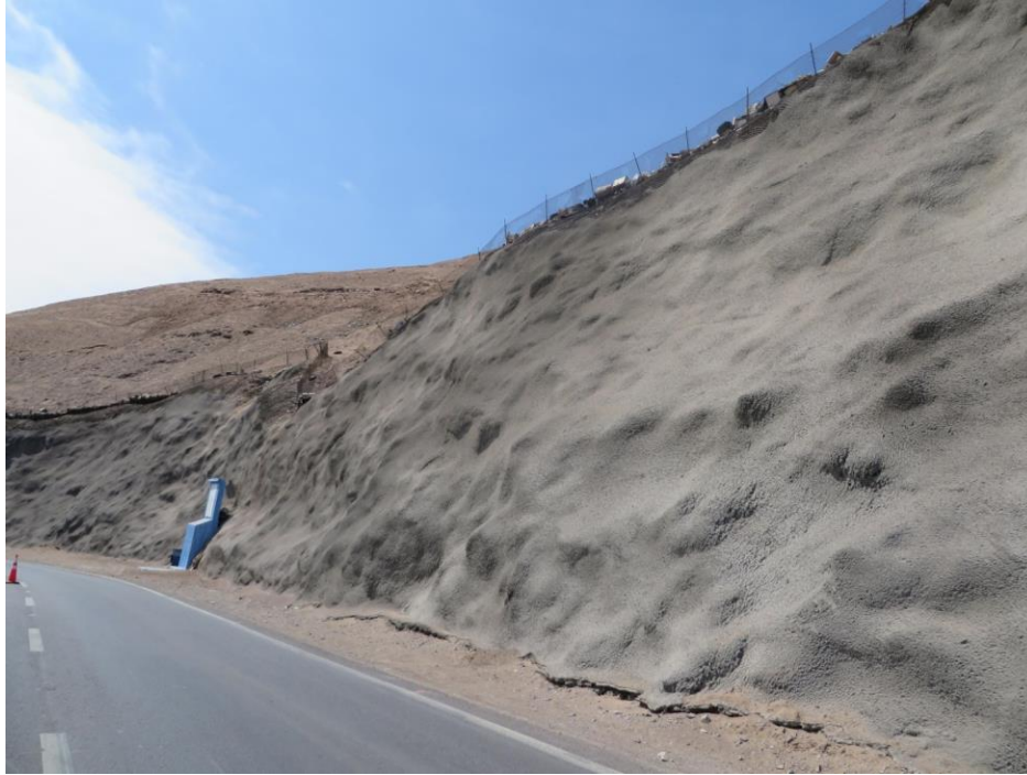
Fig. 6.8. Undamaged steep cuts stabilized with wire mesh and shotcrete (-20.263819°, -70.112042°)
