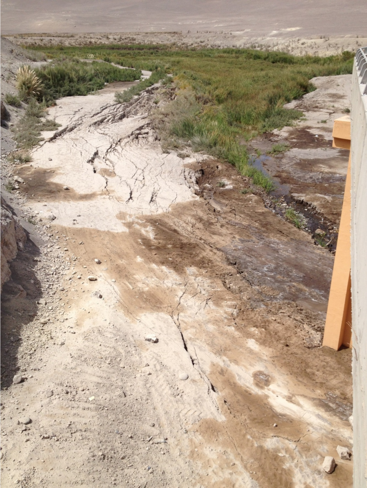
Fig. 3.11. Photograph showing lateral spreading running parallel to stream channel flowing under the Tana bridge. (19.454013°, -69.946349°)
