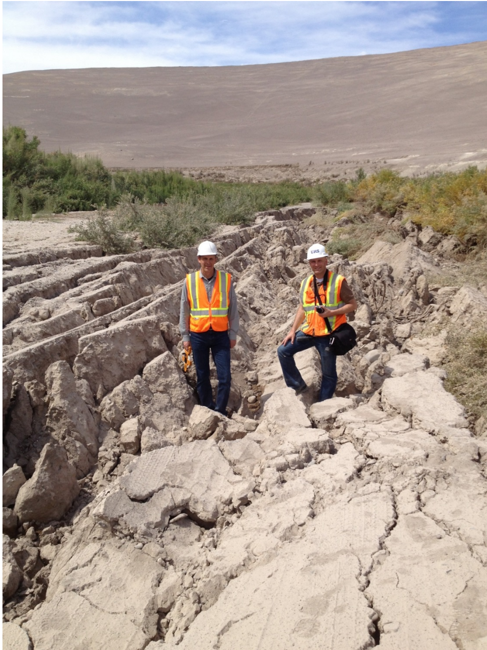
Fig. 3.12 Photograph showing closer view of lateral spreading running parallel to stream channel flowing under the Tana bridge. (19.454418°, -69.945864°)
