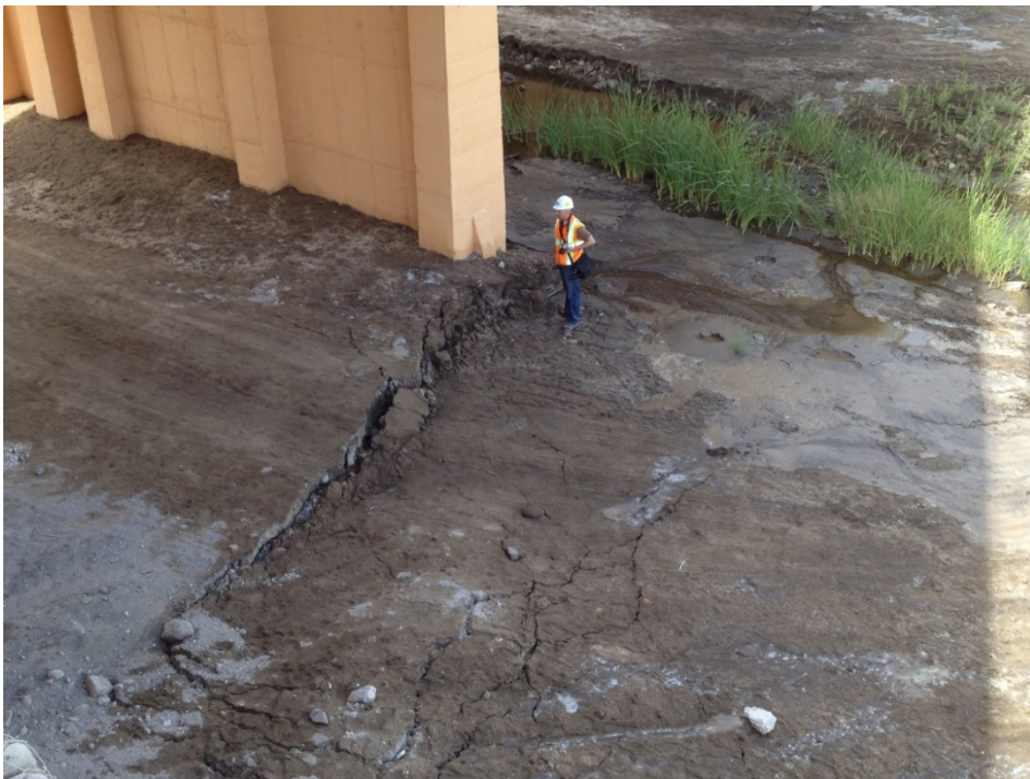
Fig. 3.10 Photograph showing settlement of soil adjacent to bridge pier as a result of liquefaction. (19.454245°, -69.946399°)
