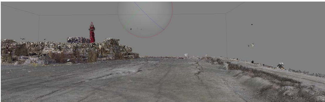
Fig. 2.16 Screenshot of cracking and slumping at the pier surface from the dense point cloud
