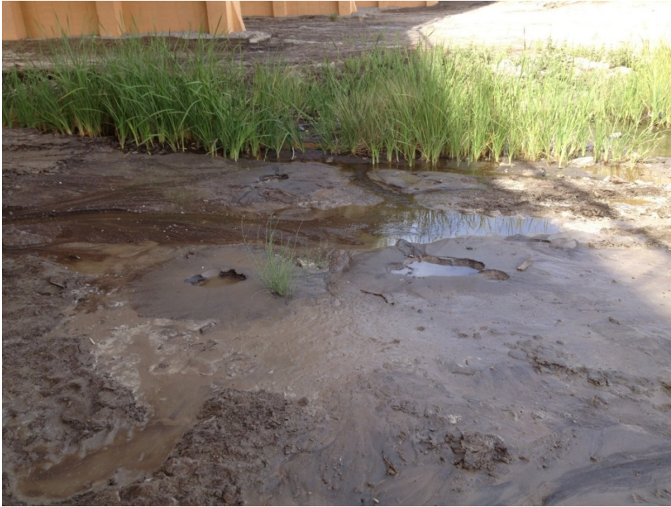
Fig. 3.9 Photograph of sand boils adjacent to small stream flowing beneath the Tana bridge. (19.454245°, -69.946399°)
