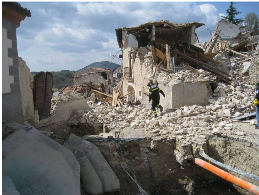
Figure 4.6. At the highest elevation of the hilltop town of Castelnuovo, almost all of the structures collapsed (D5) or were near collapse (D4). (42.2947°, 13.629°)
