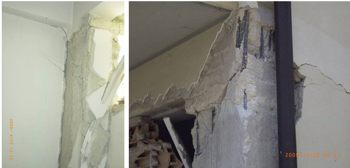
Figure 4.52. Example of D3 damage in the building at waypoint GB-88-1.
