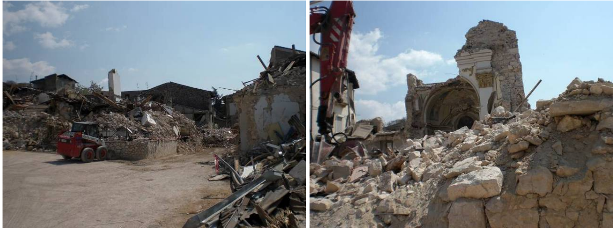
Fig. 4.19. San Gregorio: (a) view of the historic center with collapsed masonry buildings; (b) remains of the church
