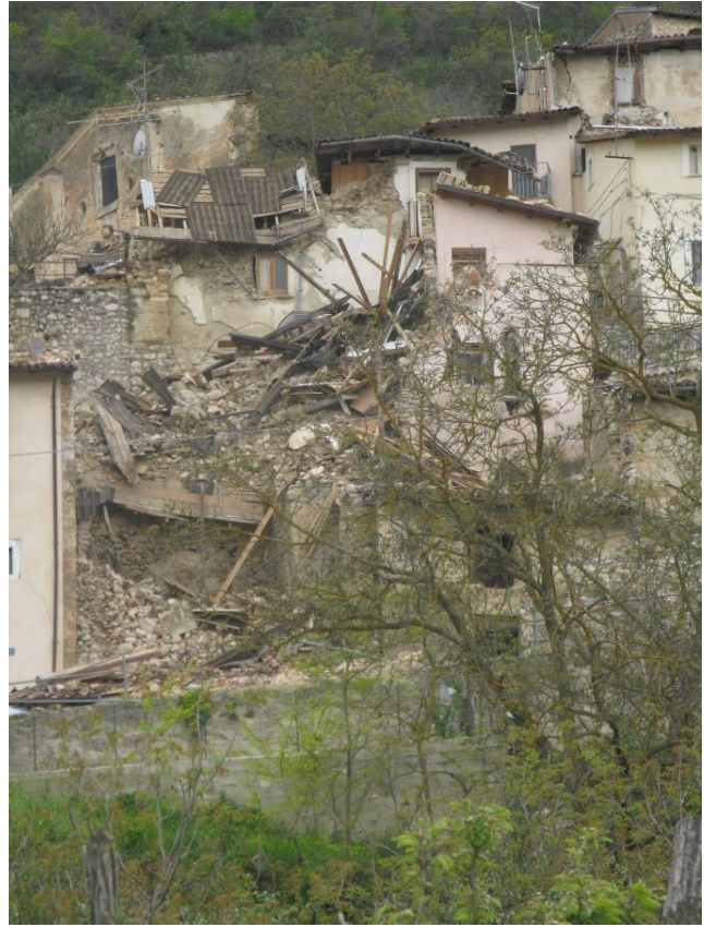
Fig. 4.29. Casentino: (a) partial collapse of the masonry building at the entrance of the village (b) collapse of old poor quality masonry buildings in the historic center.
