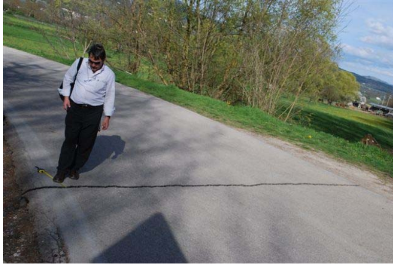
Figure 5.30. Characteristic crack developed in bridge approach road directly south of Onna, at distances of 15 m to 160 m from the Aterno River (42.324N, 13.478E).
