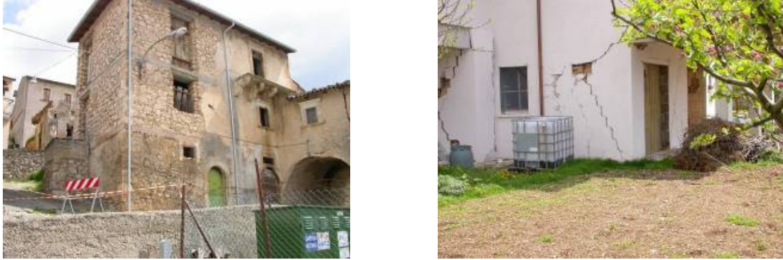
Fig. 4.43. Barisciano: (a) collapse (D5) of an old masonry building in background; (b) damages (D1/2) to RC buildings.
