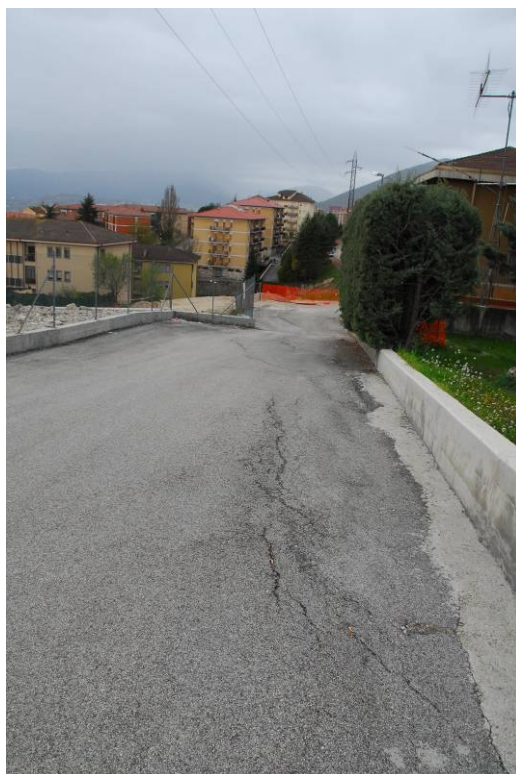
Figure 5.43. Cracks in the overlying asphaltic surfaces and a narrow settlement trend along the sidewall of the cut-and-cover structure (42.358N 13.415E).
