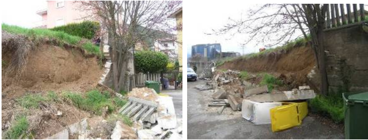
Figure 6.18. Toppling of masonry retaining wall at the outskirts of L'Aquila (42.366803°N, 13.376561°E).
