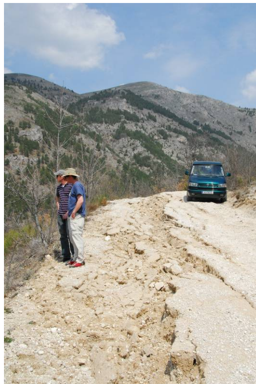
Figure 5.28. Failure of side-hill fill embankment (42.420N 13.376E).
