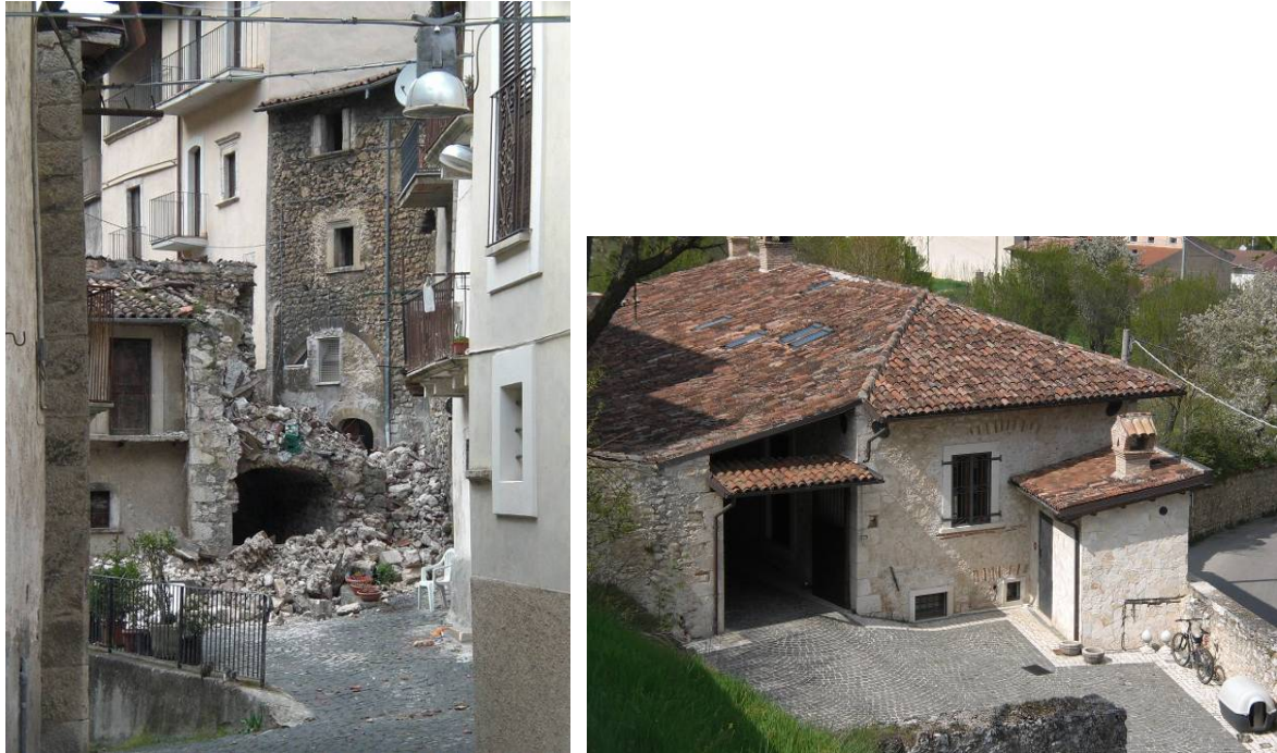
Fig. 4.24. Fossa: (left) collapse of masonry constructions in the historic center; (right) strengthened masonry construction with no damage.
