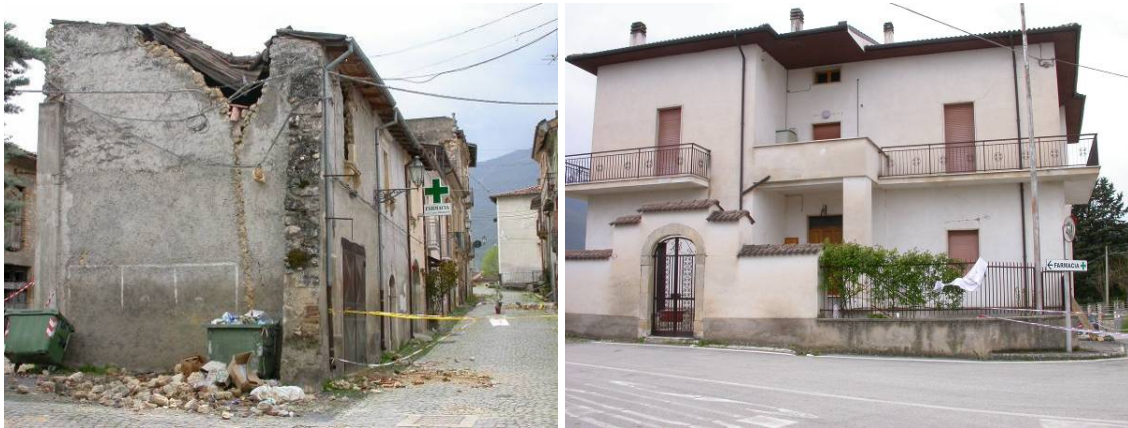
Fig. 4.26. S. Eusanio Forconese village: (a) partial collapse of masonry building (D4) and (b) slight damage to a RC building nearby (D1).
