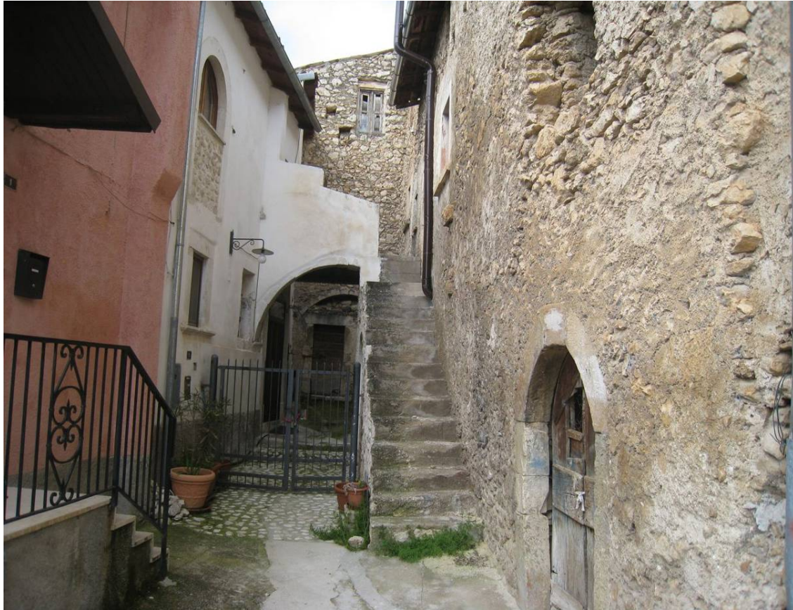
Figure 4.9. Typical unreinforced masonry structures in the village of San Pio delle Camere suffered no damage (D0), or slight cracking (D1). Structures in this village are similar to those in Castelnovo. San Pio delle Camere is built on limestone bedrock.
