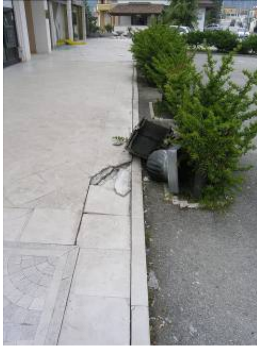
Figure 2.33. Separation cracks at sidewalk on front of building (42.359335°N, 13.468954°E).
