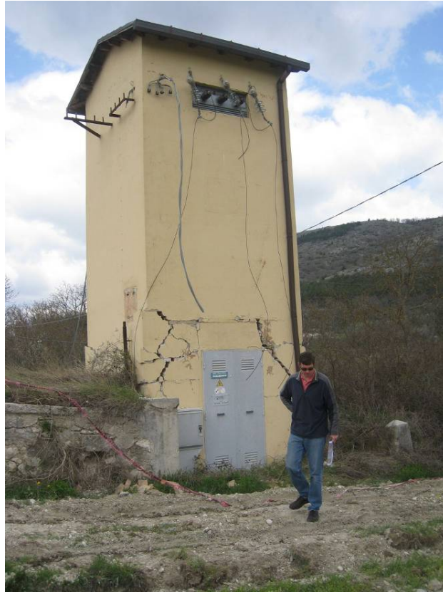
Figure 4.4. Heavily damaged Seismometer station box (not in use at the time of the earthquake, no recording) on the northeast valley beneath the town of Castelnuovo. (42.2982°, 13.6295°).
