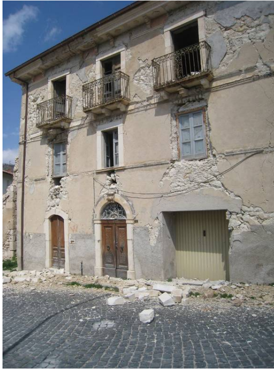
Figure 4.5. A typical heavily damaged structure in the lower elevation of Castelnuovo. Many structures in the lower elevation neighborhood had less observable damage. (42.2956°, 13.6274°)
