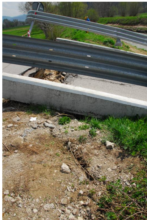
Figure 5.37. Ground cracking in levee directly beneath western abutment along northern side of Aterno River (42.325N, 13.463E).
