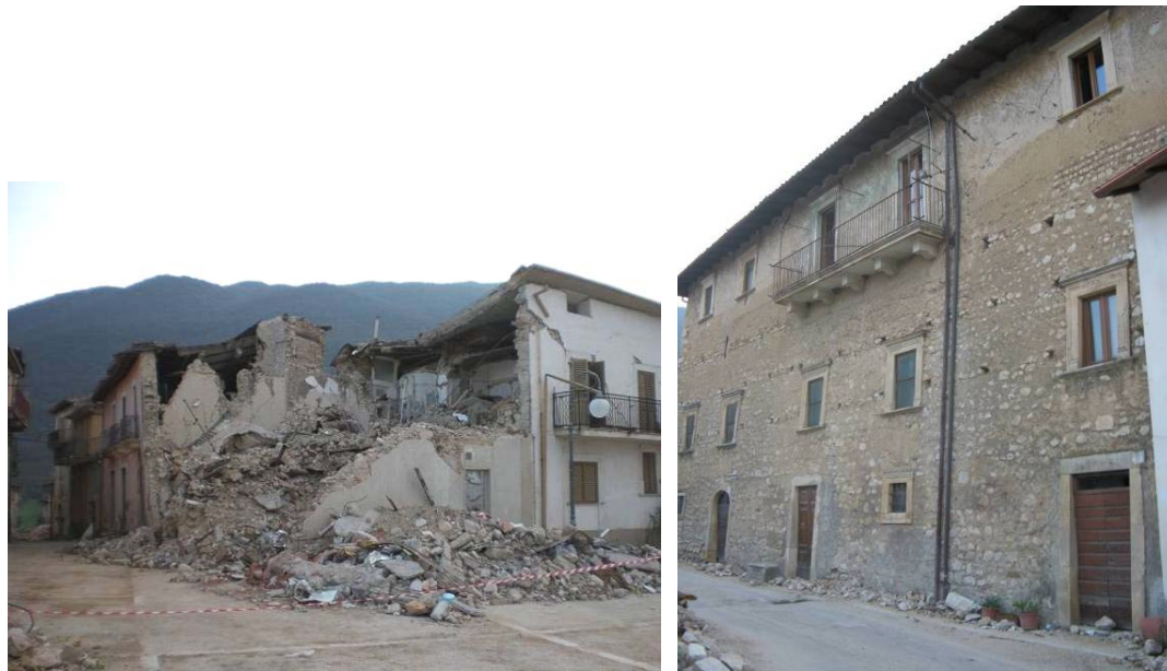
Fig. 4.35. Villa S. Angelo: (a) collapsed masonry buildings (D5) in the historic center; (b) reinforced masonry in the historic center with minor cracks in the highest story (D2).
