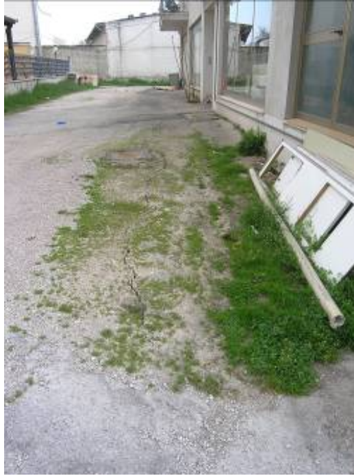
Figure 2.31. Ground fissures at the side of the building (42.359817°N, 13.468649°E).
