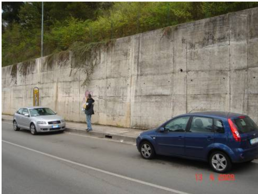
Figure 6.19. Undamaged retaining wall at the city of L'Aquila (42.343672°N, 13.398821°E)
