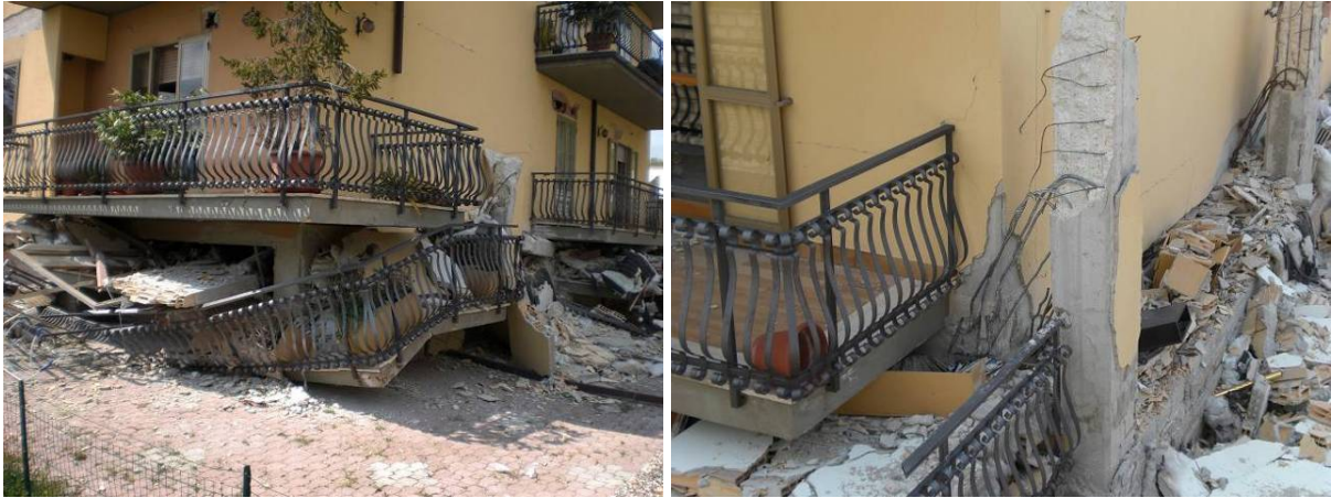
Fig. 4.21. San Gregorio eastern part: (a) RC building “pancake” collapse; (b) detail of sheared pillars.
