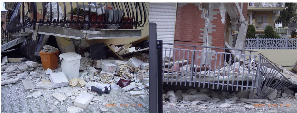
Figure 4.53. Example of D5 damage in the building at waypoints GB-27-1 and GB-28-1.
