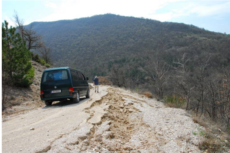
Figure 5.27. Failure of side-hill fill embankment (42.420N 13.376E).
