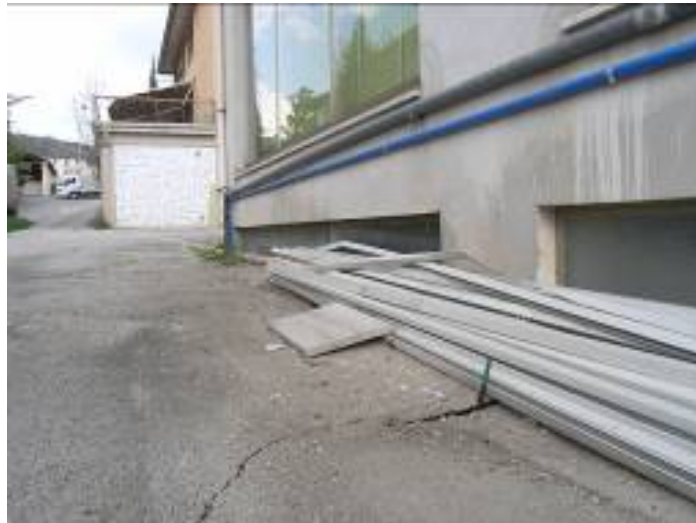
Figure 2.32. Ground fissures and settlement at the side of the building (42.359817°N, 13.468649°E).
