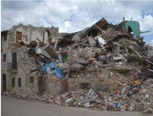
Figure 4.14 Onna: (a) D5 damage level on masonry building structures; (b) D0 damage on a RC building (except for the tilting of the chimney).
