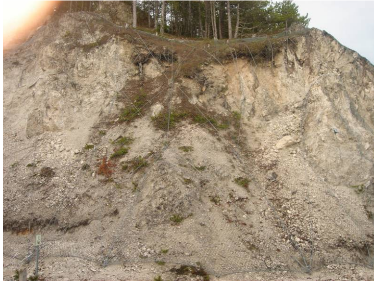
Figure 5.20. Raveling in pervasively fractured/cataclastic limestones on a road cut retained by steel-net protections on SS80 at km 18.2: (DC-18-1) (42.4281N, 13.3460E).
