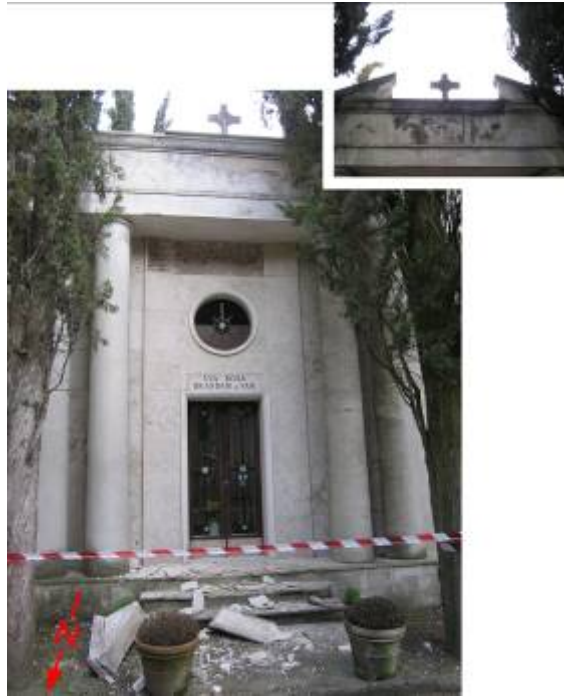
Figure 3.13. Breakage and fall of ornamental objects from a tomb roof.
