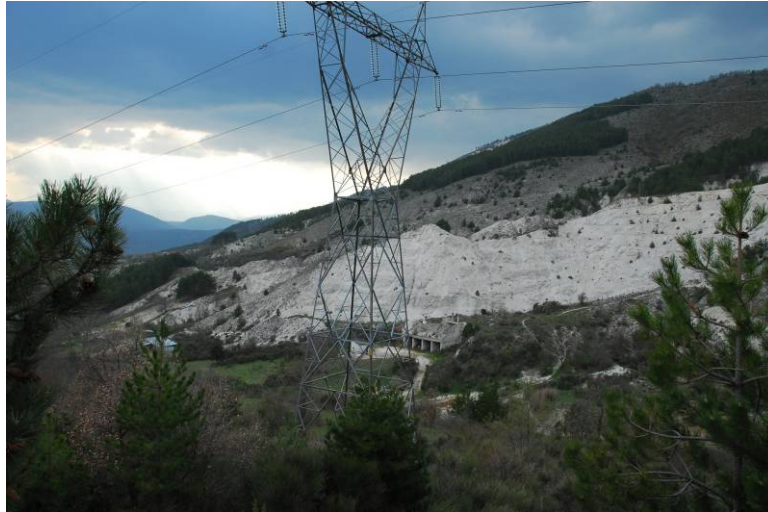
Figure 5.18. Quarry in Cataclasite with estimated 50^{\circ} slopes up to approximately 60 m high, located northeast of Colle (42.437N, 13.328E).
