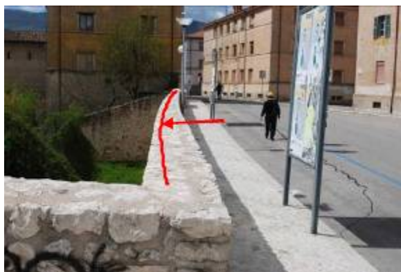
Figure 6.11. Stone masonry wall at L'Aquila city (42.348710°N, 13.403900°E). Note the (tolerable) outward movement at the center of the wall and the pavement cracks behind the wall.
