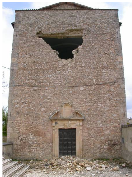
Fig. 4.28. S. Eusanio Forconese suffered partial collapse of the masonry church (D4).
