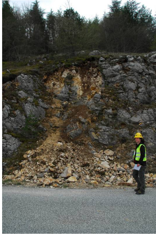
Figure 5.7. Shallow raveling-type failure of weathered limestone blocks (42.278N, 13.468E)
