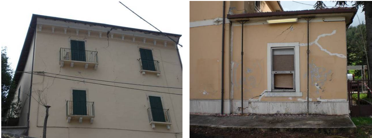
Fig. 4.45. Goriano Sicoli: (a) diagonal cracks in a masonry building (D3) and (b) at the railway station (D3).
