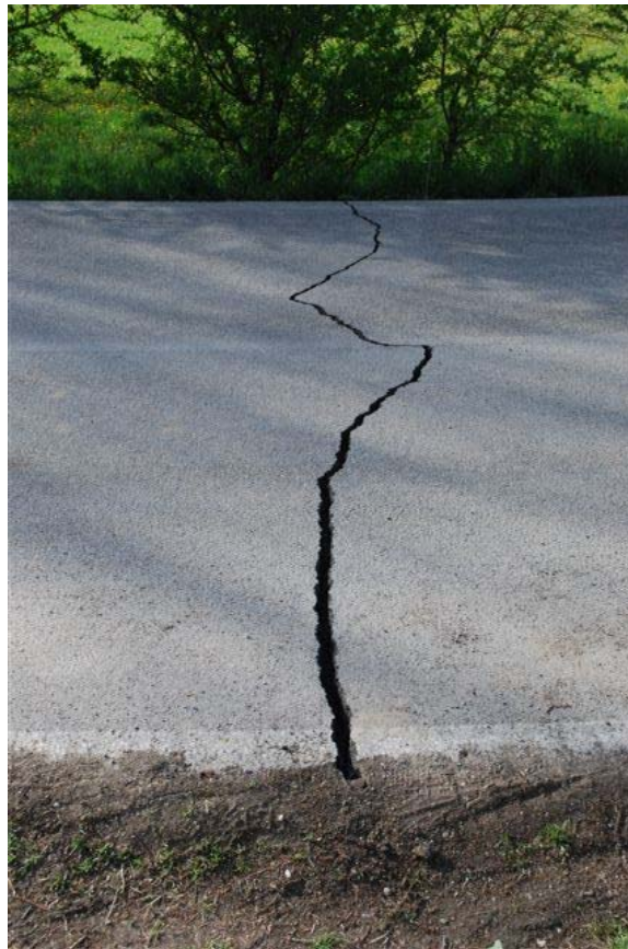
Figure 5.31. Typical tensile condition of road cracks such as depicted in Figure 5.15, not extending into neighboring sub-base or approach fill embankment (42.324N, 13.478E).
