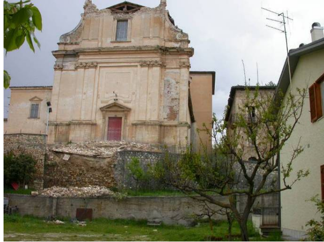
Fig. 4.40. San Demetrio ne' Vestini: (a) "Caserma dei Carabinieri" with cracks (not evident in the picture) and falls from the highest story, (b) partial collapse of the tympanum of the facade of the Madonna dei Raccomandati church.
