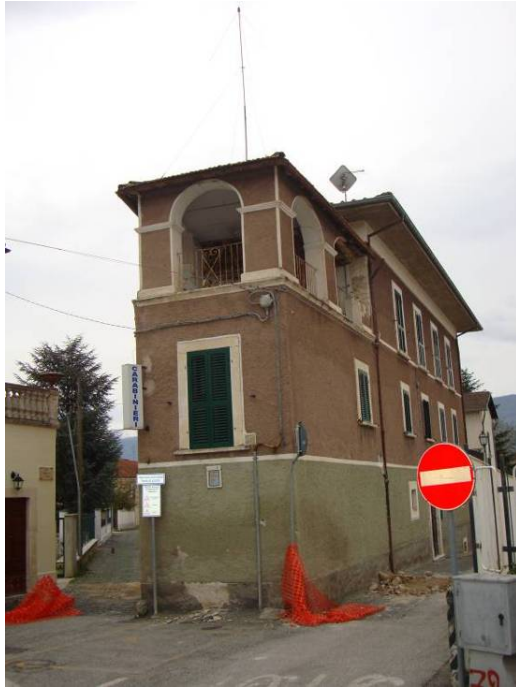
Fig. 4.40. San Demetrio ne' Vestini: (a) "Caserma dei Carabinieri" with cracks (not evident in the picture) and falls from the highest story, (b) partial collapse of the tympanum of the facade of the Madonna dei Raccomandati church.
