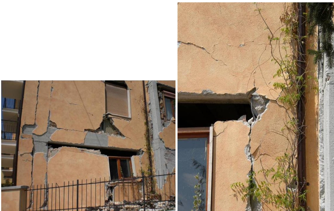
Fig. 4.22. San Gregorio eastern part: (a) RC building with structural damage; (b) detail of the damage to the beam-column connection.
