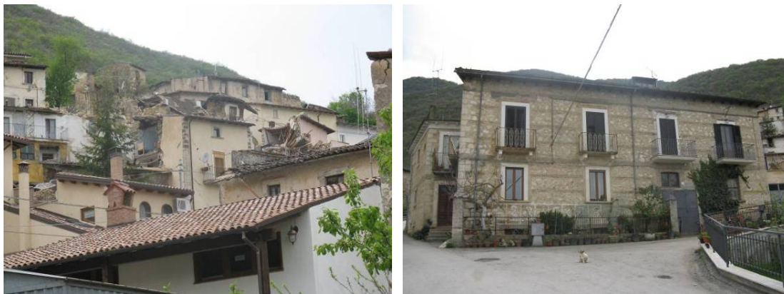
Fig. 4.37. Tussillo: (a) view of the historic center with some collapsed masonry buildings on the background; (b) masonry building at the entrance of the village showing no damage.
