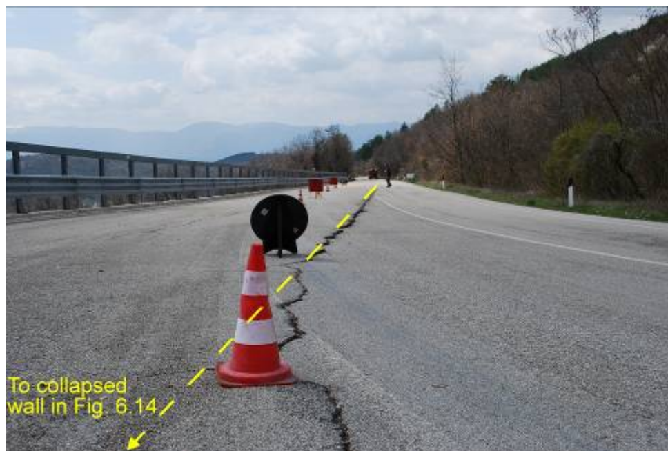
Figure 6.15. Pavement cracking in SS80 roadway (from L'Aquila to Campotosto) in the location of collapsed masonry retaining wall (42.420510°N, 13.358394°E).
