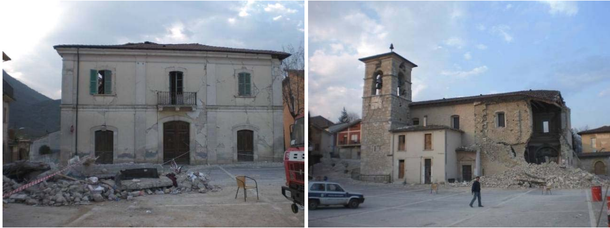
Fig. 4.36. Villa S. Angelo, historic center with (a) masonry building cracks; (b) partly collapsed church.
