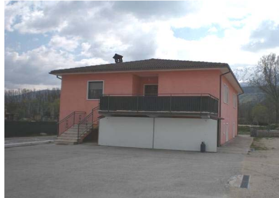
Figure 4.14 Onna: (a) D5 damage level on masonry building structures; (b) D0 damage on a RC building (except for the tilting of the chimney).
