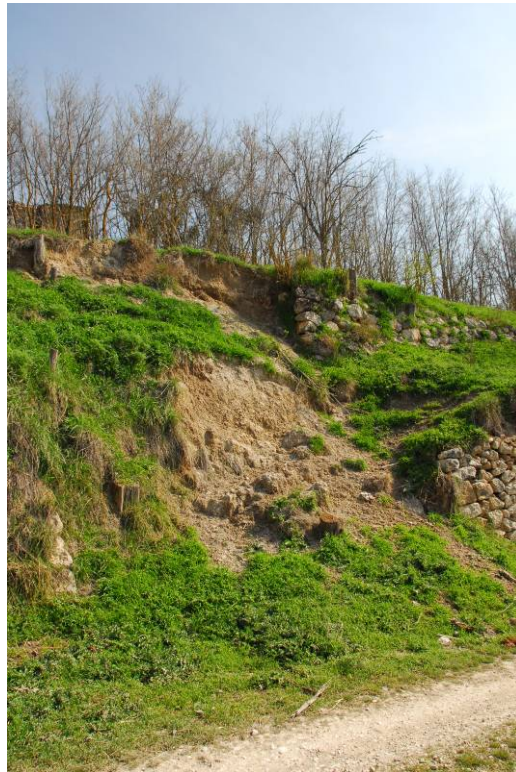
Figure 5.12. Shallow sloughing of regolith along road cut (southern flank of Castelnuovo N42.294, E13.628).
