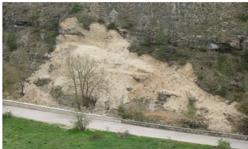
Figure 5.11. Raveling along the road from S. Demetrio to Lake Sinizzo (42.28845N,13.56442E)
