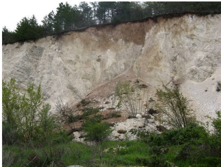
Fig. 5.19. Slide of a small wedge in cataclastic limestones on the SS80 at km 16.5 , uphill from Arischia (42.41973N, 13.34926E)
