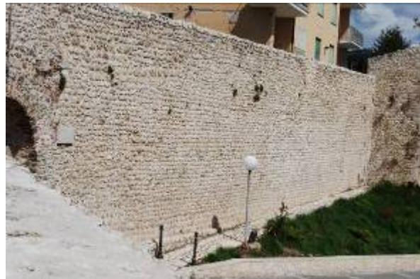
Figure 6.11. Stone masonry wall at L'Aquila city (42.348710°N, 13.403900°E). Note the (tolerable) outward movement at the center of the wall and the pavement cracks behind the wall.
