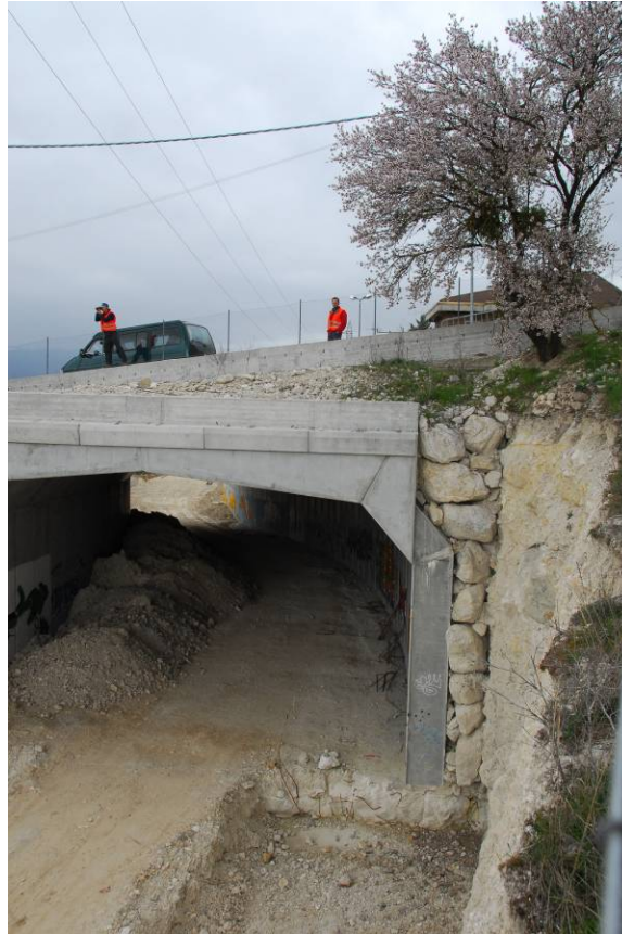
Figure 5.41. Boulder fill placed along side wall of cut-and-cover structure (42.358N 13.415E)
