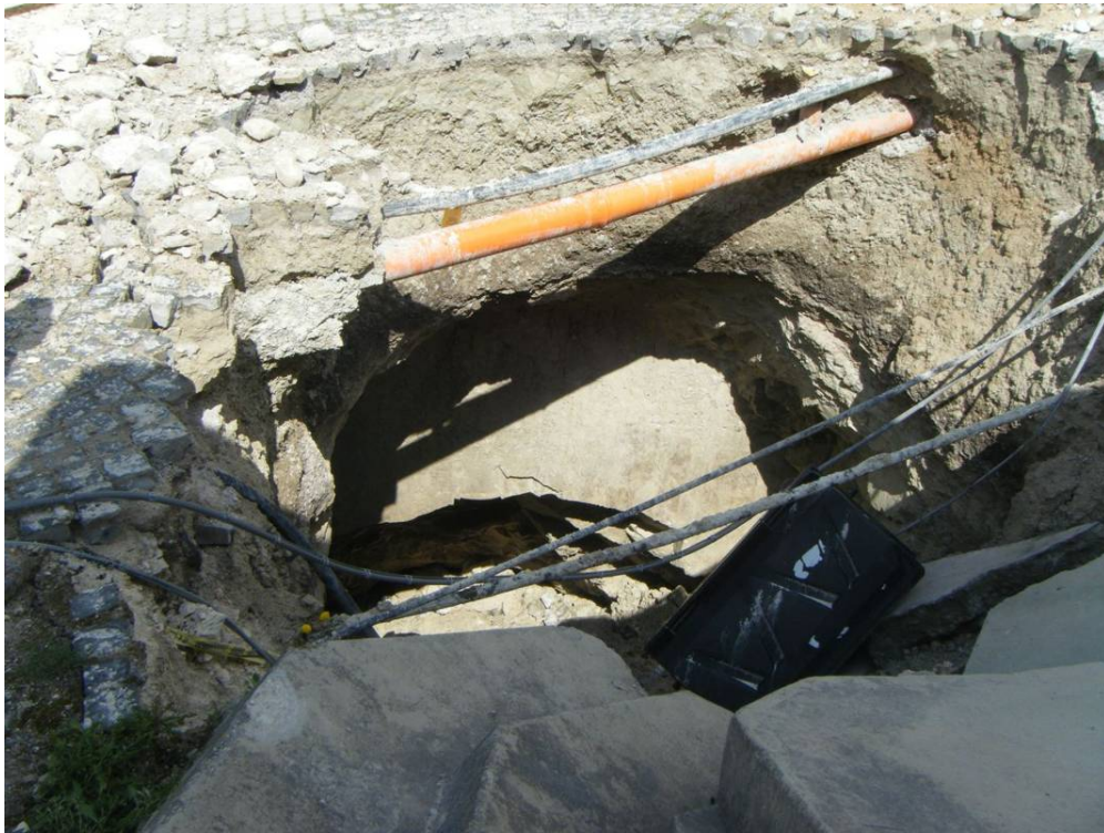
Figure 4.7. In the foreground of Figure 4.6 at the top of the hill in the center of Castelnuovo, a large sinkhole formed beneath the road exposing the weakly cemented Pleistocene sandstone that underlies the village. Water draining through the sinkhole was actively eroding a large void approximately 3-5 m in diameter and at least 6 m in depth. Cementation was strong enough to support small overhangs, at least temporarily (42.2947°, 13.629°).
