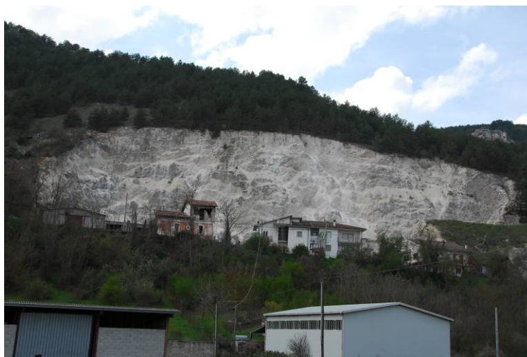
Figure 5.16. Quarry in Cataclasite with estimated 60^\circ slopes up to approximately 35 m high, located in Fossa (42.300N, 13.485E)
