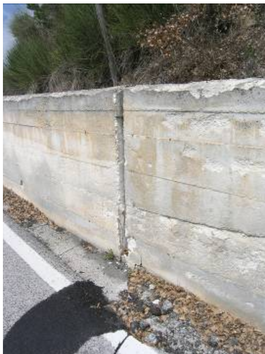
Figure 6.17. Ruptured retaining wall due to slope instability at SS80 highway between L'Aquila and Campotosto (42.418117°N, 13.351591°E).
