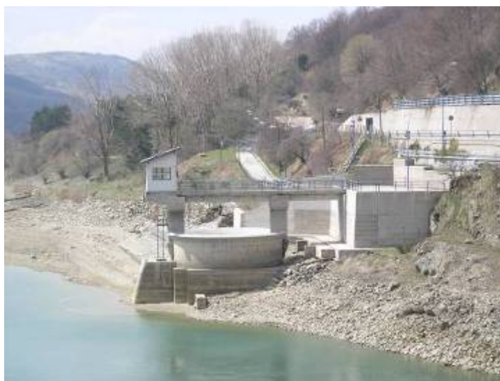
Figure 6.5. View of the outlet tower of Rio Fucino dam (42.535047°N, 13.410323°E).
