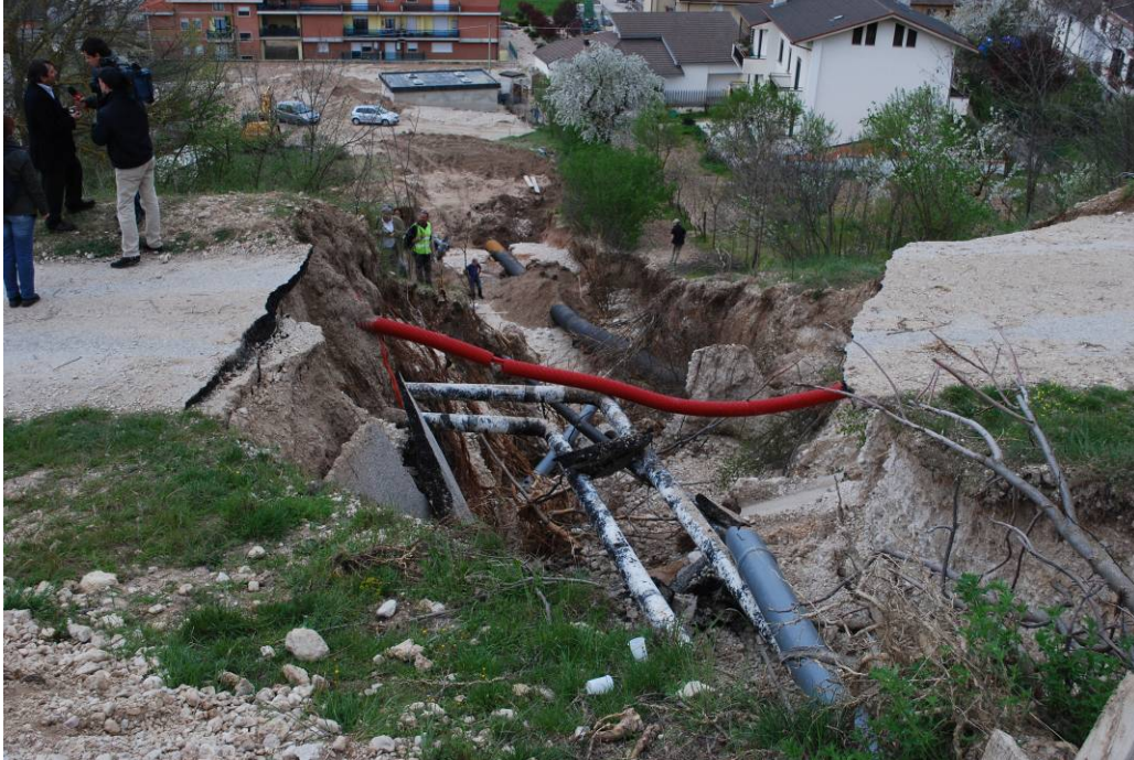
Figure 2.27. Paganica village: broken major water pipe (repaired) due to co-seismic rupture (Lat. 42,36537N Long. 13,46803E). Photo by Mylonakis G.
