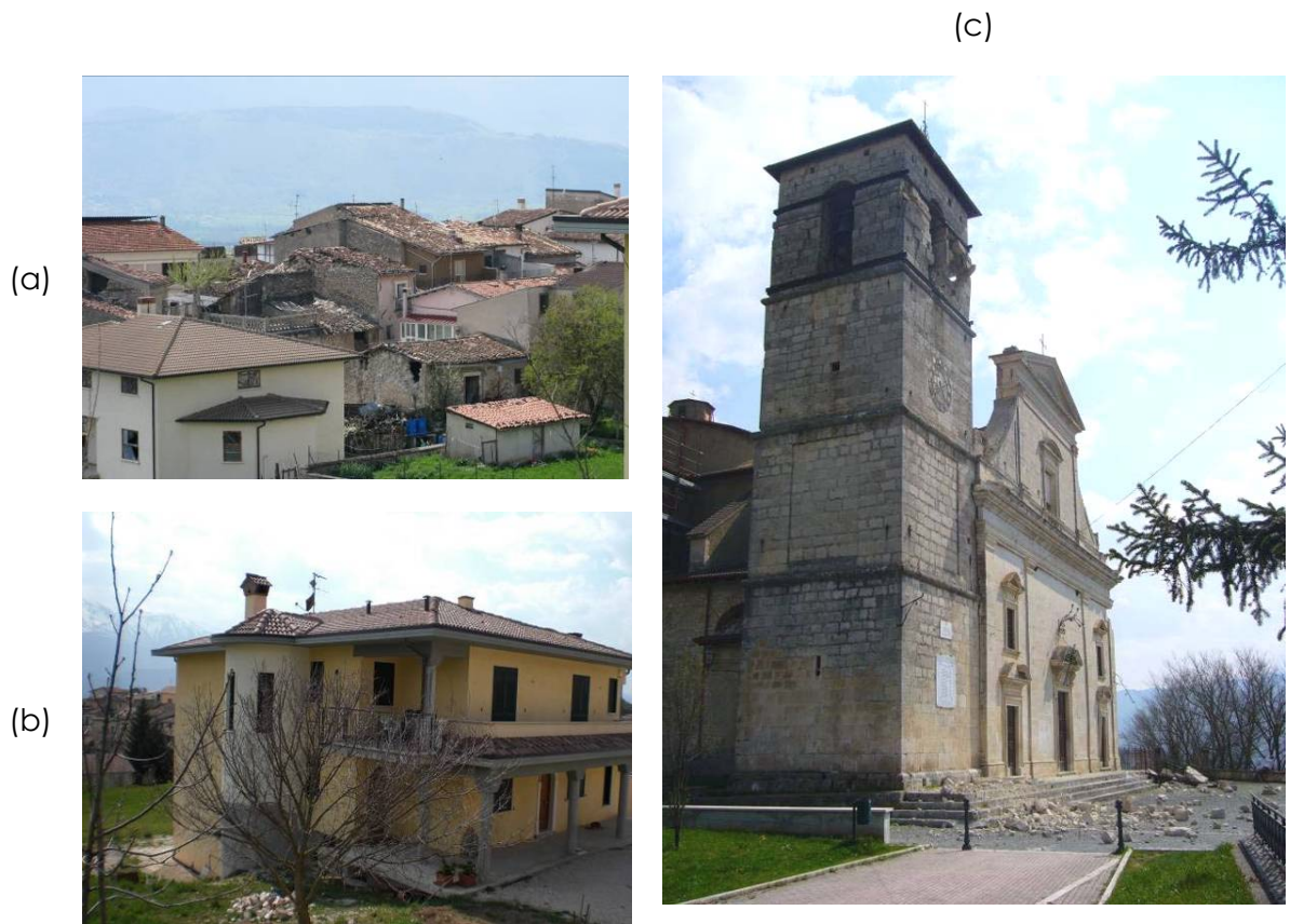
Fig. 4.33. Poggio Picenze: (a) variable damage (D3-D4) on masonry buildings of different style, (b) undamaged RC house (D0) close to the (c) monumental church (D3).
