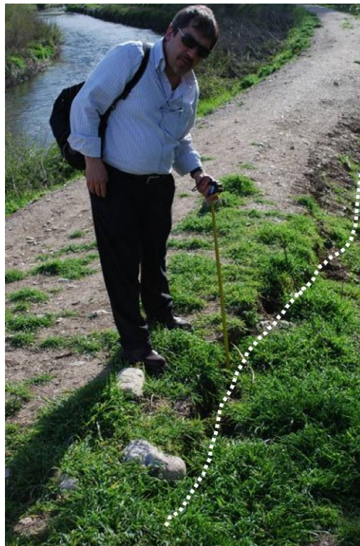
Figure 5.33. Ground cracks developed along levee crest adjacent to bridge abutment (42.324N, 13.478E).
