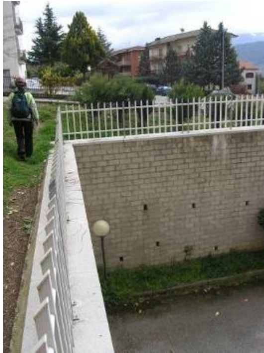
Figure 6.12. Undamaged wall at the severely shaken Pettino area (42.373050°N, 13.366106°E).
