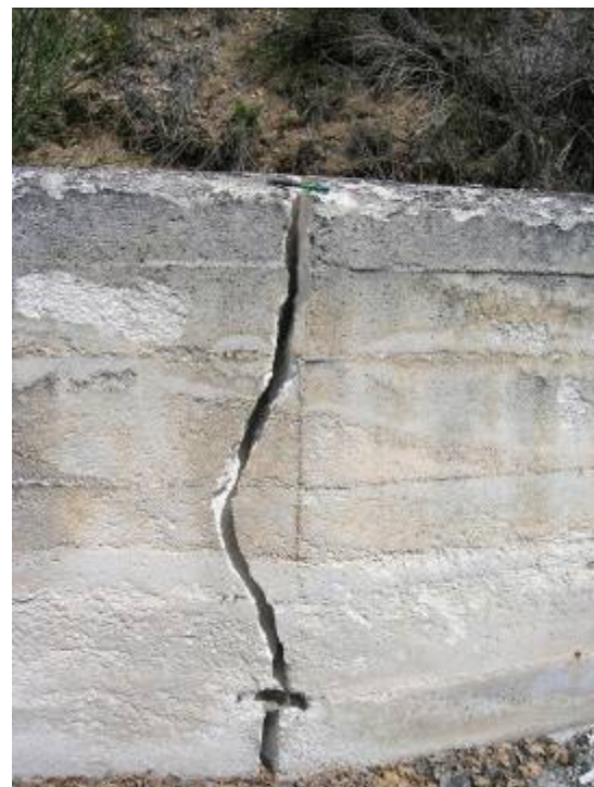
Figure 6.17. Ruptured retaining wall due to slope instability at SS80 highway between L'Aquila and Campotosto (42.418117°N, 13.351591°E).
