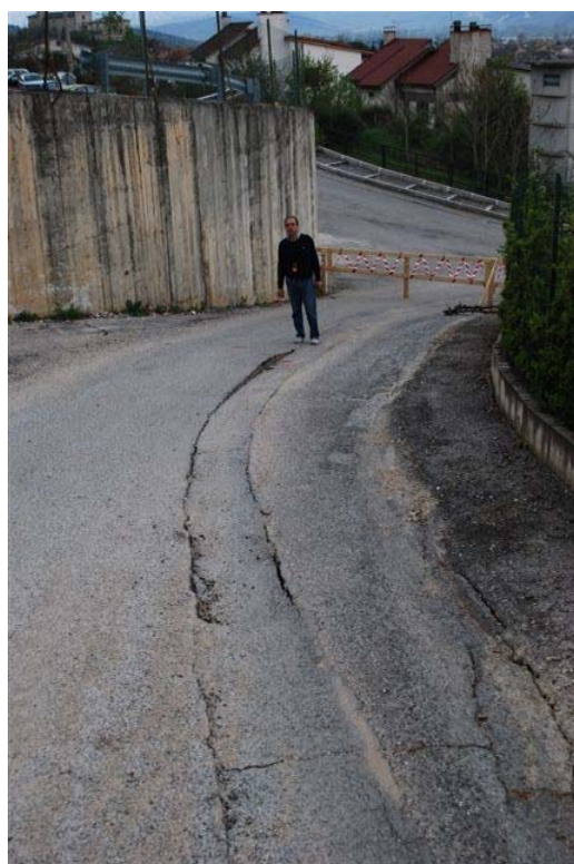
Figure 5.44. Seismic compression of trench backfill in the town of Paganica (42.365N, 13.465E).
