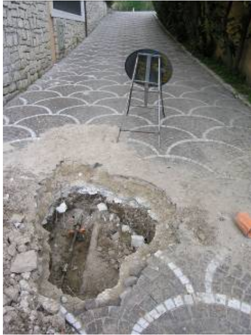
Figure 2.29. Failure of water pipe. (42.359335°N, 13.468954°E).
