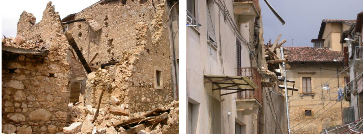
Fig. 4.27. S. Eusanio Forconese: (a) collapse of old masonry building (D5), and (b) partial collapse of masonry building (D4)
