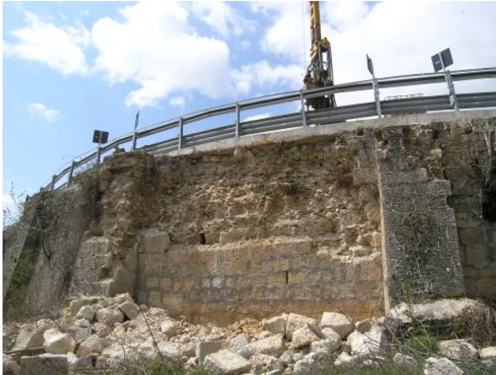
Figure 6.14. Partially collapsed wall at SS80 highway between L'Aquila and Campotosto (42.420510°N, 13.358394°E).
