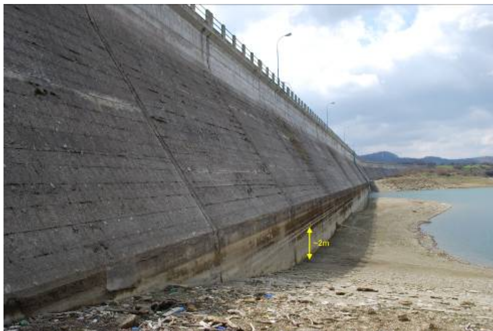
Figure 6.3. Upstream face of Sella Pedicate dam . The reduction in water level decided by ENEL following the main shock is evident in the photo (42.514954°N, 13.369194°E).
