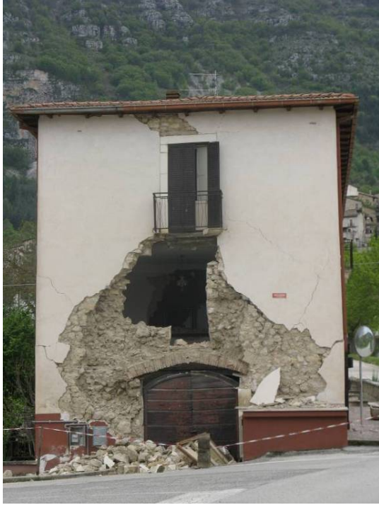
Fig. 4.29. Casentino: (a) partial collapse of the masonry building at the entrance of the village (b) collapse of old poor quality masonry buildings in the historic center.
