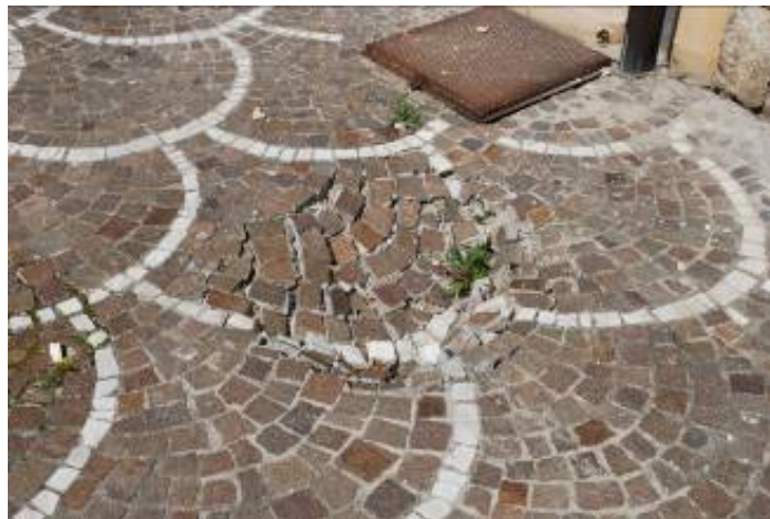
Figure 2.30. Local settlement close to piping system (42.359335°N, 13.468954°E).
