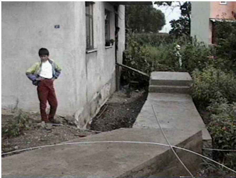
The concrete stair separated 1.5 m (58 in) from the house and moved 3.2 m (126 in) diagonally due to the fault surface rupture which went beneath the house. The house was only slightly damaged (south of Adapazari, N40°42.581', E30°21.495', 8/25/99, 15:40:56).
