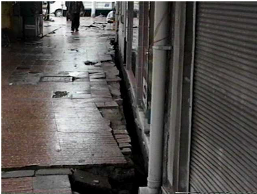
The building adjacent to the leaning building settled and shifted laterally, opening a gap between the sidewalk and the building (Adapazari) (N40°47.068', E30°23.976', 8/25/99, 12:36:00).
