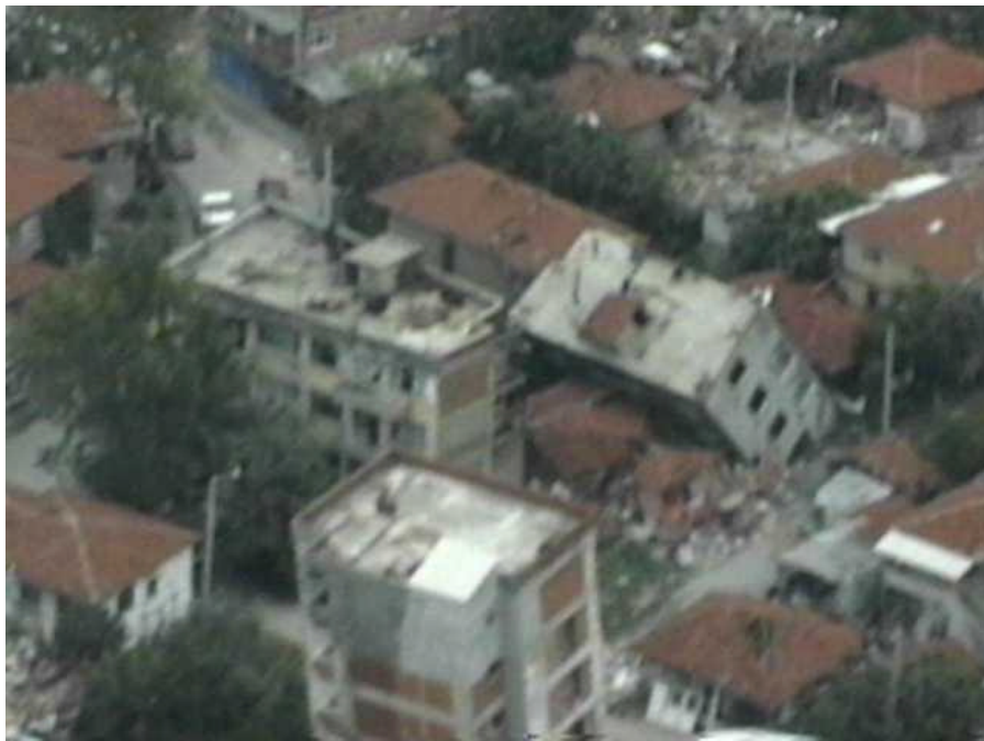
An apartment building leaned sideways against another building in Adapazari (N40°47.811', E30°22.625', 8/24/99, 15:54:29).
