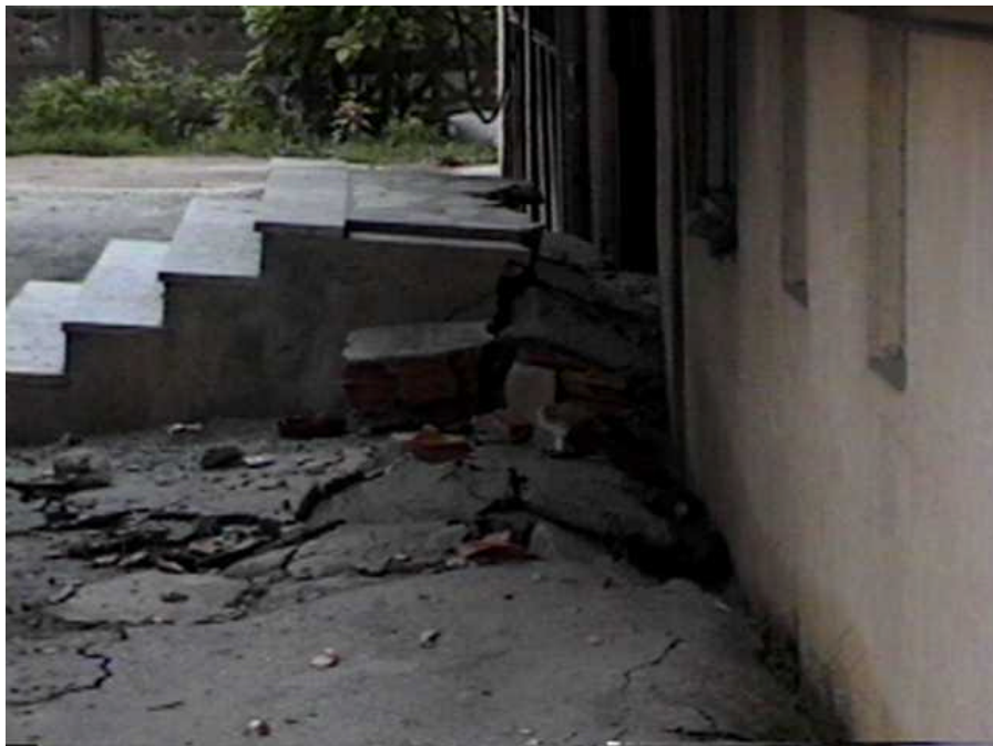
The building settled due to liquefaction, and the connection to the staircase was sheared (Adapazari, N40°46.561', E30°24.626', 8/27/99, 14:19:57).
