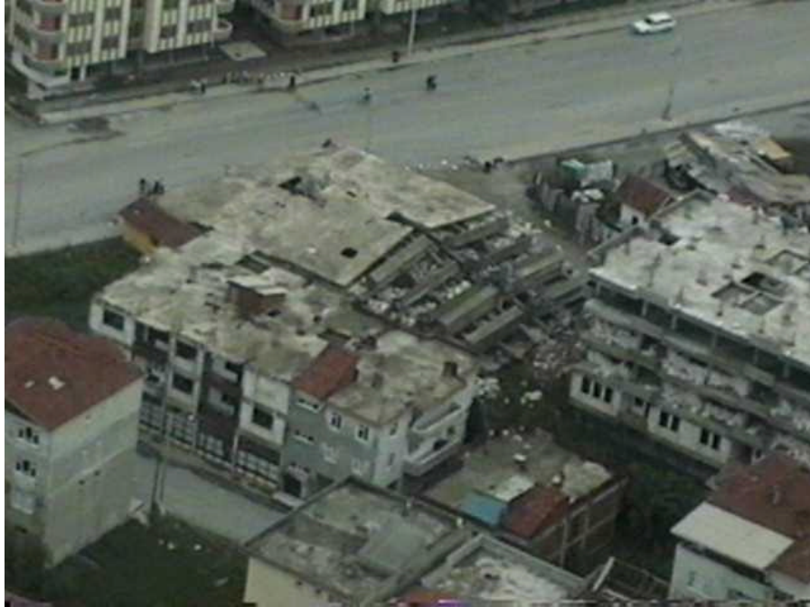
Lateral collapse of an apartment building in Adapazari. The rescue efforts were impeded by the collapsed concrete slabs that trapped many occupants (N40°46.329', E30°24.328', 8/24/99, 15:47:42).
