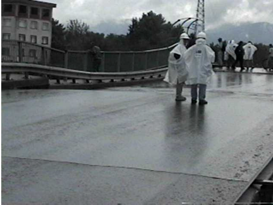
The road on top of the mechanically stabilized earth abutment sagged, possibly due to the failure of the reinforced concrete box culvert passing under it (South of Adapazari, N40^{\circ}42.581' , E30^{\circ}21.495' , 8/25/99, 15:40:56).
