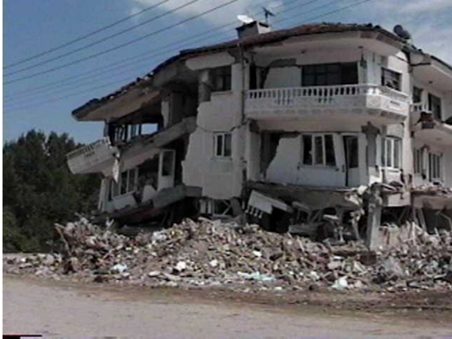
The first floors of this apartment building in Yalova collapsed ( N40^{\circ}39.08' , E29^{\circ}15.712' , 8/26/99, 13:11:25).
