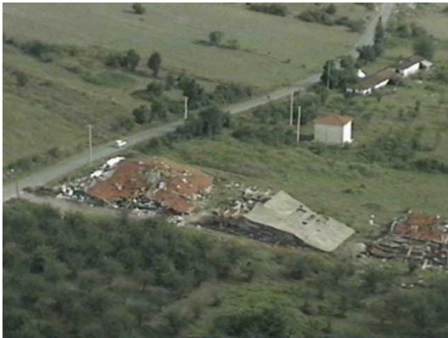
Three apartment buildings collapsed in the Arifye area (N40°42.829', E29°23.768', 8/24/99, 16:59:06).
