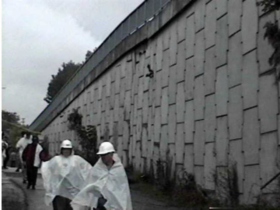
The overall performance of the mechanically stabilized earth abutment of the bridge was remarkable (South of Adapazari, N40°42.581', E30°21.495', 8/25/99, 15:40:56).
