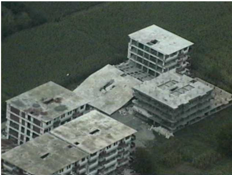
One of these apartment buildings collapsed laterally while the others withstood the earthquake forces (Arifiye area, N40°46.329', E30°24.328', 8/24/99, 15:47:42).
