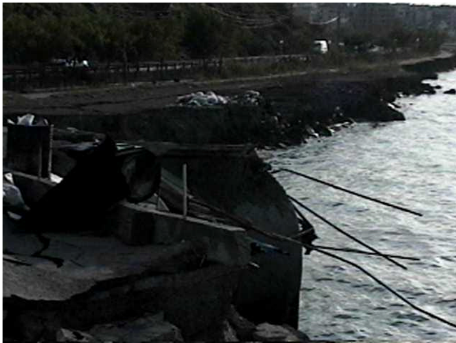
To the west of Golcuk, a piece of land slid into the sea. There were ground cracks parallel to the new shoreline (N40°43.074', E29°46.083', 8/28/99, 16:20:48).
