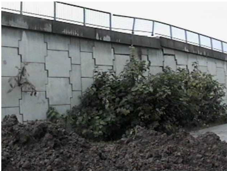
At the location where the road sagged, one side of the mechanically stabilized earth abutment displayed relative motion between face plates (South of Adapazari, N40^{\circ}42.581' , E30^{\circ}21.495' , 8/25/99, 15:40:56).
