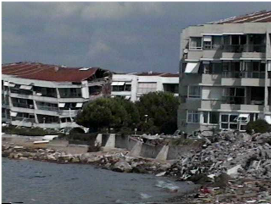
Along the shoreline in Yalova, many apartment buildings collapsed. The retaining wall in front of the apartment building on the right settled and shifted laterally due to the liquefaction of its foundation. However, there were no sign of lateral spread which could have damaged the building. ( N40^{\circ}40.913' , E29^{\circ}21.234' , 8/26/99, 14:42:20).
