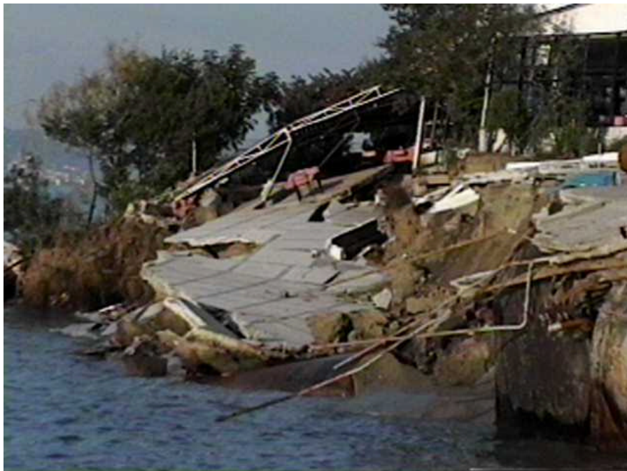
To the west of Golcuk, the waterfront slid into the sea. The slide must have occurred gently as the red table and chair were still standing on the inclined concrete floor (N40°43.074', E29°46.083', 8/28/99, 16:20:48).
