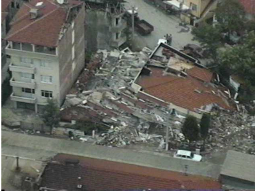
Lateral collapse of an apartment building next to an intact building in Adapazari (N40°47.811', E30°22.625', 8/24/99, 15:54:29).
