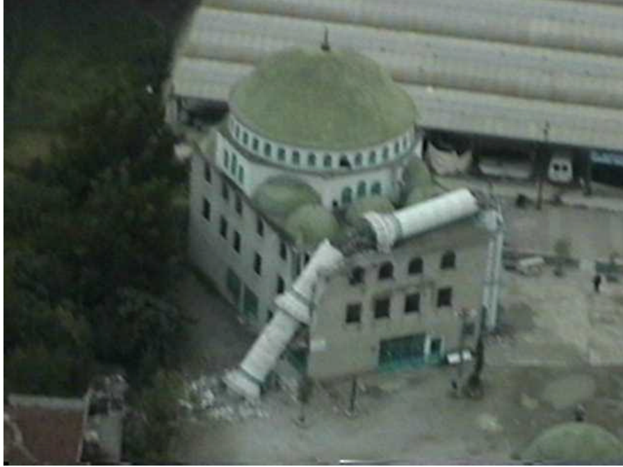
The minaret of the mosque tipped over and broke in the Arifye area ( N40^{\circ}42.41' , E30^{\circ}22.808' , 8/24/99, 16:26:18).
