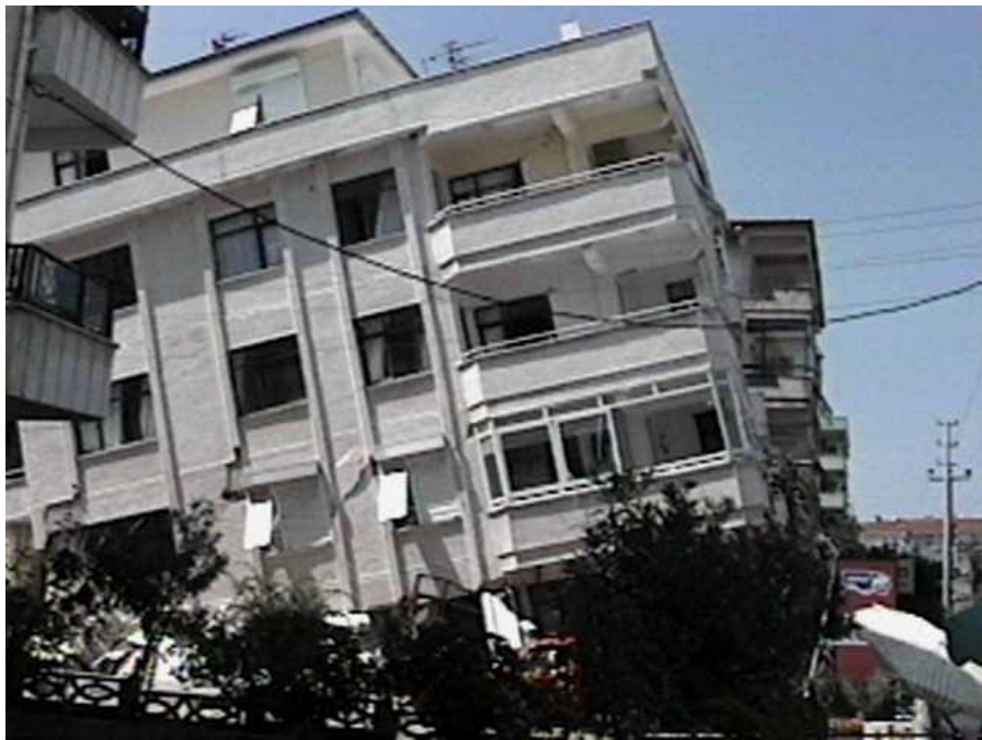
The bottom floors of this apartment building in Yalova failed (N40°38.845', E29°7.448', 8/26/99, 12:01:06).
