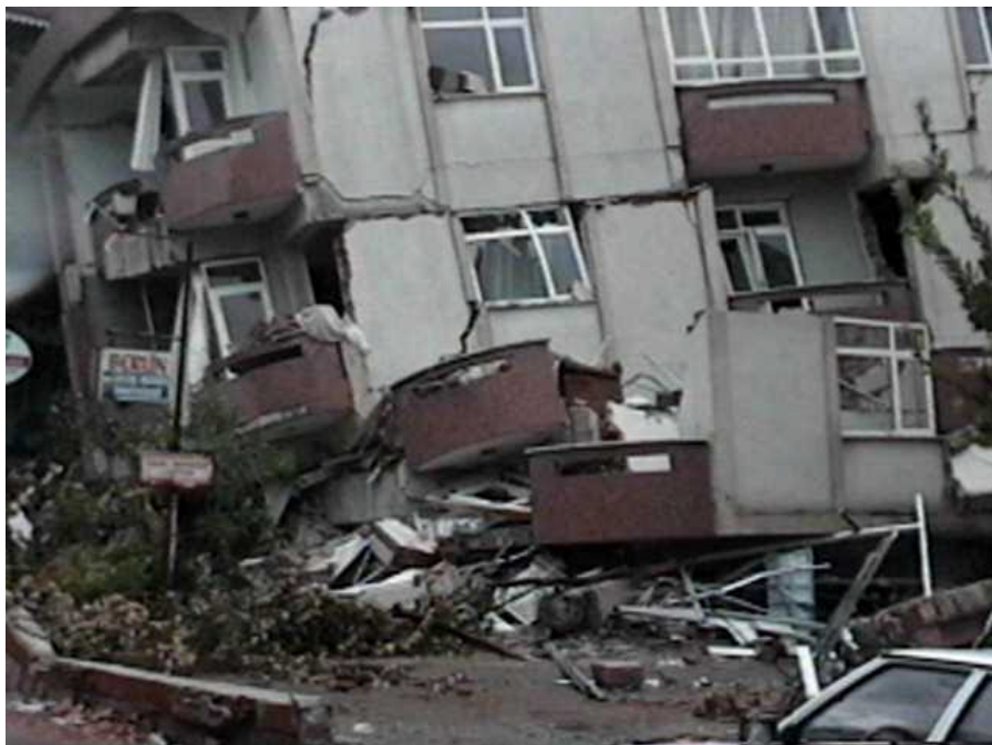
The collapse of the lower floors of an apartment building in Adapazari crushed a car (N40°46.716', E30°23.821', 8/25/99, 12:15:17).
