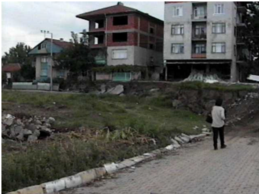
In Golcuk, the ground rupture passed in front of three houses without apparently damaging them ( N40^{\circ}43.245' , E29^{\circ}50.477' , 8/28/99, 16:01:42).
