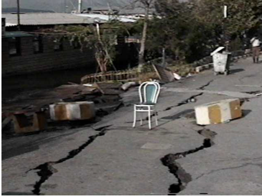
In Halidere, part of the waterfront subsided into the sea and the rest spread laterally (N40°43.064', E29°45.019', 8/26/99, 18:01:02).
