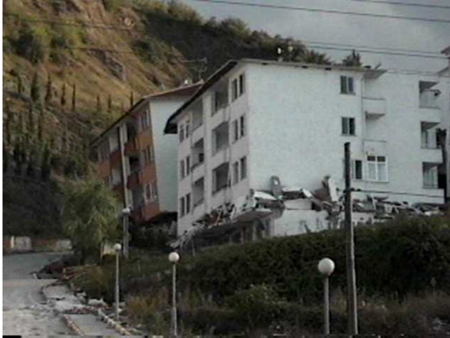
To the west of Golcuk, the second floor of two apartment buildings collapsed and their upper floors moved laterally (N40°43.315', E29°46.832', 8/28/99, 17:53:39).
