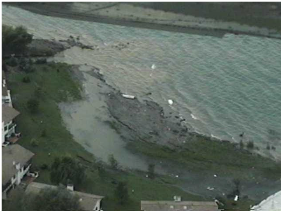
Lateral spread on the southern shore of Lake Sapanca (N40°41.448', E30°16.733', 8/24/99, 16:31:54).
