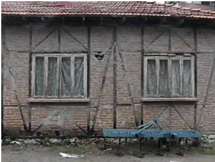
Some old wood structures with masonry brick infills performed remarkably well during the earthquake, whereas nearby more modern reinforced concrete buildings collapsed (Adapazari, N40°47.027', E30°24.085', 8/25/99, 13:18:20).
