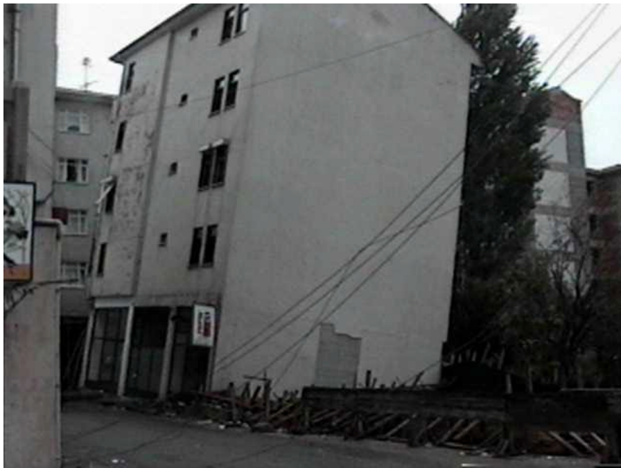
Another view of the building which underwent foundation failure (Adapazari) (N40°46.862', E30°24.133', 8/25/99, 13:47:00).
