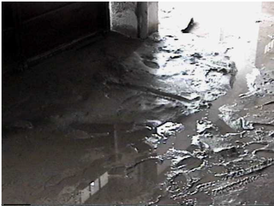
In the garage at the first floor of an apartment building, silty sand had littered the concrete slab. Water was reported to have flooded the garage after the earthquake (N40°46.651', E30°24.598', 8/27/99, 13:09:48).
