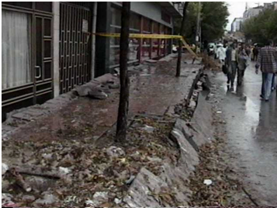
The buildings settled. The sidewalk heaved and lifted up part of the asphalt pavement (Adapazari, N40°46.742', E30°24.185', 8/25/99, 14:12:59).
