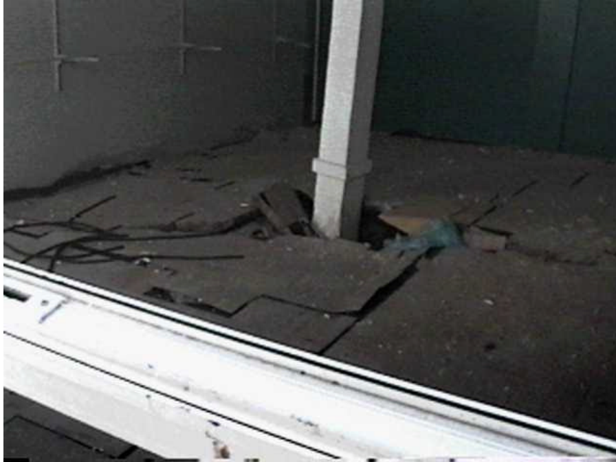
The column punched through the floor of the building which settled (Adapazari, N40°46.614', E30°24.287', 8/27/99, 13:02:07).
