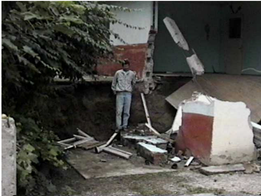
In Golcuk, the ground rupture passed beneath the corner of a house, and the corner of the house detached from the house (N40°43.178', E29°50.555', 8/28/99, 15:45:11).
