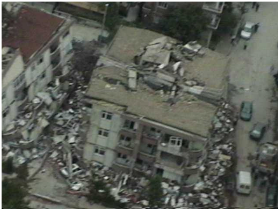
Many apartment buildings underwent failure of the lower floors (Adapazari, N40°46.329', E30°24.328', 8/24/99, 15:47:42).
