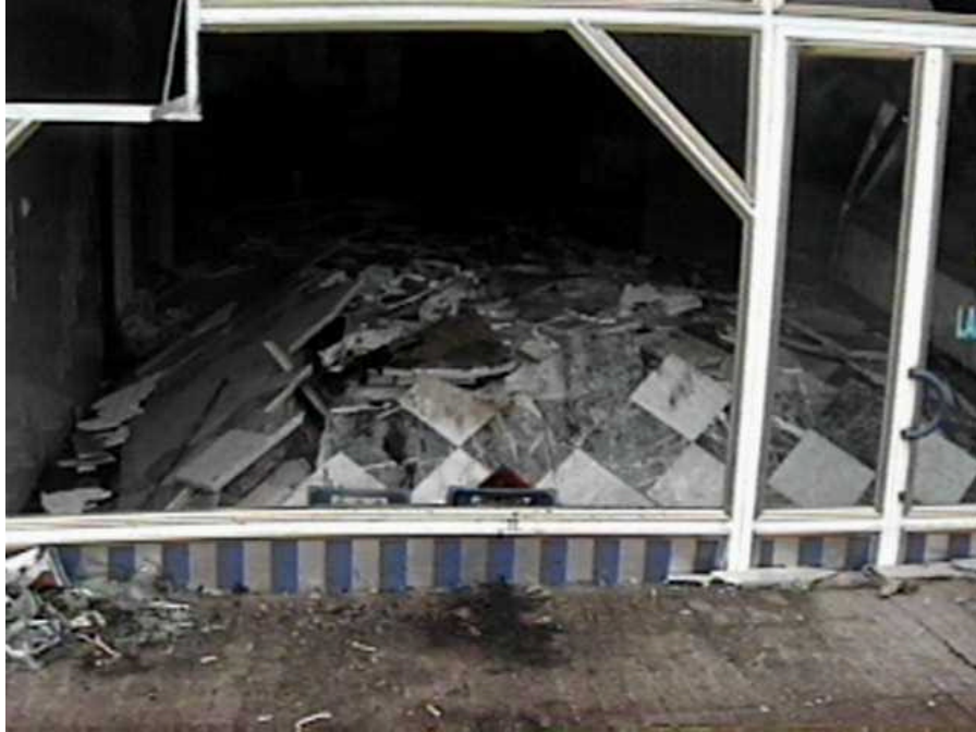
The marble tile floor of the shop bulged as the building settled into the ground (Adapazari, N40°46.662', E30°24.163', 8/25/99, 14:17:45).
