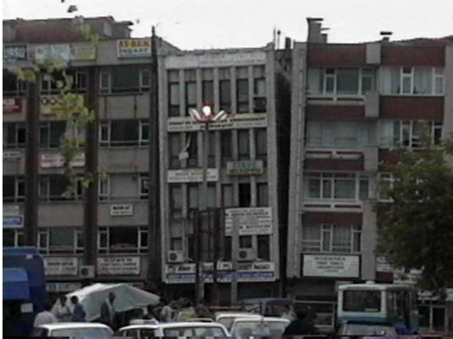
The office building in the center leaned sideways due to differential settlement (N40°46.719', E30°24.215', 8/27/99, 17:07:46).
