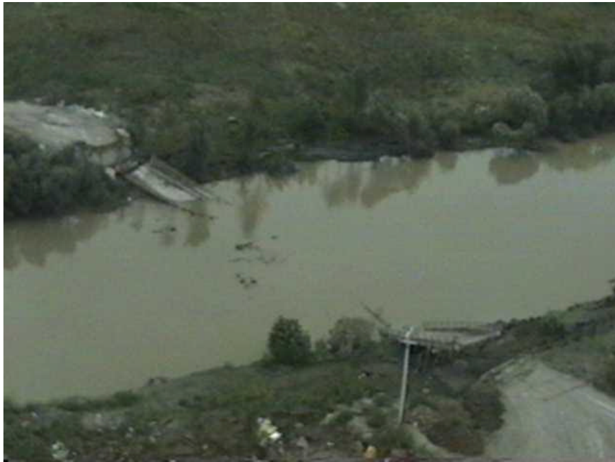
Collapse of the bridge on the Sakarya river in the Arifiye area (N40°42.41', E30°22.808', 8/24/99, 16:26:18).
