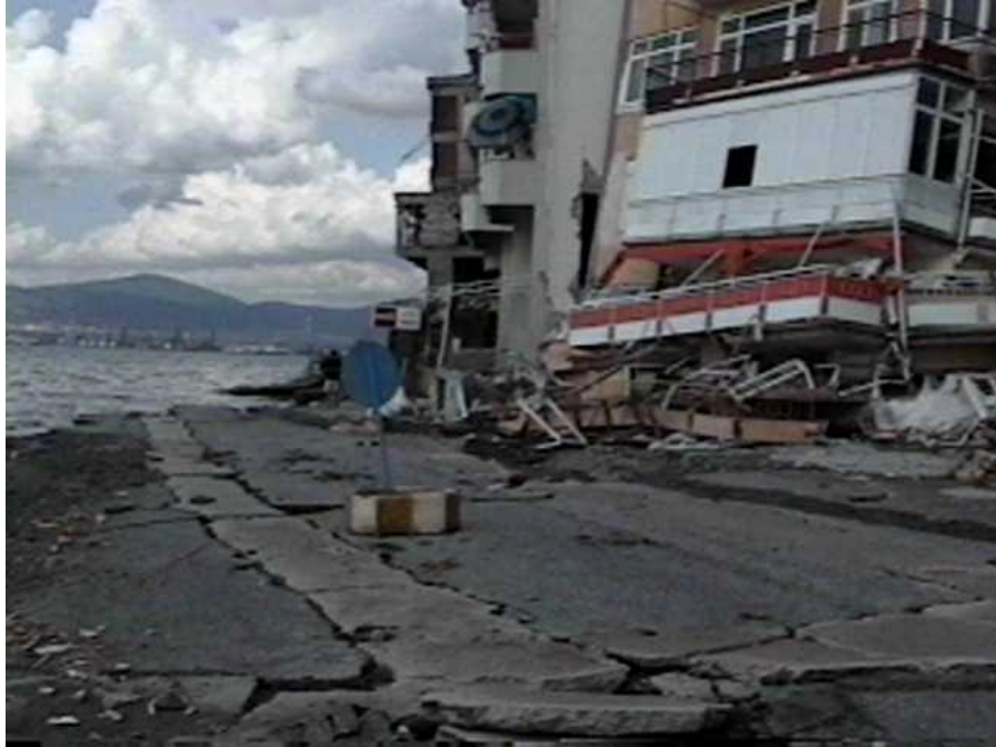
In Halidere, an apartment building collapsed., and the waterfront spread laterally toward the Marmara Sea (N40°42.961', E29°44.805', 8/26/99, 17:33:58).
