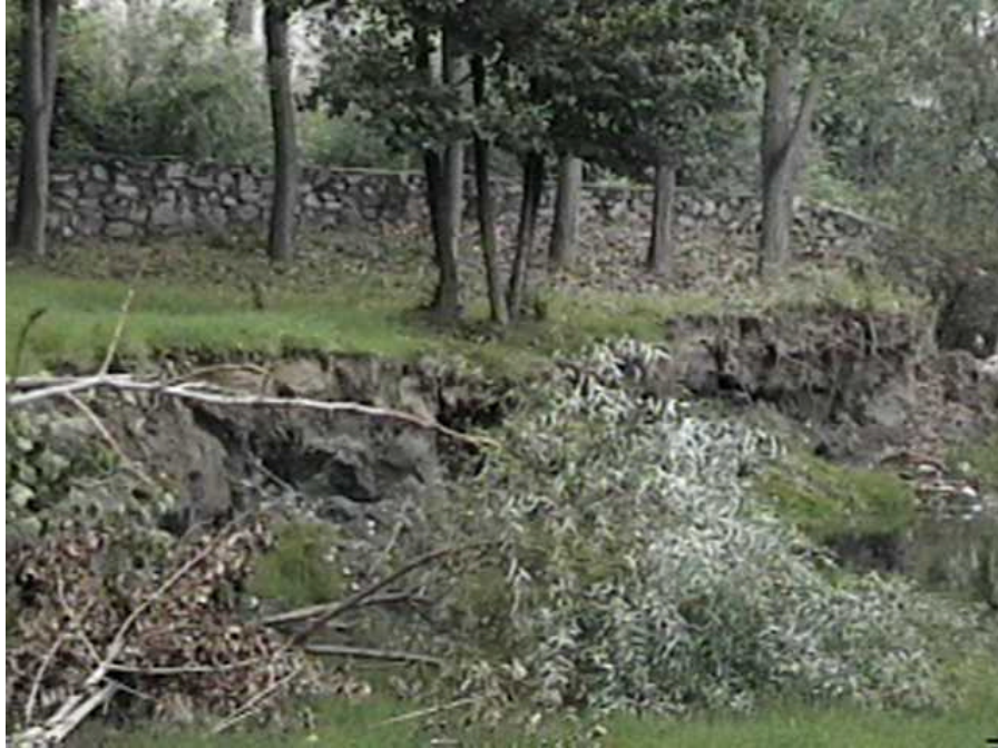
In Golcuk, the ground rupture passed close to a wall, intersected it, and sheared it. Most of the wall remained intact ( N40^{\circ}43.245' , E29^{\circ}50.477' , 8/28/99, 16:01:42).
