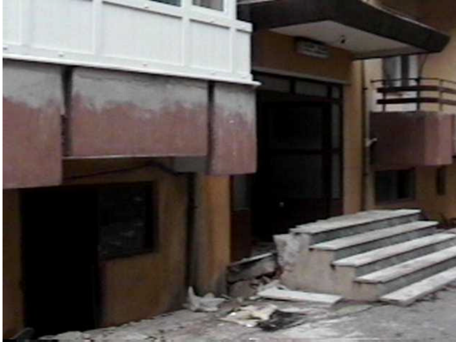
The staircase of the building was sheared as the building settled due to liquefaction (Adapazari, N40°46.561', E30°24.626', 8/27/99, 14:19:57).
