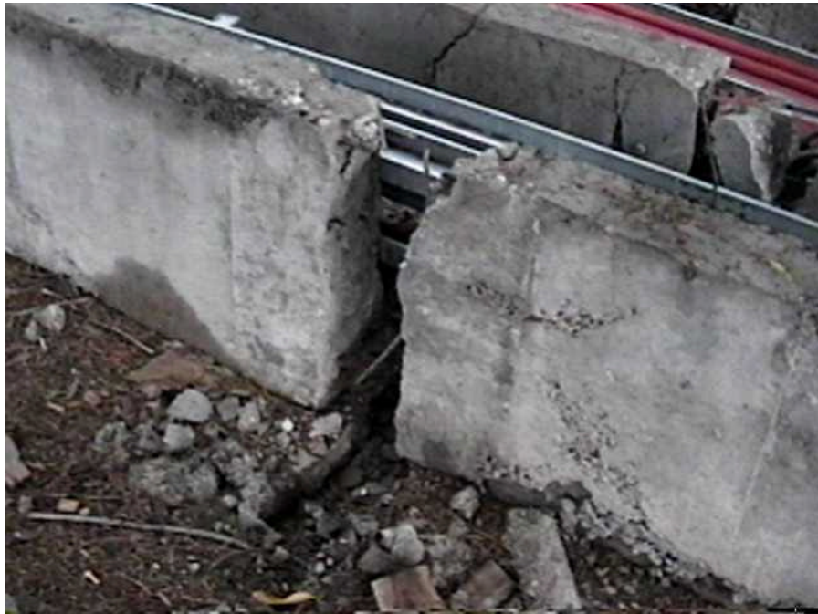
In the Ford plant in Golcuk, the U-shaped utilities corridor was subjected to tension and failed due to ground displacement (N40°42.818', E29°51.098', 8/28/99, 13:49:32).
