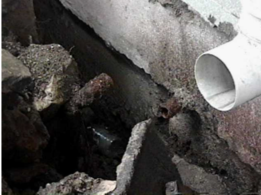
The buried metal pipe broke down at the interface between soil and building due to the building settlement and lateral movement (Adapazari, N40°47.038', E30°24.033', 8/25/99, 12:51:04).
