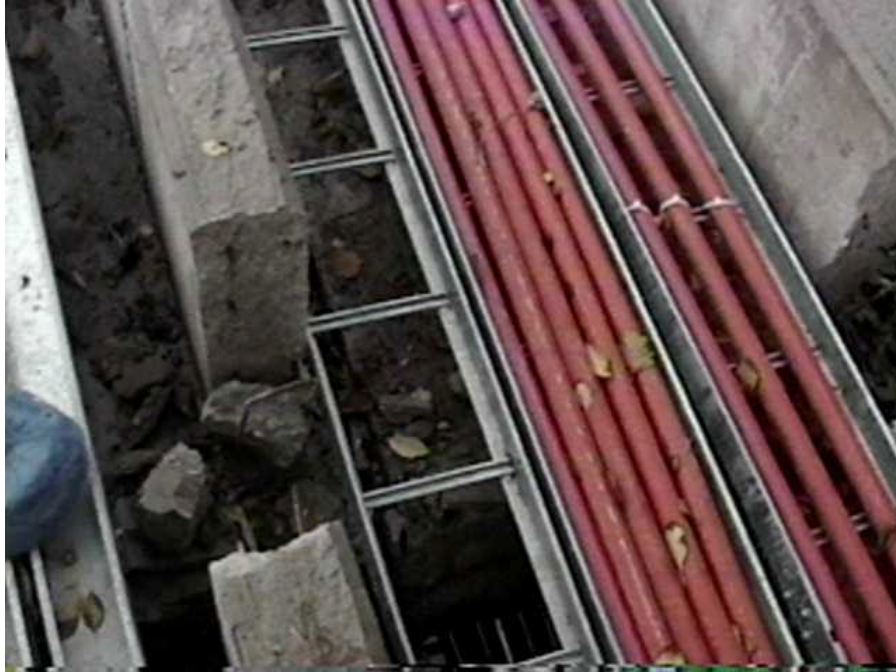
In the Ford plant of Golcuk, the utility corridor was broken and separated due to tensile strain (N40°42.818', E29°51.098', 8/28/99, 13:49:32).
