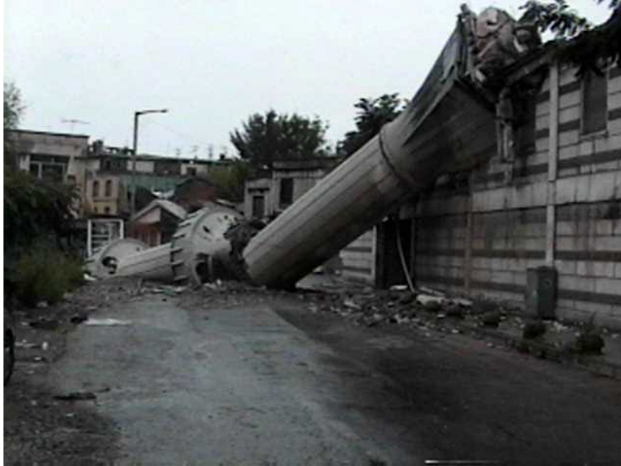
The minaret of the mosque tipped over and broke (Adapazari, N40^{\circ}46.822' , E30^{\circ}24.128' , 8/25/99, 13:53:21).
