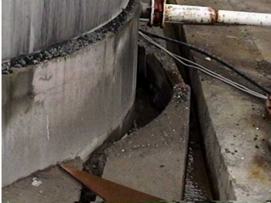
In a glue factory to the east of Golcuk, there was relative displacement and cracking between the foundation of the tank and the concrete slabs (N40°42.755', E29°53.139', 8/28/99, 12:07:23).
