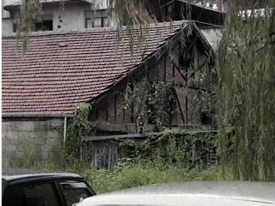
The unreinforced building with wood-frame and masonry infill performed well during the earthquake. (Adapazari, N40°46.822', E30°24.128', 8/25/99, 13:53:21).
