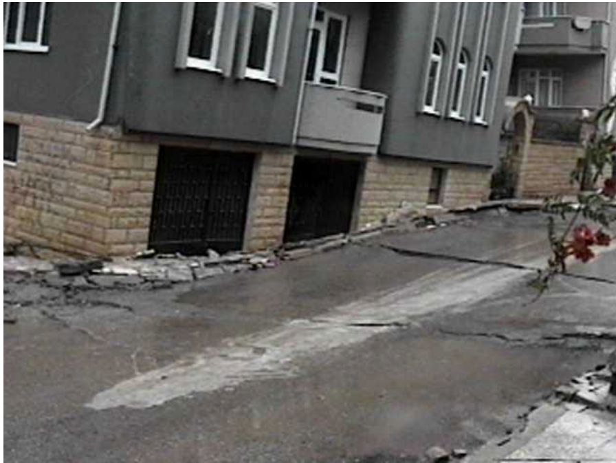
An apartment building in downtown Adapazari that has tilted due to differential settlement (N40°46.485', E30°23.807', 8/25/99, 11:53:51).
