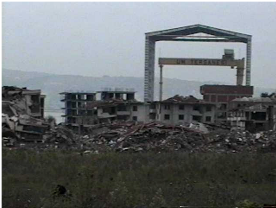
In Golcuk, the crane and steel frame of a construction site were standing apparently undamaged while many reinforced concrete buildings in the foreground had been destroyed by the earthquake (N40°42.385', E29°52.456', 8/28/99, 12:20:10).
