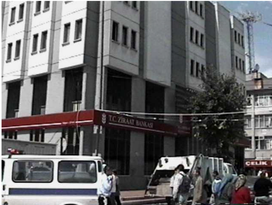
The Ziraat bank building in Adapazari is one of the few buildings founded on piles. There were no apparent signs of damage to this building (N40°46.6', E30°24.062', 8/27/99, 12:37:58).
