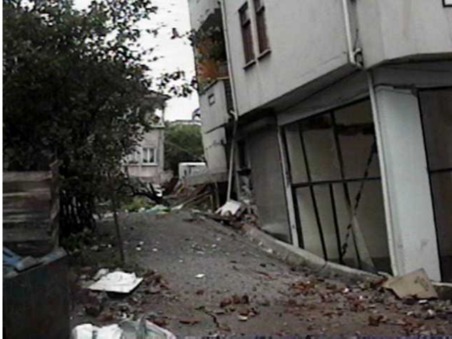
The foundation of the building failed and the building tilted in the east/west direction (Adapazari) (N40°46.862', E30°24.133', 8/25/99, 13:47:00).
