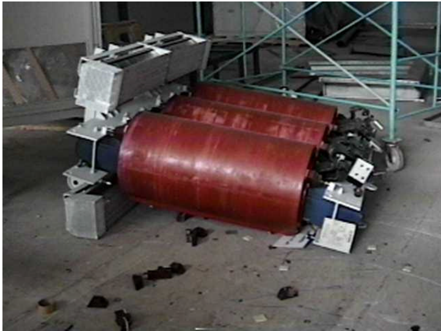
Located 80 m above the ground in the painting building of the Ford plant of Golcuk, the 5-ton transformer jumped out of its housing, and scraped the floor due to earthquake acceleration (N40°43.165', E29°50.596', 8/28/99, 15:42:14).
