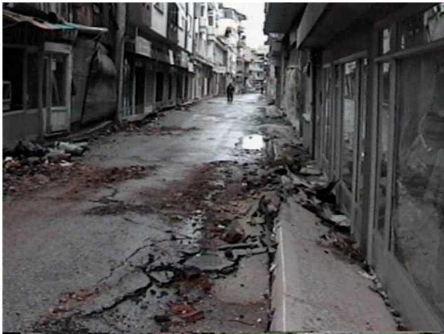
All the buildings in this street in Adapazari settled at least one foot (N40°46.779', E30°24.266', 8/25/99, 14:04:14).
