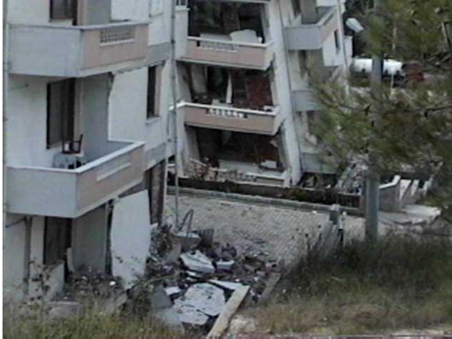
The first floors of the apartment buildings on the hillside east of Yalova were damaged or collapsed. There was no evidence of slope stability problems or ground failure (N40°41.274', E29°35.257', 8/26/99, 16:23:52).
