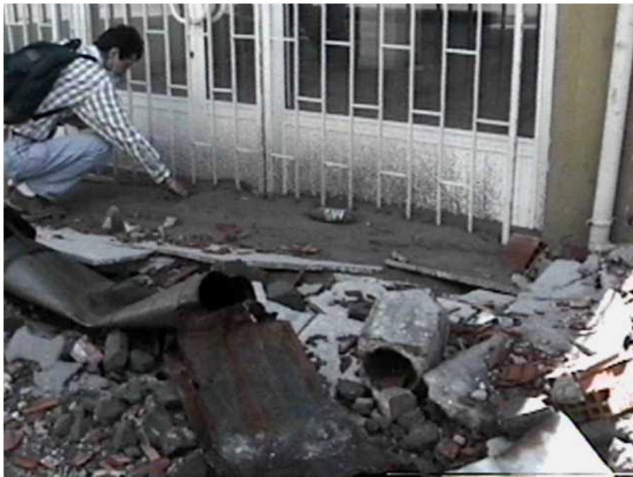
A deposit of ejected sand was observed in front of this building which settled into the ground. This was not systematically observed for all settled buildings (Adapazari, N40°46.612', E30°24.257', 8/27/99, 12:54:13).
