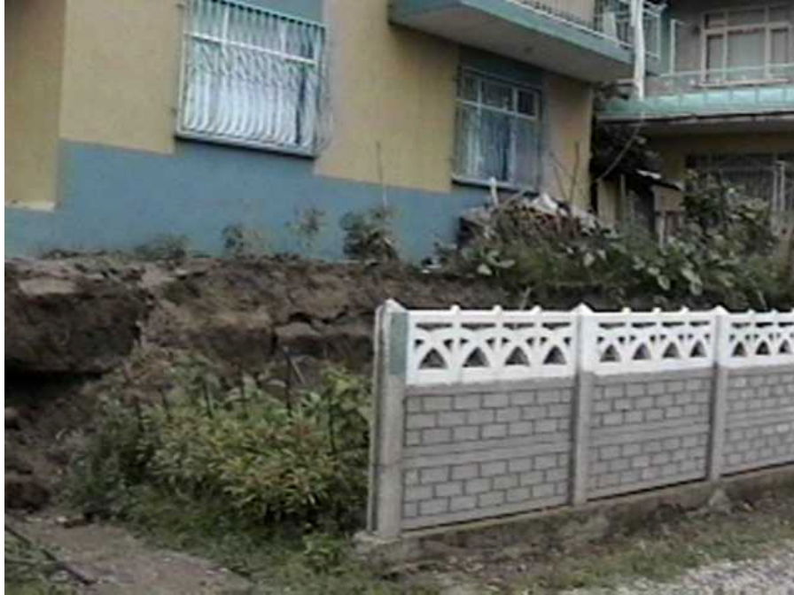
In Golcuk, the ground rupture passed very close to the house, causing almost no visible damage to the house. Some plants were still hanging to the soil close to the house (N40°43.178', E29°50.555', 8/28/99, 15:45:11).
