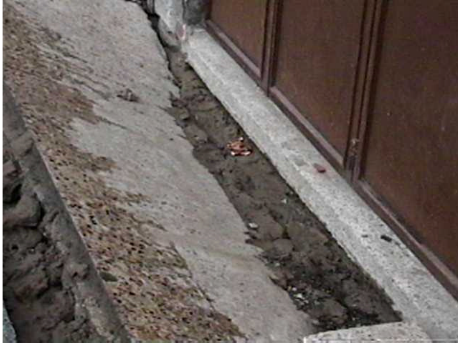
At the entrance of the garage door of an apartment building that has settled close to 1 foot, there were traces of silty soil which had been ejected during the earthquake. The sidewalk has caved in towards the building (N40°46.689', E30°23.762', 8/25/99, 12:01:29).
