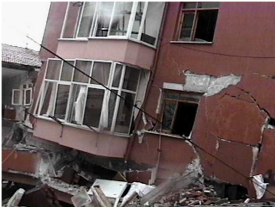
The bottom floors of the reinforced concrete building collapsed in Adapazari (N40°55.202', E29°21.011', 8/25/99, 11:38:40, poor GPS coverage).
