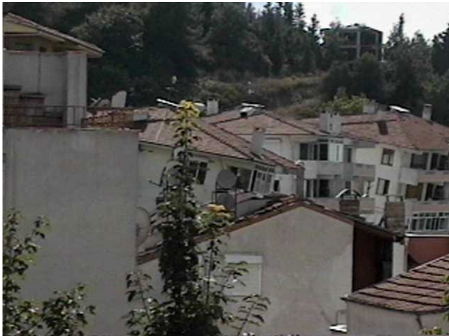
Some of the apartment buildings on the hillside east of Yalova leaned toward the sea due to the failure of their first floor (N40°41.274', E29°35.257', 8/26/99, 16:23:52).
