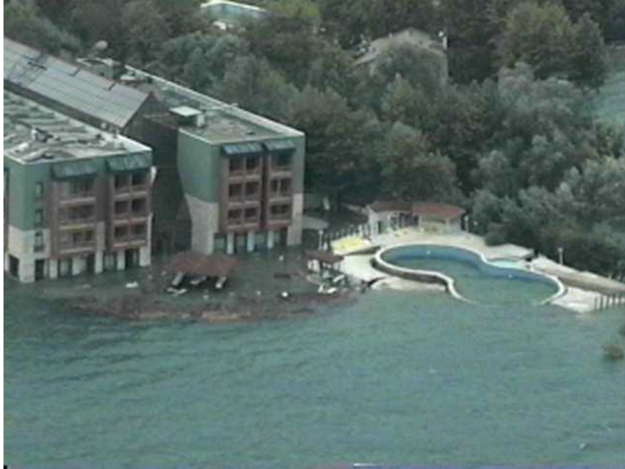
Subsidence of hotel Sapanca on the shore of the Sapanca lake (N40°41.448', E30°16.733', 8/24/99, 16:31:54).
