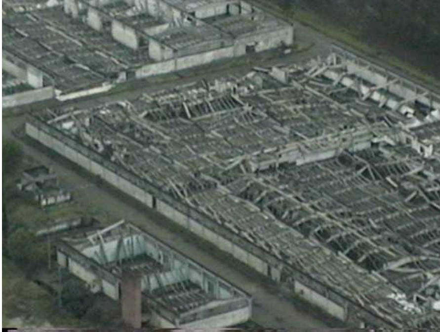
The roof of this warehouse in the Izmit area caved in due to the earthquake shaking. The Izmit bay area is the heart of Turkey's industry (N40°45.406', E29°58.063', 8/24/99, 15:31:05).
