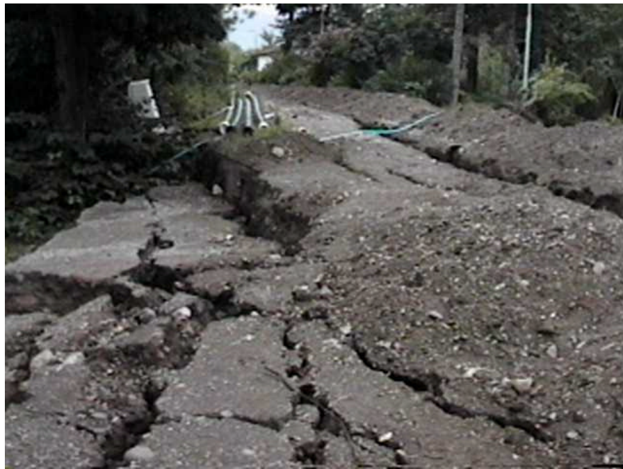
The ground spread laterally close to the ground rupture that went along the fence of the Ford plant in Golcuk (N40°42.818', E29°51.098', 8/28/99, 13:49:32).
