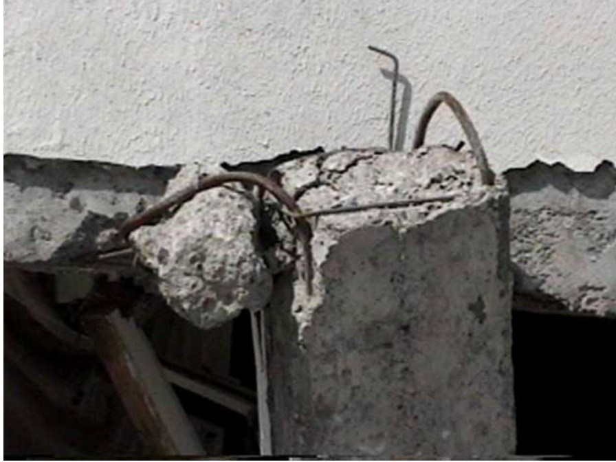
The steel rebars at the connection between the reinforced concrete columns and beams of some of the apartment buildings along the shoreline of Yalova were smooth and totally insufficient (N40°40.913', E29°21.234', 8/26/99, 14:42:20)
