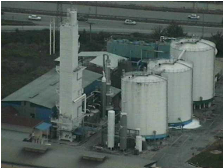
Damage to the middle tank of this chemical plant in the Kosekoy area. The short-column support of the middle tank collapsed and the tank leaned slightly and leaked (N40°45.549', E30°02.344', 8/24/99, 15:33:25).
