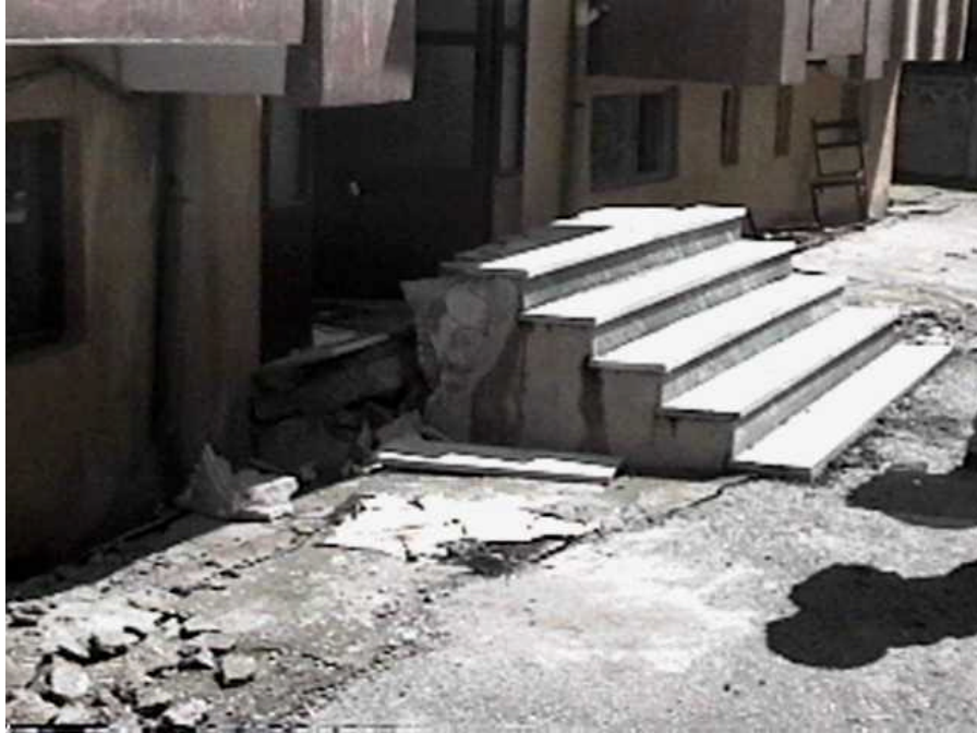
The building settled due to liquefaction, and the connection to the staircase was sheared (Adapazari, N40°46.499', E30°24.646', 8/27/99, 13:47:19).
