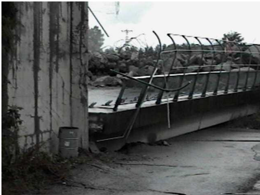
The deck of the bridge fell down on the ground as the fault surface ruptured beneath the bridge (South of Adapazari, N40°42.581', E30°21.495', 8/25/99, 15:40:56).
