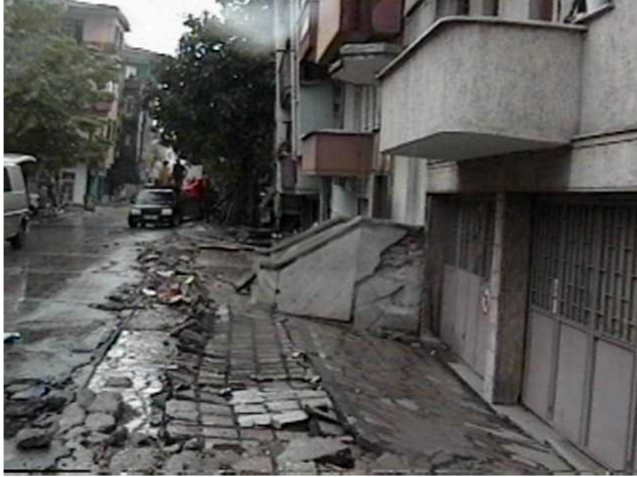
Settlement of building in downtown Adapazari. The staircase was sheared due to settlement (N40°55.202', E29°21.011', 8/25/99, 11:50:23). (The GPS has some problem).
