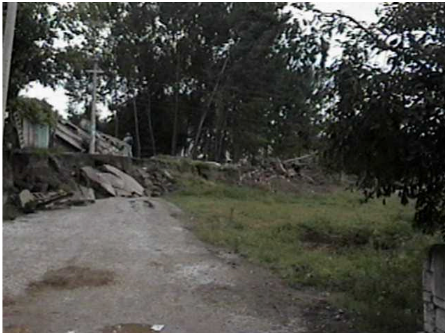
In Golcuk, the ground rupture crossed the road. The vertical offset was about 2 m (N40°43.132', E29°50.52', 8/28/99, 15:51:45).
