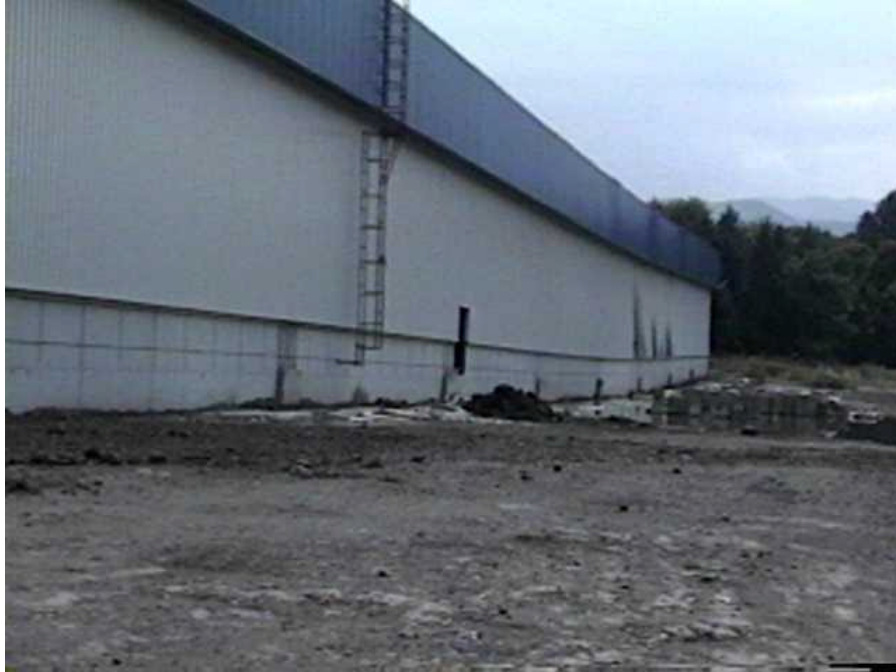
In Golcuk, the Ford plant was under construction. There was obvious evidence of ground rupture in the site. One side of the building subsided differentially, and the wall buckled (N40°42.947', E29°50.89', 8/28/99, 13:21:46).
