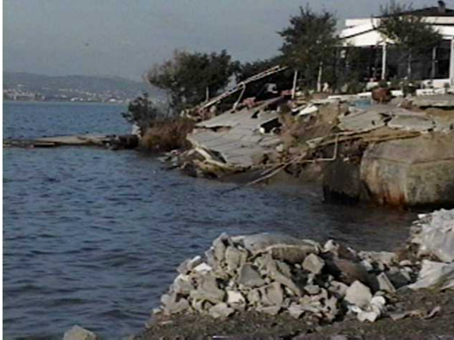
To the west of Golcuk, the waterfront slid into the sea, and exposed two tanks of a gas station (N40°43.074', E29°46.083', 8/28/99, 16:20:48).
