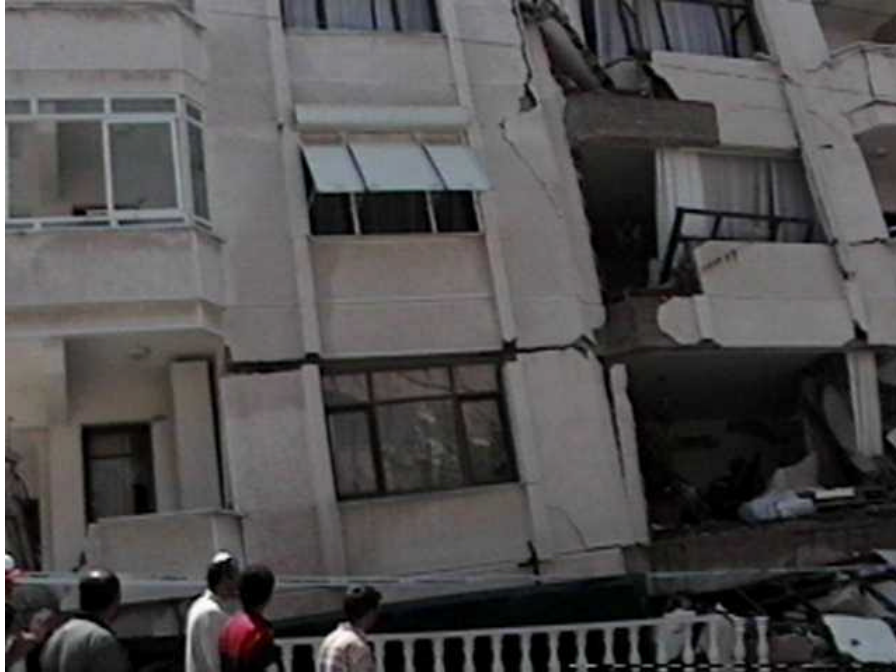
The apartment buildings in Yalova also underwent failure of their first floors (N40°38.845', E29°7.448', 8/26/99, 12:01:06).
