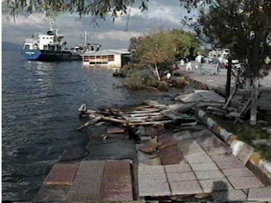
Along the shoreline of Halidere, part of the sidewalk of the waterfront subsided into the sea. The restaurant in the background settled into the sea (N40°43.064', E29°45.019', 8/26/99, 18:01:02).
