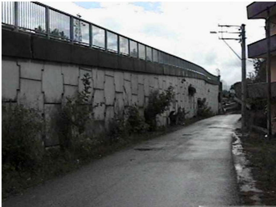
One side of the mechanically stabilized earth abutment showed very few signs of damage (South of Adapazari, N40°42.581', E30°21.495', 8/25/99, 15:40:56).
