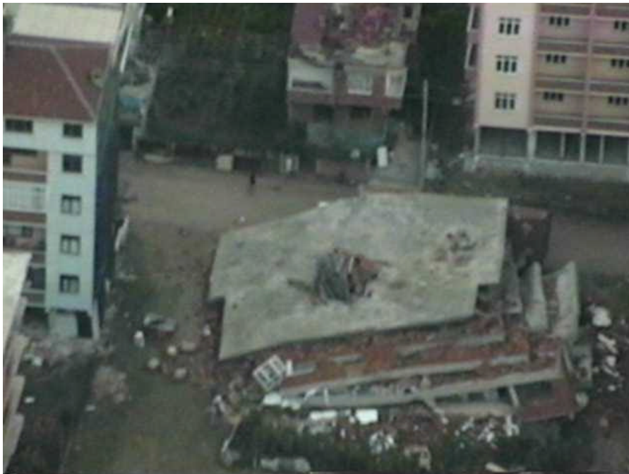
Collapse of a reinforced concrete apartment in the Izmit area. This type of failure was commonly observed after the earthquake, and caused many casualties (N40°45.759', E29°51.987', 8/24/99, 15:27:36).
