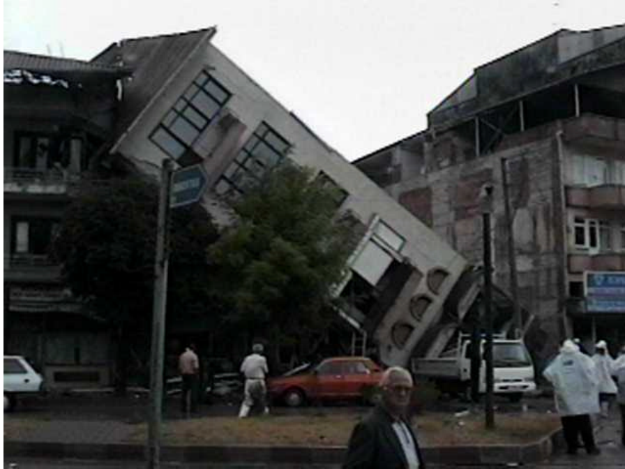
The foundation of this slender building in Adapazari failed and the building leaned onto its neighbor (N40°47.068', E30°23.976', 8/25/99, 12:36:00).
