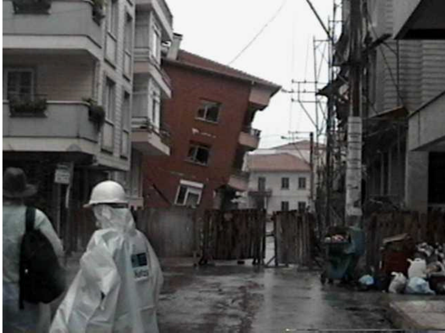
The reinforced concrete apartment building leaned sideways due to the unsymmetric failure of its first floor (N40°55.202', E29°21.011', 8/25/99, 11:38:40, poor GPS coverage).
