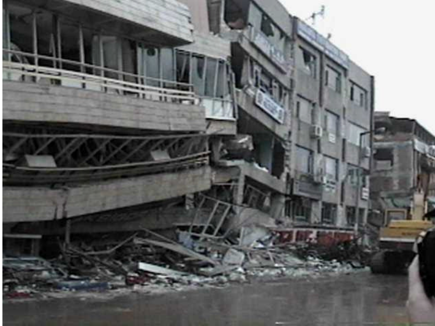
The bottom floors of the reinforced concrete office buildings collapsed in the city of Adapazarı (N40°42.527', E30°21.62', 8/25/99, 10:43:17).
