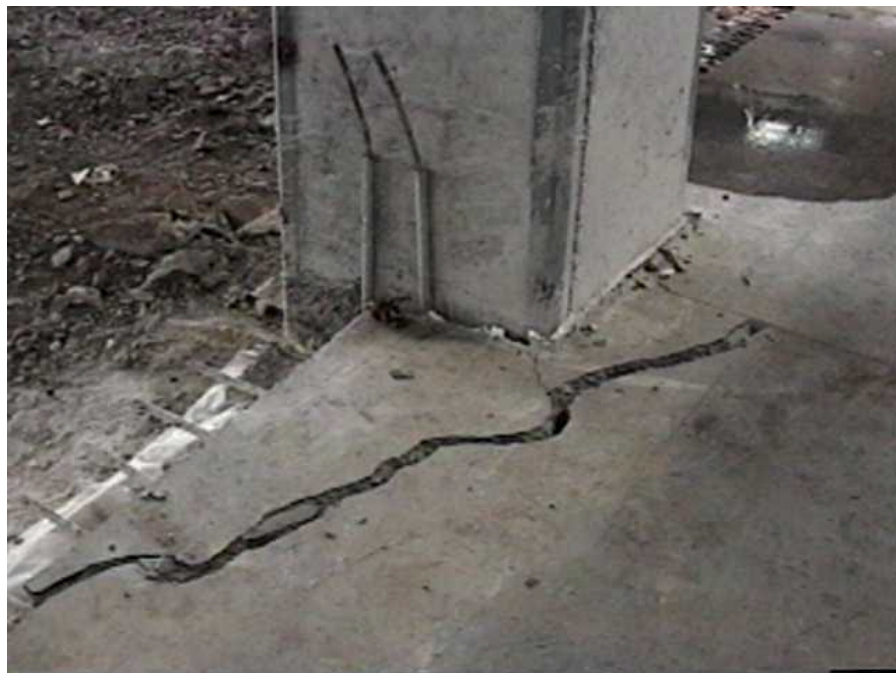
In the reinforced concrete slab inside the Ford plant in Golcuk, there were cracks caused by differential ground displacements (N40°42.947', E29°50.89', 8/28/99, 13:21:46).
