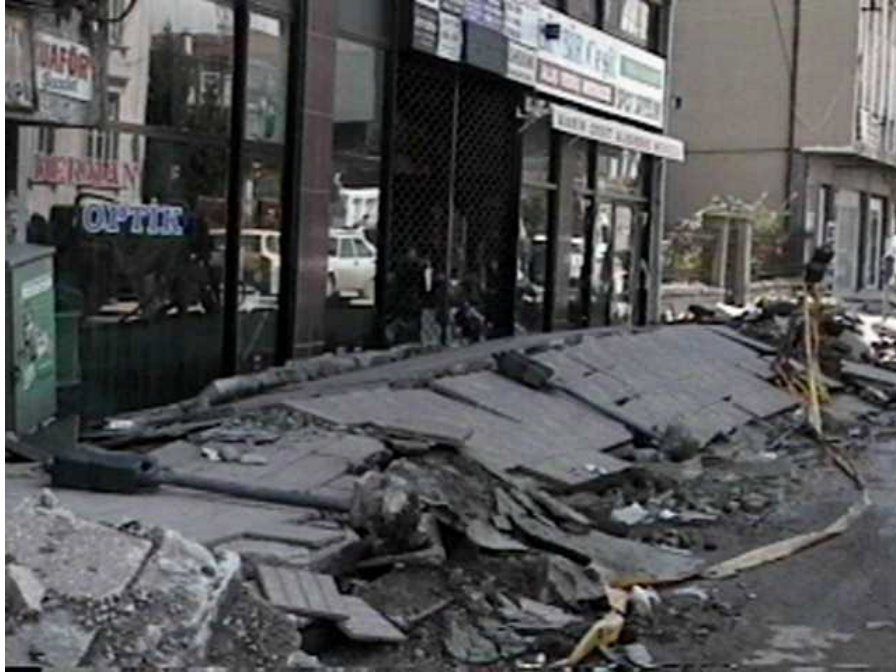
The heaving of sidewalks and settlement of buildings were a common sight in Adapazari (N40°42.581', E30°21.495', 8/25/99, 15:40:56).
