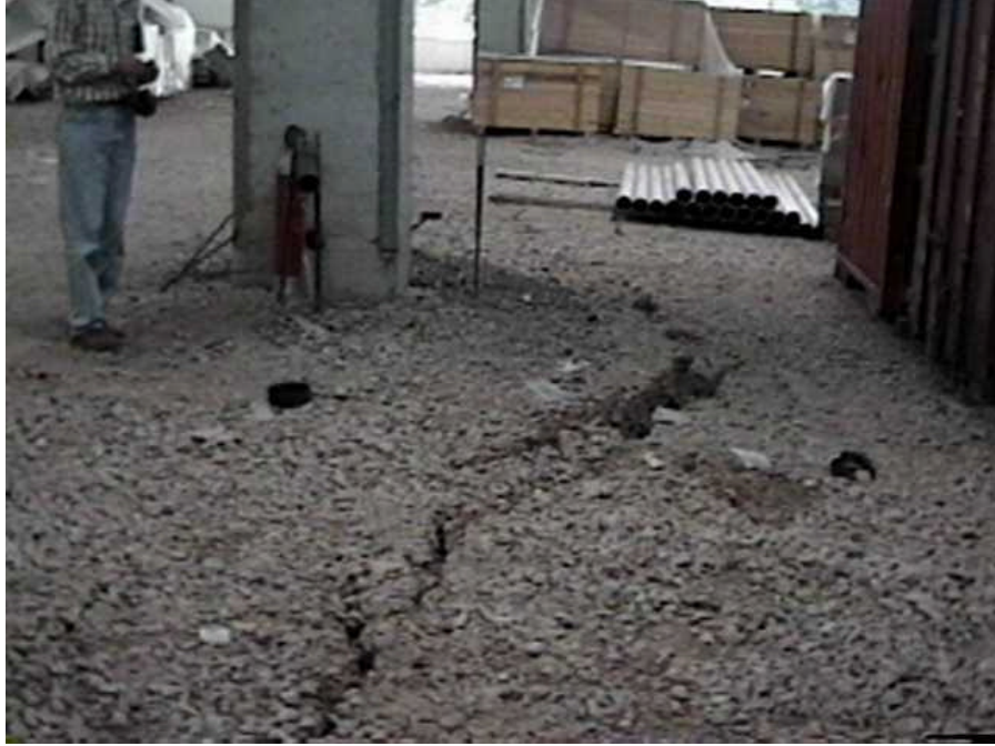
In the unpaved ground of the Ford plant in Golcuk, there were ground cracks (N40°42.947', E29°50.89', 8/28/99, 13:21:46).
