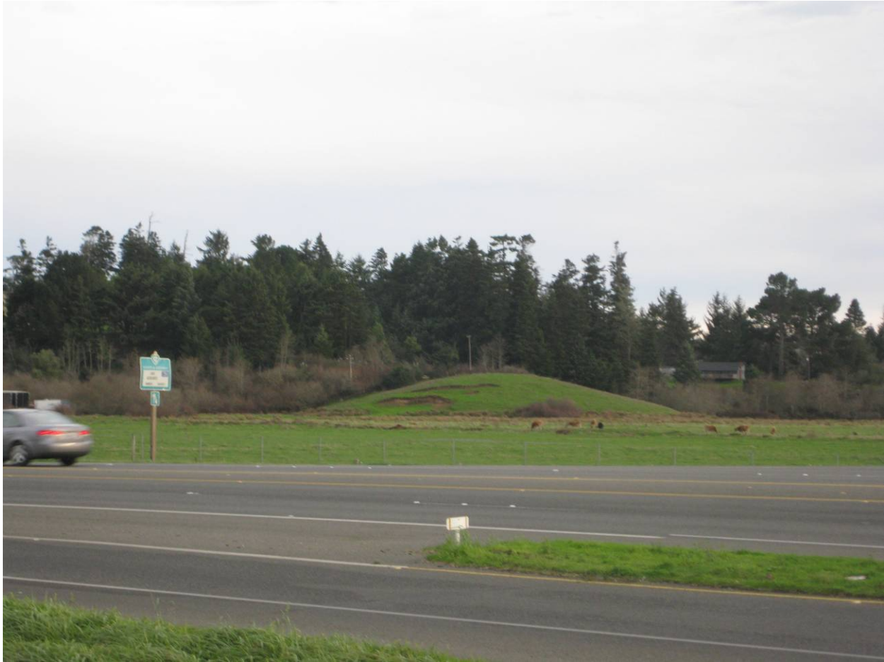
Figure 17 Landslide features on an earthen slope at the east of HWY 101, approximately 640 m north of Pound Road (40.763860N; 124.186335W). It was not possible to easily access the site, so it was not possible to ascertain potential for seismic induced movement.
