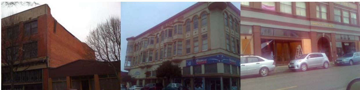
Figure 29 Damaged URMs in downtown Eureka.
