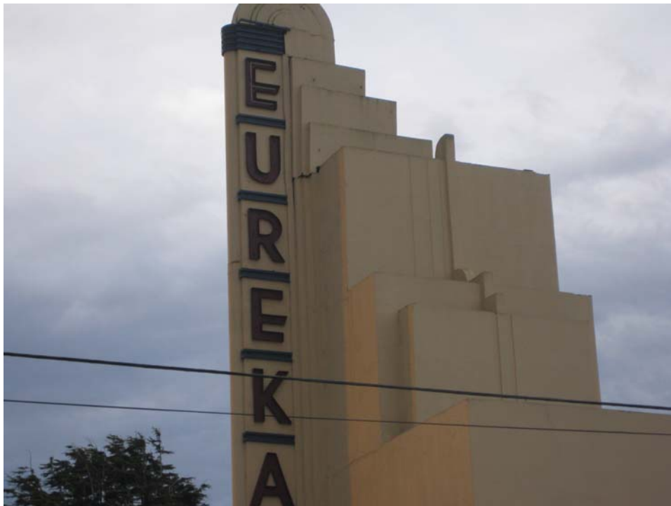
Structural damage to the Eureka Theater building at the corner of 6 th and F Street in Eureka, California.
