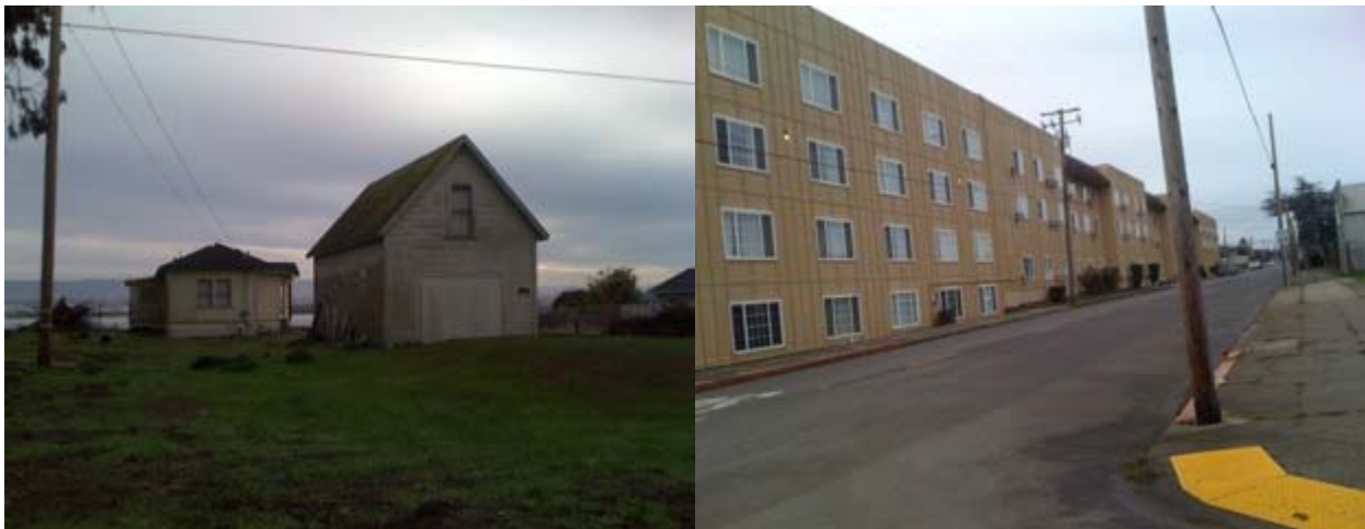
Figure 27 Many types of multistory wood buildings were undamaged.
