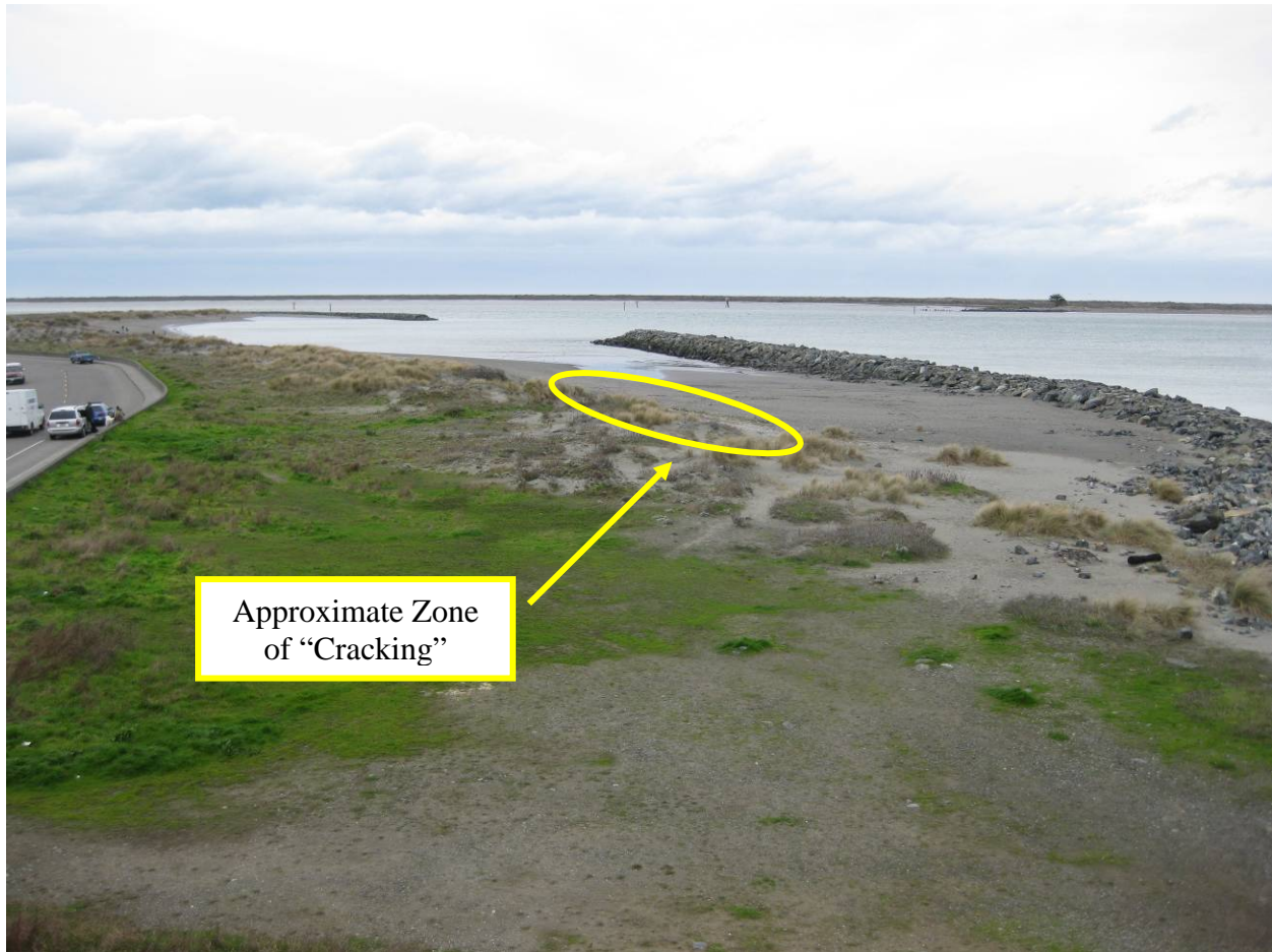
Figure 20 Approximate extents of the 'cracking features' shown in Figure 19.
