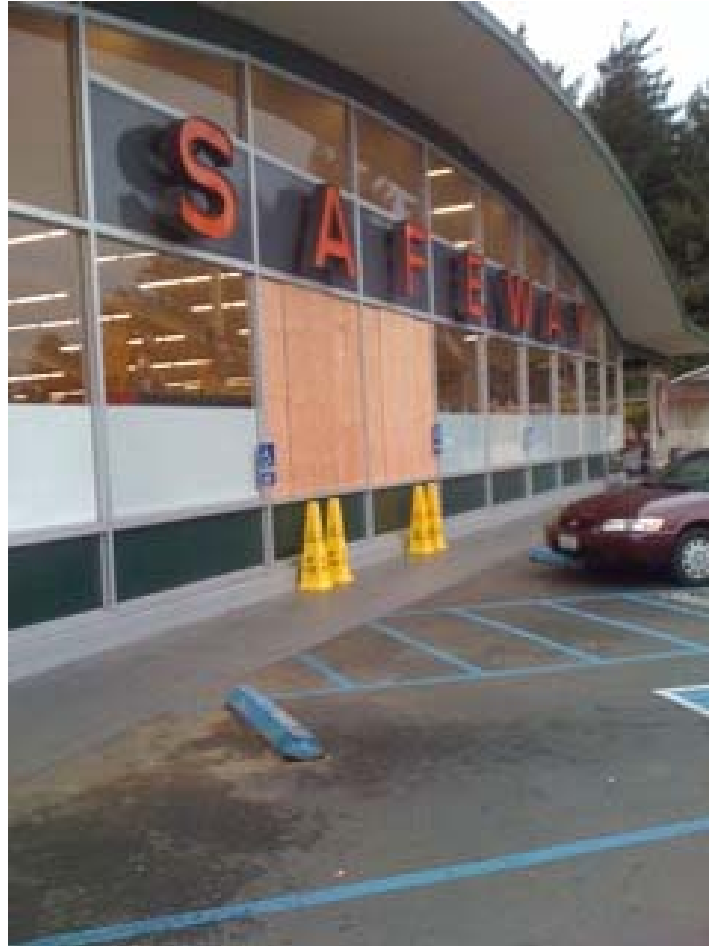
Figure 31 A Safeway grocery store with two broken windows.
