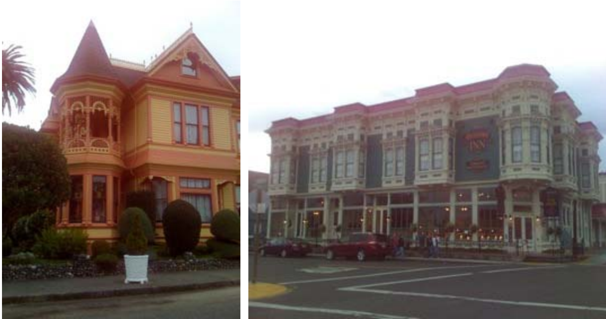
Figure 34 There seemed to be a lot of nice Victorian houses and commercial buildings that appeared to have soft stories or cripple walls. No damage was seen.
