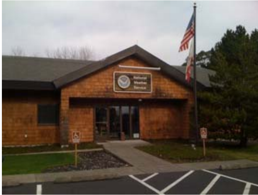
Figure 33 Wood-framed buildings on Woodley Island appeared to suffer no physical damage.
