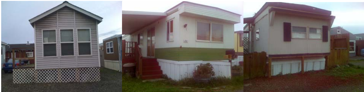
Figure 28 Evidence of lateral displacements on mobile homes in the Eureka area.
