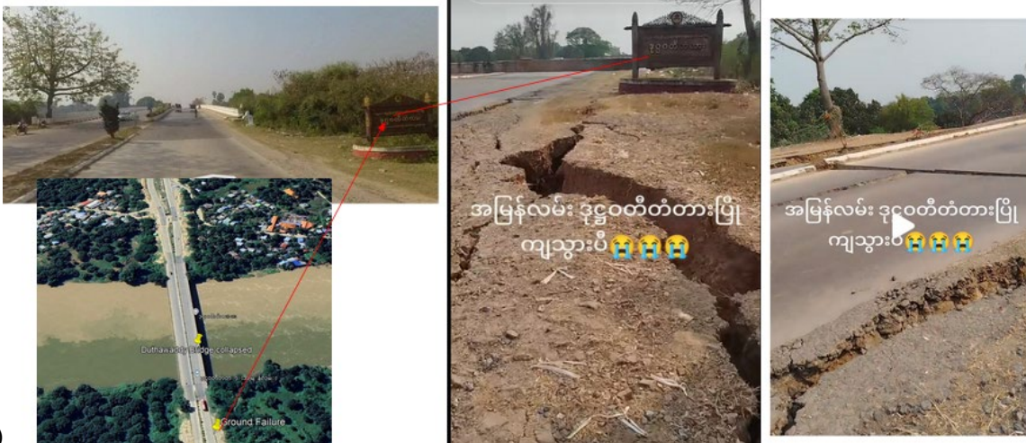
Figure 6.2.4. Dutthawaddy (U Man Lay) Bridge crossing Myitnge River: (a) roadway and abutment damage (Source: Extracted from video from @fri4800 on TikTok ); (b) approach and shoulder road failure with wide separation (Source: Extracted from video from @aungsl1 on TikTok ).
