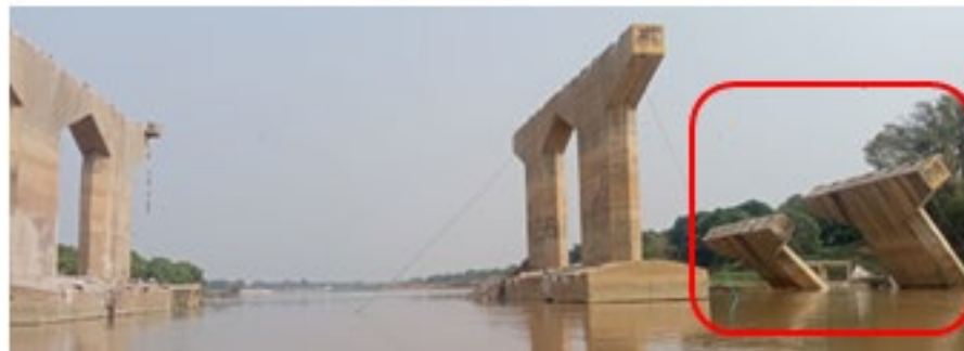
Figure 6.2.3. Dutthawaddy (U Man Lay) Bridge crossing Myitnge River: (a) satellite images before (top) and after (bottom) the earthquake (Credit: Gansu Data and Application Center for High-Resolution Earth Observation System); (b) unseated bridge decks and overturned piers (Source: Khit Thit Media on Facebook ).
