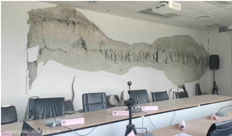
Figure 5.5.2. Shear wall compression and bar buckling failure (Source: CSI LA Facebook post ).
