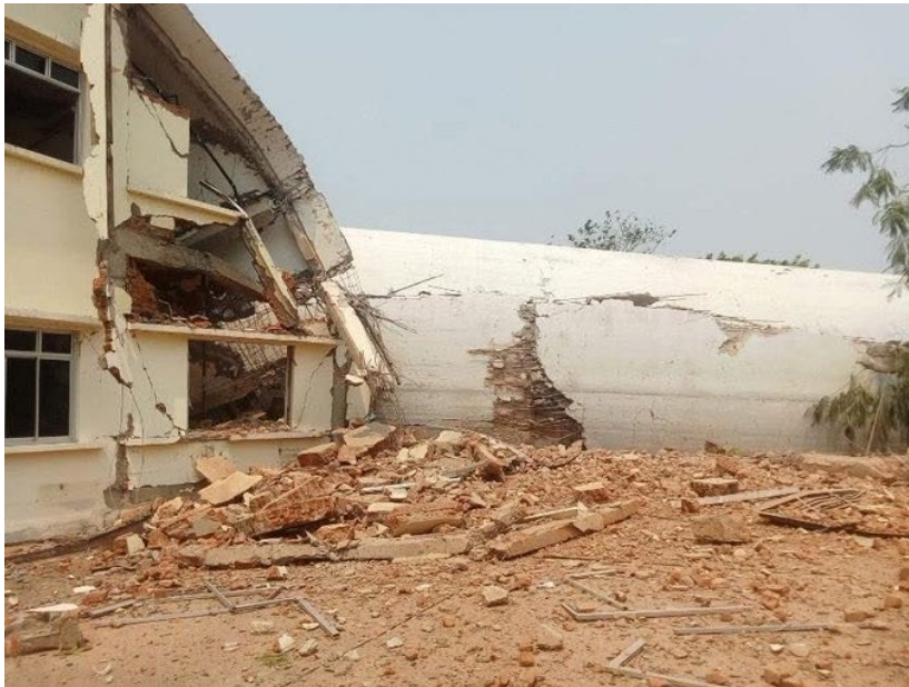
Figure 6.2.7. Collapsed airport control tower of the Nay Pyi Taw airport due to biaxial bending resulting from combined effect of horizontal ground motion components (Source: @heungburma on X ), with aerial imagery of condition before and after earthquake (Sources: before, Airbus, Maxar Technologies; after, Maxar Technologies).
