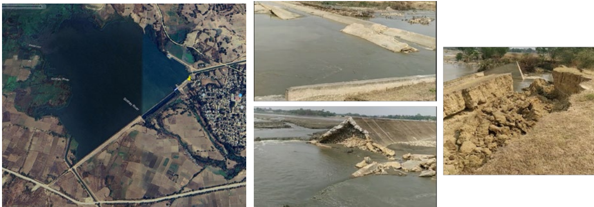
Figure 4.5.1. SinThe Dam aerial view (left) with images of post-earthquake damage. [Location 20.159054, 96.121426] (Sources: Google Earth (left) with still images extracted from video posted by @heinwaisoe073 on TikTok).
