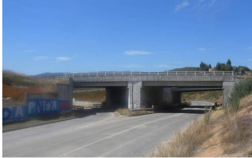
Figure 12.5. Multiple retaining structures for highway overpass structures south end of Coronel (37.0455°S, 73.1421°W)
