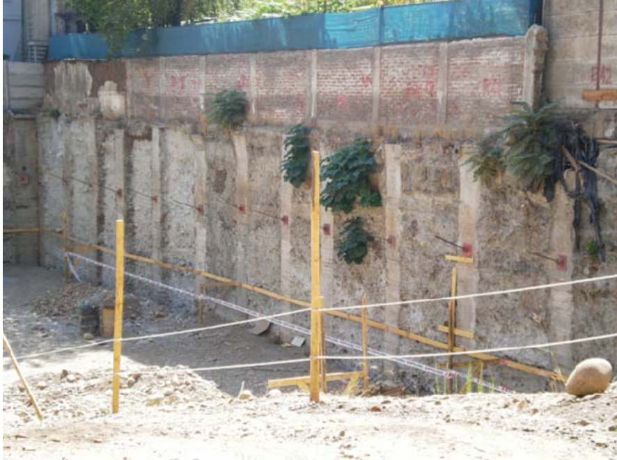
Figure 12.11. Undamaged temporary retaining structure in Santiago.
