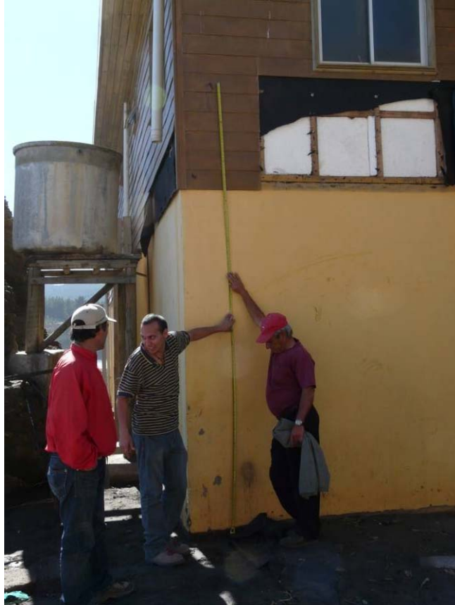
Figure 13.27. Damaged siding on this building suggests tsunami flow depths reached at least 3.5 m at the west end of Bucalemu (S34.640097° W72.044194°, 1130 hrs on 03/15/2010).
