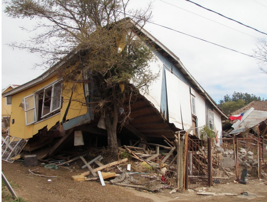
Figure 13.17 The home in this picture was lifted by the 3rd wave and dropped onto a tree (S36.547°, W72.939°, 2010 hrs, 3/13/10).
