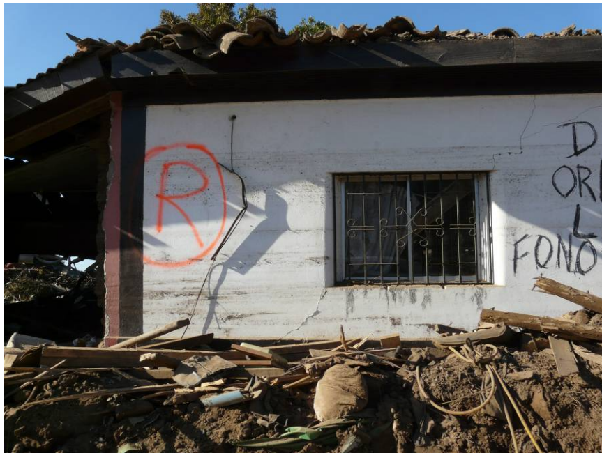
Figure 13.25. Watermarks on damaged buildings in Constitución indicate tsunami flow depths reached at least 2 m along the waterfront on Calle Blanco (S35.336 W72.403, 1757 hrs on 03/15/2010).
