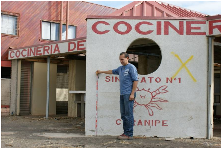
Figure 13.21. Watermarks on a restaurant in Curanipe indicate minimum tsunami flow depths of 1 m at this location (S35.8436°, W72.6365°, 03/17/2010).
