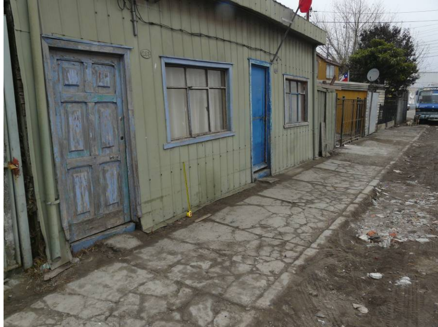
Figure 13.4. Tsunami flow depths reached a minimum of 0.63 m at this green house on El Morro Street in Talcahuano (S36.727354° W73.109530°, 1206 hrs on 03/16/2010).
