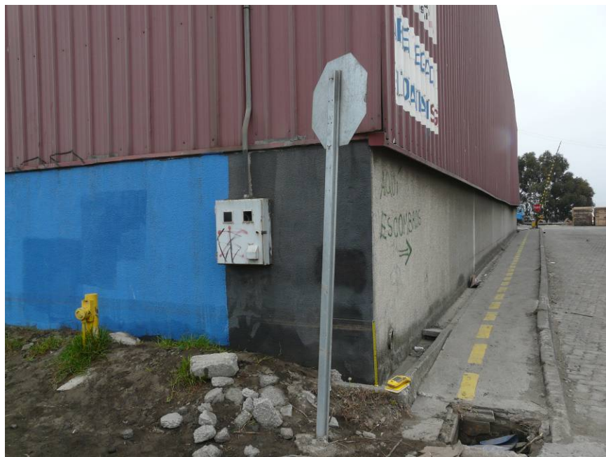
Figure 13.3. Tsunami flow depths reached a minimum of 0.65 m at this waterfront warehouse in Talcahuano along Perez Gacitua Street (S36.728263° W73.109199°, 1136 hrs on 03/16/2010).
