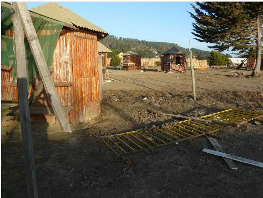
Figure 13.30. At Puente Cahuil tsunami flow depths reached a minimum of 0.3 to 0.4 m and pushed kiosks at a campground several tens of meters landward (S34.479276° W72.017610°, 1922 hrs on 03/14/2010).
