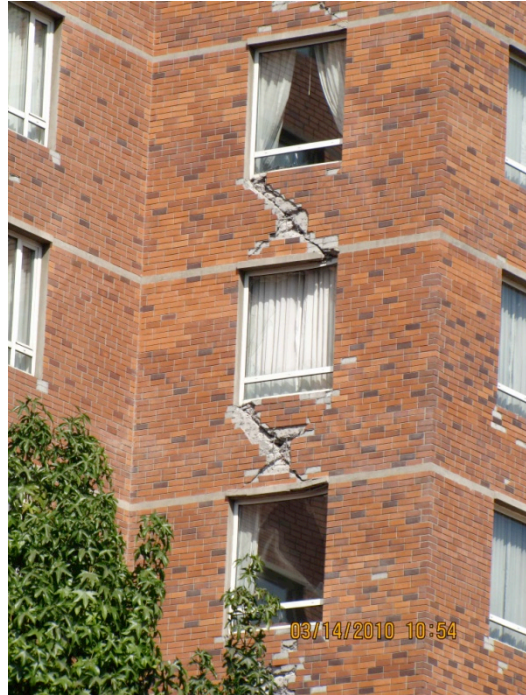
Figure 5.14. Site DA005 ( S33.387652^{\circ} W70.617123^{\circ} , 1054 hrs on 03/14/2010) 12-story building with severe structural damage.
