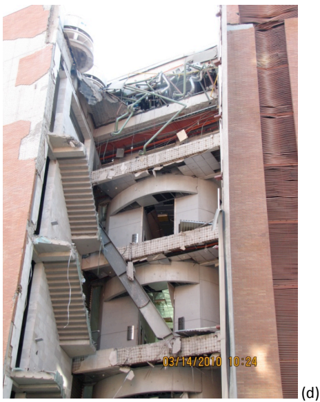
Figure 5.11. Site DA003 ( S33.387985^{\circ} W70.618815^{\circ} , 1015 hrs on 03/14/2010) 6-story commercial building. Damage of non-structural elements (glass windows, red brick façade) (Figures 11a,b) and emergency staircase (Figures 11c,d). Evidence of ground deformation (Figure 11e).
