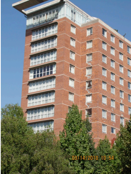
Figure 5.14. Site DA005 ( S33.387652^{\circ} W70.617123^{\circ} , 1054 hrs on 03/14/2010) 12-story building with severe structural damage.
