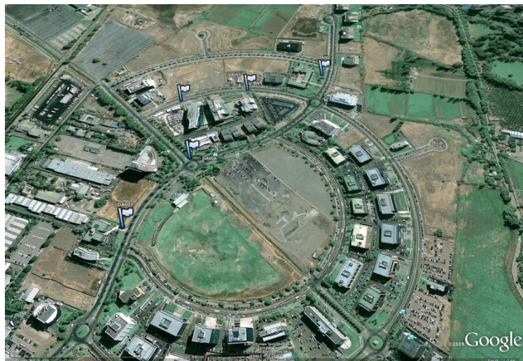
Figure 5.9. Aerial view of Ciudad Empresarial, depicting the structures that were inspected during reconnaissance.
