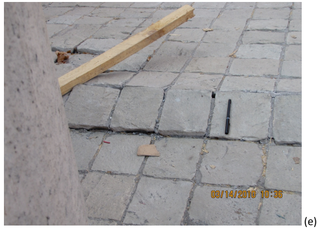
Figure 5.11. Site DA003 ( S33.387985^{\circ} W70.618815^{\circ} , 1015 hrs on 03/14/2010) 6-story commercial building. Damage of non-structural elements (glass windows, red brick façade) (Figures 11a,b) and emergency staircase (Figures 11c,d). Evidence of ground deformation (Figure 11e).
