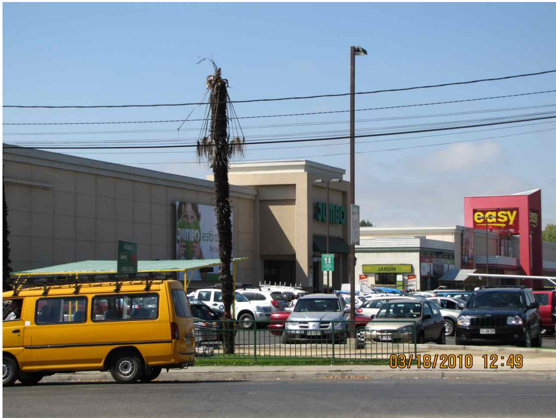
Figure 5.29. Modern (engineered) structures adjacent to the river that showed no or minor damage (S 35.437897° W 71.660151°, 1249 hrs on 03/18/2010).
