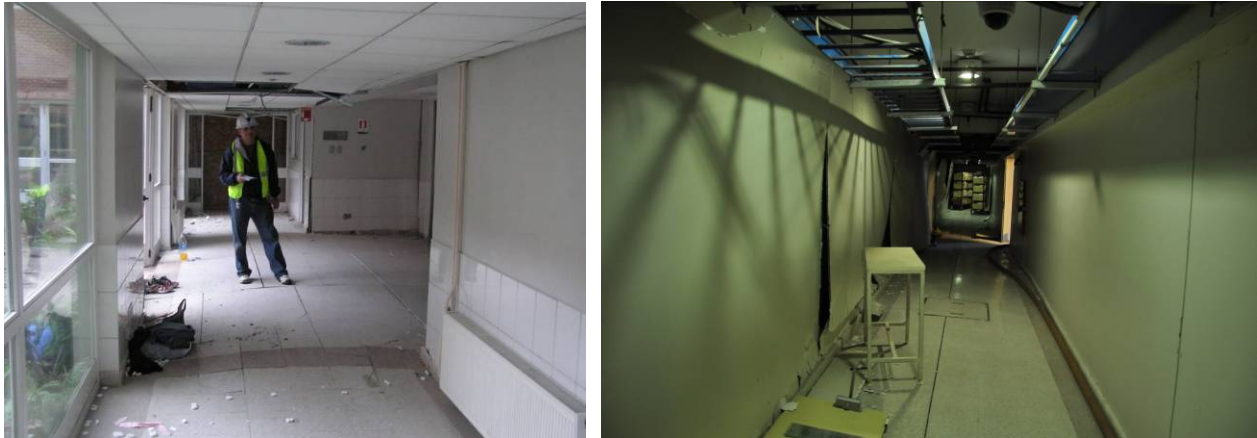
Figure 7.9. Distortion of the slab-on-grade: (a) floor bulging in front of elevator shaft in Wing 1C (S37.47345°, W73.34835°), and (b) floor distortion in eastern hallway of Wing 1B (S37.4733°, W73.3478°).
