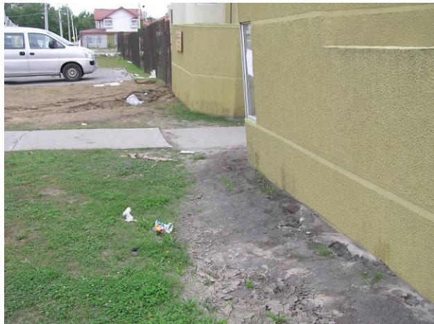
Figure 7.19. Sediment ejecta, ground cracks, and other evidence of liquefaction of the sandy fill were found throughout the condominium site; however, street curbs around the property did not show evidence of liquefaction (S36.79107°, W73.08149°; 1300 hrs on 03/17/10).
