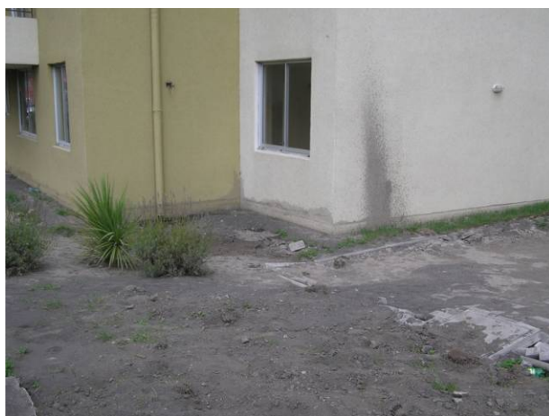
Figure 7.20. Riesco building that underwent most significant liquefaction-induced movement. Left photo shows evidence of large sediment ejecta at its northeast corner (S36.79077°, W73.08124°; 1330 hrs on 03/17/10). Right photo shows entrance to the building in the middle of its east facing side (S36.79089°, W73.08131°; 1310 hrs on 03/17/10).
