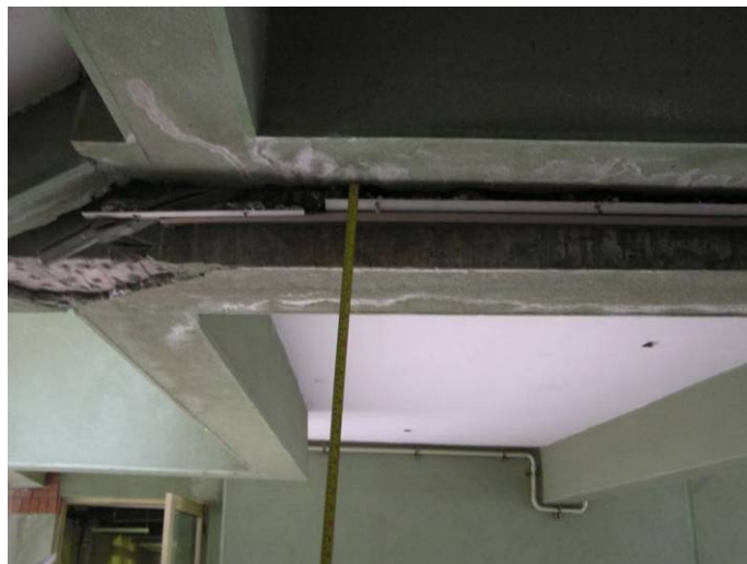
Figure 7.10. Relative movement between Wing 1B (in the background) and Wing 2G (in the foreground) (S37.47335°, W73.34786°; 03/16/10).
