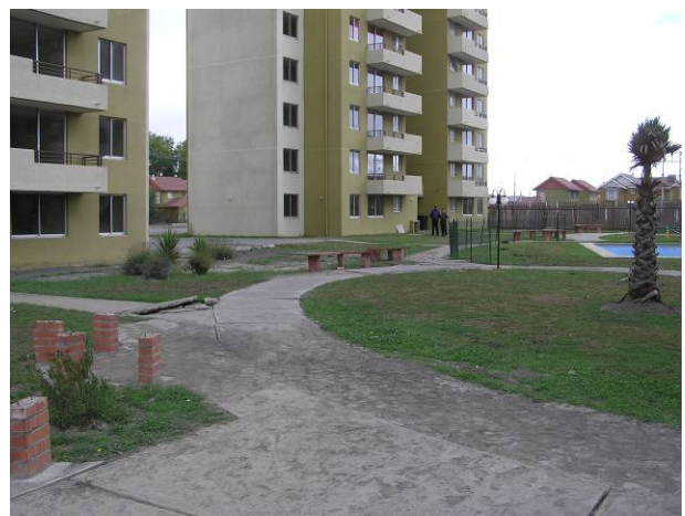
Figure 7.19. Sediment ejecta, ground cracks, and other evidence of liquefaction of the sandy fill were found throughout the condominium site; however, street curbs around the property did not show evidence of liquefaction (S36.79107°, W73.08149°; 1300 hrs on 03/17/10).
