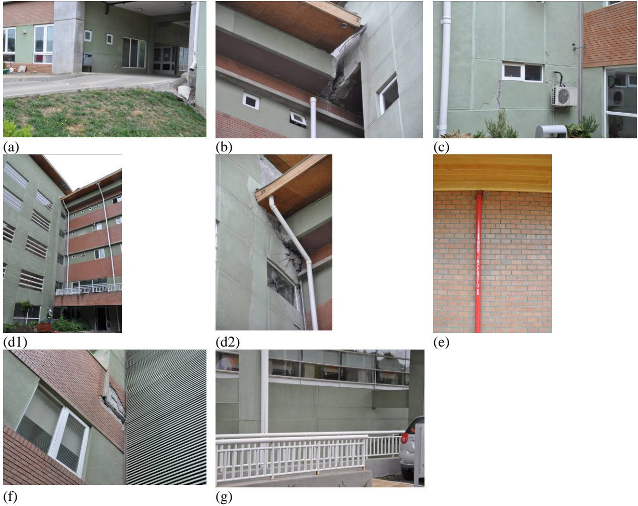
Figure 7.12 Most pronounced structural damage observations. (a) approach ramp to entrance bay at wing 1A (S37.473084°,W73.348712°), (b) pounding damage and resulting permanent gap developed between wings 1A-1C due to the easterly rocking of wing 1C (note the gap was measured by hospital staff as 37 cm after the main event on February 27, 2010) (S37.473376°, W73.348452°), (c) damage to shear wall of wing 1C due to contact with wing 1D (S37.473537°, W73.348488°), (d1) elevation view of the interface between wing 1B-1C and (d2) local view at the roof line of wing 1B observing the pounding between these two wings (S37.473406°,W73.348304°), (e) vertical cracks in masonry in-fill of wing 2H (S37.473713°, W73.347839°), (f) fallen masonry façade and spalling of structural wall of wing 1F due to impact with wing 1B (S37.473494°, W73.347948°), and (g) cracking damage at in-fill and structural shear wall interface at front of wing 2I-2J (S37.473528°, W73.347363°). Images taken at 1430, 1715, 1415, 1725, 1725, 1350, 1625, and 1645 hrs, respectively, on 3/16/2010.
