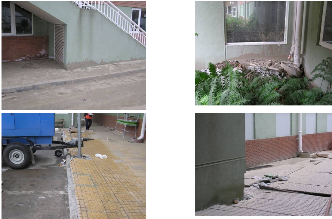
Figure 7.7. Sediment ejecta observed around hospital wings; (a) ejecta observed along exterior staircase of Wing 1D (S37.47358°, W73.34890°), (b) ejecta observed along exterior of Wing 1C (S37.47342°, W73.34829°), (c) ejecta observed along south side of Wing 1D(S37.47375°, W73.34851°), and (d) ejecta observed along east side of Wing 2G (S37.47343°, W73.34788°).
