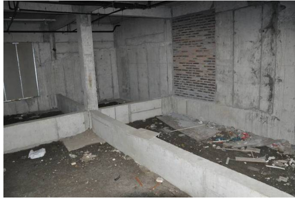
Figure 7.6. General configuration of the foundation, perimeter structural shear walls and interior gravity columns (view at ground floor of wing 2I looking east) (S37.47366°, W73.34761°; 1625 hrs on 3/16/2010)
