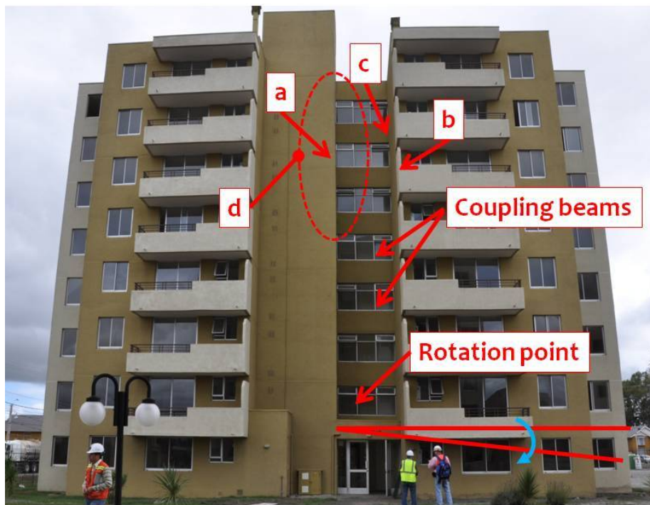
Figure 7.23. Elevation of the Riesco building depicting the movement characteristics (about transverse axis only) and resulting damage map – refer to Figure 7.24 for images of a-d (image taken at S36.790929°, W73.081296°; 1400 hrs on 3/17/2010).
