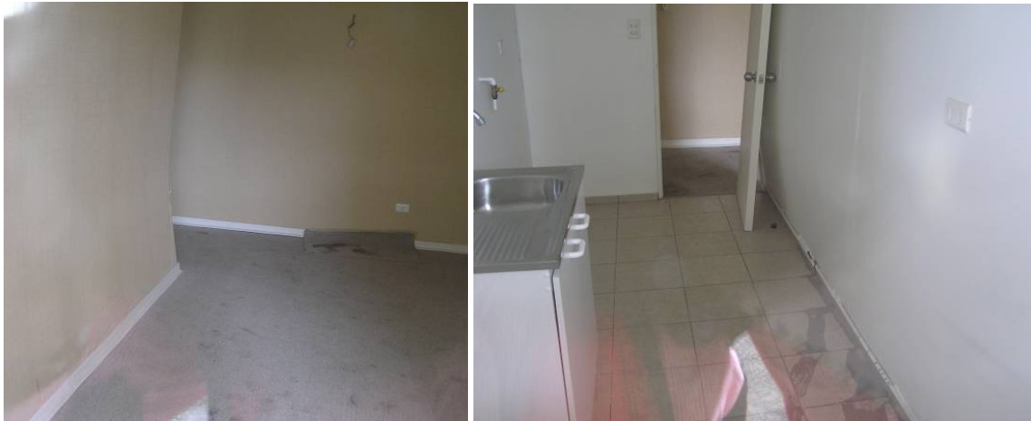
Figure 7.21. Evidence of interior damage to Riesco Building due to differential foundation movement (S36.79085°, W73.08128°; 1320 hrs on 03/17/10).
