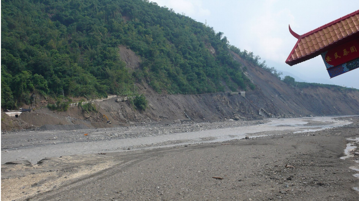
Photo 2-3-2. Large scale landslides along Shinbao Road [Location 2]
