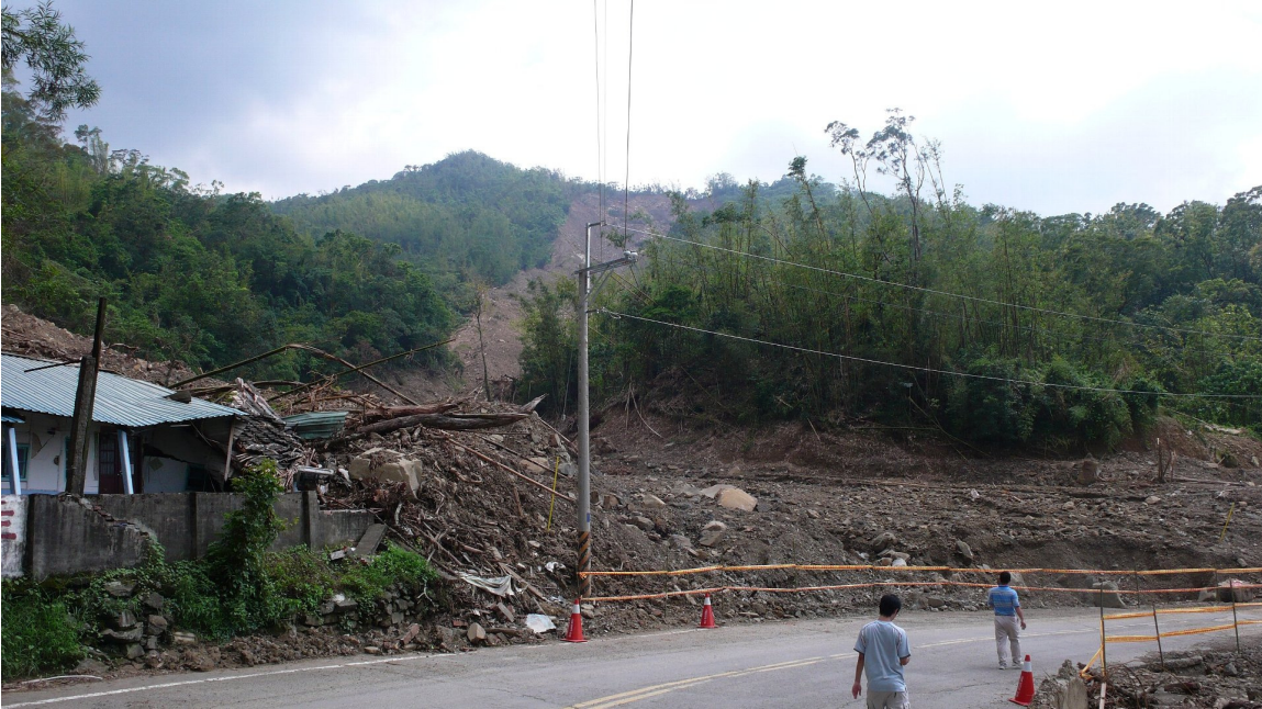
Photo 2-1-9. Debris flow that originated from the mountain buried a home.
