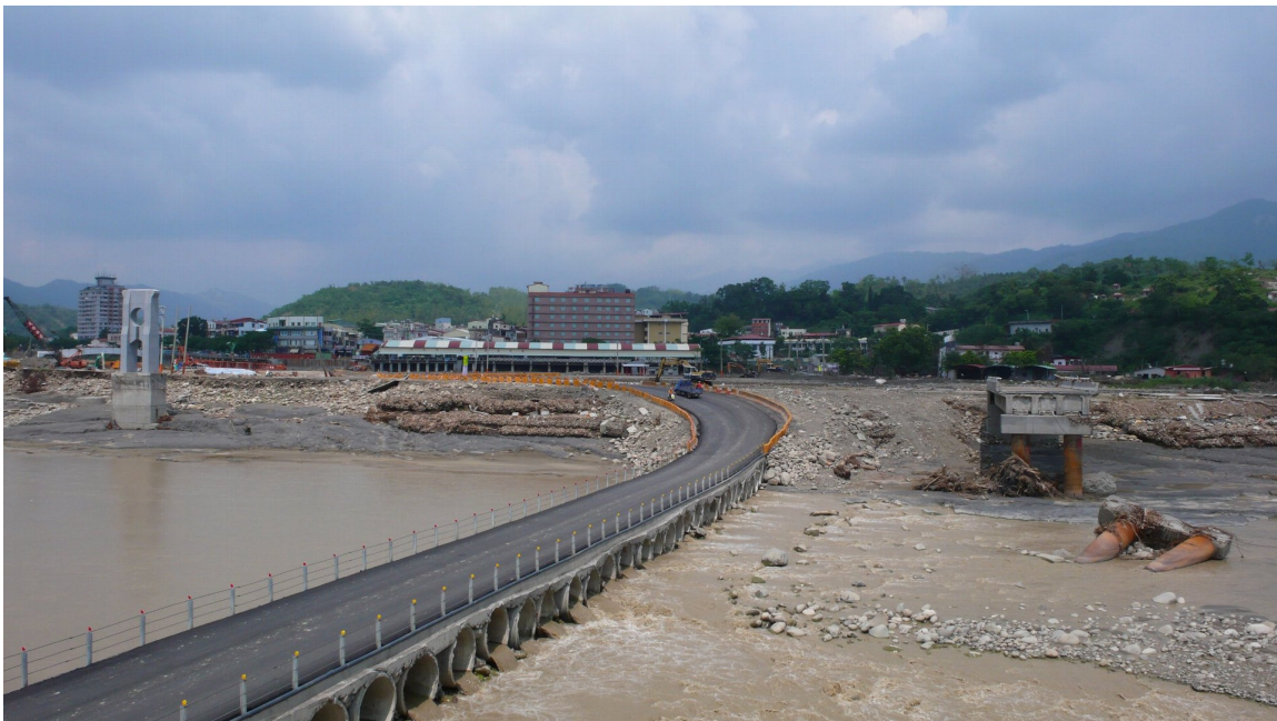
Photo 2-1-2. Temporary access bridge near Jia Xian Bridge.
