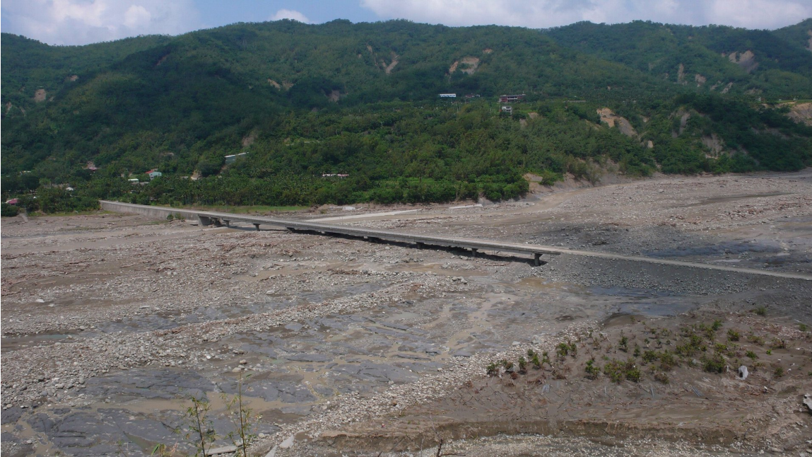
Photo 2-1-7. A bridge nearby Jia Xian Bridge remained intact. The river was filled with debris.
