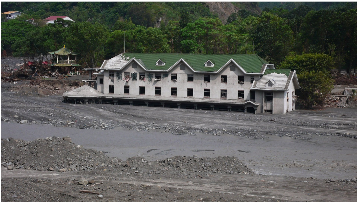
Photo 2-3-3. First floor of a hotel buried by debris [Location 3]
