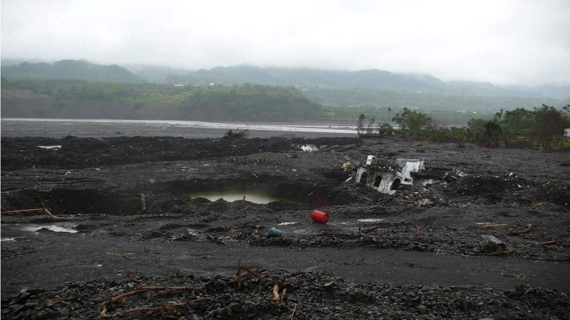
Photo 2-4-2. Excavation of buried buildings.
