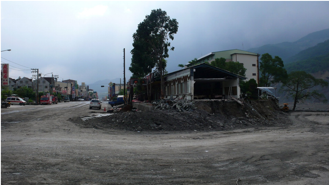
Photo 2-3-7. A building near Bridge #2 was damaged by the debris flow.
