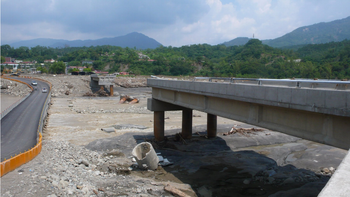
Photo 2-1-1. Collapsed Jia Xian Bridge.
