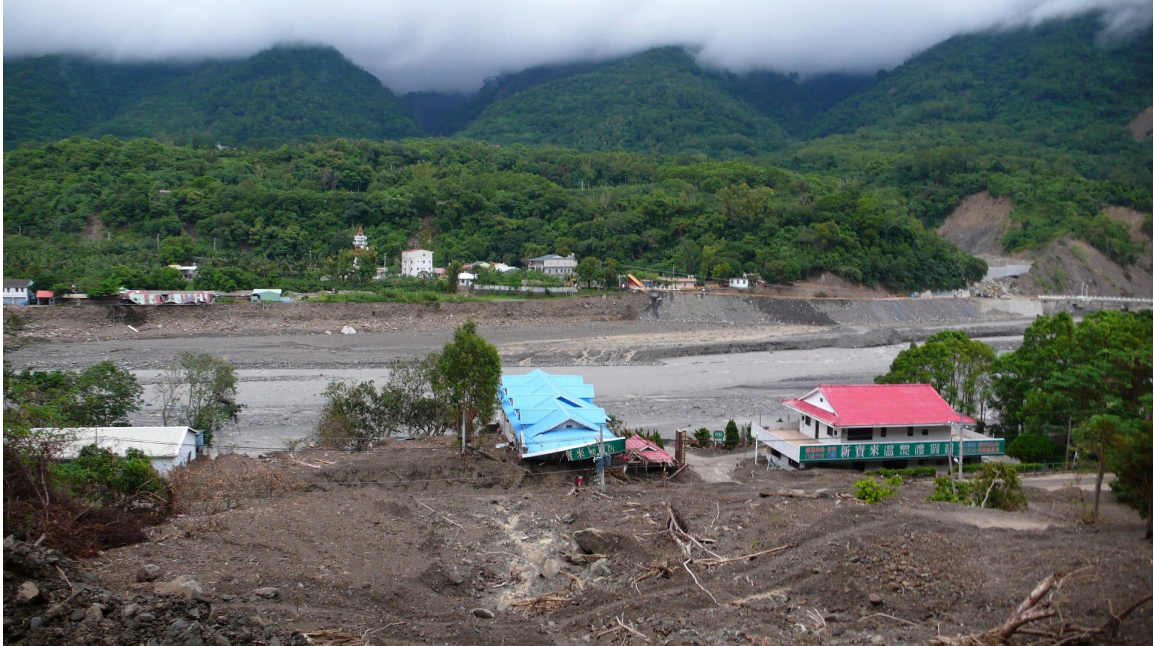
Photo 2-3-4. Buildings damaged by scouring and debris flow [Location 3]
