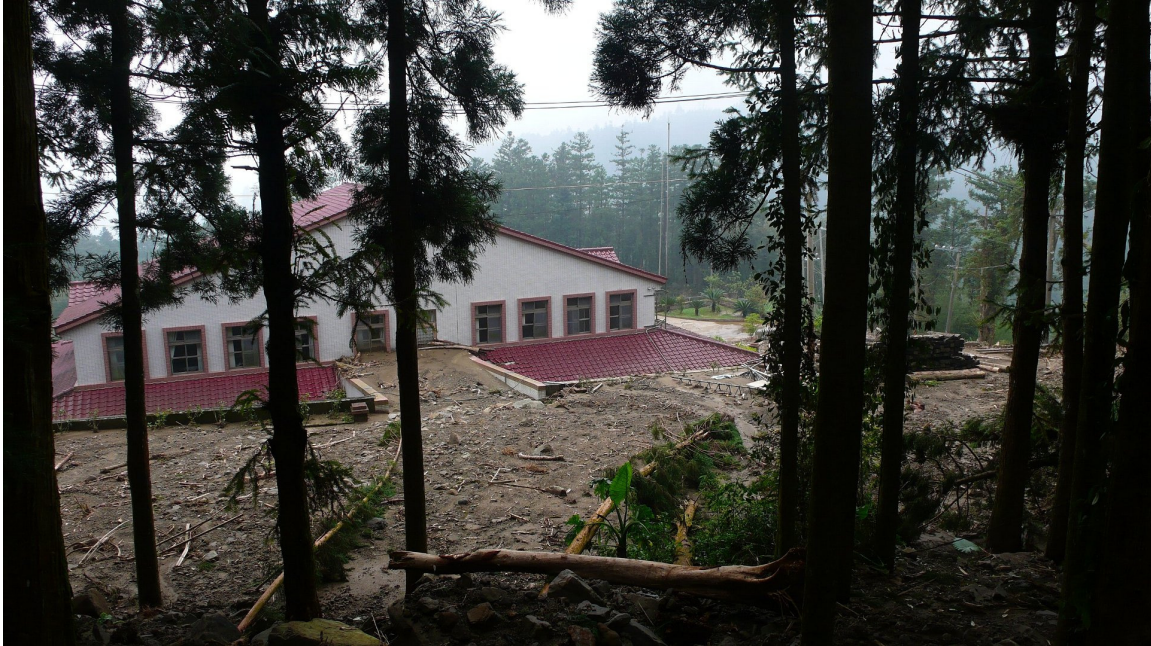
Photo 5-6-3. A building partially buried by debris flow
