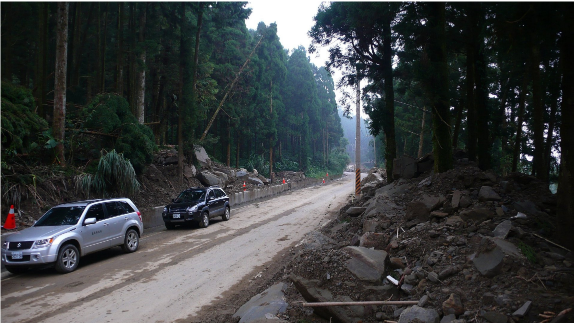
Photo 5-6-2. Debris flow with boulders and gravel of various sizes. The road has been cleared for traffic.
