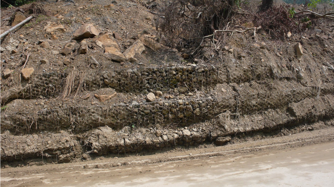
Photo 5-2-4. Gabions were used in the lower part of the slope.
