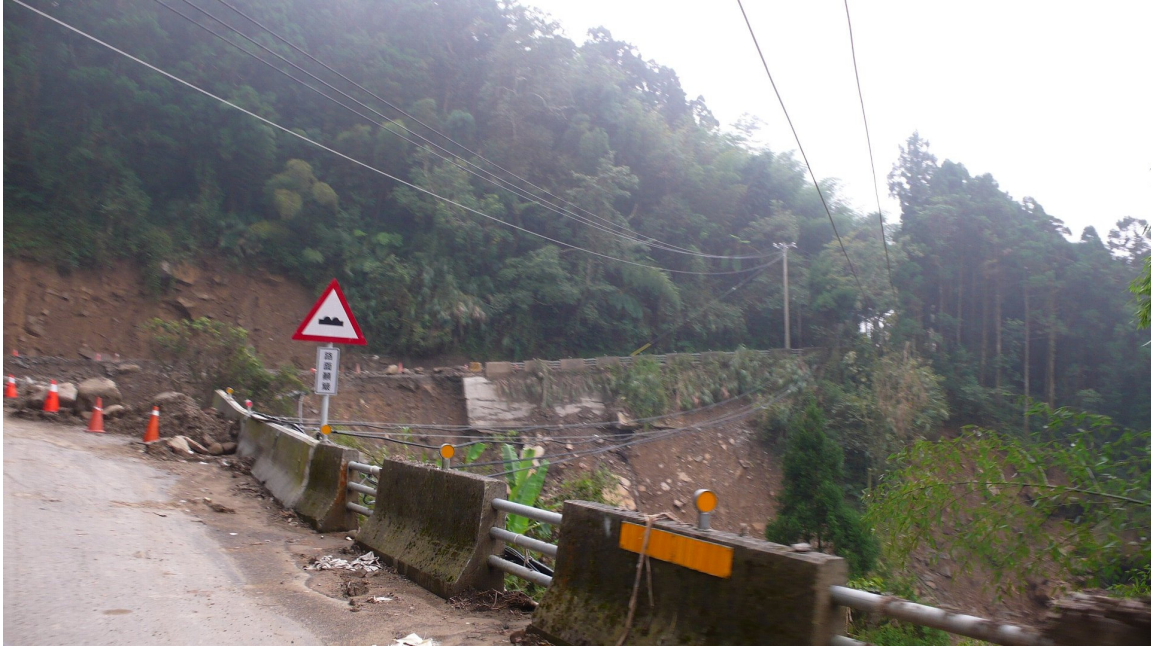
Photo 5-6-5. A different form of barrier which allowed free drainage of rainwater.
