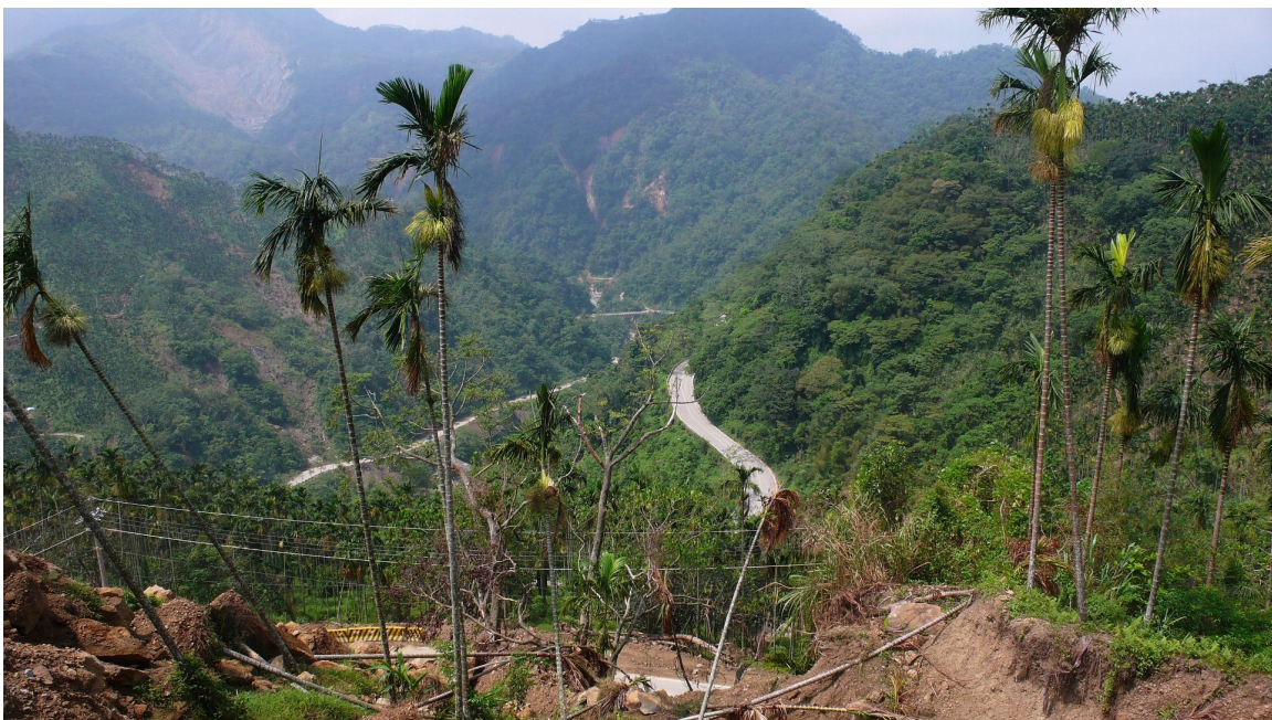
Photo 5-2-7. The beetle nut plantation was damaged by soil movement. Part of Route 18 and other landslide sites can be seen in the photo.
