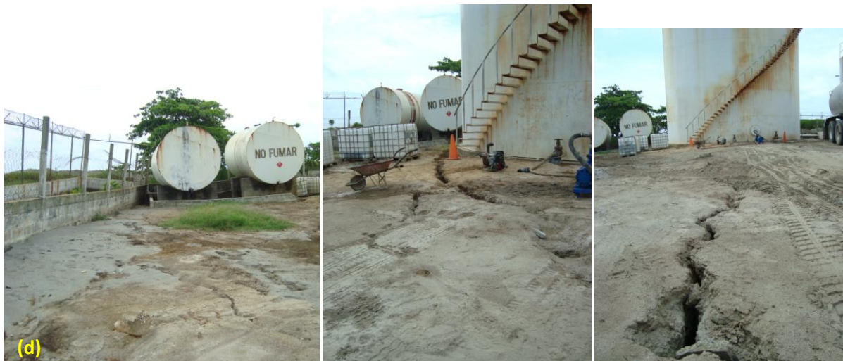
(d) Three view of fuel tanks and multiple ground fissures due to wide spread liquefaction [06/20/2009, 3:12PM, N15.846936, W87.963225]
