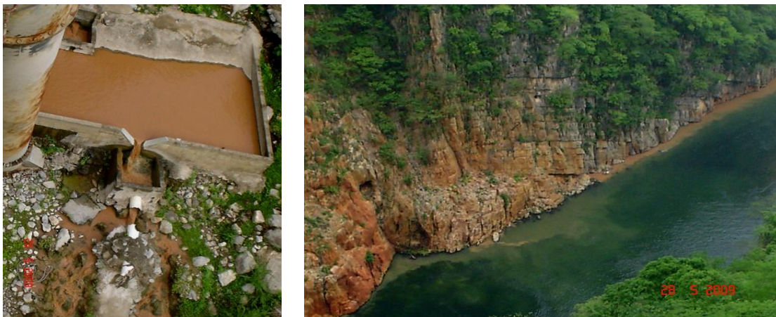
Figure 16 – (a) Weir passing turbid water at base of dam [05/28/2009, N15.03096, W87.747885], and (b) reflected in downstream river [05/28/2009, N15.03096, W87.747885].
