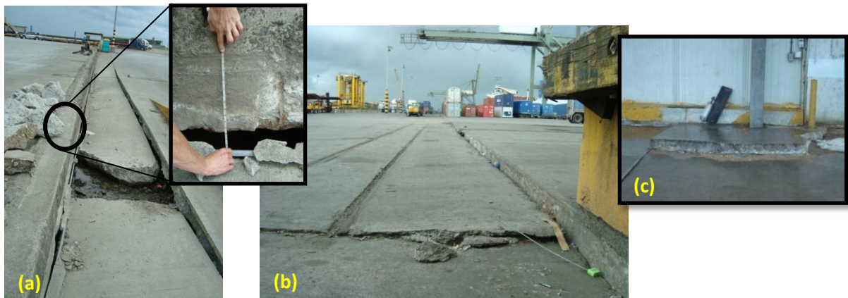
(a) Up to 0.46m at the main dock [06/20/2009, 3:37PM, N15.843718, W87.951739], (b) 0.2m near port warehouses [06/20/2009, 3:49PM, N15.8424, W87.94941], and (c) Relative foundation displacement up to 0.15m [06/20/2009, 4:00PM, N15.841912, W87.941644].
