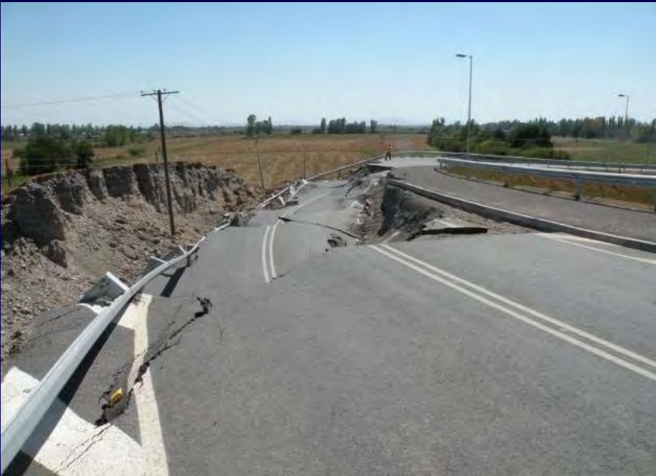
Optical & LIDAR Images: failed embankment on Ruta 5 (2010 Chile EQ - Kayen in Bray & Frost 2010)
