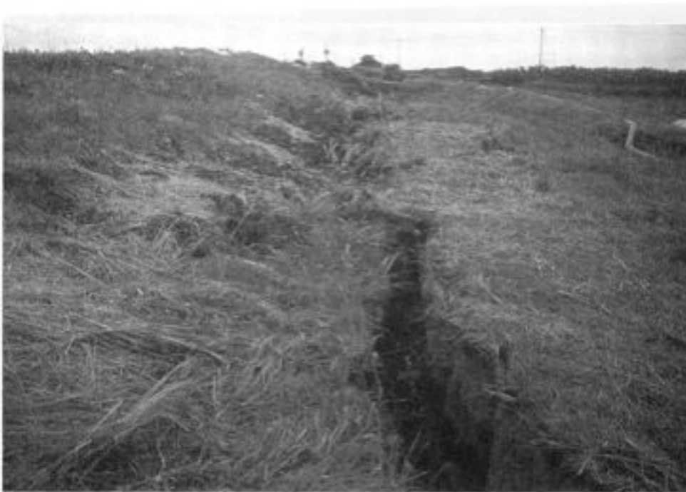
Figure 6-58 Dike along north bank of Assabu River: view along north flank showing fissure with southward-facing scarp (facing toward dike), indicating flank had risen relative to dike.
