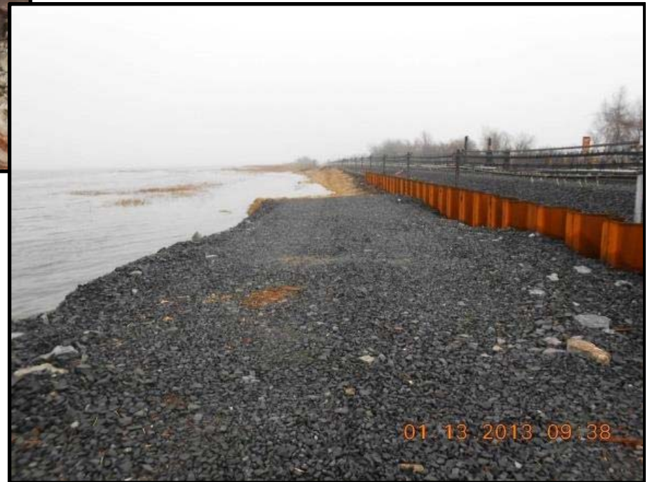
Washout and Damage to earth embankment exposed old LIRR infrastructure
