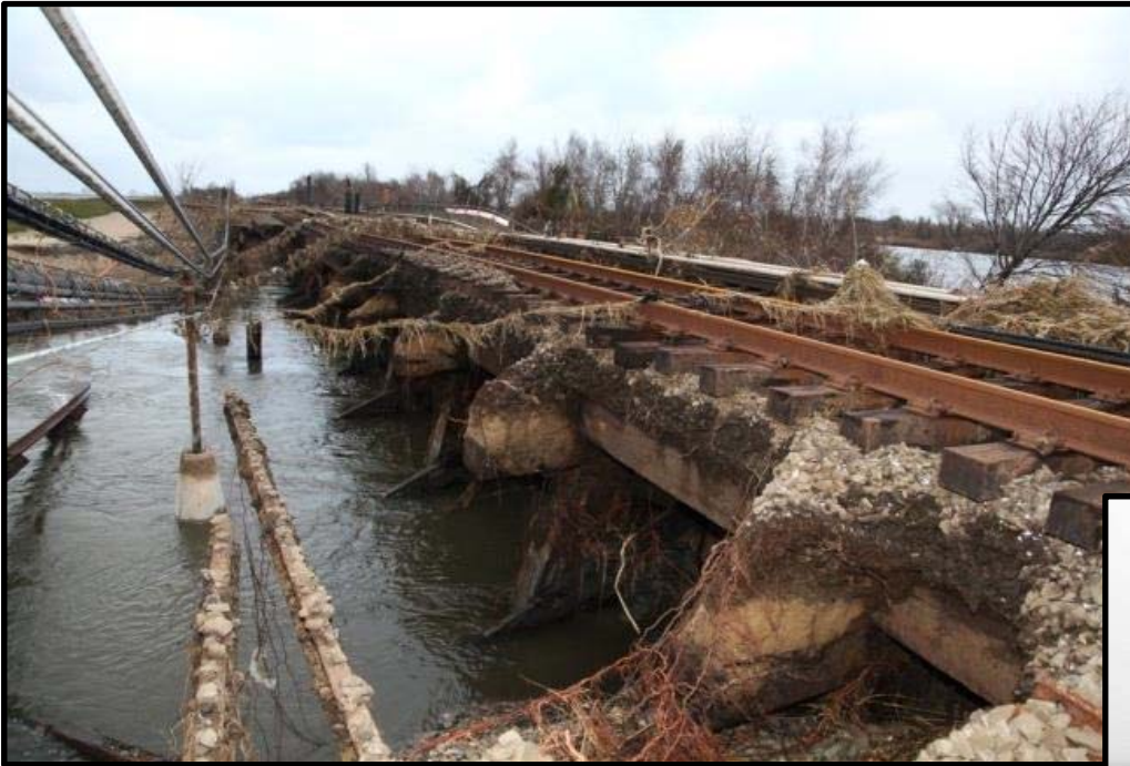
Washout and Damage to earth embankment exposed old LIRR infrastructure
