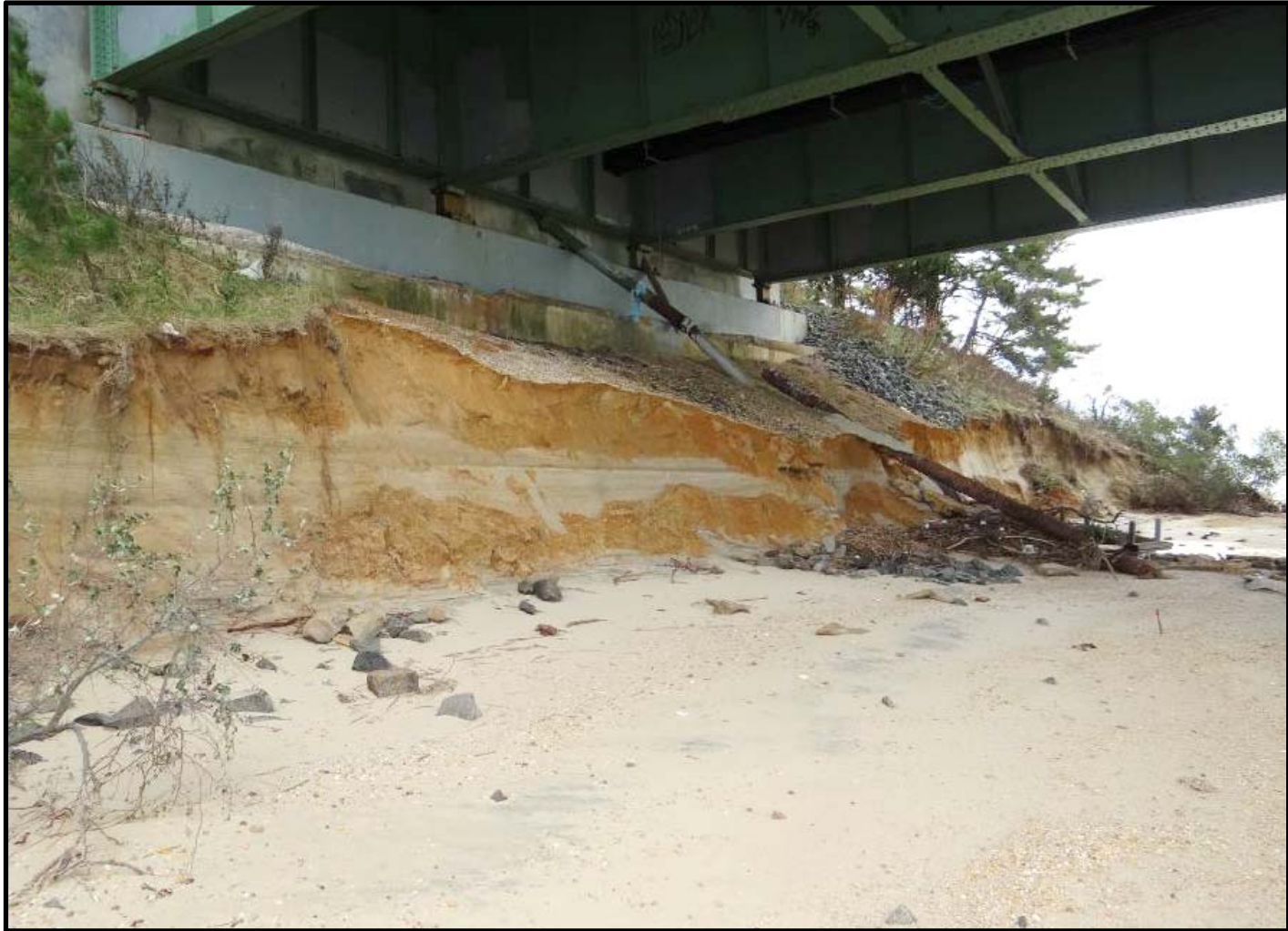
Severe erosion observed at Rt. 72 east abutment, looking south-east (NJDOT 2012a)
